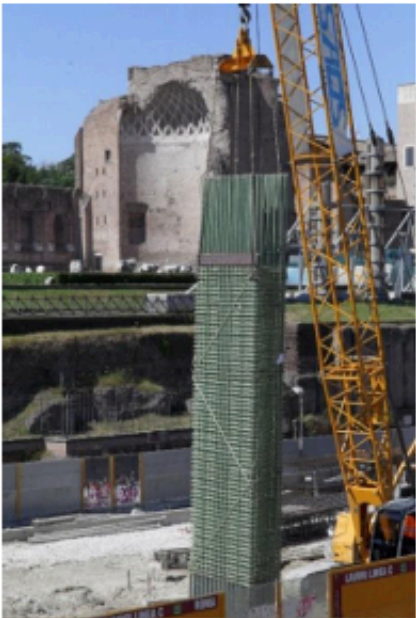
Figure 19. Installation of a GFRP cage
