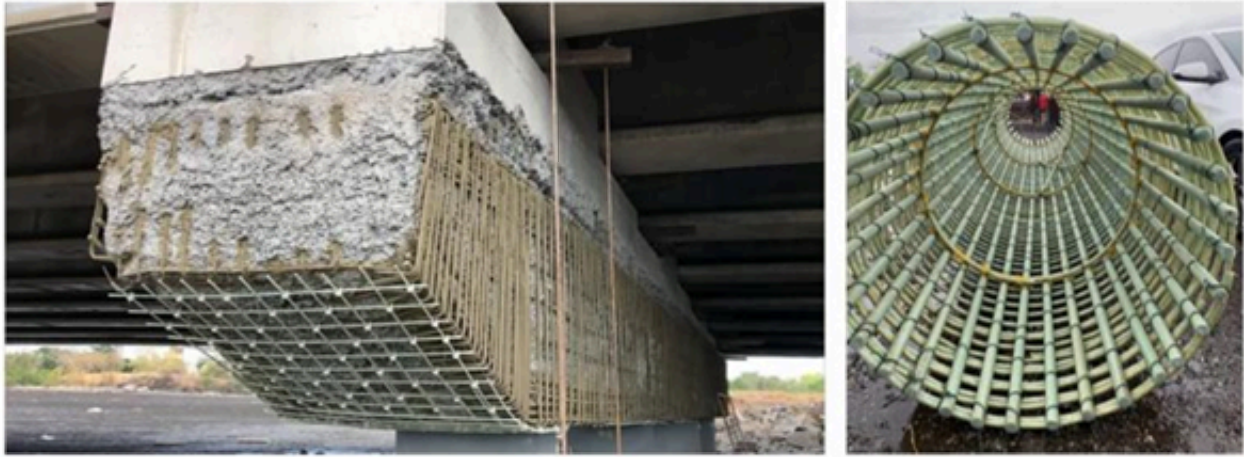
Figure 21. Pier cap retrofitting (left) and pier cage GFRP reinforcement (right) [40]
