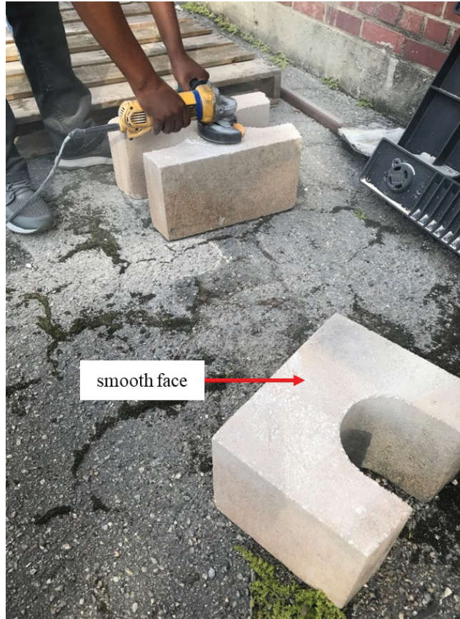
Figure 3-25. Grinding the lug off the tops of the Vertica Straight Face blocks.
