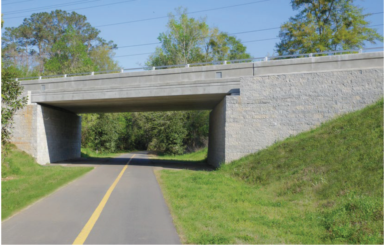
Figure 2-8. Orange Avenue Bridge in Tallahassee, Florida. ( https://ncma.org/updates/projects/florida-manages-orange-avenue-bridge-with-grs-ibs/ ).
