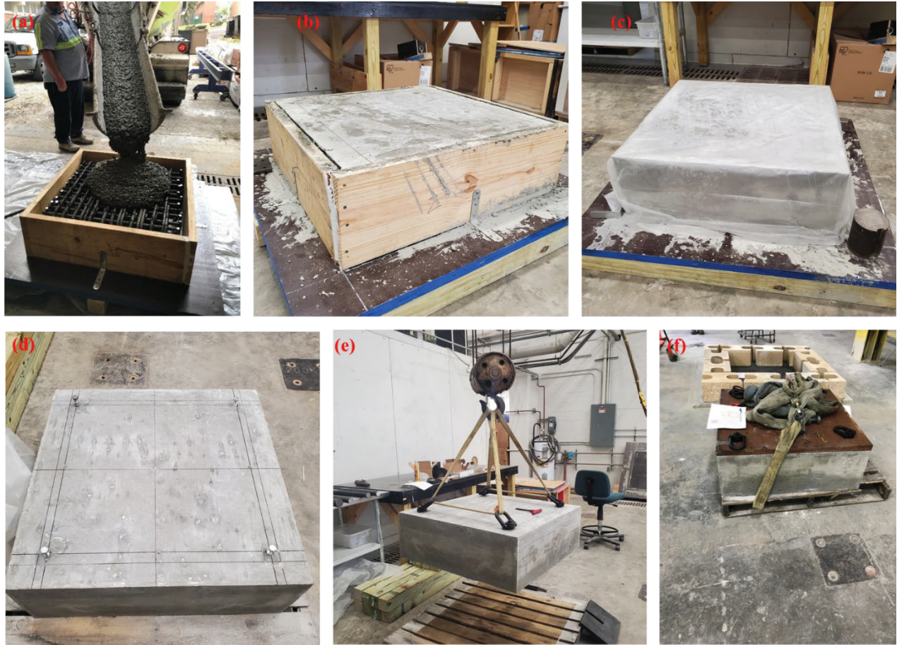
Figure 3-26. Casting of a concrete footing.
