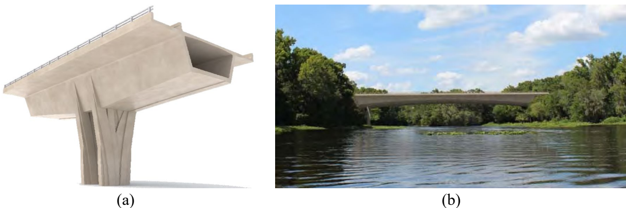
Figure 3.22: Wekiva River Bridge: (a) fixed pier table; (b) bridge elevation [52]
