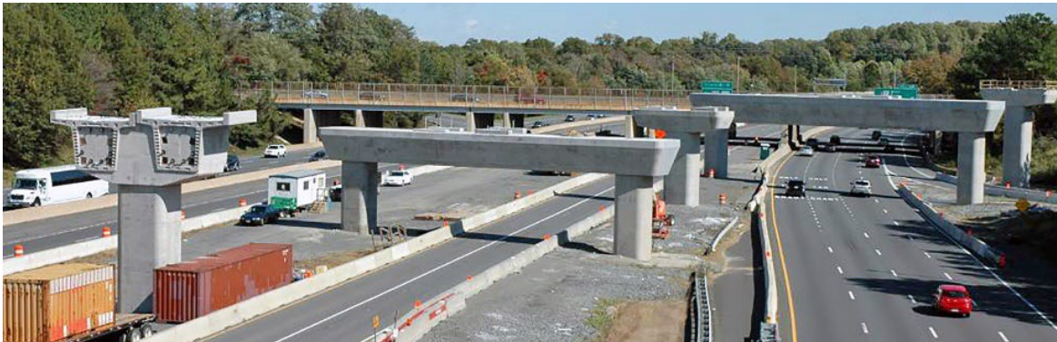
Figure 3.44: Straddle bent (courtesy of Corven Engineering).
