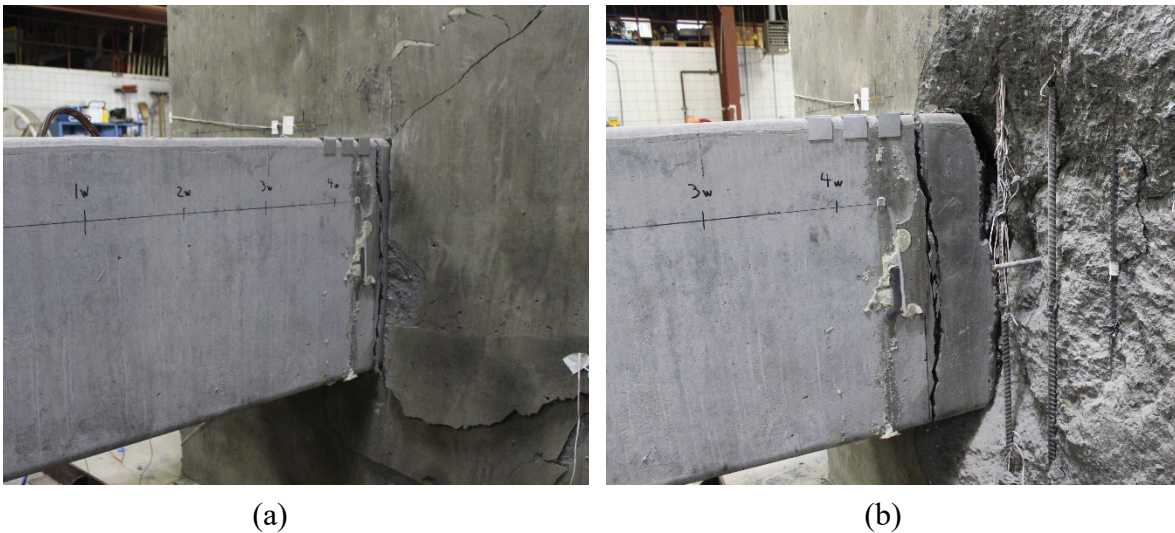
Figure 5.52: SP-09 strand development failure: (a) SP-09 failure; (b) after removing spalled concrete in the cap.
