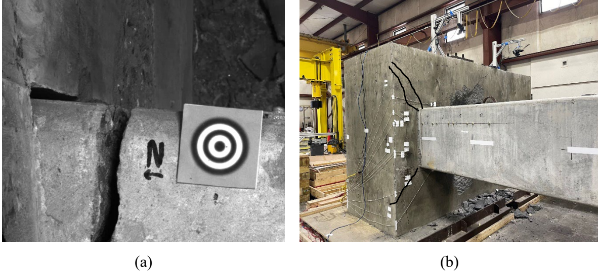
Figure 5.53: SP-09 failure: (a) pile slipping out of pile cap; (b) damage in pile cap.
