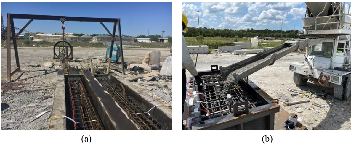
Figure 5.32: 18-inch specimen construction: (a) pile casting; (b) pile cap casting.
