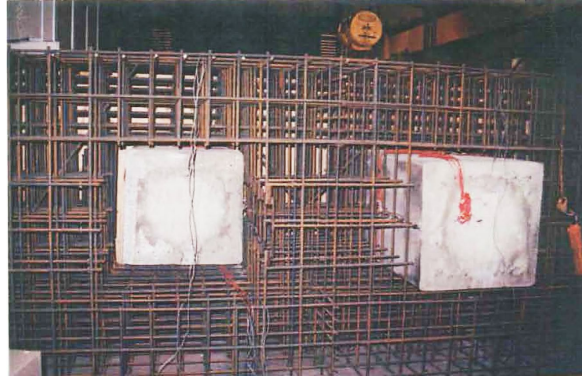
Figure 5.9: Photograph of pile cap reinforcement used by Issa [2].
