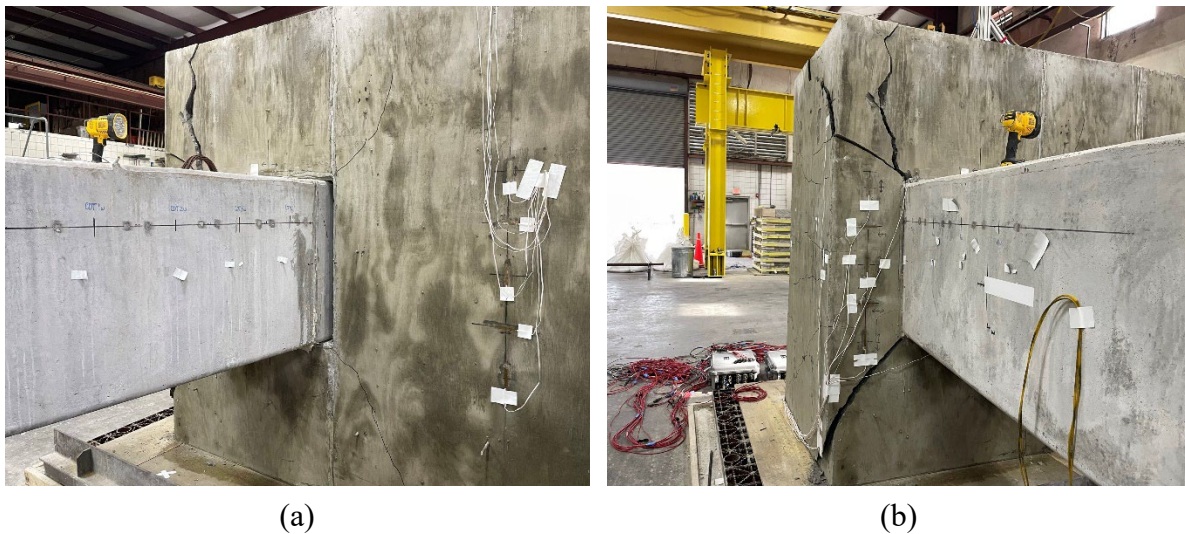
Figure 5.54: SP-10 failure: (a) pile slipping out of pile cap; (b) punching shear failure.
