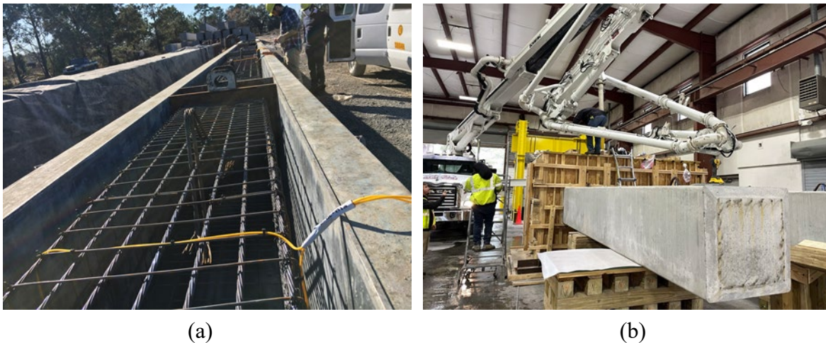
Figure 5.33: Construction of the 30-inch specimens: (a) pile casting at CDS; (b) pile cap casting at FDOT SRC.
