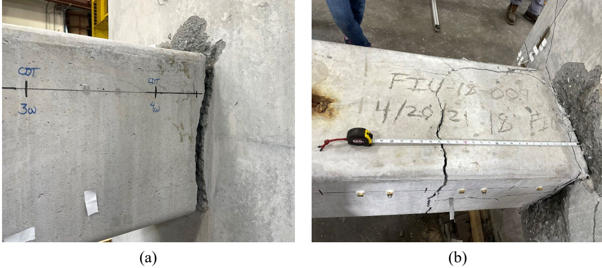
Figure 5.51: Photographs after failure for: (a) SP-04; (b) SP-03 with observed strand development failure.
