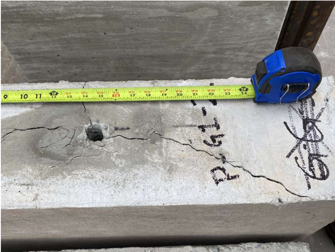
Figure A-32: P-G1-2 specimen concrete after anchor breakout
