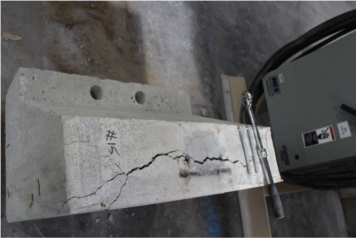
Figure A-120: G-G-38 specimen concrete after breakout
