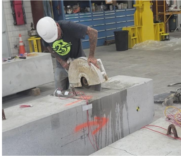
Figure 4.39: Pile cutting process
