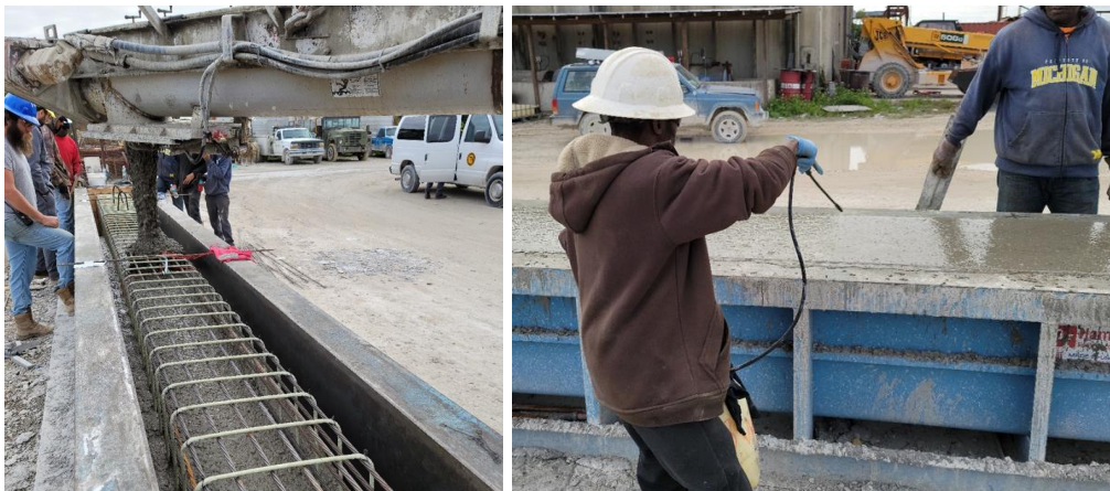
Figure 4.8: Pile casting
