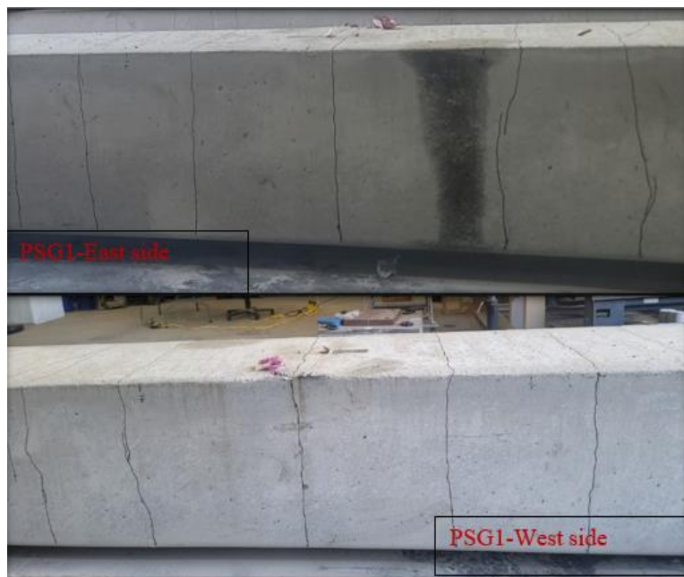
Figure 4.36: Crack pattern after final impact for PSG1
