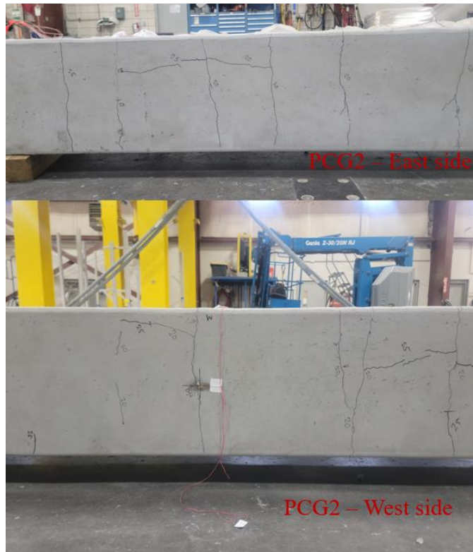
Figure 6.42: Crack pattern after final impact for PCG2
