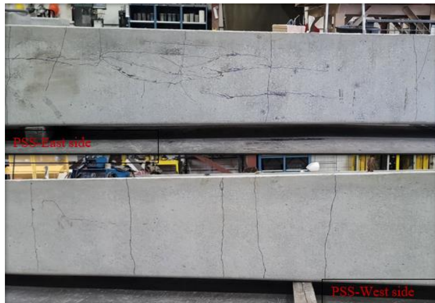
Figure 4.34: Crack pattern after final impact for PSS
