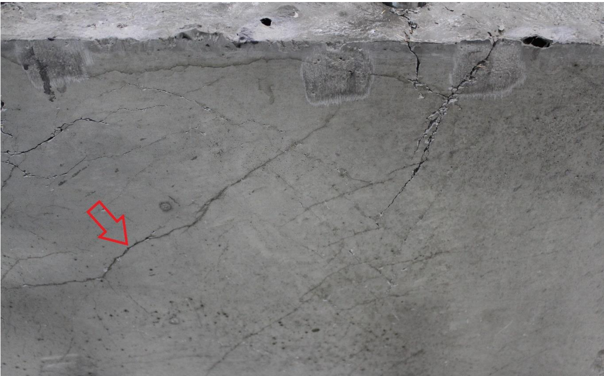
Figure 21: Cracking in Slab 2, Row 3 after testing
