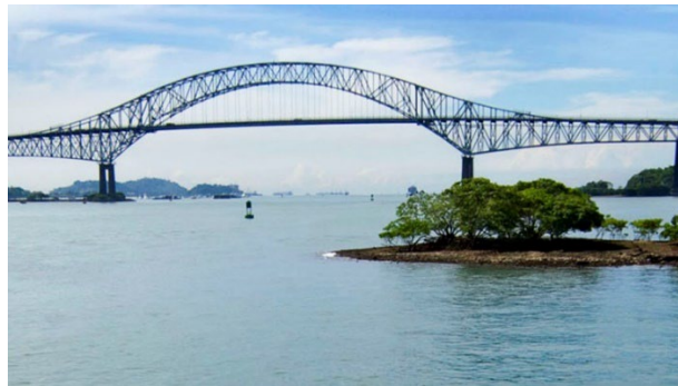
Figure 2.9 The Bridge of the Americas stands on artificial islands made to protect the piers from ships transiting the Panama Canal (Wikipedia)
