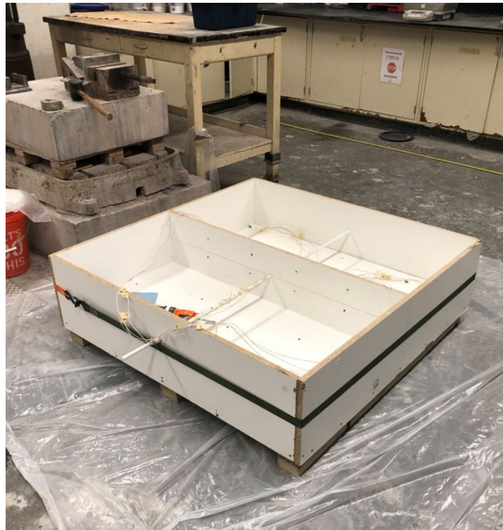
Figure 51: Formwork for slabs construction
