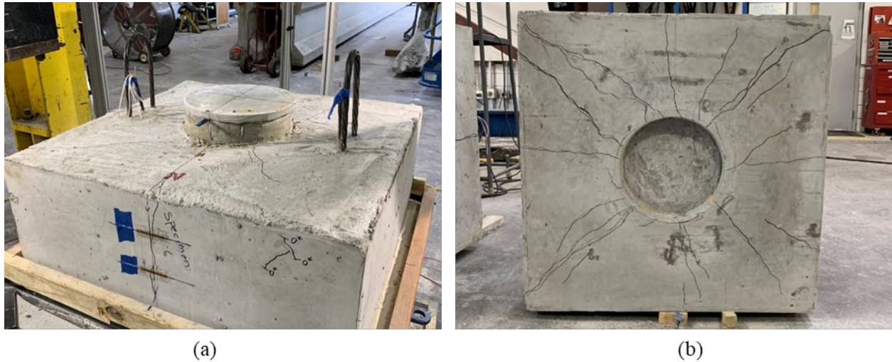
Figure A.59: Cracking on (a) cap and (b) bottom of the Specimen S2-6
