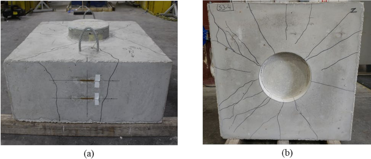
Figure A.163: Cracking on (a) cap and (b) bottom of Specimen S3-4
