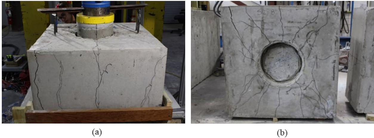
Figure A.73: Cracking on (a) cap and (b) bottom of Specimen S2-8
