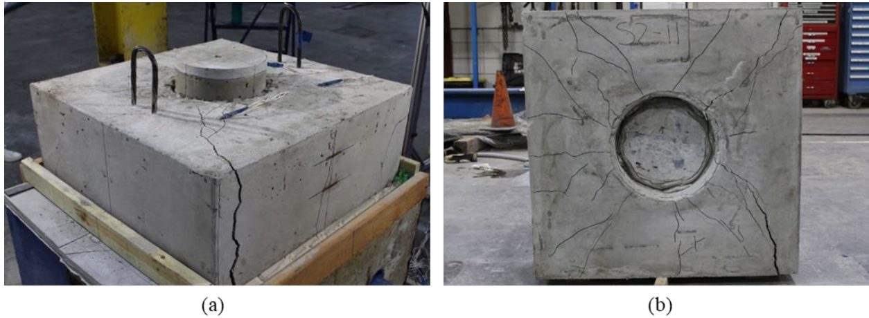
Figure A.95: Cracking on (a) cap and (b) bottom of Specimen S2-11
