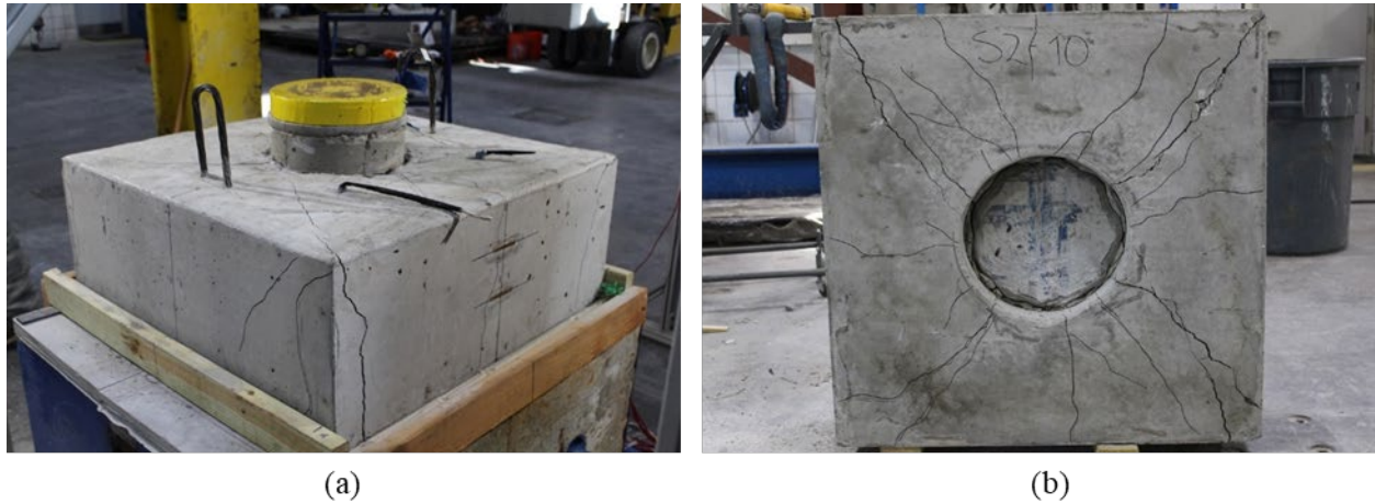
Figure A.88: Cracking on (a) cap and (b) bottom of Specimen S2-10
