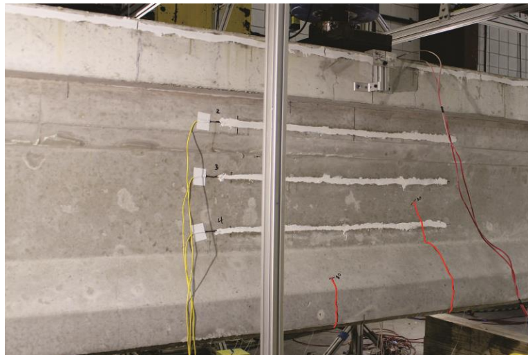
Figure 8.44 Specimen SS-4: First observed cracks (marked in red) at P = 80 kip
