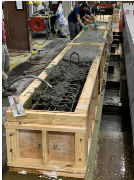
Figure 6.3 Concrete placement: CIP beam specimen SS-5
