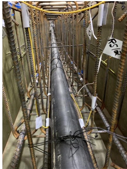
Figure 6.2 Rebar cage and HDPE duct installation for CIP beam specimen SS-5
