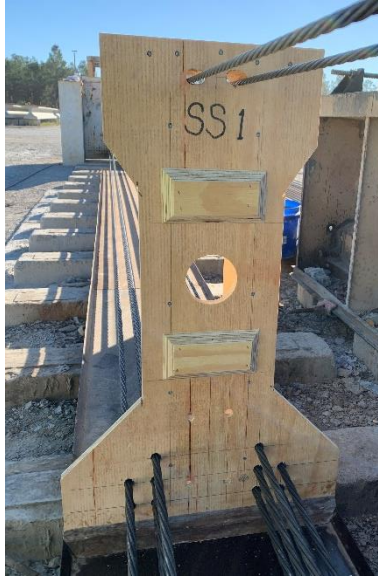
Figure 5.2 Custom plywood bulkheads for SS precast beams
