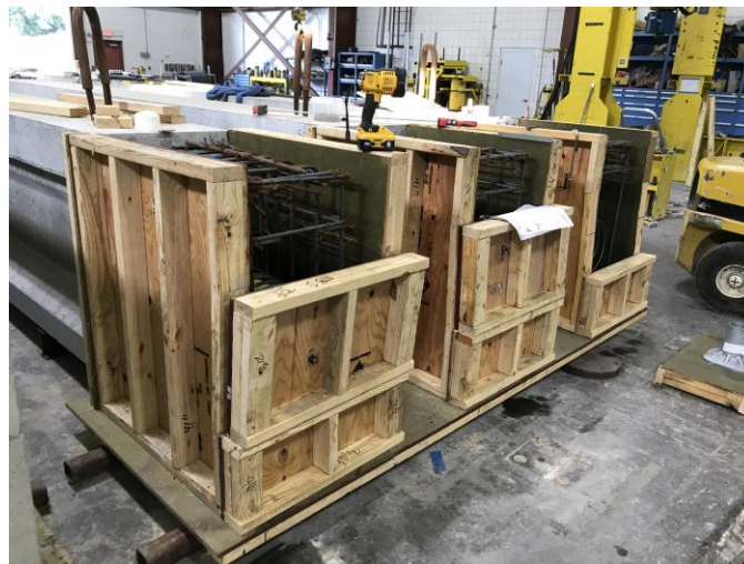
Figure 5.20 Installation of formwork for fabrication of end blocks for precast SS specimens
