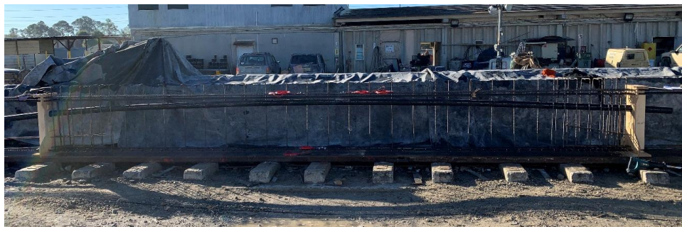
Figure 7.6 Rebar cage and HDPE duct installation for NB precast beams (before the ducts were tied for final configuration of tendon profile)
