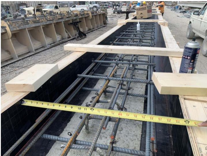
Figure 5.13 Mild steel reinforcement for concrete deck
