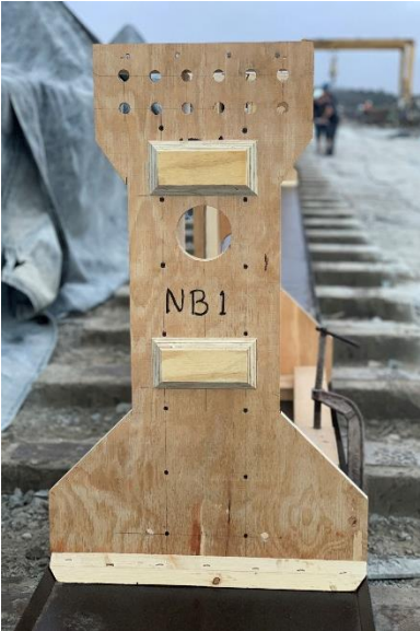
Figure 7.2 Custom plywood bulkheads for NB precast beams
