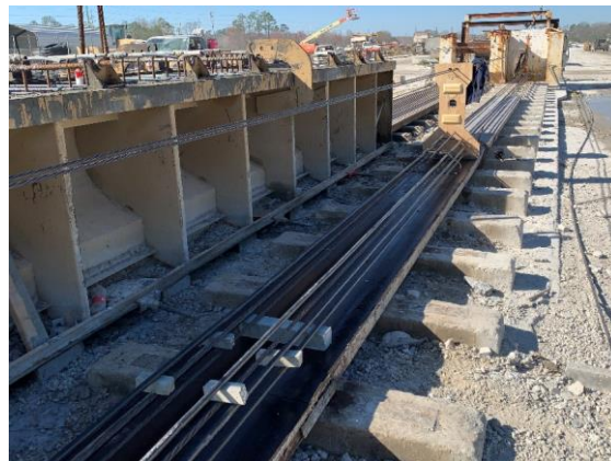
Figure 5.4 Pre-fabricated concrete pieces used to provide separation for prestressing strands
