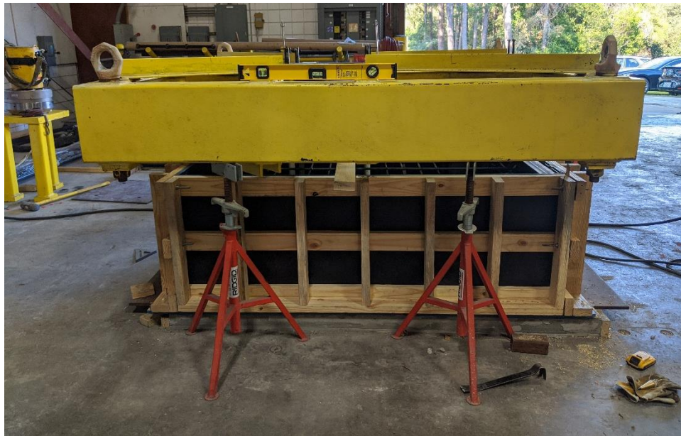
Figure 4.16 Steel hanger frame and concrete formwork ready for concrete placement
