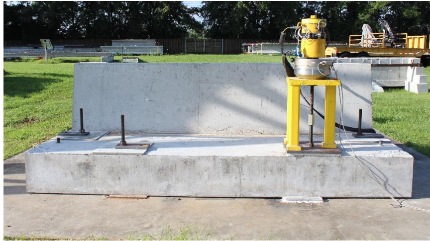
Figure 5.17 Post-tensioning fourth (front right) threaded bar for anchoring test specimen to pendulum foundation with the FDOT loading assembly
