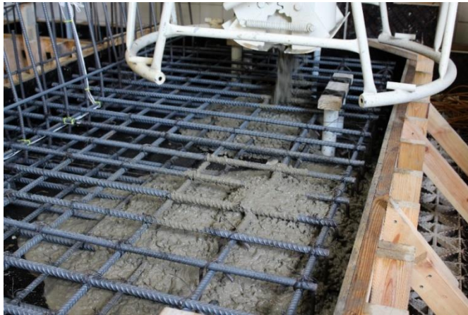
Figure 5.8 Deck concrete placement
