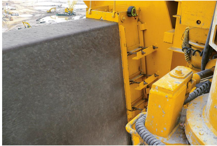
Figure 2.8 Retained railing shape after slip-forming (Photo credit: Gomaco)
