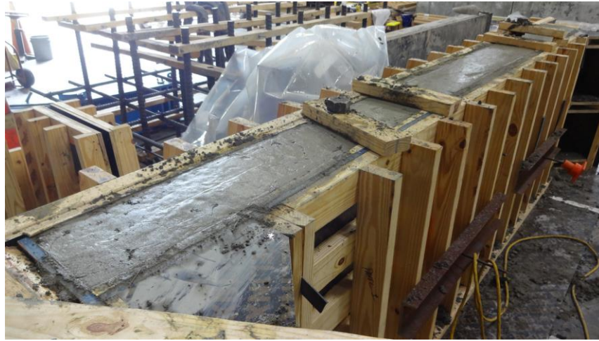
Figure 3.24 Filled FRC railing formwork after trial FRC production
