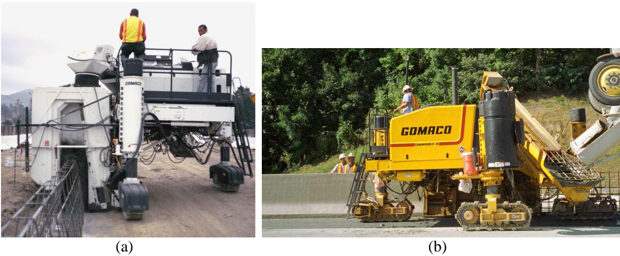
Figure 1.2 Slip-formed construction of conventionally rebar-reinforced traffic railings (Photo Credit: Gomaco)
