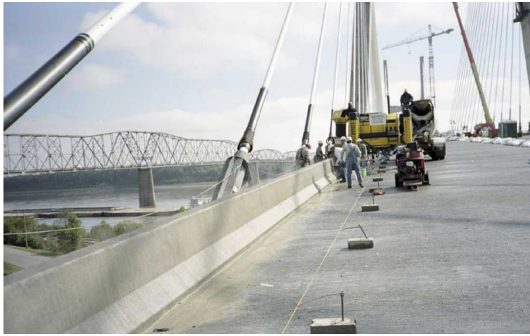
Figure 1.1 Slip-formed concrete traffic railing (Photo credit: Gomaco)
