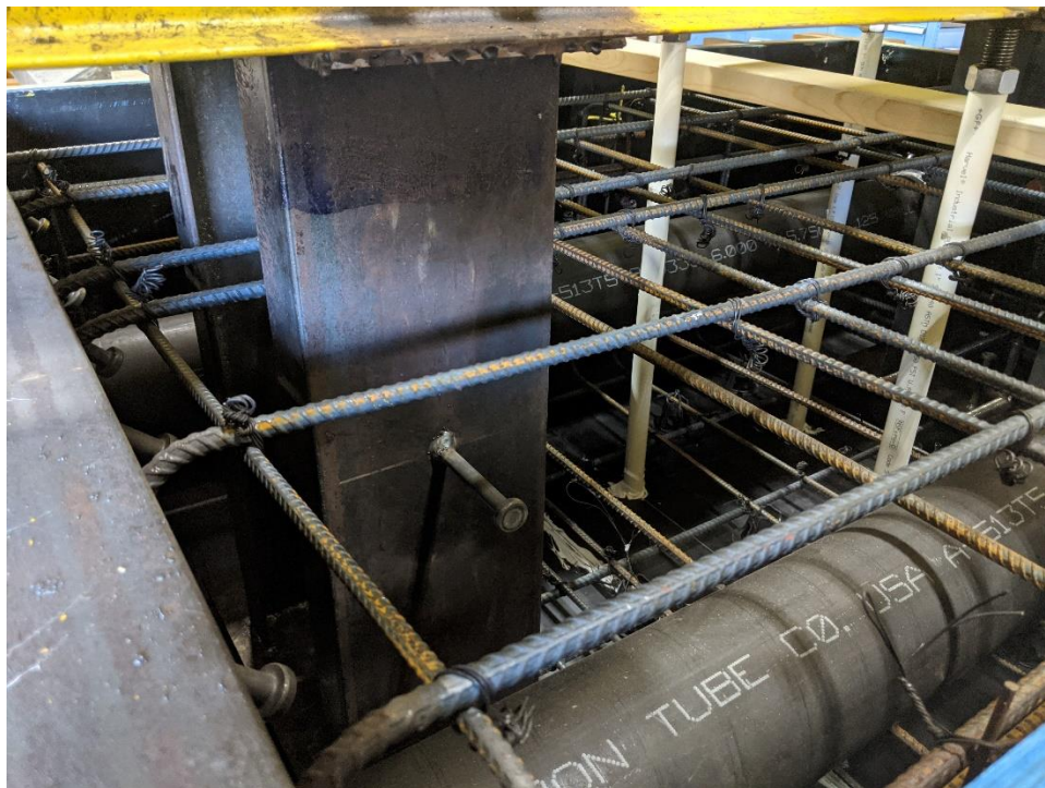
Figure 4.14 Embedded steel components within the concrete block formwork
