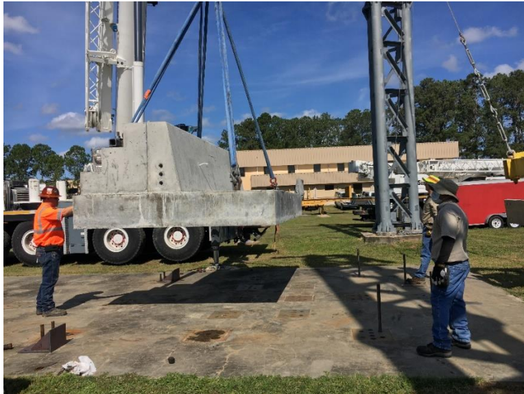
Figure 5.13 Test specimen being moved into position on the pendulum foundation
