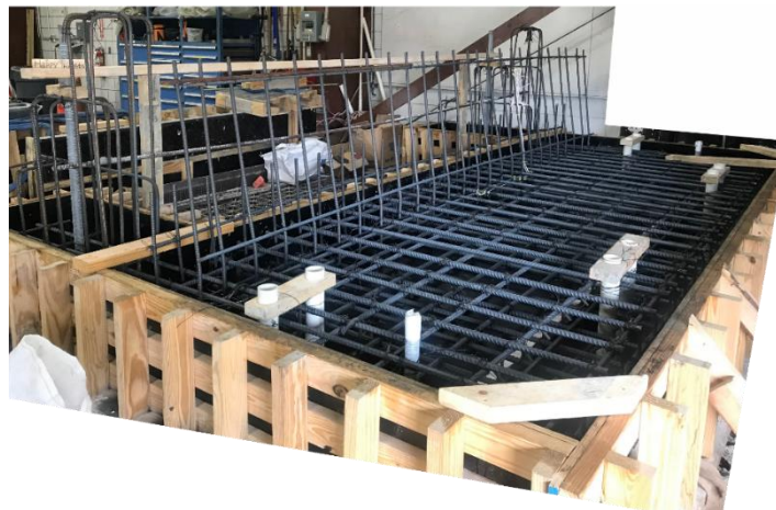
Figure 5.6 Reinforcing bars positioned inside deck formwork
