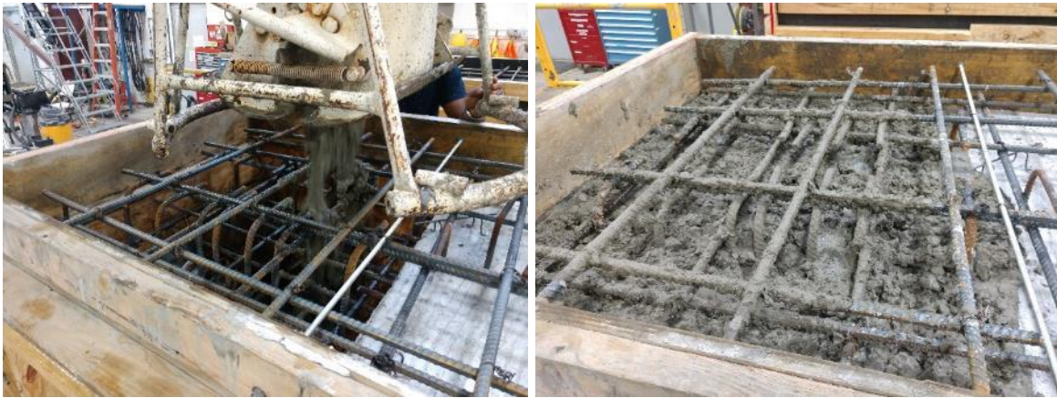
Figure 5-34 End block concrete placement
