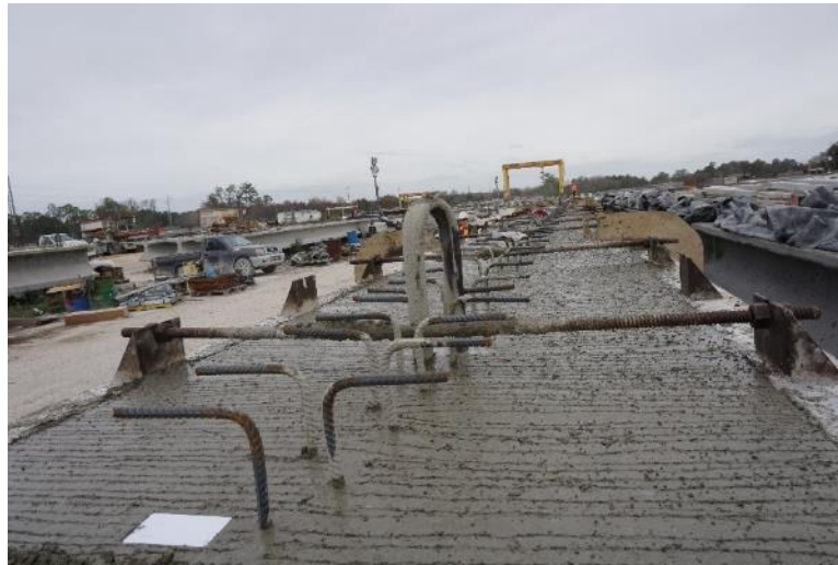
Figure 5-27 Roughened top surface
