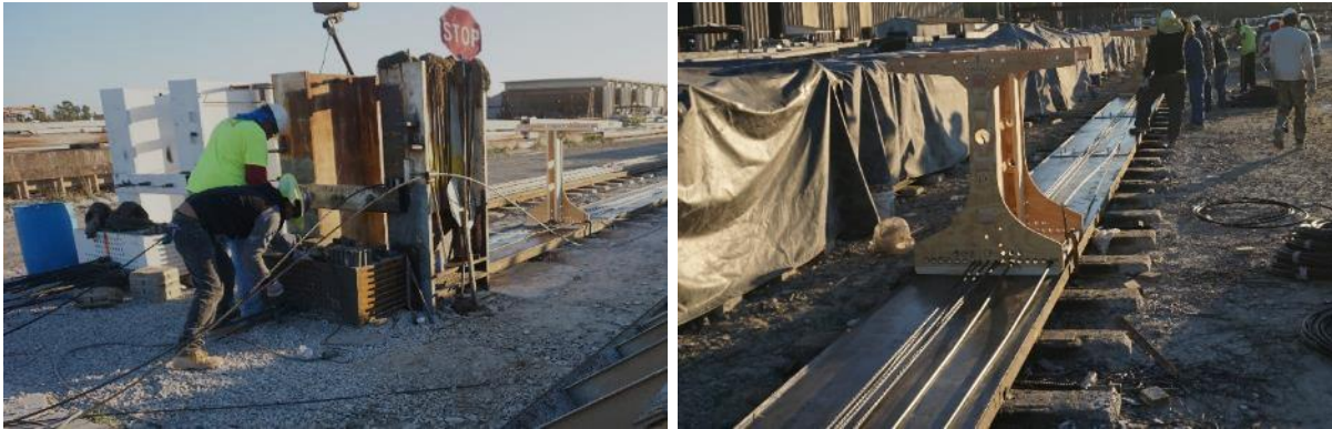
Figure 5-10 Prestressing strand insertion
