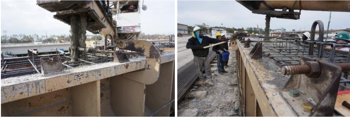
Figure 5-26 Concrete placement at girder bed for specimens
