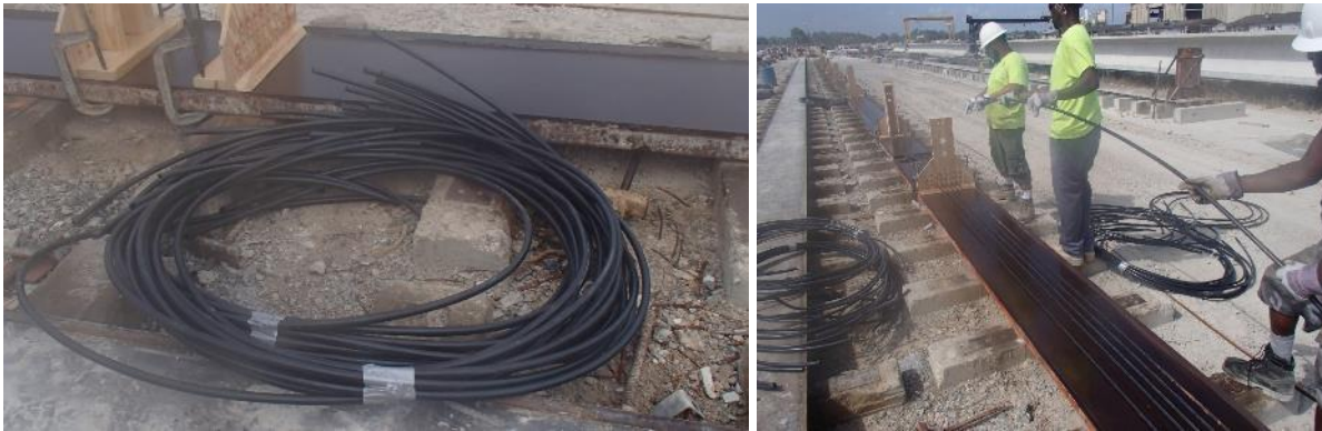
Figure 4-8 PVC sheathing for strand debonding.
