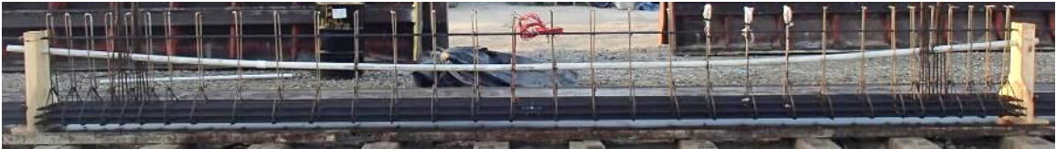
Figure 4-17 SS2 rebar cage assembly
