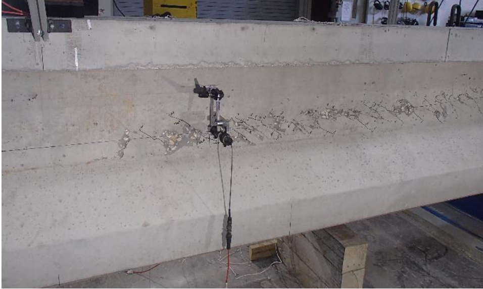
Figure 4-56 Concrete spalling at web
