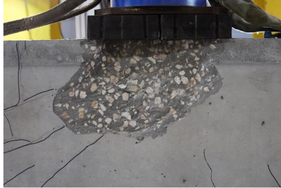
Figure 4-40 Concrete spalling under load point at peak load
