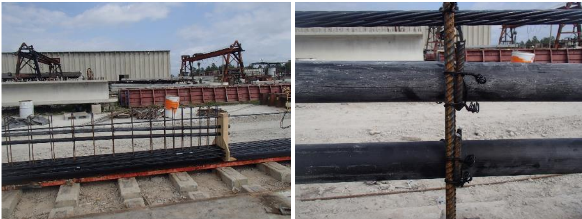
Figure 4-14 Rebar cage assembly
