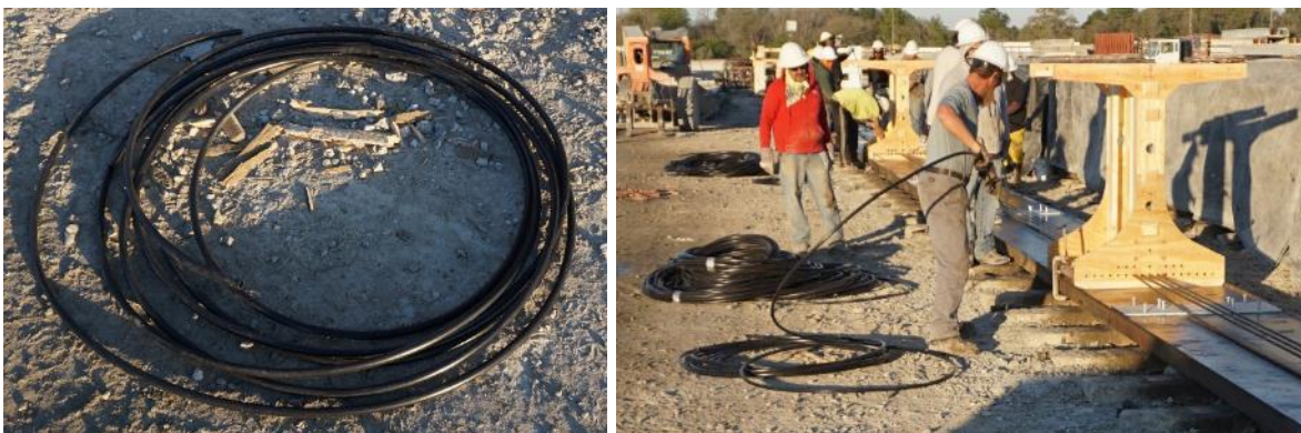
Figure 5-11 PVC Sheathing for strand debonding
