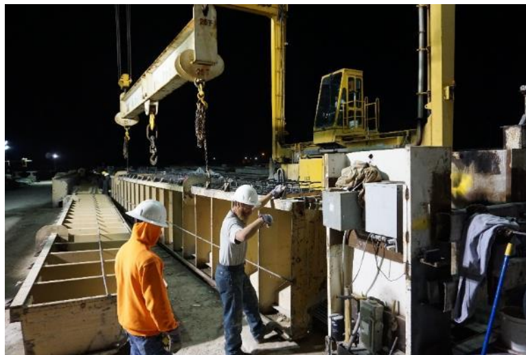
Figure 5-25 FIB-54 side form installation.
