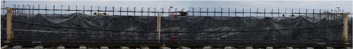
Figure 5-19 P34 rebar cage assembly.
