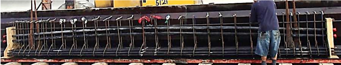
Figure 4-21 NB1 rebar cage assembly
