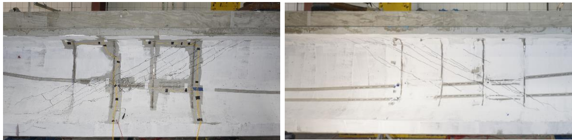
Figure 5-58 Specimen P34 crack pattern for test (a) P34-1 (b) P34-2
