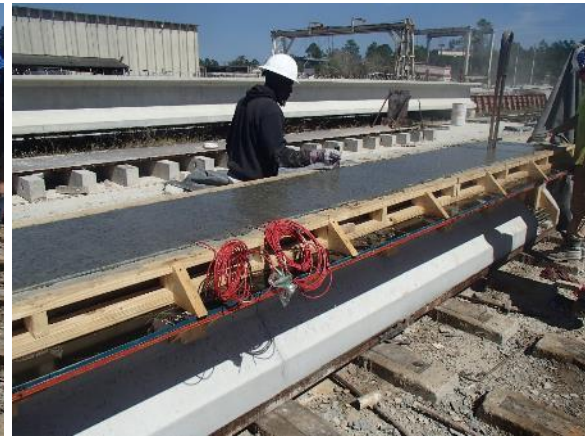
Figure 4-28 Concrete placement and finished surface
