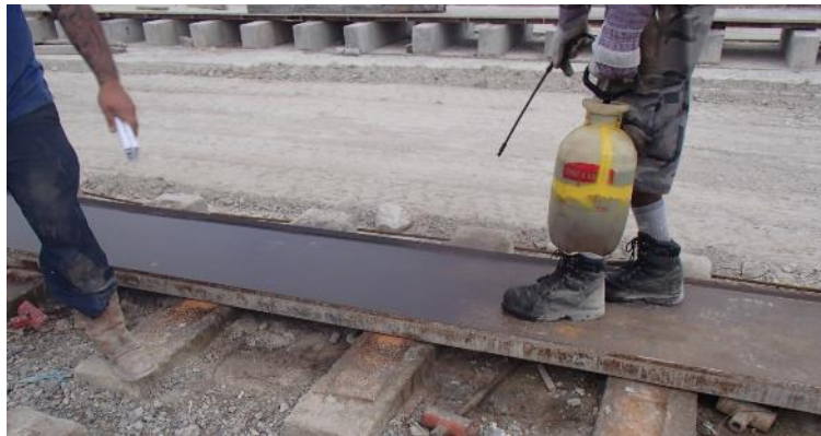
Figure 4-5 Form release being sprayed on bottom liner
