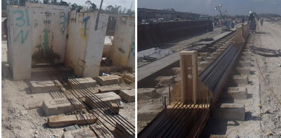
Figure 4-7 Prestressing strand insertion.
