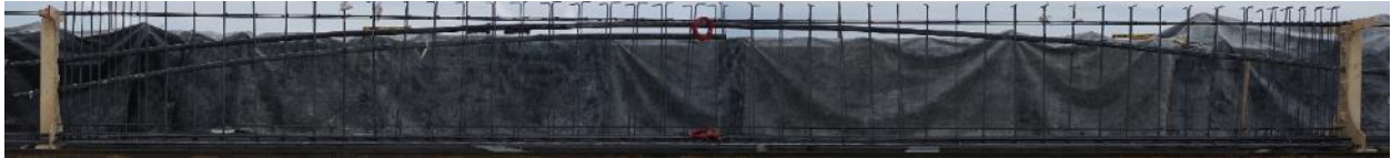
Figure 5-23 N34 rebar cage assembly.
