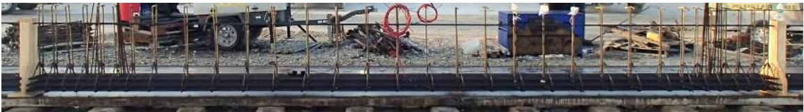
Figure 4-19 SS4 rebar cage assembly
