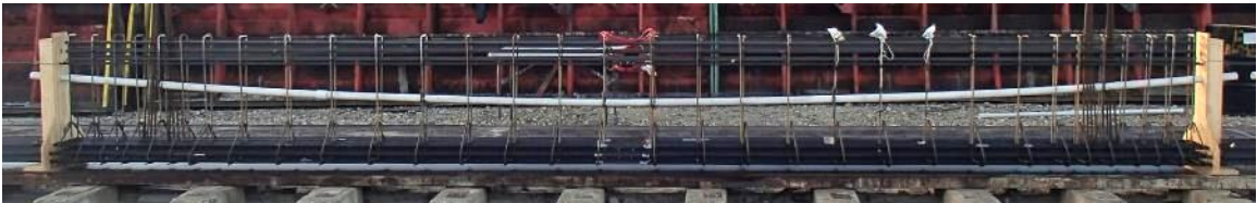
Figure 4-16 SS1 rebar cage assembly
