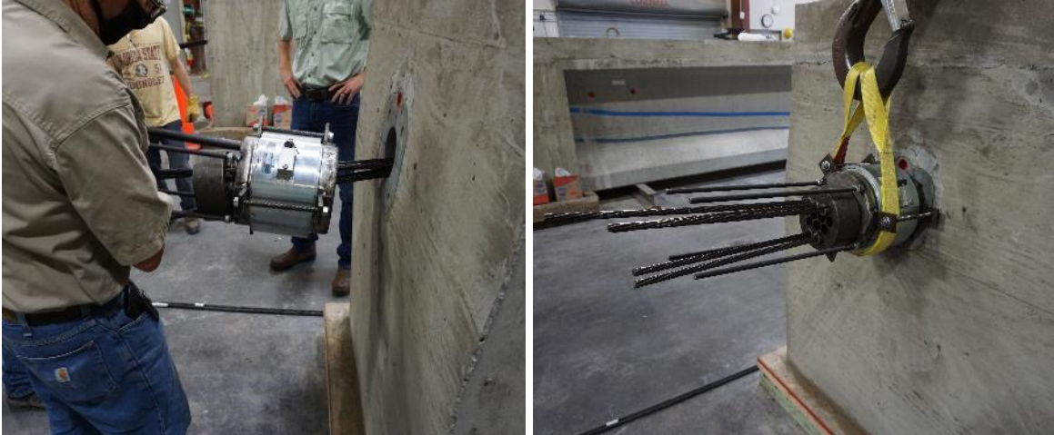
Figure 5-43 Geokon 850-kip hollow load cell and anchor head installation at dead-end
