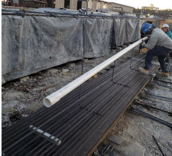
Figure 5-15 Duct installation.
