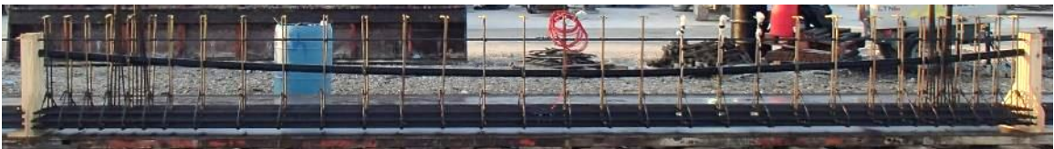
Figure 4-18 SS3 rebar cage assembly
