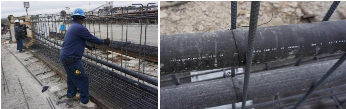
Figure 5-16 Rebar cage assembly.
