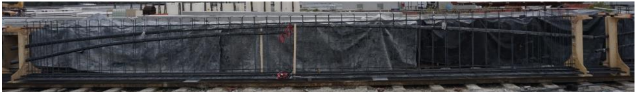
Figure 5-24 N50 rebar cage assembly.
