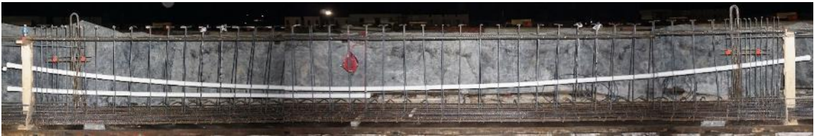
Figure 5-20 P41 rebar cage assembly.
