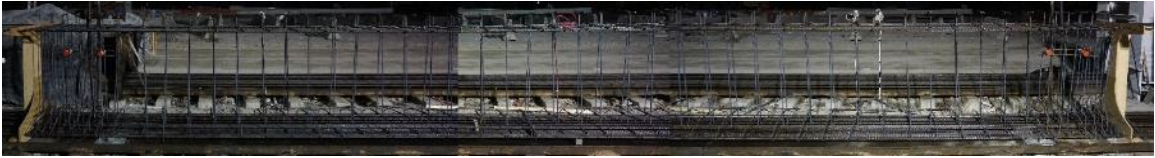
Figure 5-18 P00 rebar cage assembly.
