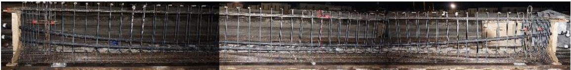
Figure 5-21 P50 rebar cage assembly.
