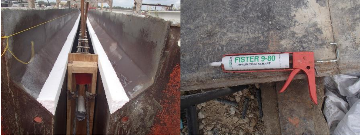
Figure 4-23 Styrofoam attached to side form and glue
