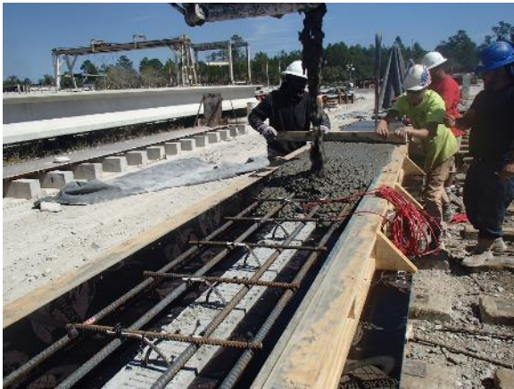
Figure 4-28 Concrete placement and finished surface
