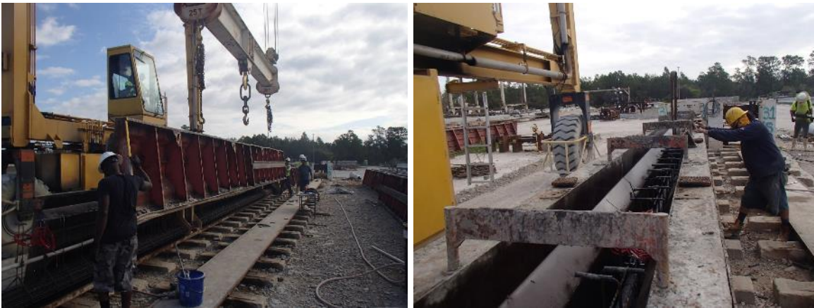
Figure 4-22 AASHTO Type III side form installation
