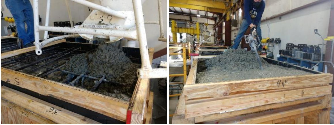
Figure 5-35 Deck concrete placement
