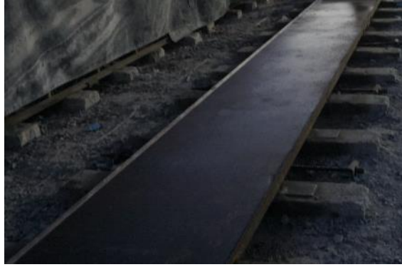
Figure 5-7 FIB 54 steel bottom liner
