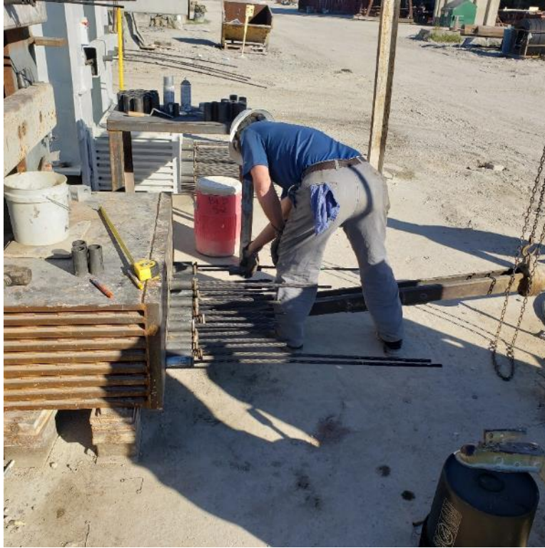
Figure 5-12 Prestressing strand stressing using monostrand jack
