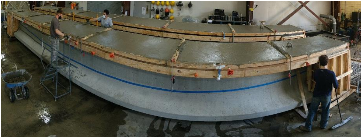
Figure 5-36 Completed concrete placement
