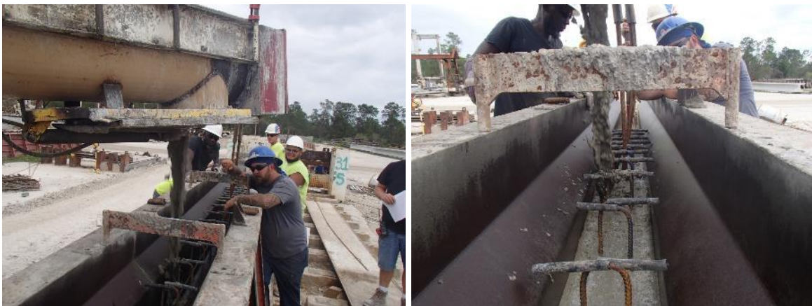
Figure 4-24 First concrete placement
