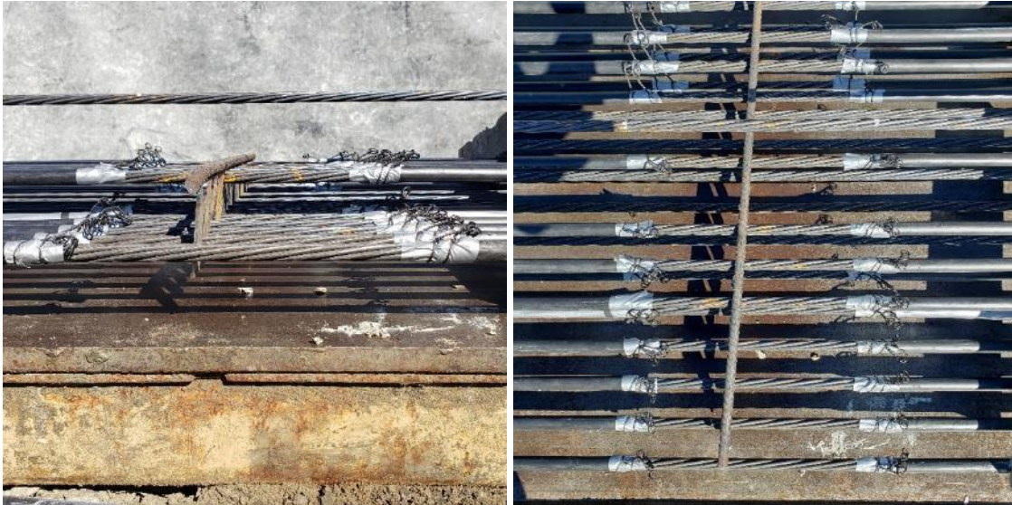
Figure 5-14 Strand debonding.
