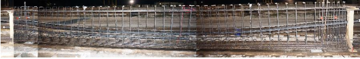
Figure 5-22 P50R rebar cage assembly.
