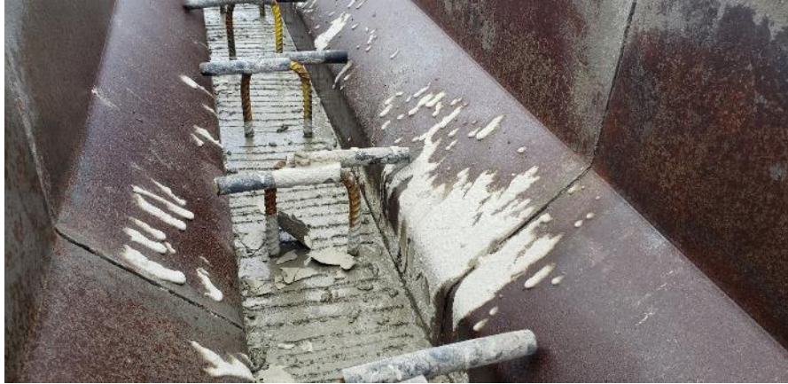
Figure 4-25 Roughened top surface
