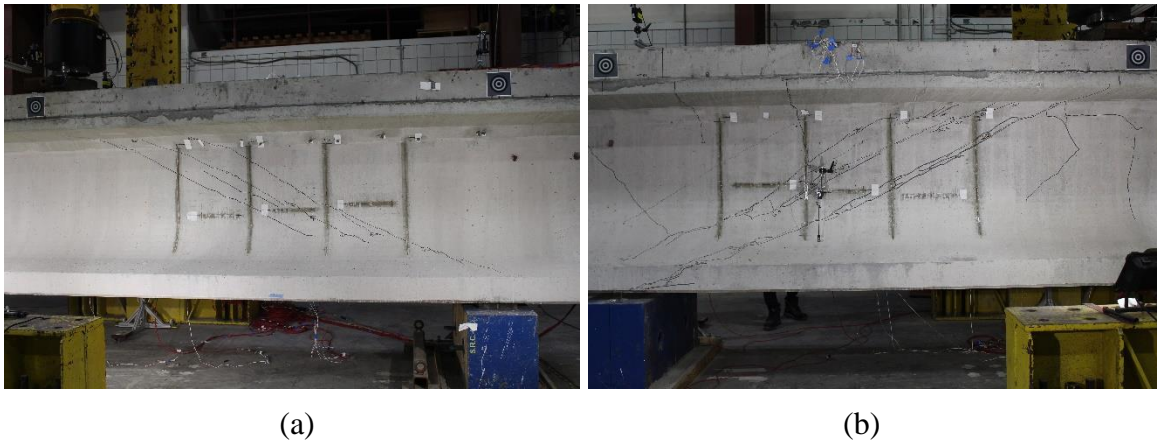
Figure 5-56 Concrete spalling at web after peak shear force and unloading (a) P00-1 (b) P00-2.
