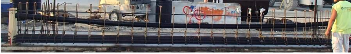
Figure 4-20 SS5 rebar cage assembly
