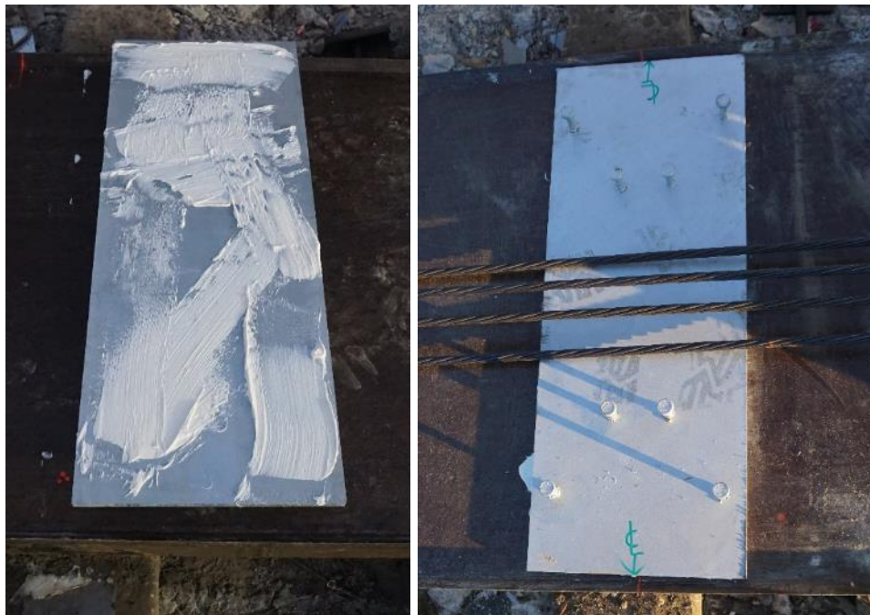
Figure 5-9 Embedded steel bearing plate
