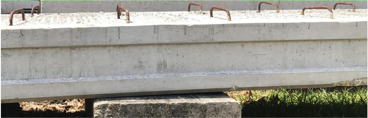
*Figure 11 Cracks Noted at the Support*
