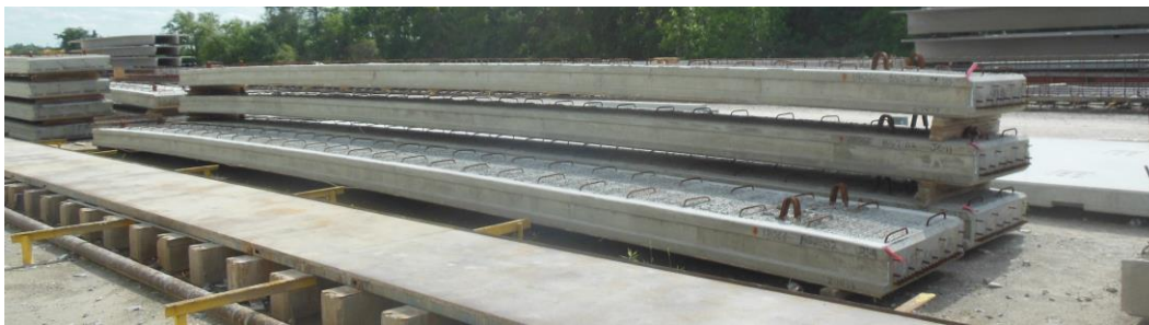
Figure 6 Slab Storage at the Precast Yard, Overall View
