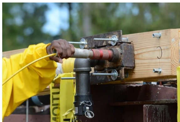
Figure A.4-5. Fitting for hydrodemolition used in trial 3
