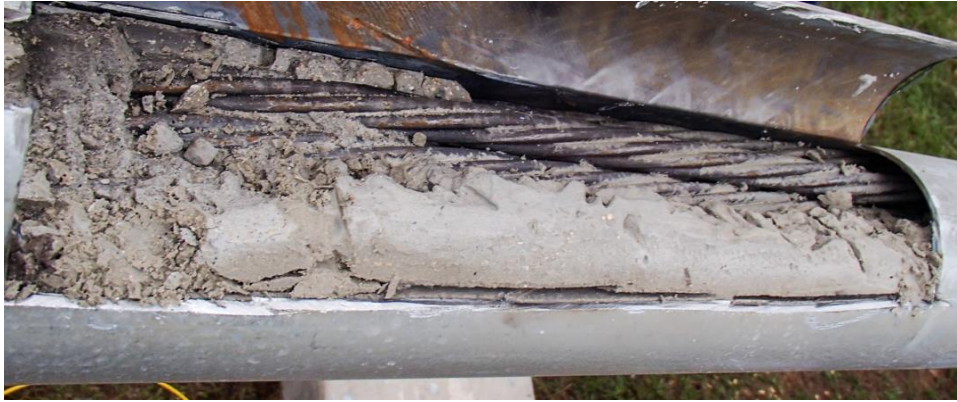
Figure A.4-8. Visual inspection of section 2 after water-blasting
