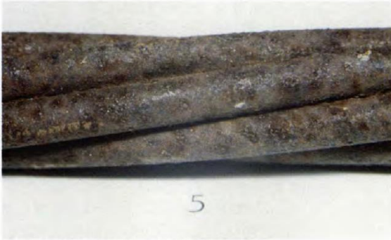
Photo 5. Strand surface before cleaning.
