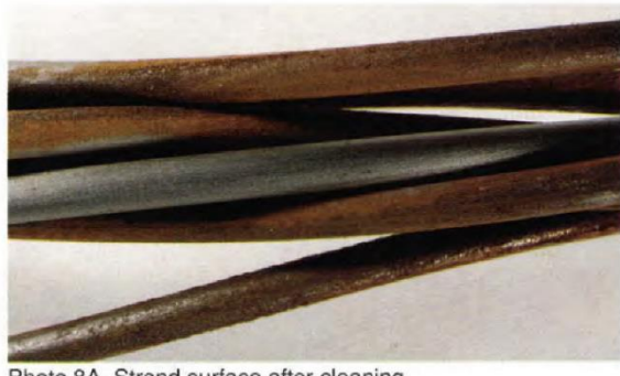
Photo 8A. Strand surface after cleaning.
