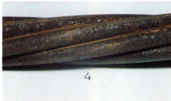
Photo 4. Strand surface before cleaning.
