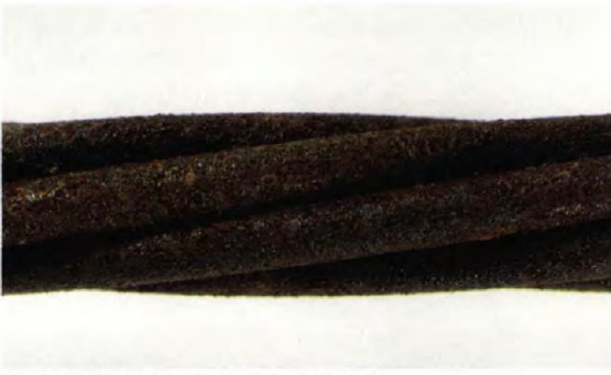
Photo 7. Strand surface before cleaning.
