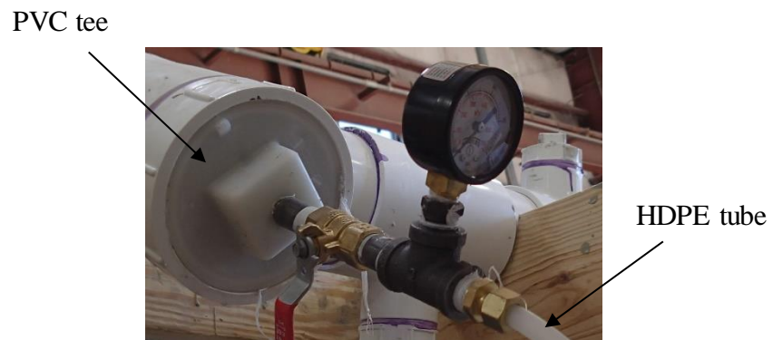
Figure 6-2. HDPE connection at PVC tee of inlet
