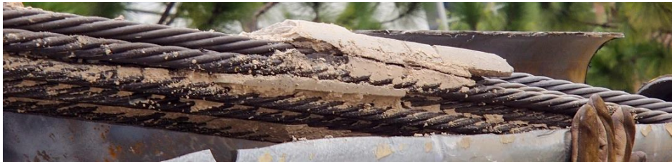
Figure A.4-12. Visual inspection of section 7 after water-blasting
