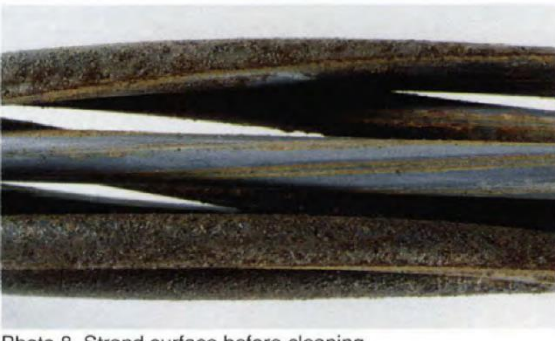
Photo 8. Strand surface before cleaning.
