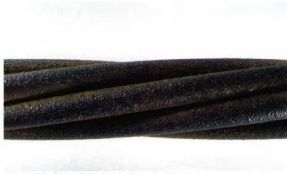
Photo 7A. Strand surface after cleaning.
