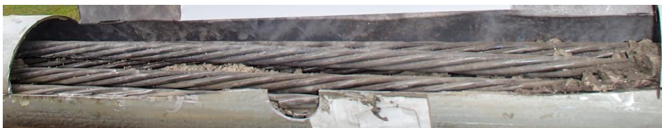
Figure A.4-10. Visual inspection of section 7 after water-blasting
