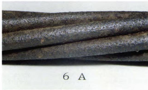
Photo 6A. Strand surface after cleaning.
