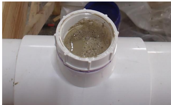
Figure 6-7. PVC tee through which grout was introduced
