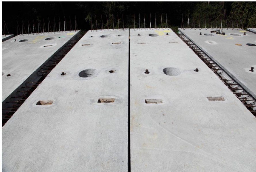
Figure 13: Precast prestressed concrete deck panels for LRWB (Roddenberry et al., 2019)
