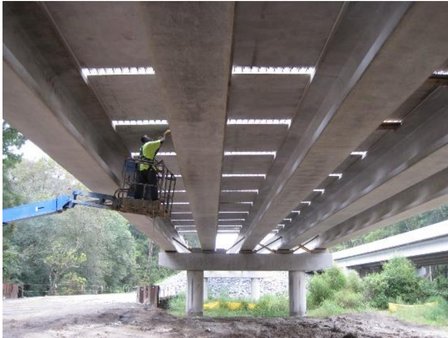
Figure 14: Precast Florida-I Beams and bridge decks
