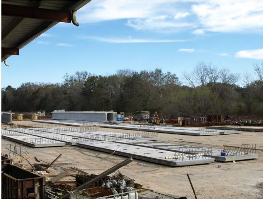
Figure 12: Non-prestressed precast concrete deck panels in casting yard (Roddenberry et al., 2019)
