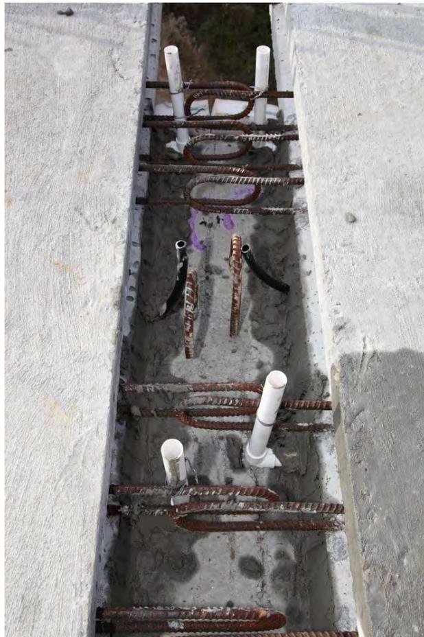
Fig. 4-20. Pipes for Grouting Shear Pockets on Little River WB
