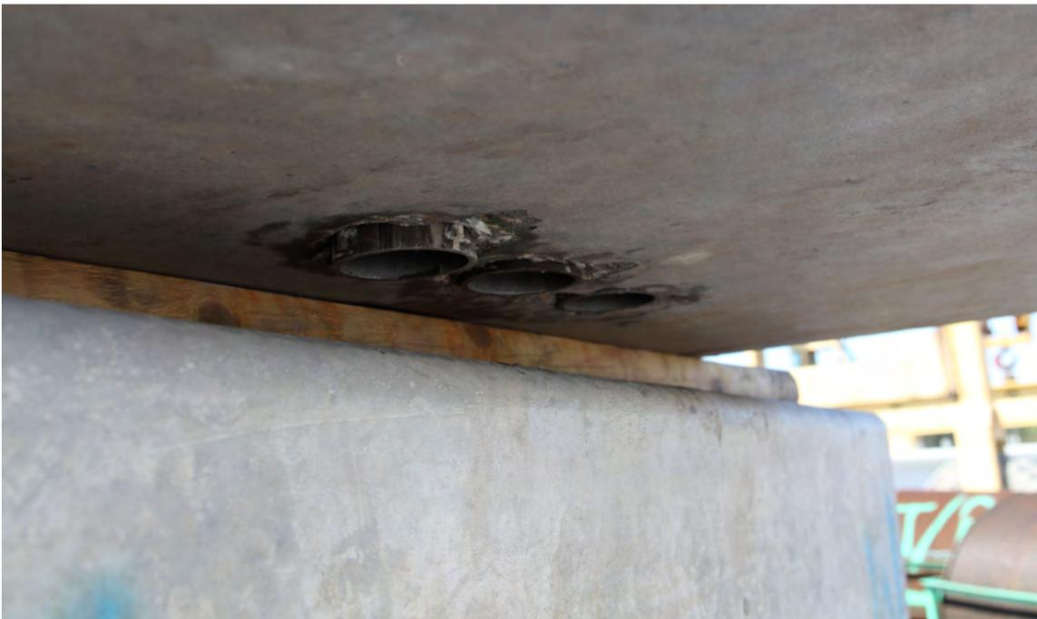
Fig. 6-15. Underside of Precast Bent Cap, Showing Pipes Protruding
