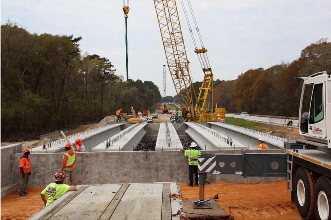
Fig. 3-8. Hurricane Creek EB – Looking West at Installed Girders (March 24, 2014)
