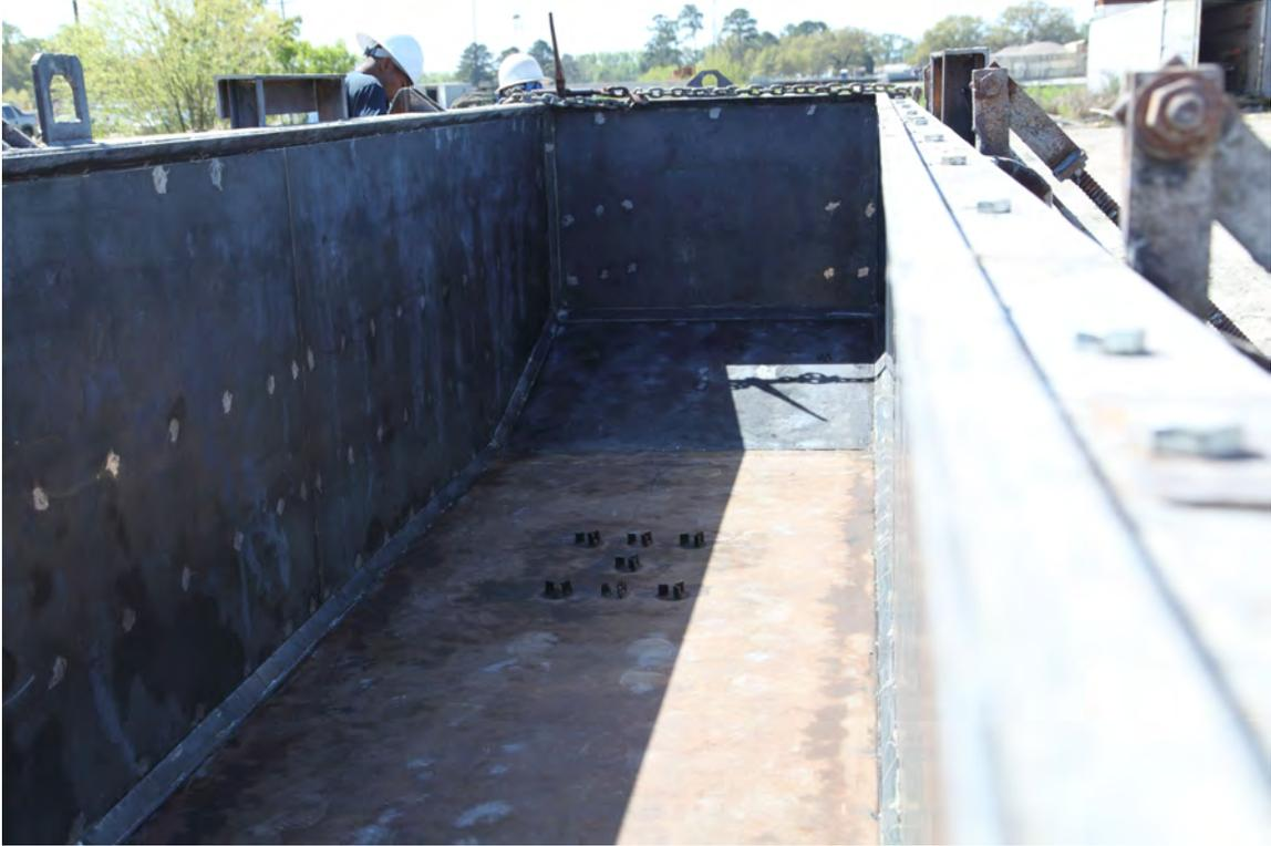
Fig. 6-12. Precast Bent Cap, End Taper in Background, and Template on Bottom to Position Pipe Forms for Dowel Bar Holes
