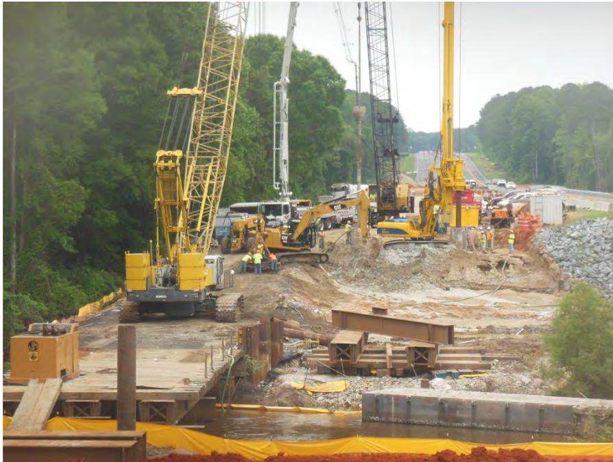
**Fig. 2-1. Drilled Shaft Construction**
