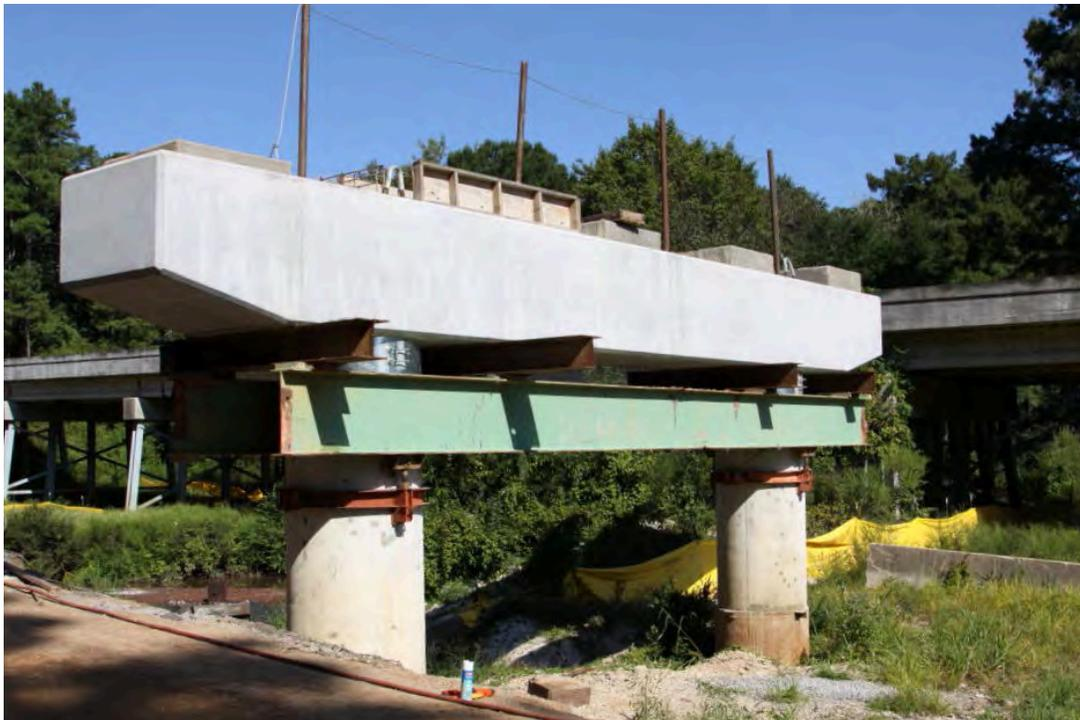
Fig. 2-29. Ready to Grout Bent Cap on Little River EB (September 11, 2014)
