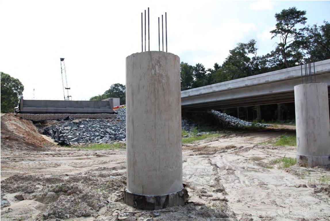
Fig. 2-15. Column and Six Dowel Bars Extending from Top on Little River WB (July 21, 2015)
