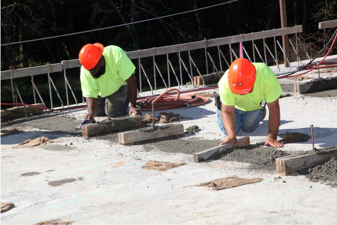
Fig. 4-44. Screeding Concrete on Closure Joint
