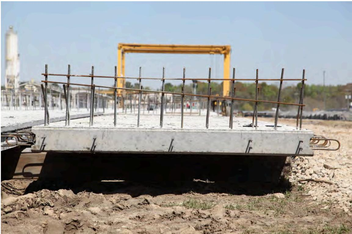
Fig. 5-13. Prestressed Precast Deck Panel, End View
