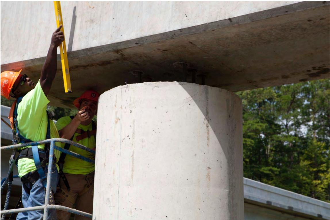
Fig. 2-24. Plumbing a Precast Bent Cap during Setting (July 24, 2015)
