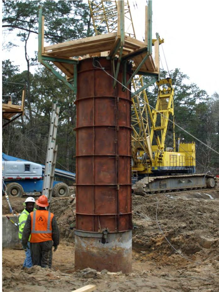
**Fig. 2-11. Column Forms for Little River EB Intermediate Bent (February 6, 2014)**
