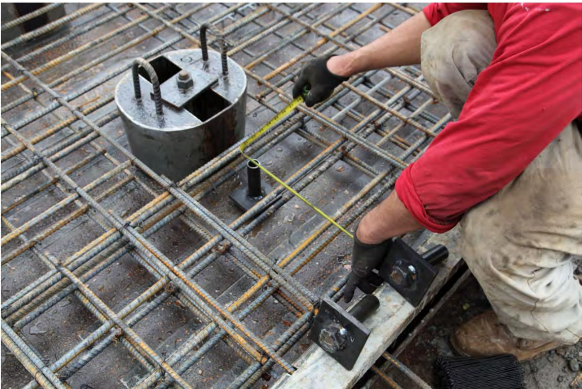
Fig. 4-5. Non-prestressed Precast Deck Panel, Reinforcement Around Shear Pocket, Positioning Leveling Bolt Embed
