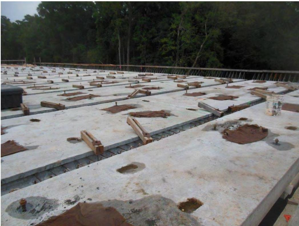
Fig. 4-29. Wet Burlap Placed Over Shear Pockets for Curing
