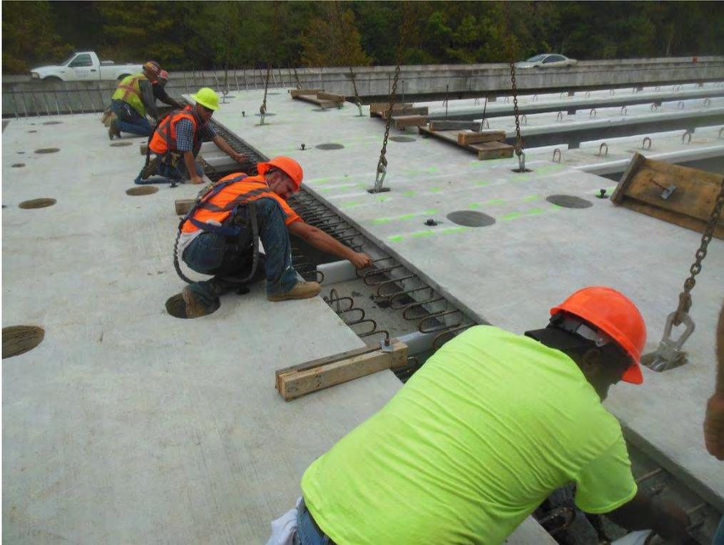
**Fig. 3-41. Carefully Positioning Panel on Polystyrene Forms on Girders**
