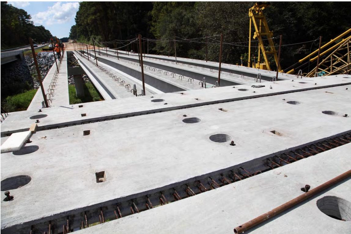
Fig. 3-39. Precast Deck Panels on Little River WB – Showing Closure Joints in Between
