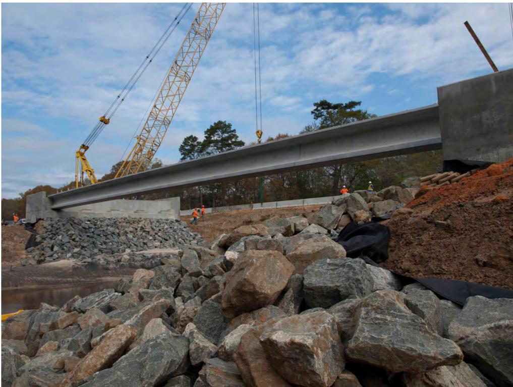
Fig. 3-5. First Girder Installed for Project – Hurricane Creek EB Bridge (March 24, 2014)
