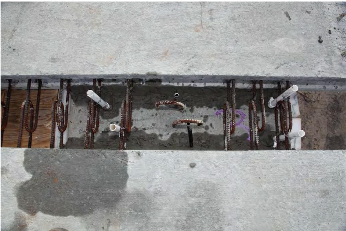
Fig. 3-64. Dry Pack Forming to Grout Shear Pockets on Little River WB
