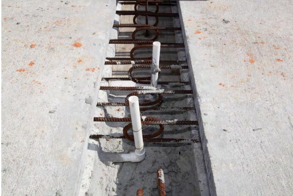
Fig. 4-19. Pipes for Grouting Shear Pockets on Hurricane Creek WB
