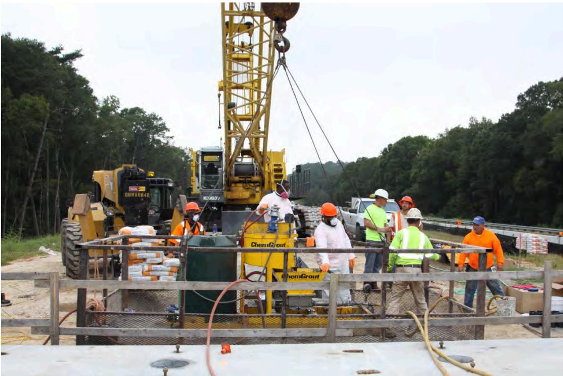
Fig. 4-8. Grouting Platform and Mixer/Pump
