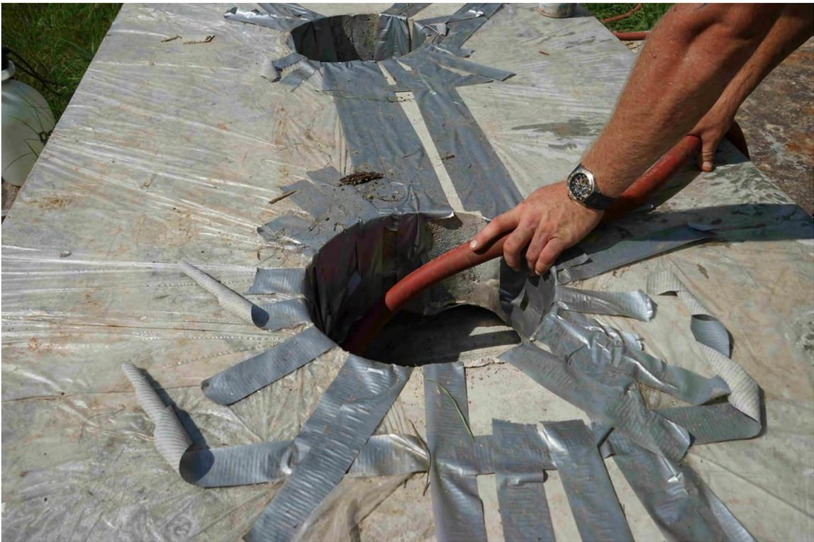
Fig. 5-16. Grout Mock-up for Precast Deck Panel, Dispensing Grout in "Panel" Shear Pocket
