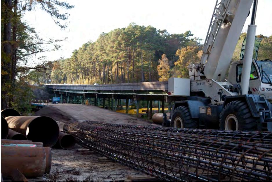
Fig. 2-2. Existing Little River EB Bridge During Construction: Drilled Shaft Reinforcing Steel Cage, Southeast Corner, Looking West (November 11, 2013)
