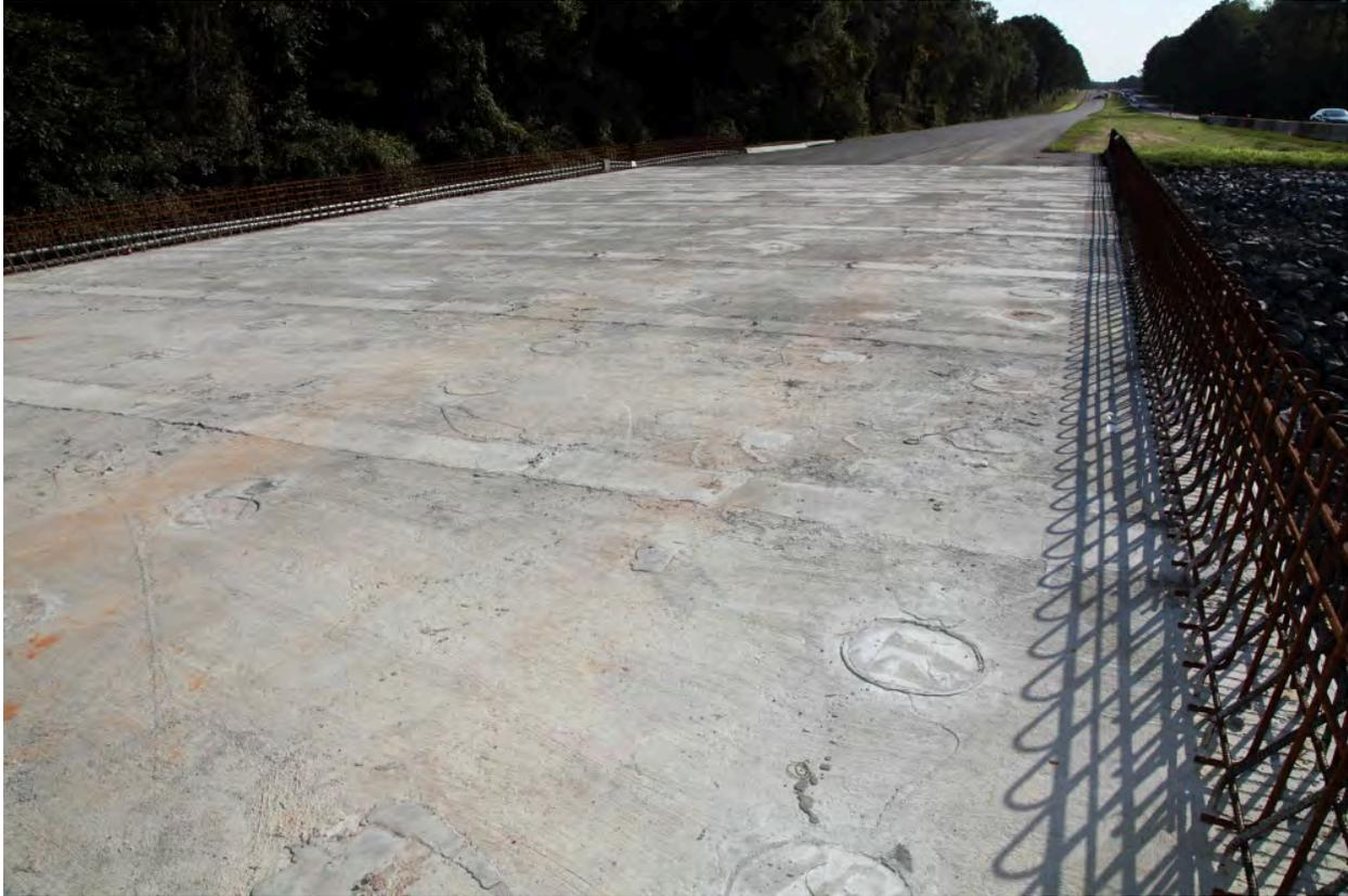
Fig. 4-46. Deck Surface of Hurricane Creek WB Bridge, Before Barriers and Milling
