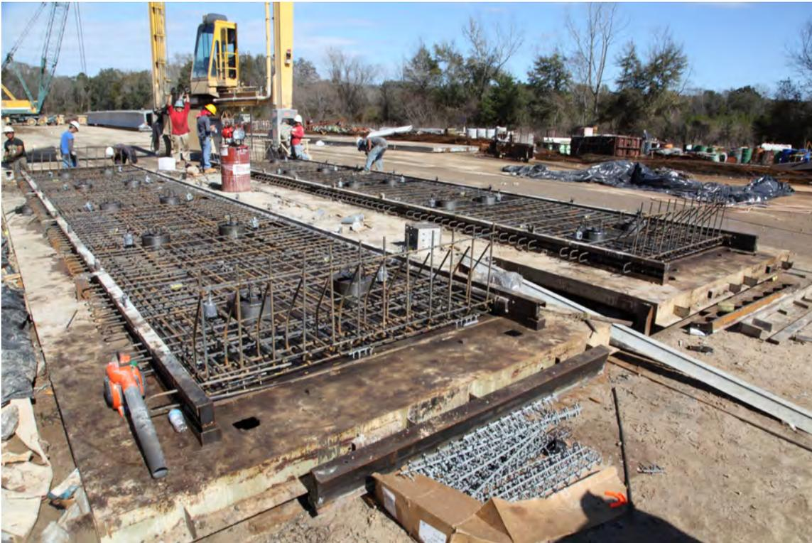
Fig. 4-3. Non-prestressed Precast Deck Panel, Twin Casting Beds
