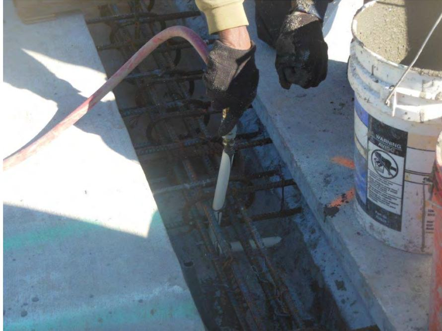
Fig. 4-21. Feeding Grout into Pipes for Shear Pockets
