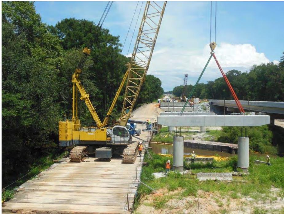
Fig. 2-20. Crane Setting a Precast Bent Cap from Temporary Work Bridge
