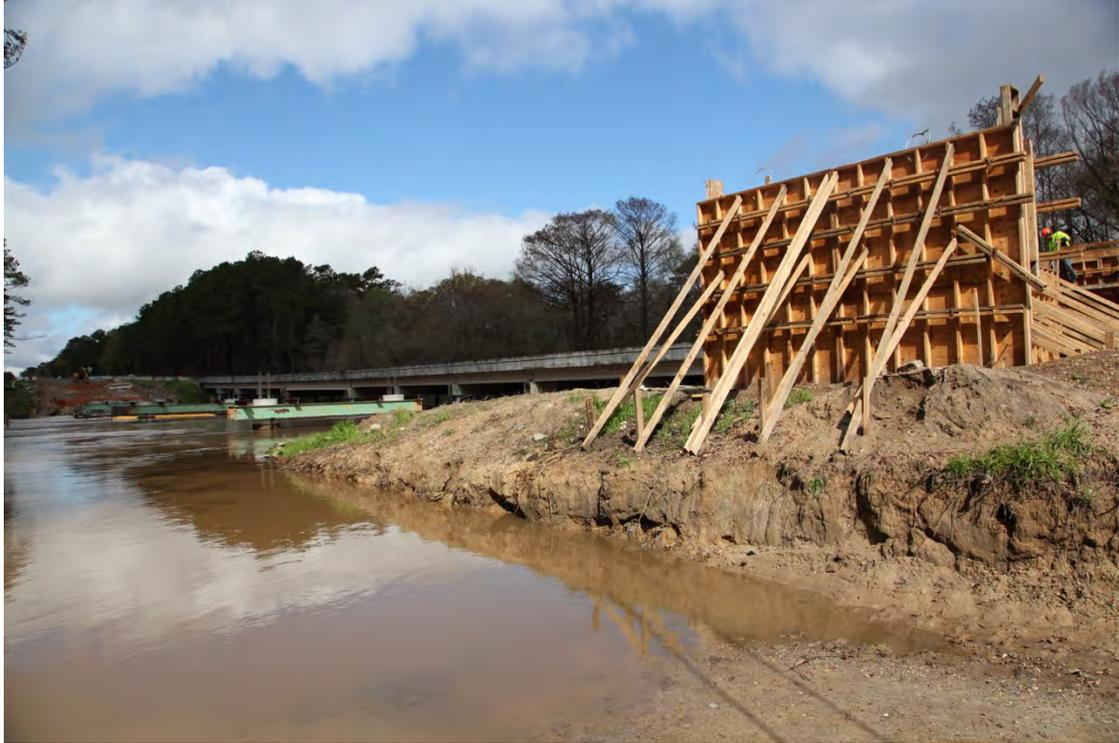
Fig. 2-4. Little River EB – Formwork for End Bent on East; High Water Level (March 18, 2014)
