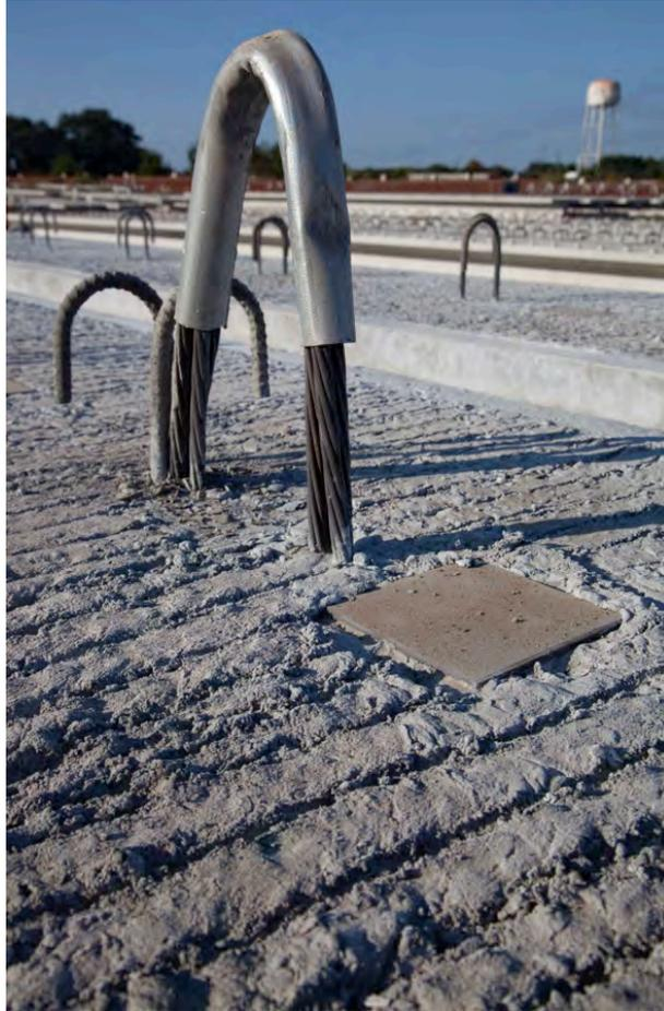
Fig. 2-14. Precasting Florida-I Beams: Close-up of Embedded Plate Assembly and a Lifting Loop; Roughened Surface on Top of FIB
