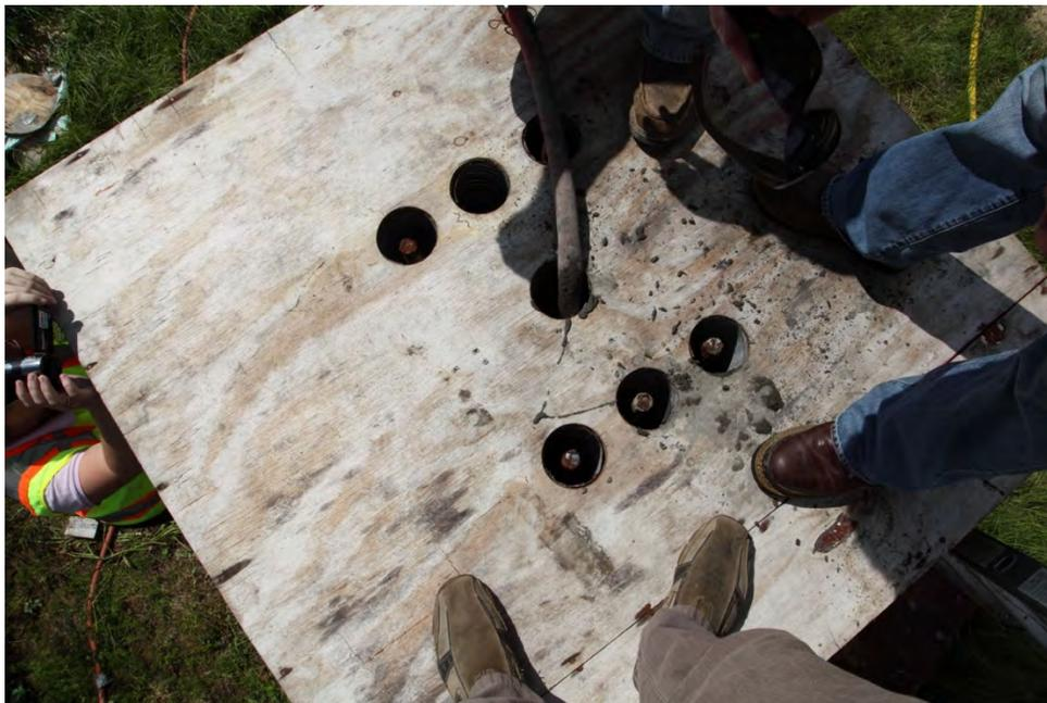
Fig. 5-4. Grout Mock-up for Precast Bent Cap, Dispensing Grout, Top View
