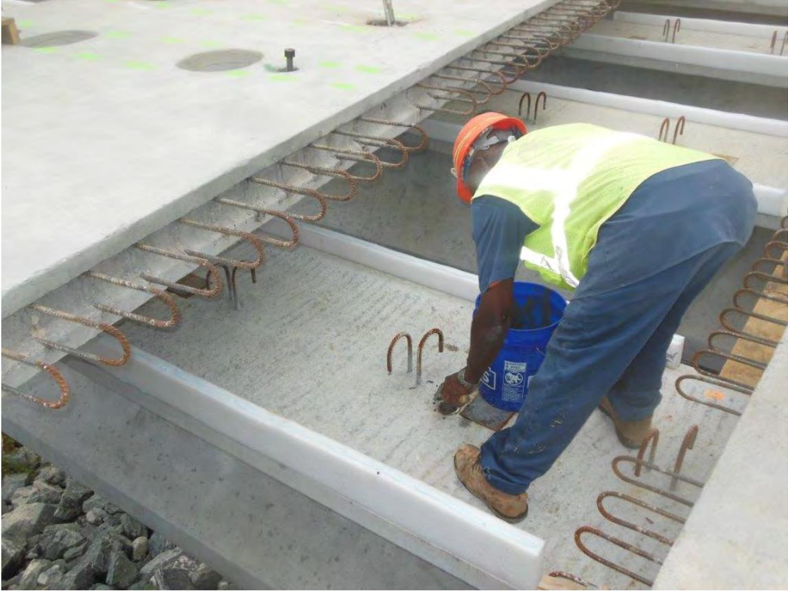
**Fig. 3-48. Filling Steel Pipes with Grout After Safety Line Pole Was Removed**
