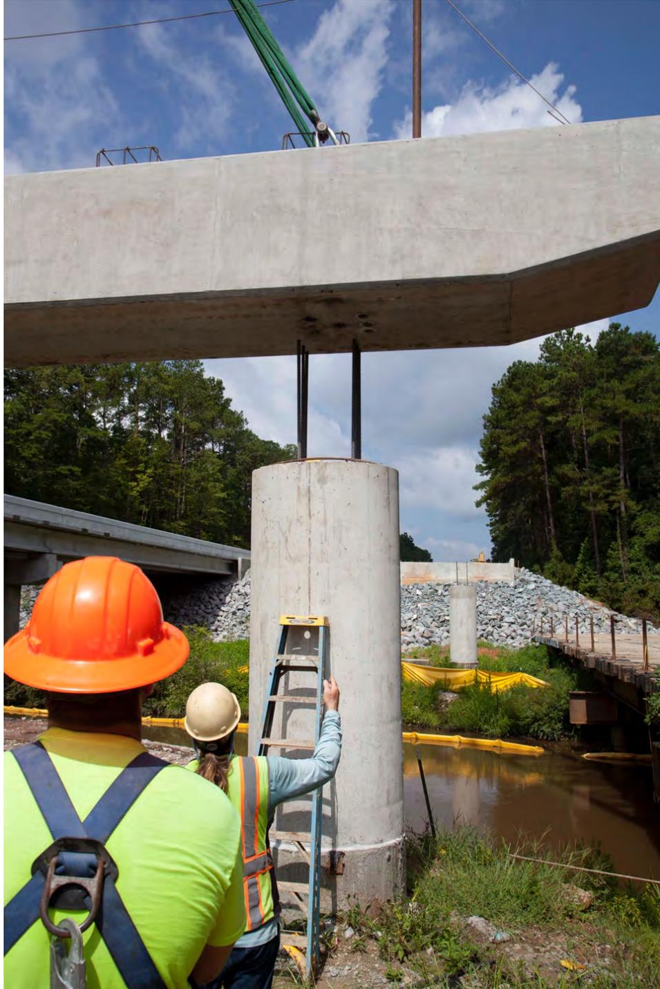
Fig. 2-22. Setting Precast Bent Cap over Dowel Bars (July 24, 2015)
