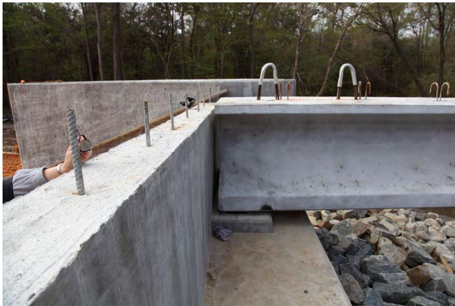
**Fig. 3-21. Girder and End Bent Pedestal – Hurricane Creek EB (March 24, 2014)**
