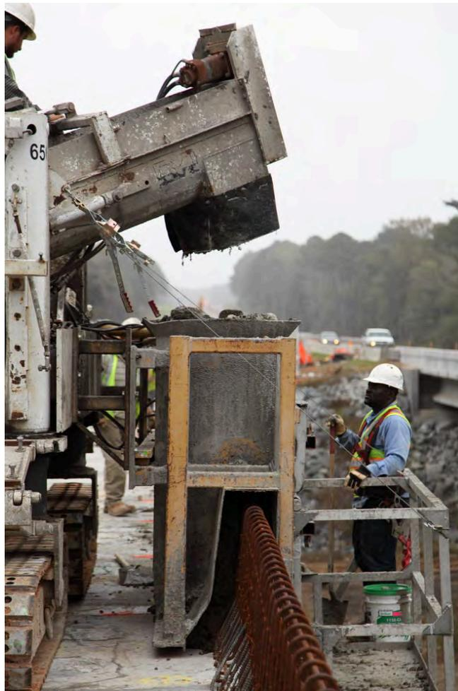
Fig. 4-50. Slip Forming Barriers on Little River WB – Slip Former
