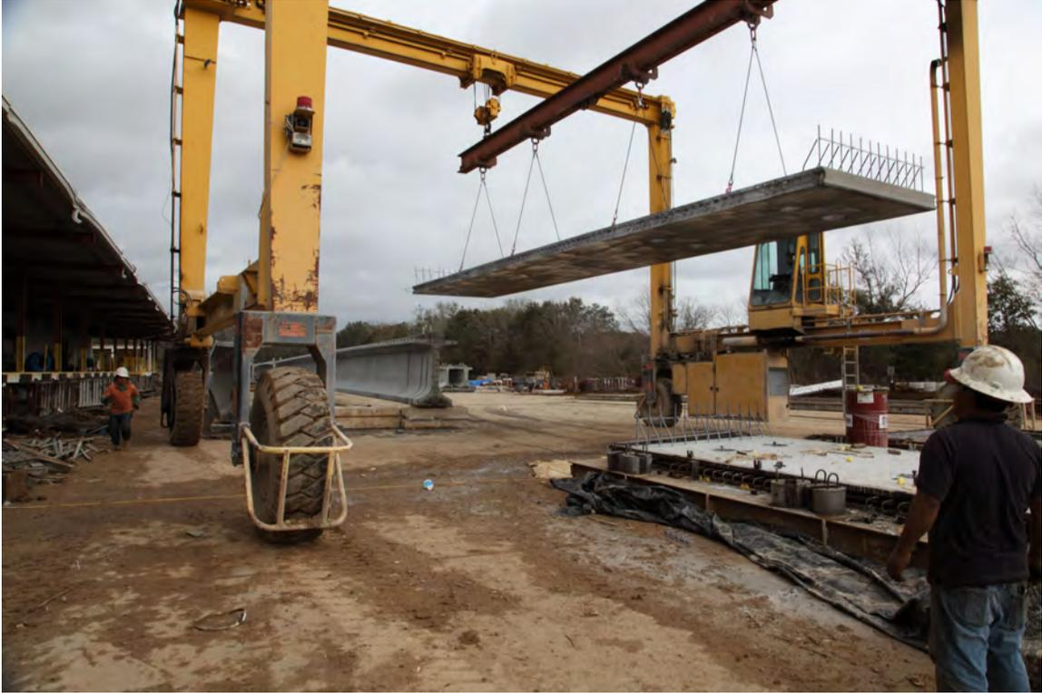
Fig. 4-6. Non-prestressed Precast Deck Panel Being Transported Around Casting Yard
