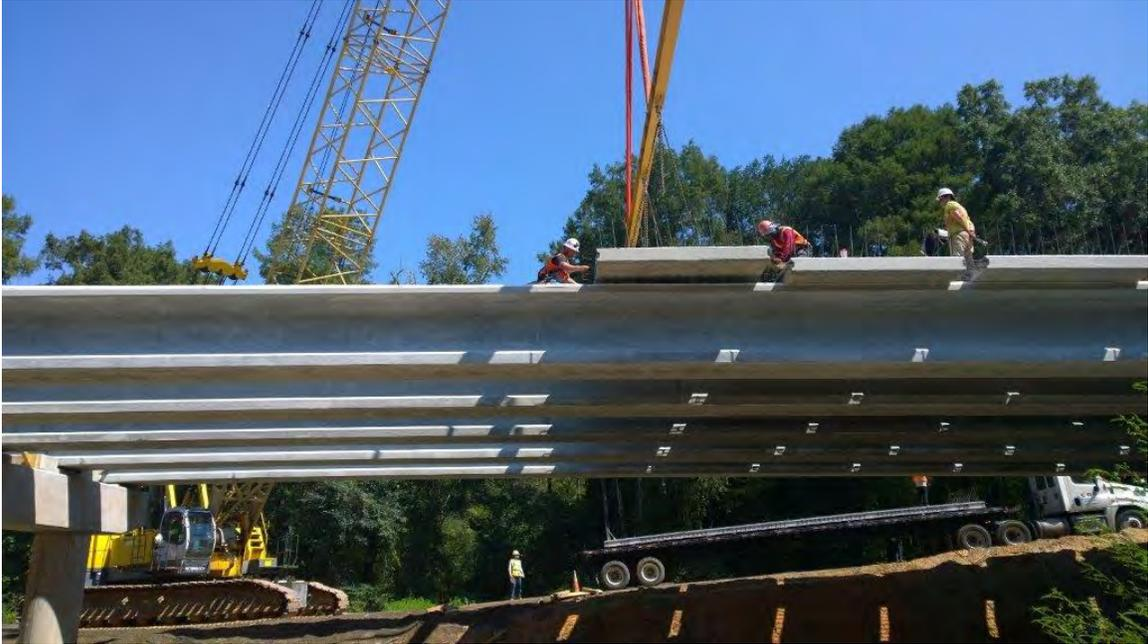
Fig. 3-38. Setting Panels on Girders, Leaving Gaps in Between for Closure Joints
