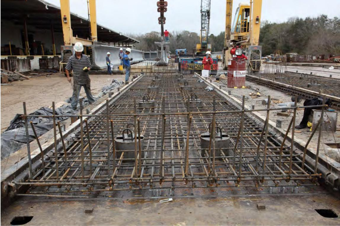
Fig. 4-4. Non-prestressed Precast Deck Panel, Reinforcing Steel
