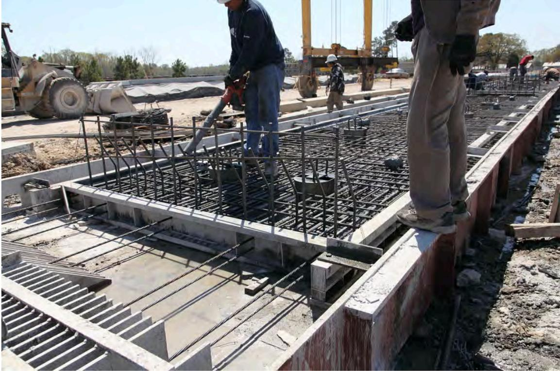
Fig. 5-8. Prestressed Precast Deck Panel Casting Bed, Oblique View of Forms
