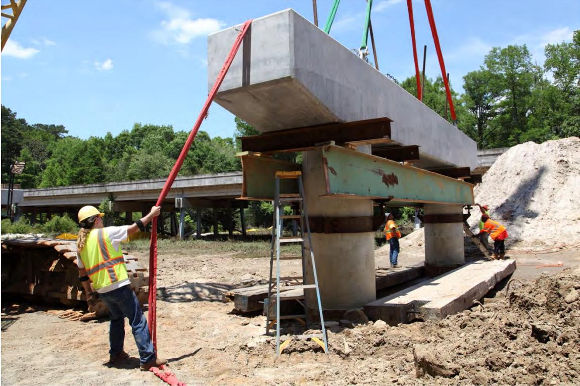
Fig. 2-23. Tethering a Precast Bent Cap while Setting (May 7, 2014)
