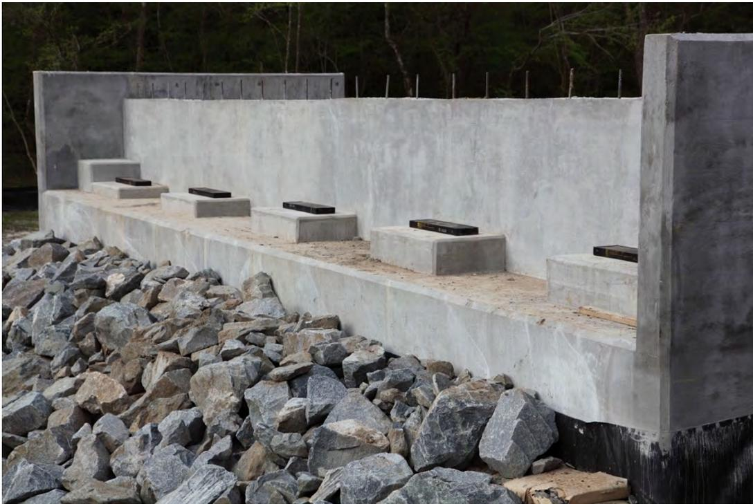
Fig. 2-9. Hurricane Creek EB – Completed End Bent on West and Rubble Rip Rap (March 24, 2014)
