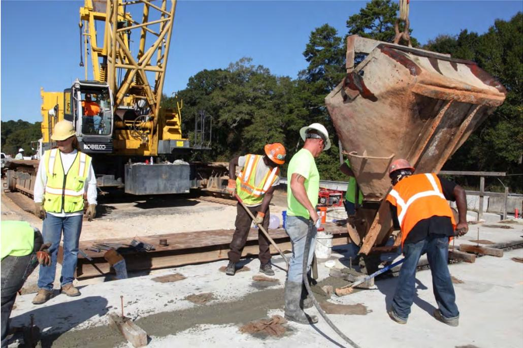
**Fig. 4-43. Leveling Out Closure Joint Concrete on Hurricane Creek EB**
