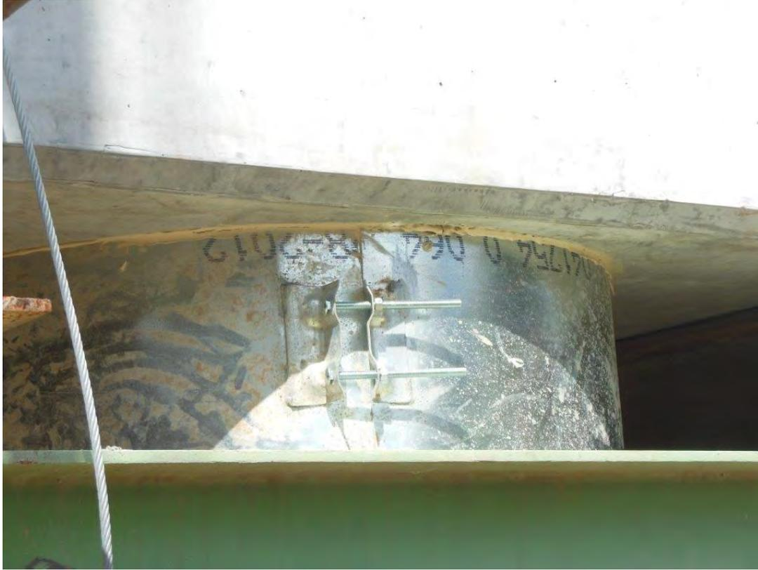
Fig. 2-28. Forms for Column-Bent Cap Connection
