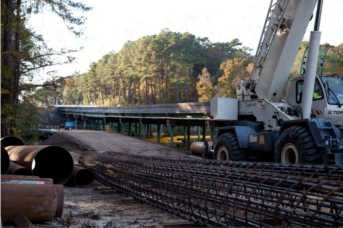
Fig. 2-8. Drilled Shaft Reinforcing Steel Cage for Little River EB Bridge, View from Southeast Corner, Looking West
