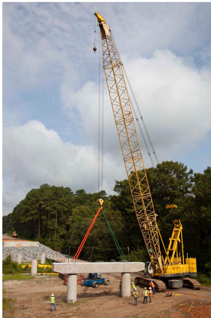
**Fig. 2-18. Setting a Precast Bent Cap Using a Two-Point Pick (July 24, 2015)**
