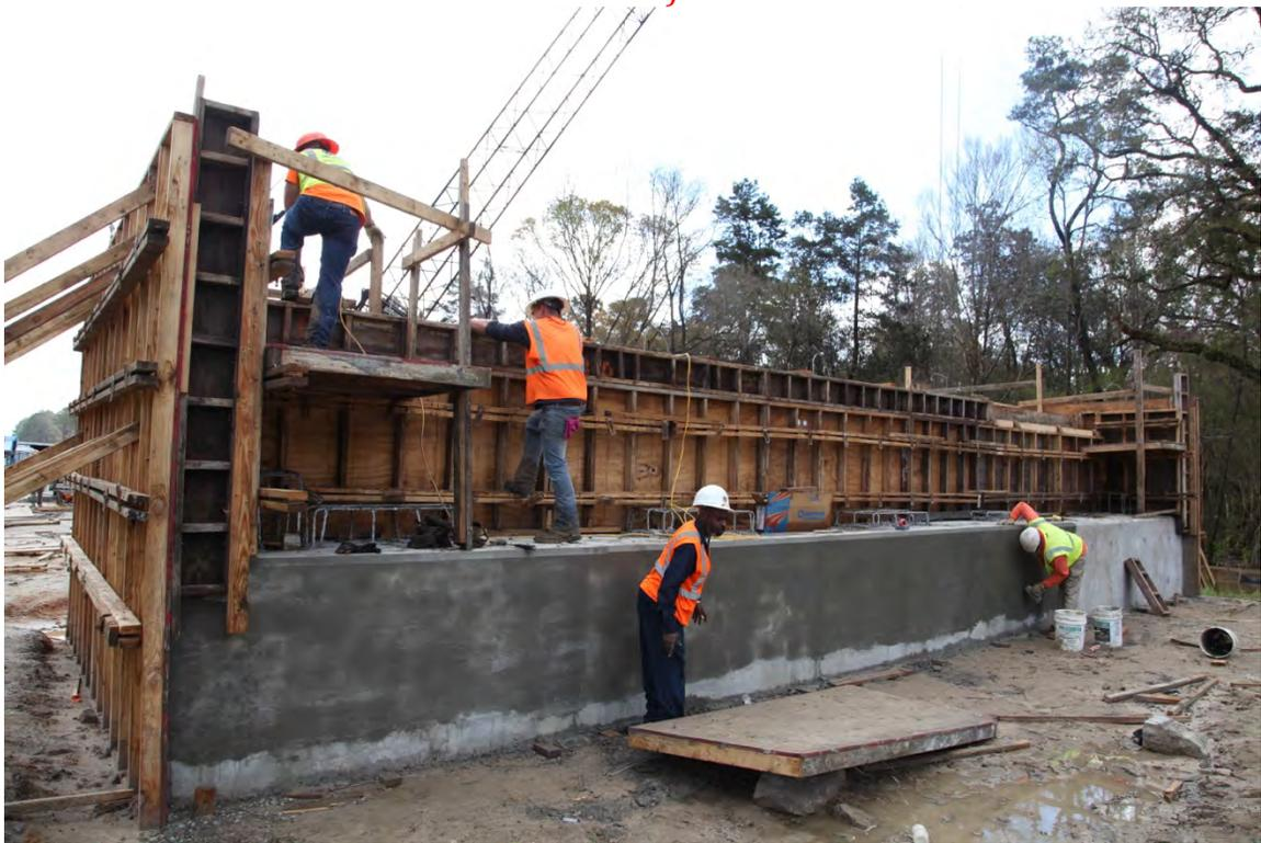
Fig. 2-5. Little River EB – Finishing Front Face of End Bent Cap on East (March 18, 2014)
