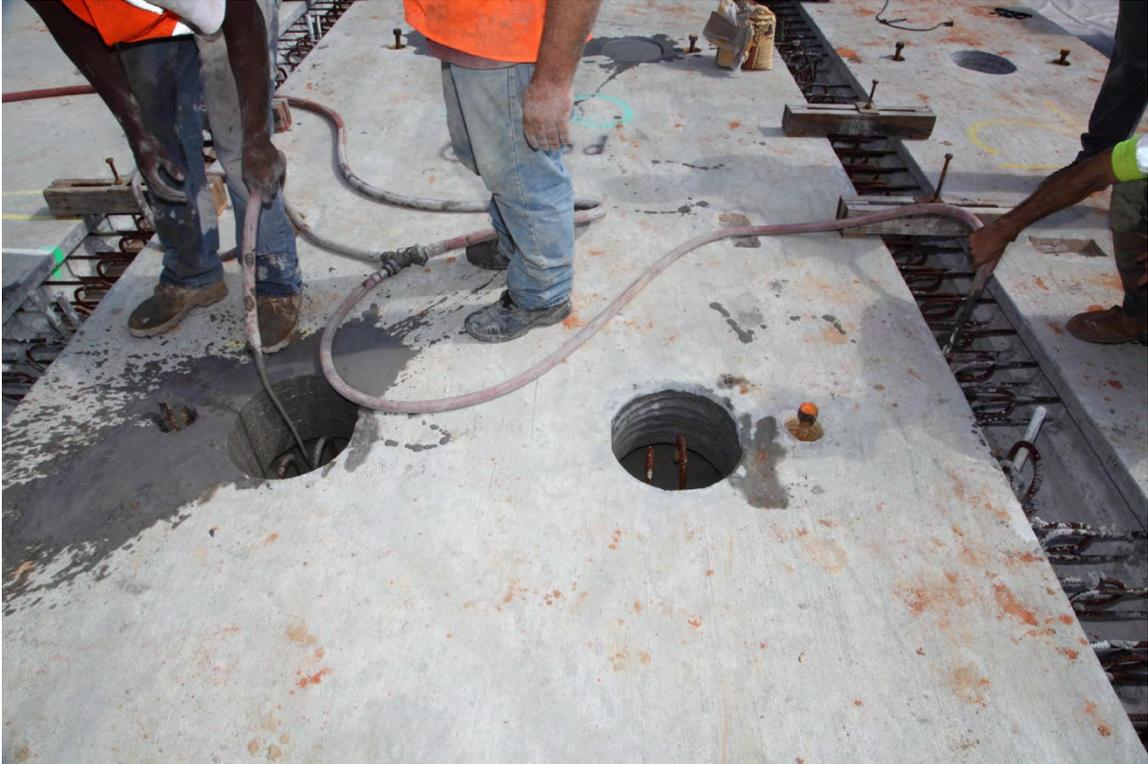
**Fig. 4-12. Grouting a Pair of Panel Pockets on Hurricane Creek WB**
