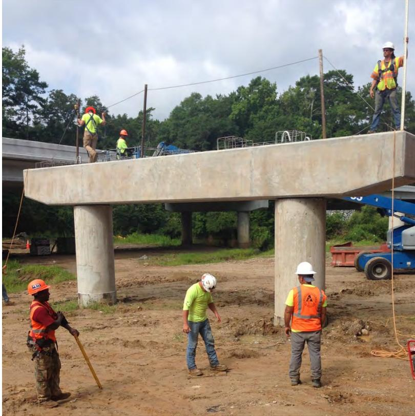
Fig. 2-25. Surveying a Precast Bent Cap
