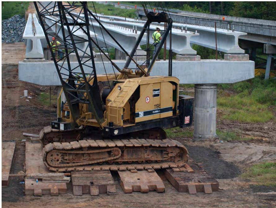
Fig. 3-13. Crane for Setting Girders on Little River EB (September 20, 2014)
