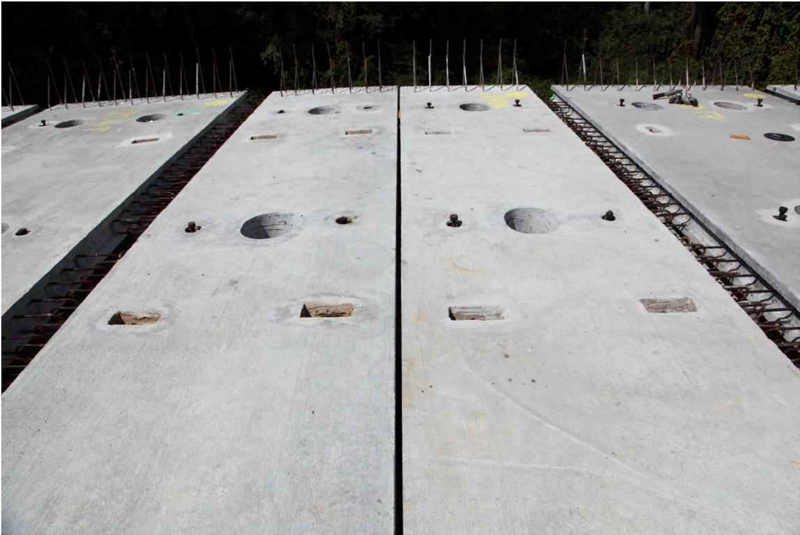
Fig. 1-3. Precast Deck Panels, Looking Transversely on Little River WB (August 31, 2015)
