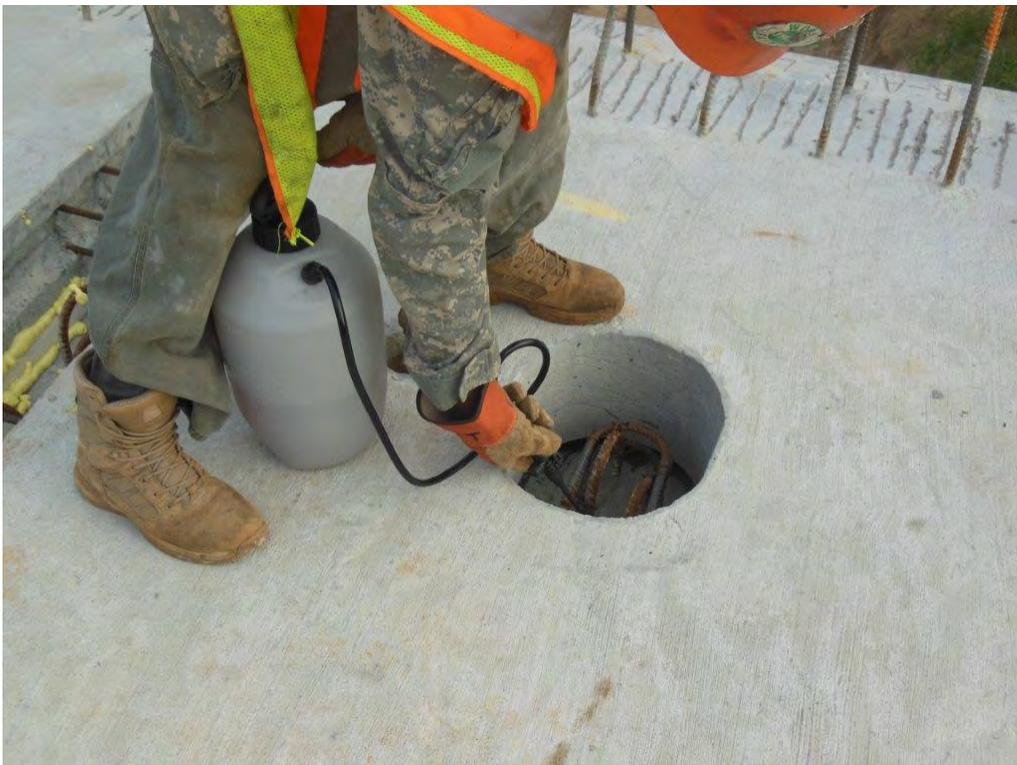
**Fig. 4-13. Spraying Epoxy Bonding Agent Around Perimeter of Shear Pocket**
