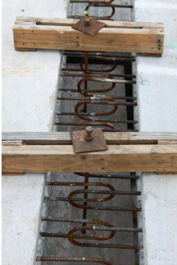
Fig. 4-38. Closure Joint Forms Suspended from Wood and Steel Rods, View from Above
