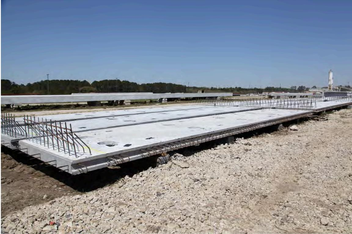
**Fig 5-14. Prestressed Precast Deck Panel Casting Bed, Barrier Reinforcement in Foreground**
