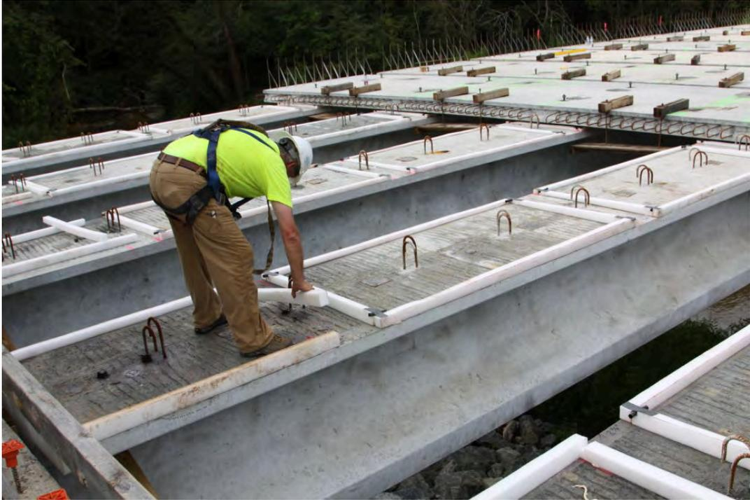
Fig. 3-50. Laying Polystyrene Forms
