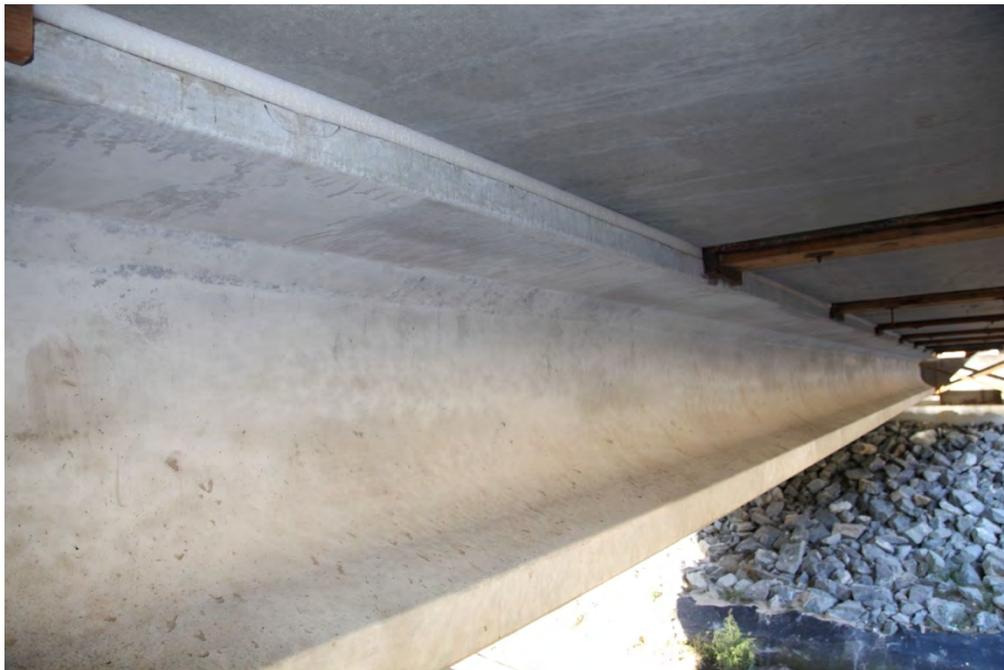
Fig. 3-57. Polystyrene Forms in Haunch
