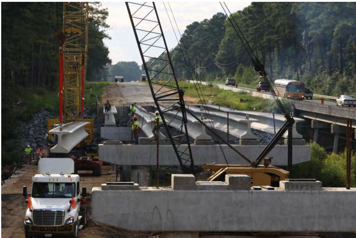
Fig. 3-11. Setting Girders on Little River EB using Access Road (September 18, 2014)
