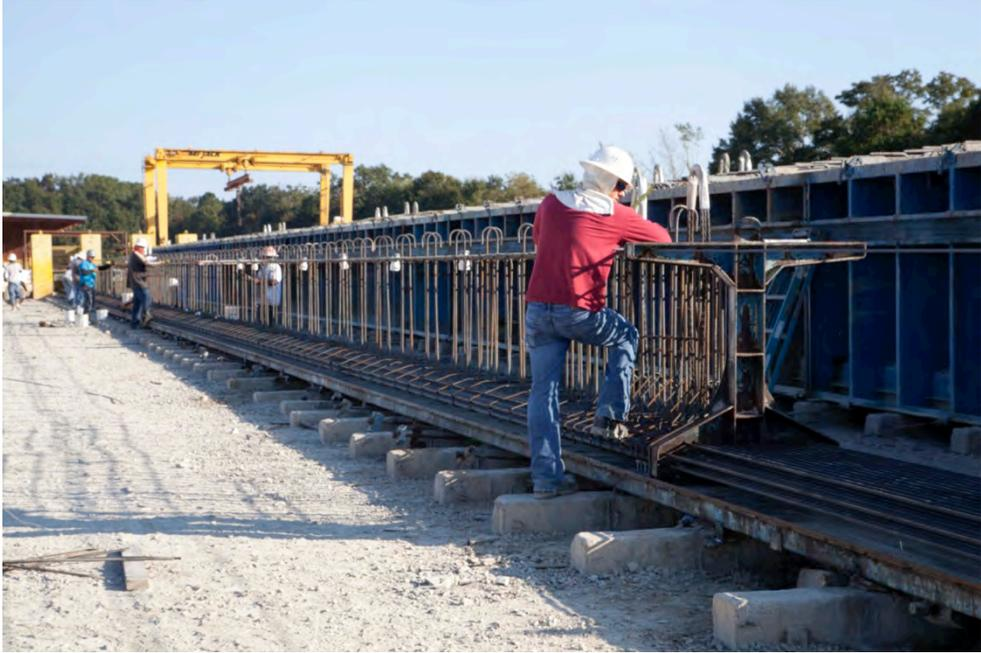
Fig. 2-4. Precasting Florida-I Beams: Precast Bed, Reinforcing Steel, and Strands
