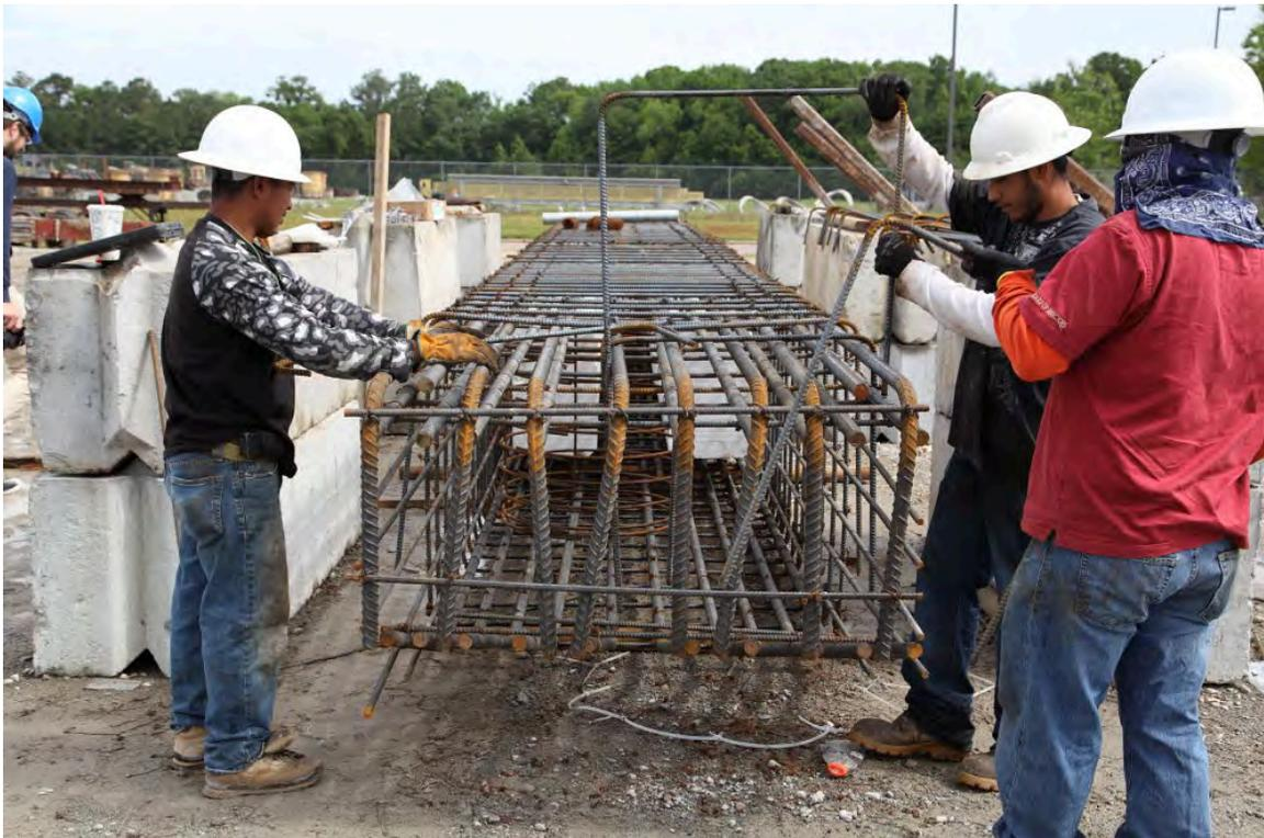
Fig. 6-10. Precast Bent Cap, Reinforcing Steel Cage, End View
