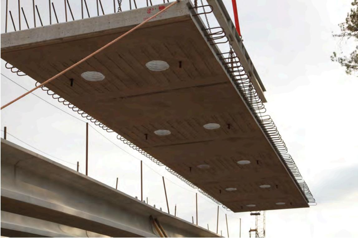
Fig. 3-34. View of Panel's Underside While Being Lifted to Set on Girders
