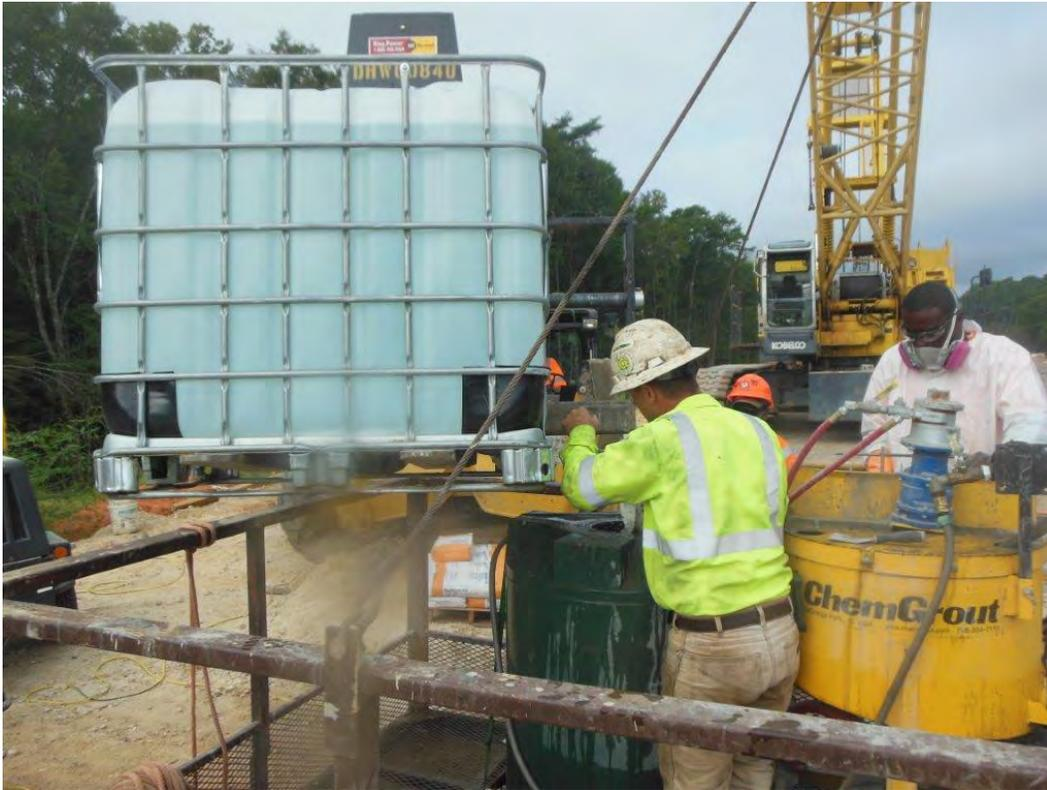
Fig. 4-5. Water Storage Unit for Grouting
