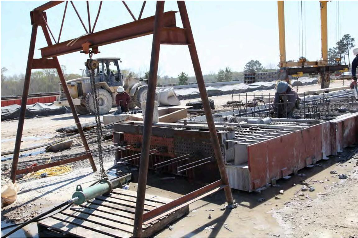
Fig. 5-6. Prestressed Precast Deck Panel Casting Bed, Showing Prestressing Jack Hanging from Frame
