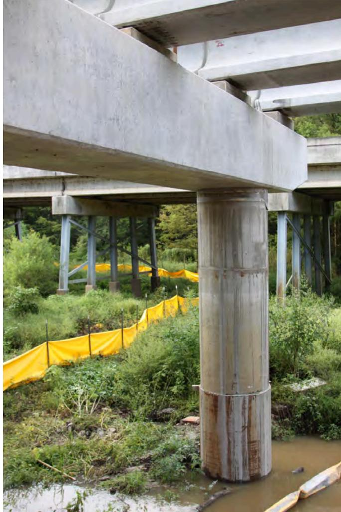
Fig. 2-17. Column, Bent Cap, and FIBs on Little River EB (September 18, 2014)
