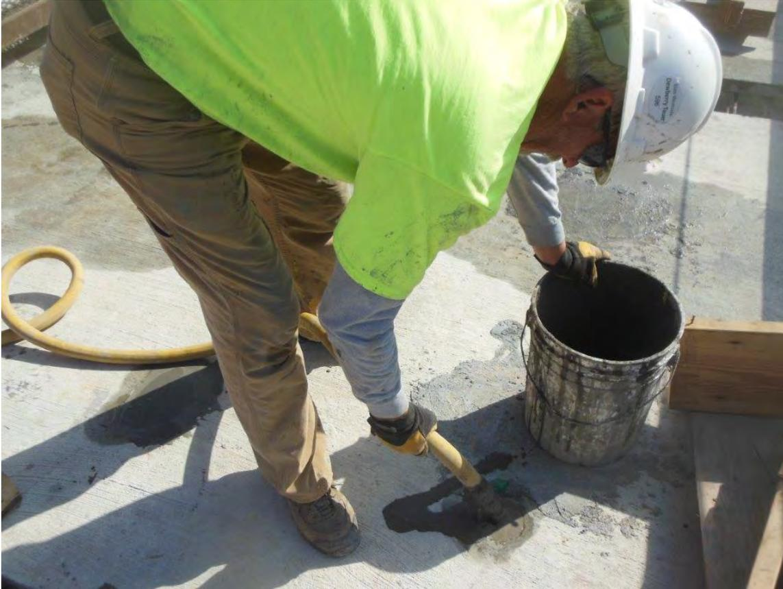
**Fig. 4-33. Grouting Lifting Eyes on Deck Panel**
