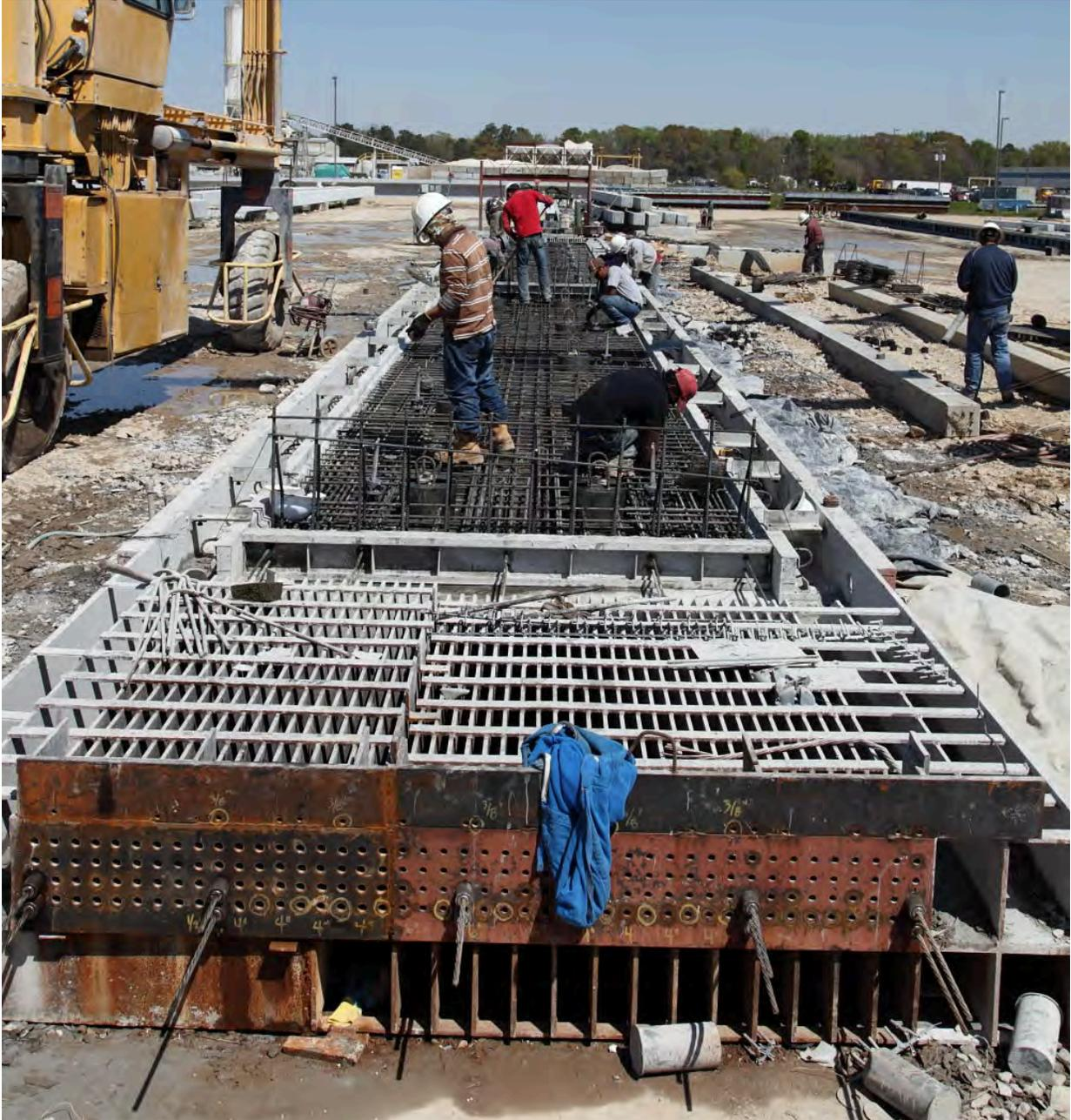
Fig. 5-4. Prestressed Precast Deck Panel Casting Bed, Strands Extending in Foreground
