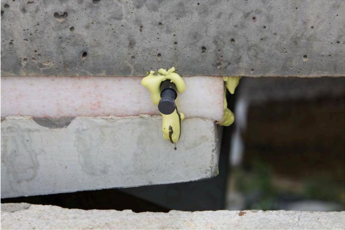
Fig. 4-17. Plugged Grout Port for Grouting Shear Pockets on Hurricane Creek EB
