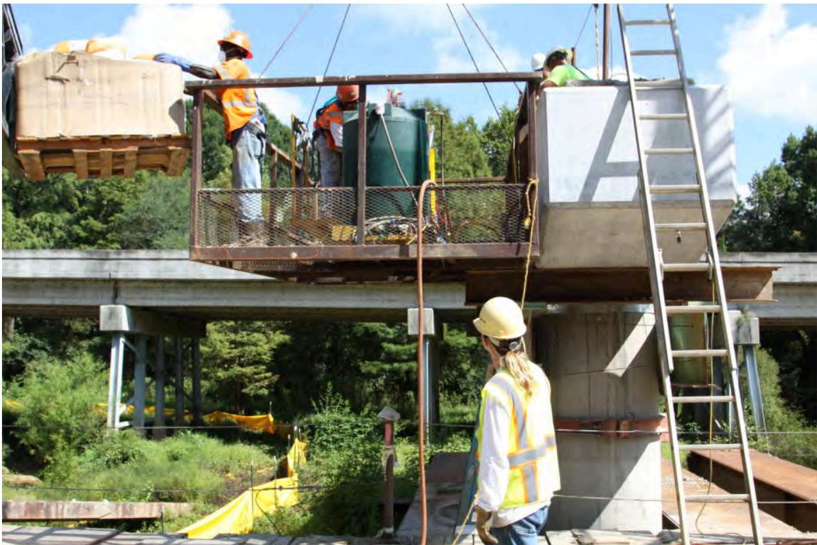
Fig. 2-31. Grouting Bent Cap on Little River EB, Grout Pump Platform Next to Bent Cap (September 11, 2014)
