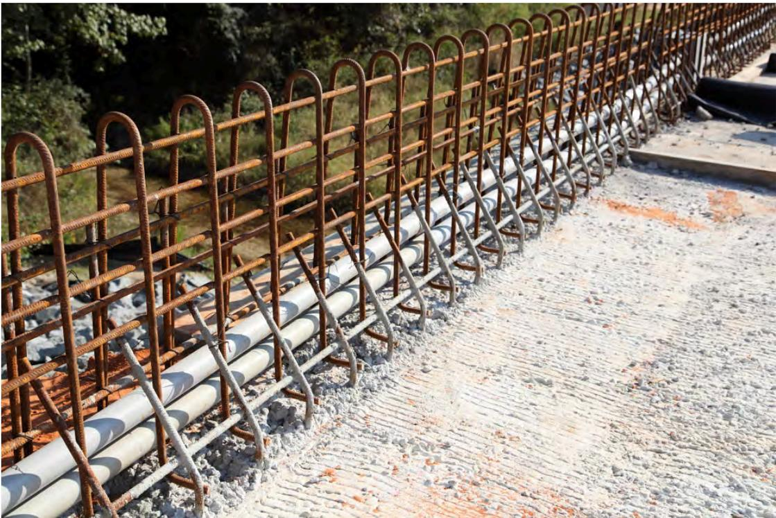
Fig. 4-48. Barrier Reinforcing Steel and Embedded Pipes for Hurricane Creek WB
