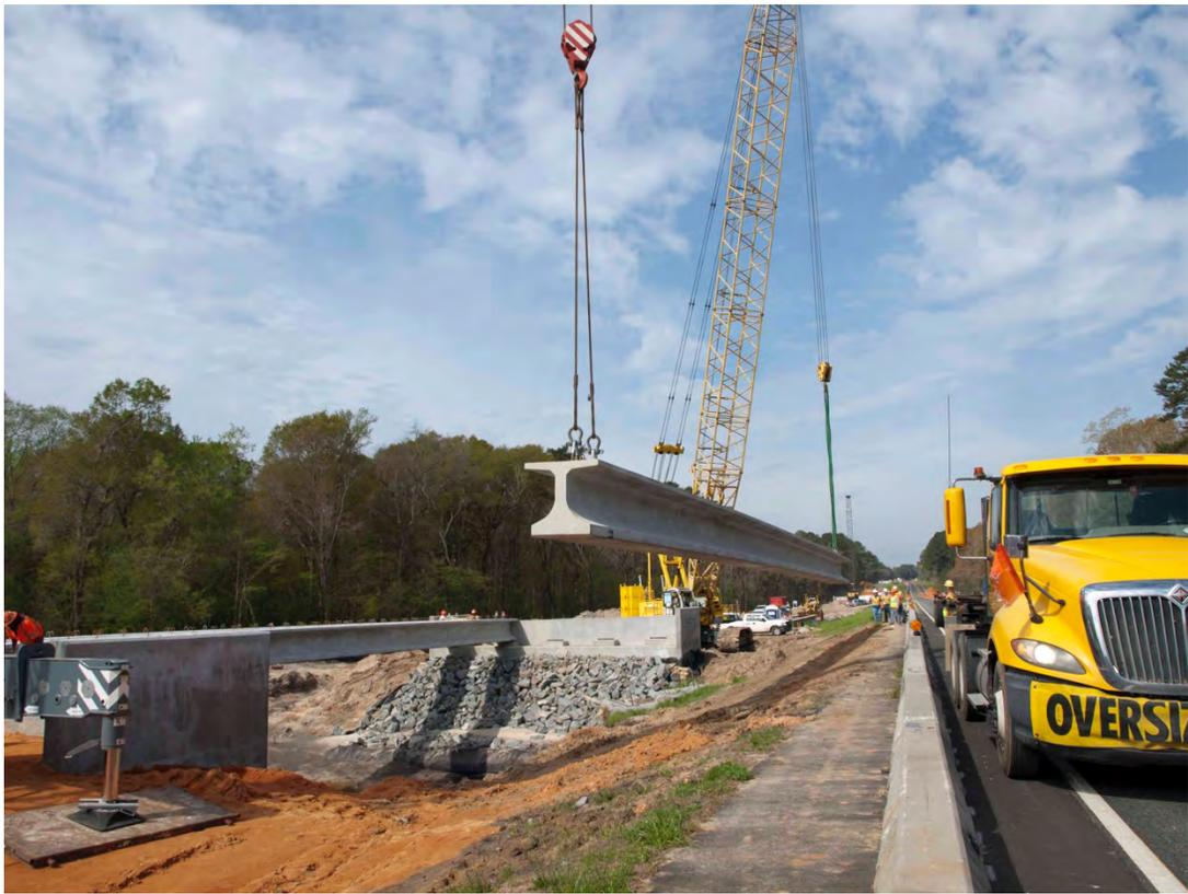
Fig. 3-3. Girder Being Lifted from Delivery Truck for Hurricane Creek EB (March 24, 2014)
