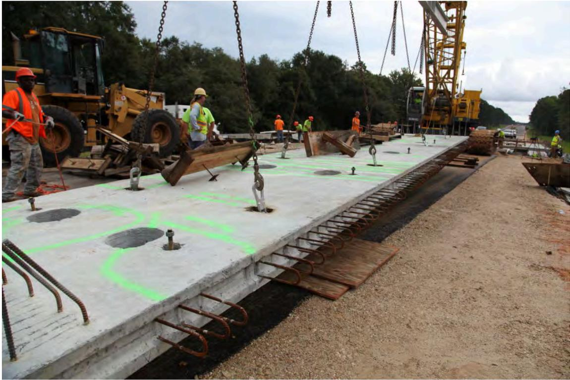
Fig. 3-29. Lifting Precast Deck Panel on Hurricane Creek EB (September 8, 2014)
