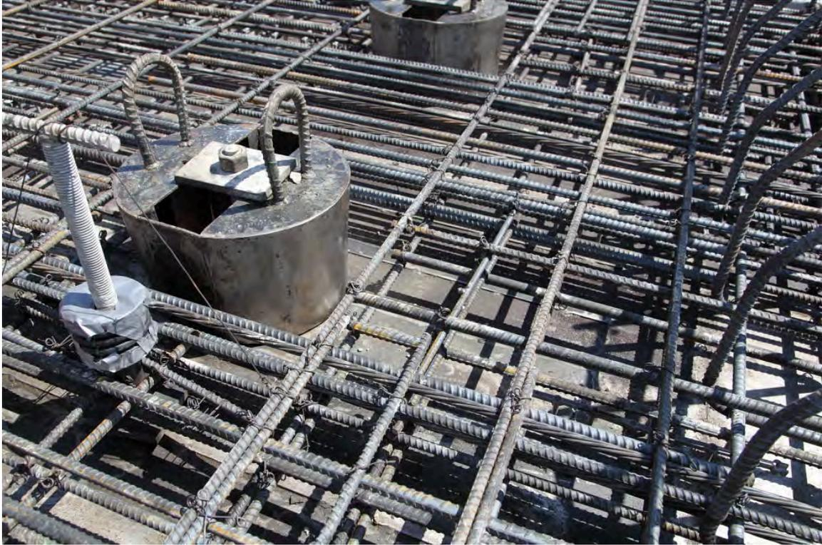
Fig. 5-12. Prestressed Precast Deck Panel, Shear Pocket and Leveling Bolt Embeds
