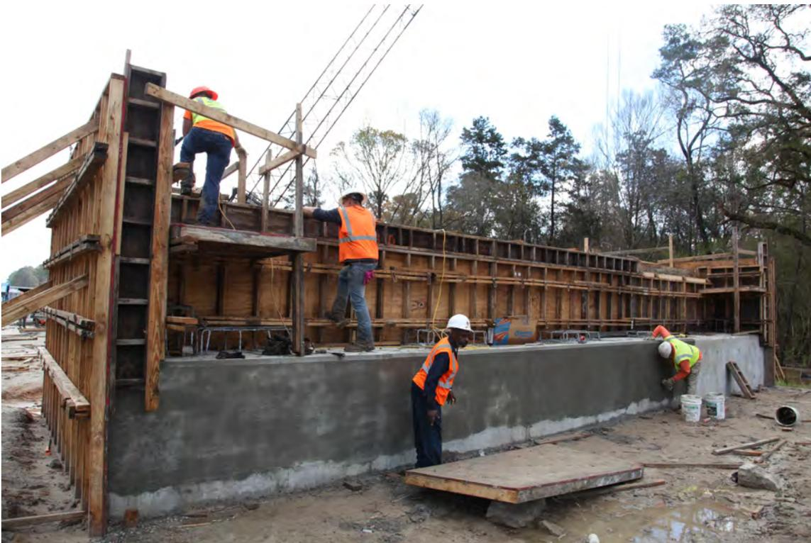
Fig. 2-11. Little River Bridge, Finishing Front Face of East End Bent
