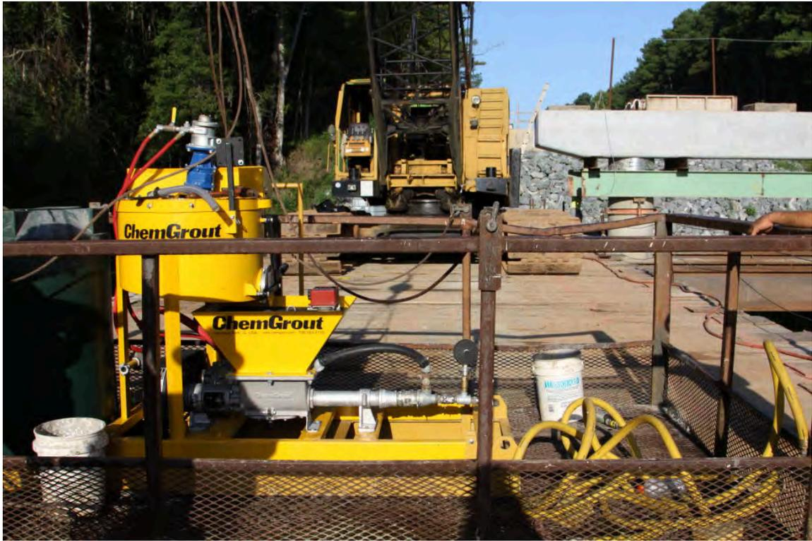
Fig. 2-30. Grouting Bent Cap on Little River EB, Grout Pump Equipment and Platform
