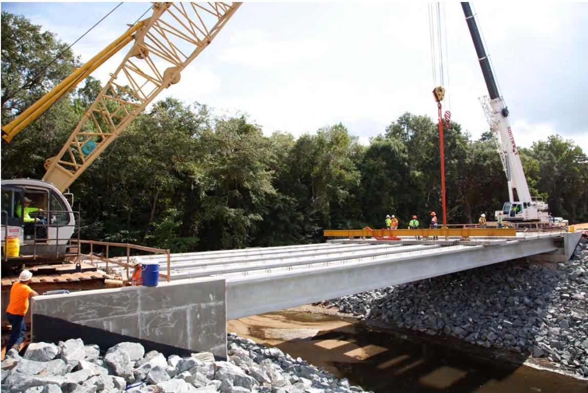
Fig. 3-35. Setting Panels on Hurricane Creek WB (June 26, 2015)
