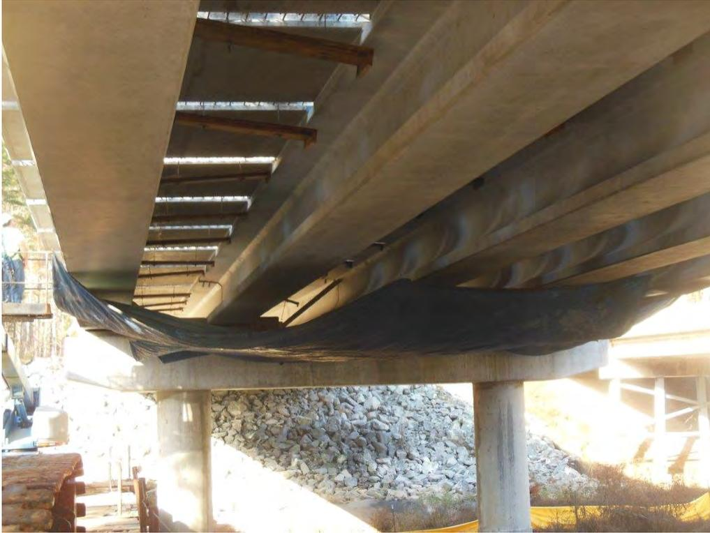
Fig. 4-14. Tarp Placed Underneath Bridge to Catch Leaking Grout
