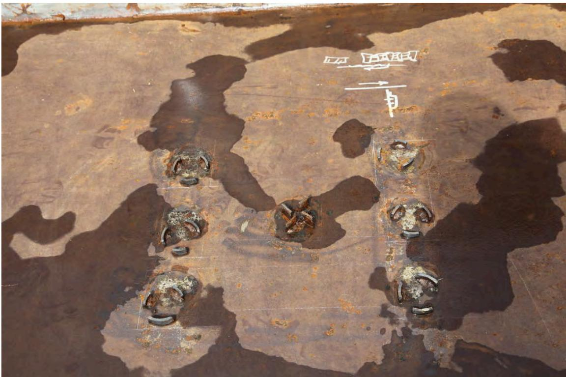
Fig. 6-13. Precast Bent Cap, Close-up of Template to Secure Pipe Forms for Dowel Bar Holes
