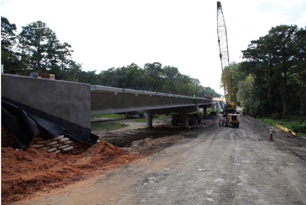
**Fig. 3-28. Precast Deck Panels Were Delivered to Access Road on Little River WB (August 31, 2015)**
