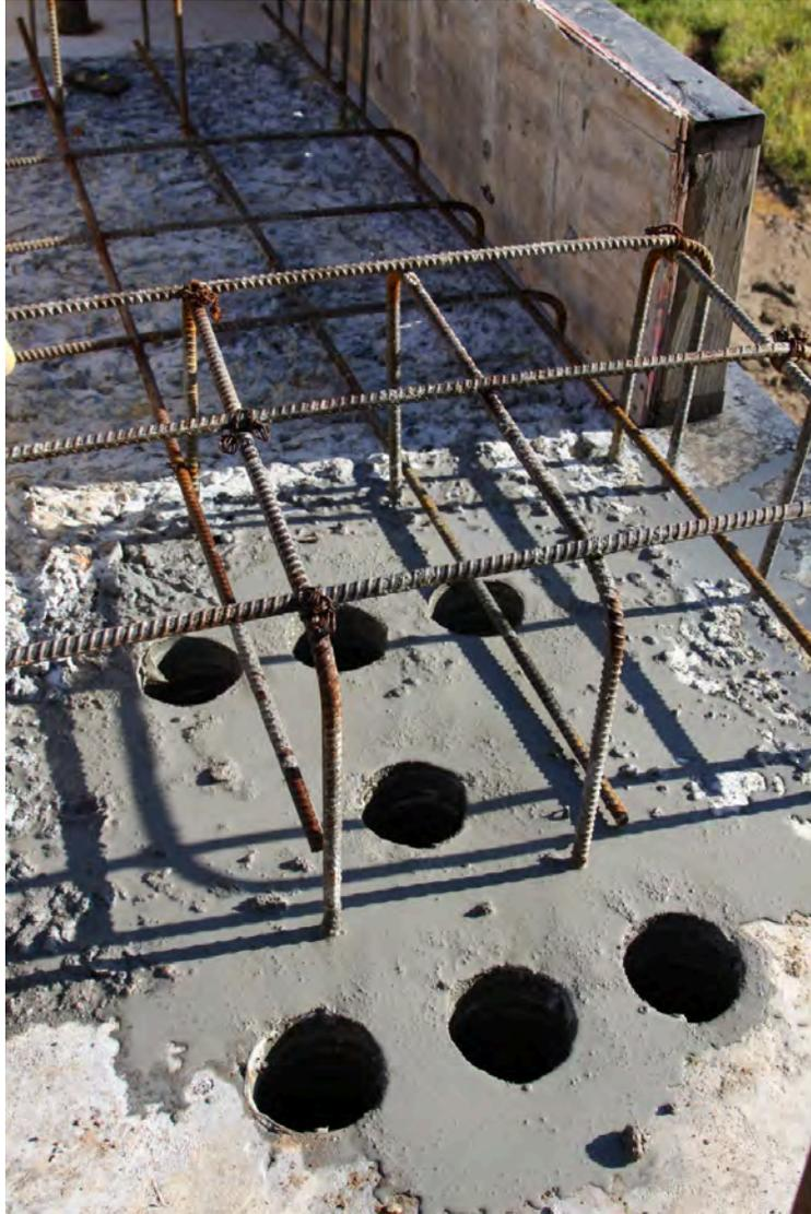
Fig. 2-34. Bent Cap on Little River EB, Holes for Grouting 6 Dowel Bars (September 14, 2014)
