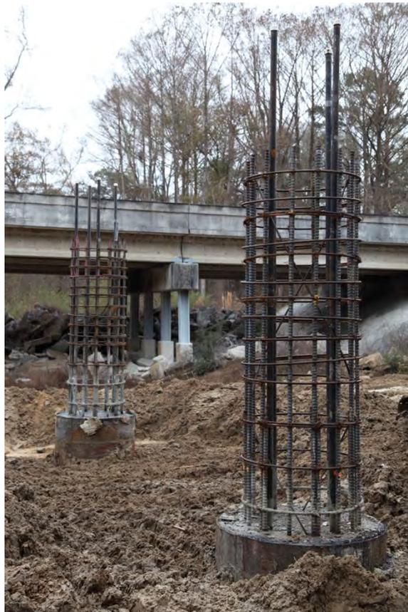
Fig. 2-3. Drilled Shaft Reinforcement for Little River EB Intermediate Bent (February 3, 2014)
