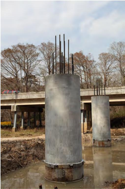
Fig. 2-18. Columns Extending from Drilled Shafts, Showing Dowel Bars to Connect to Bent Cap, for Little River Bridge Intermediate Bent
