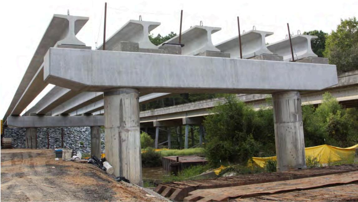
Fig. 3-24. Girders and Intermediate Bent on Little River EB (September 18, 2014)
