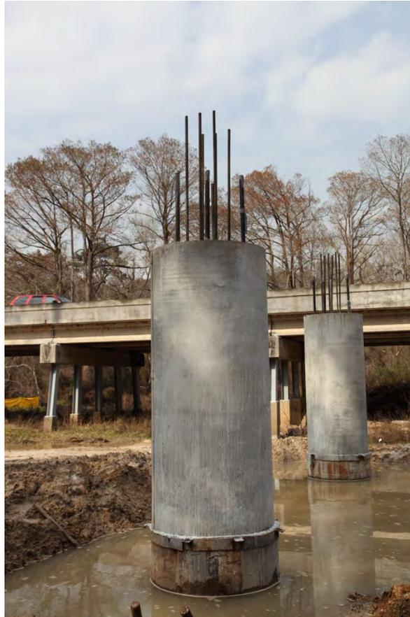
**Fig. 2-14. Completed Columns for a Little River EB Intermediate Bent (February 14, 2014)**
