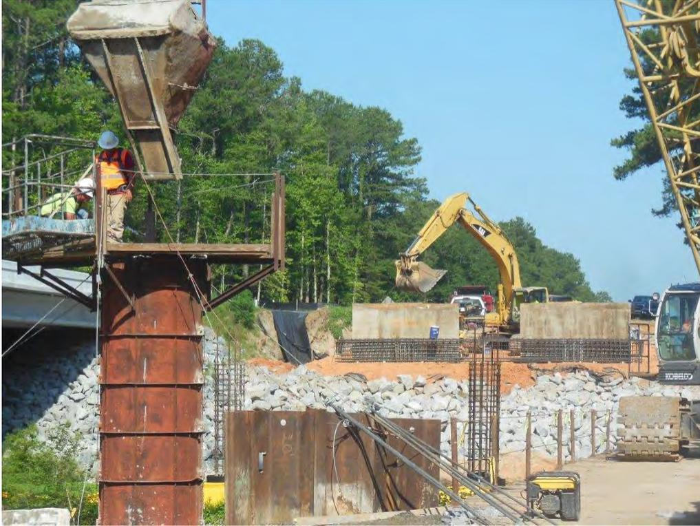
Fig. 2-12. Casting a Column for an Intermediate Bent
