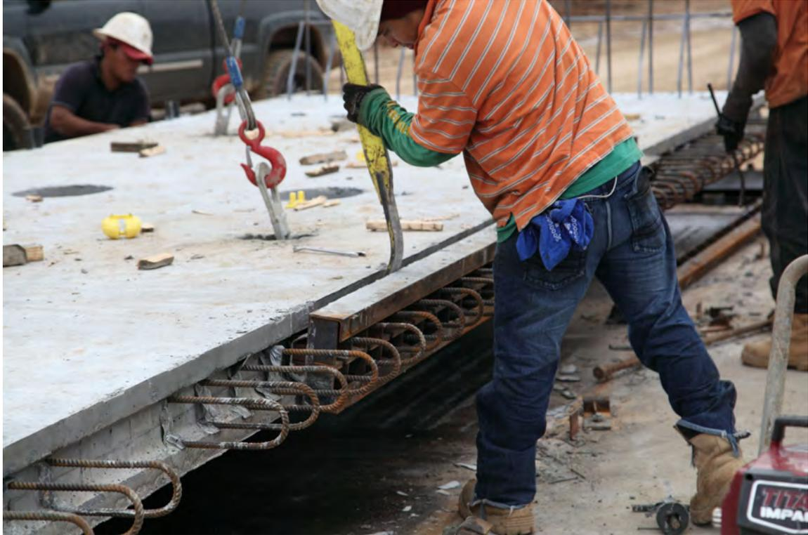
Fig. 3-6 Precast Deck Panel Being Removed from Forms. Keyway and Closure Joint Bars 4C Shown
