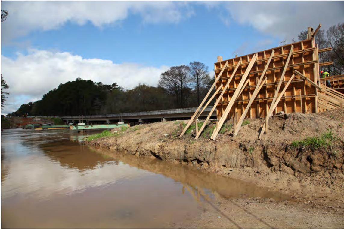
Fig. 2-10. Little River Bridge, East End Bent Formwork and High Water Level
