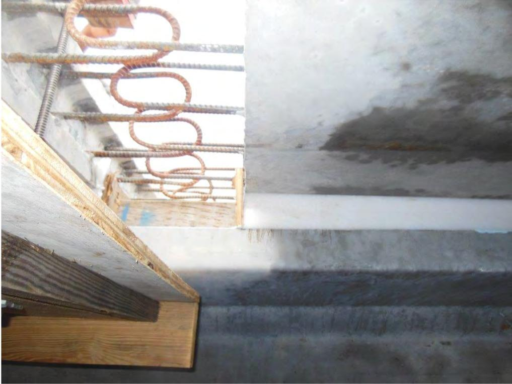
Fig. 4-36. Closure Joint Forms Left Hanging After Panels Were Placed (View from Underneath Panel)
