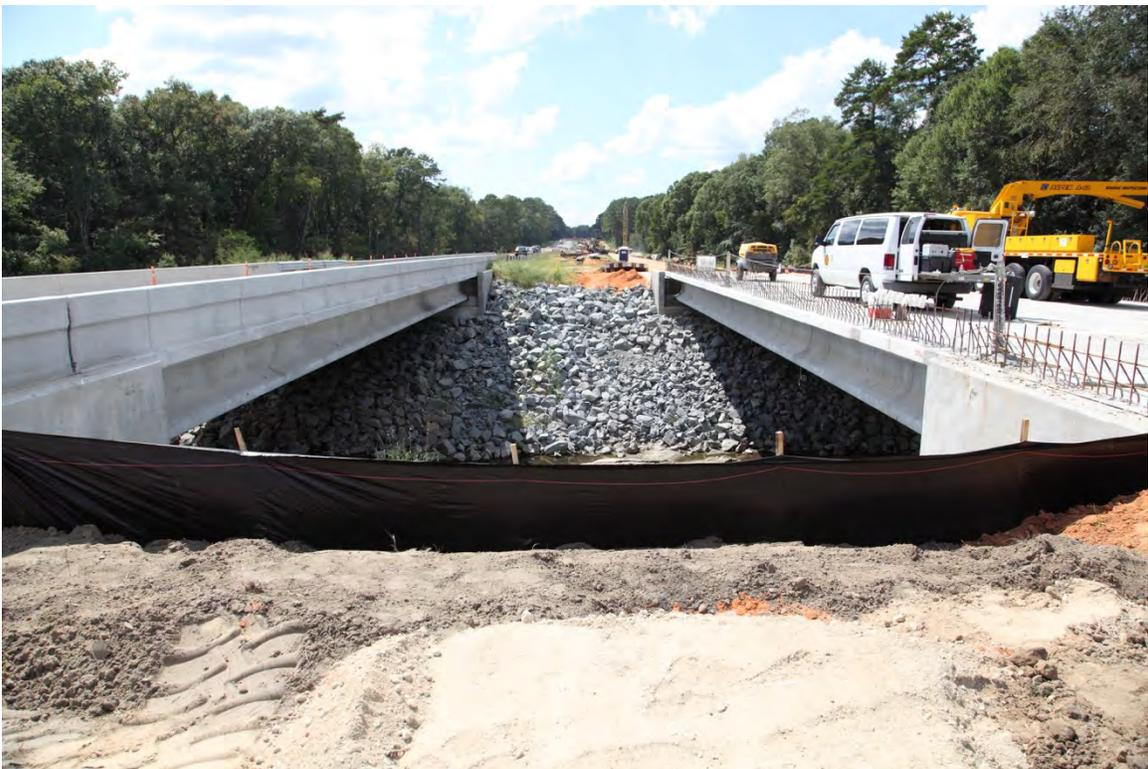
Fig. 4-52. Completed Barrier on Hurricane Creek EB (on Left) While Load Test is Being Performed on Hurricane Creek WB (on Right)
