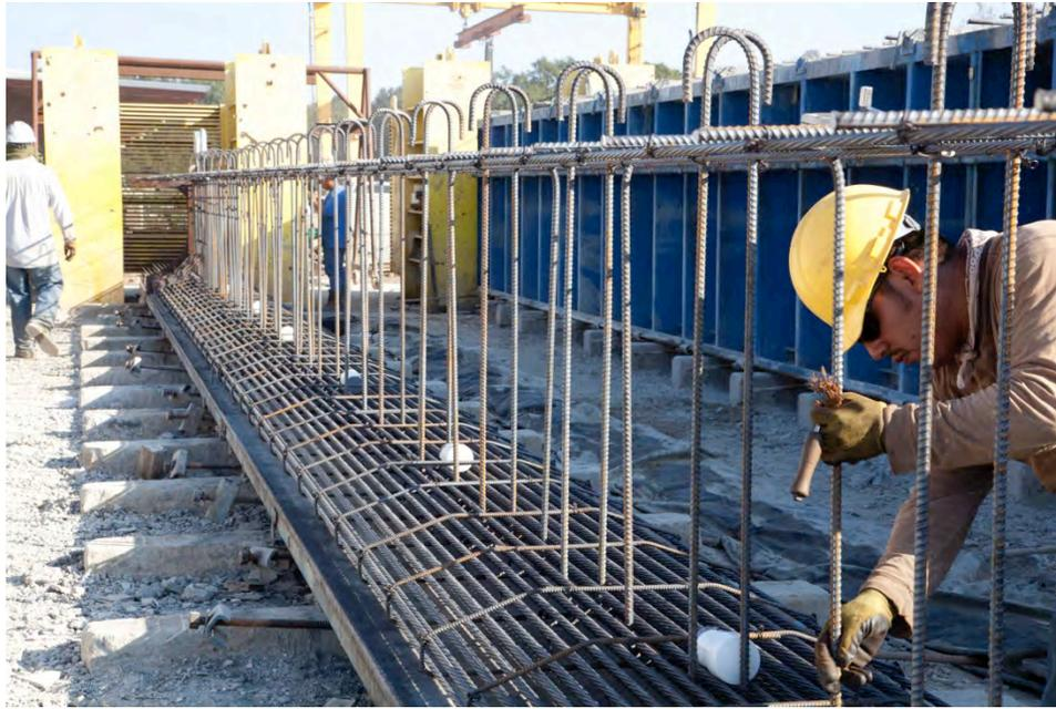
Fig. 2-6. Precasting Florida-I Beams: Getting Bars 5Z in Position
