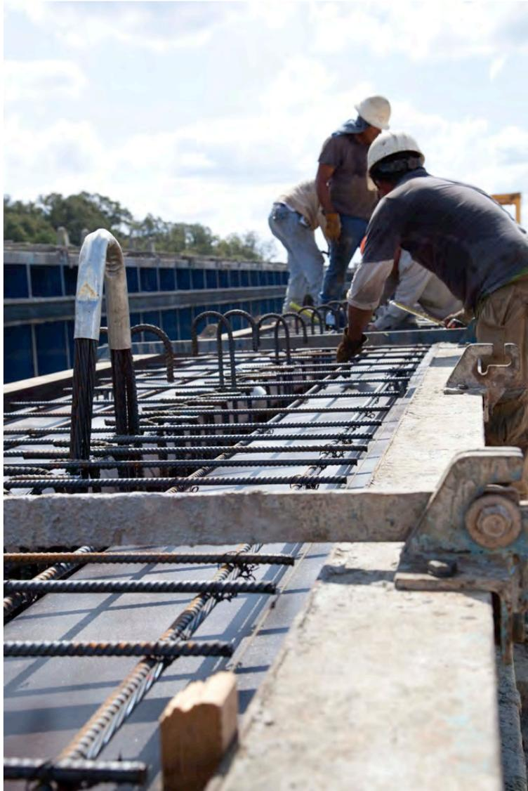
Fig. 2-13. Precasting Florida-I Beams: Showing Top Mat of Reinforcing Steel, Lifting Loop, and Formwork Sides & Bracing
