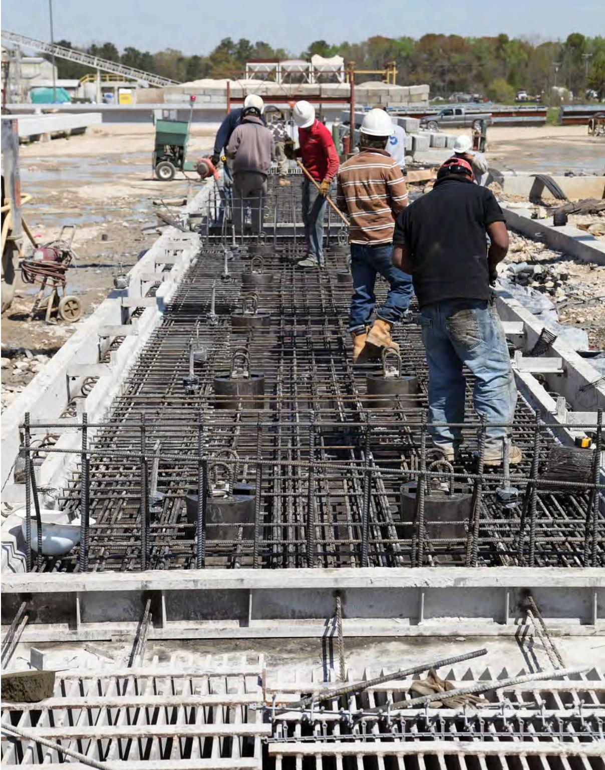
Fig. 5-5. Prestressed Precast Deck Panel Casting Bed, Barrier Reinforcement in Foreground
