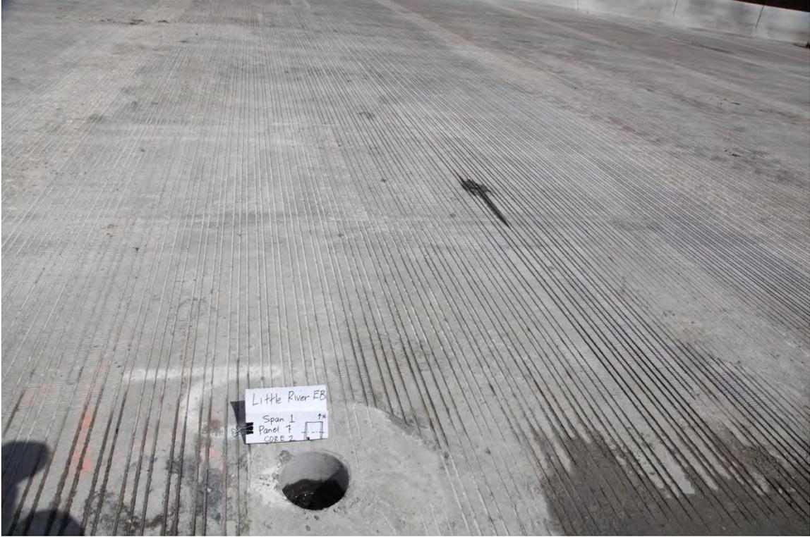
Fig. 6-8. Core 2, Little River EB, Span 1, Panel 7 (Shear Pocket-to-Panel Interface) (3)
