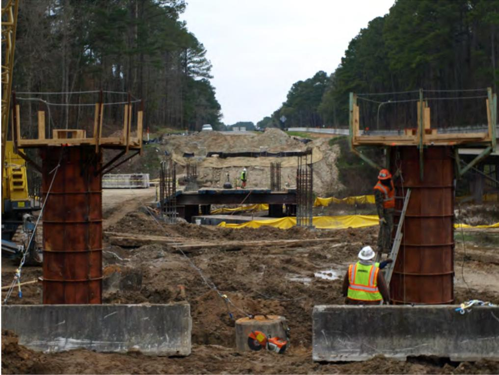
Fig. 2-17. Both Columns for a Little River Bridge Intermediate Bent, Columns for Two Other End Bents In Background
