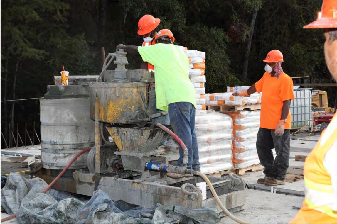
Fig. 4-9. Grout Mixer/Pump and Bags of Grout
