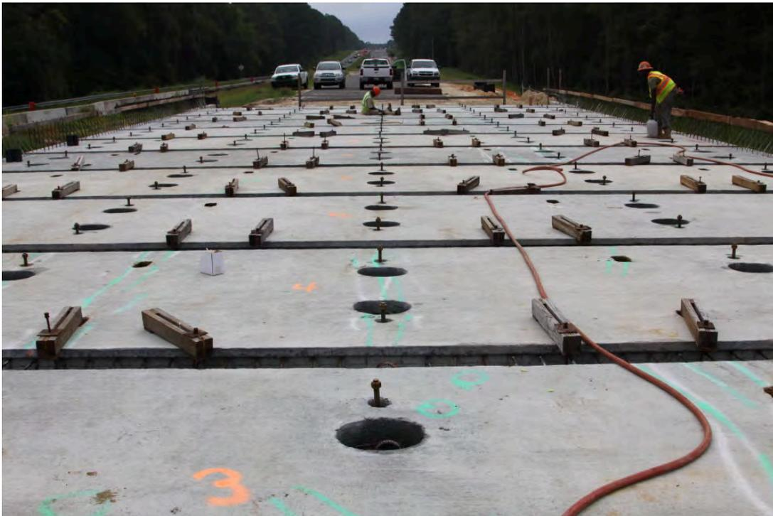
Fig. 4-1. Panels Installed and Getting Ready to Grout Shear Pockets on Hurricane Creek EB
