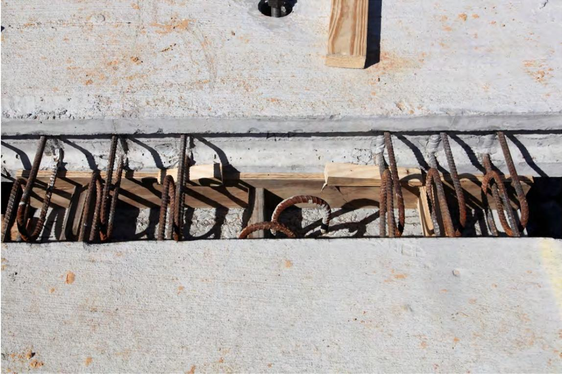
Fig. 3-63. Revised Forming Method to Grout Shear Pockets on Little River EB
