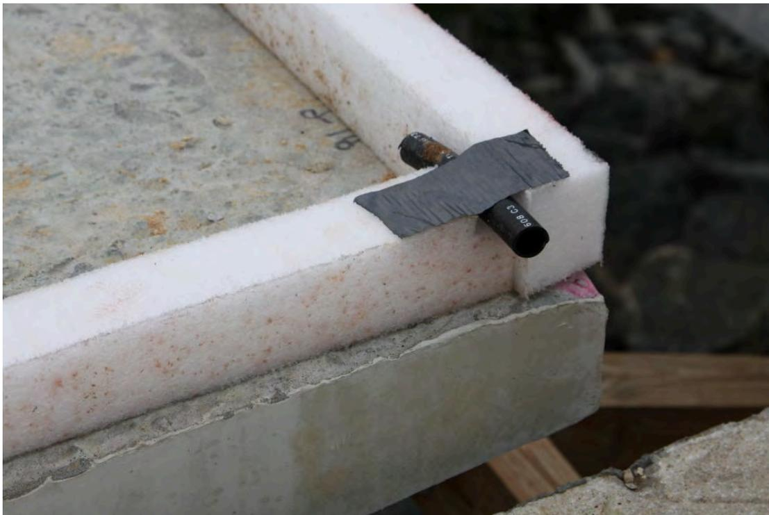
**Fig. 4-16. Grout Port in Polystyrene Forms for Grouting Shear Pockets on Hurricane Creek EB, Before Placing Deck Panel**
