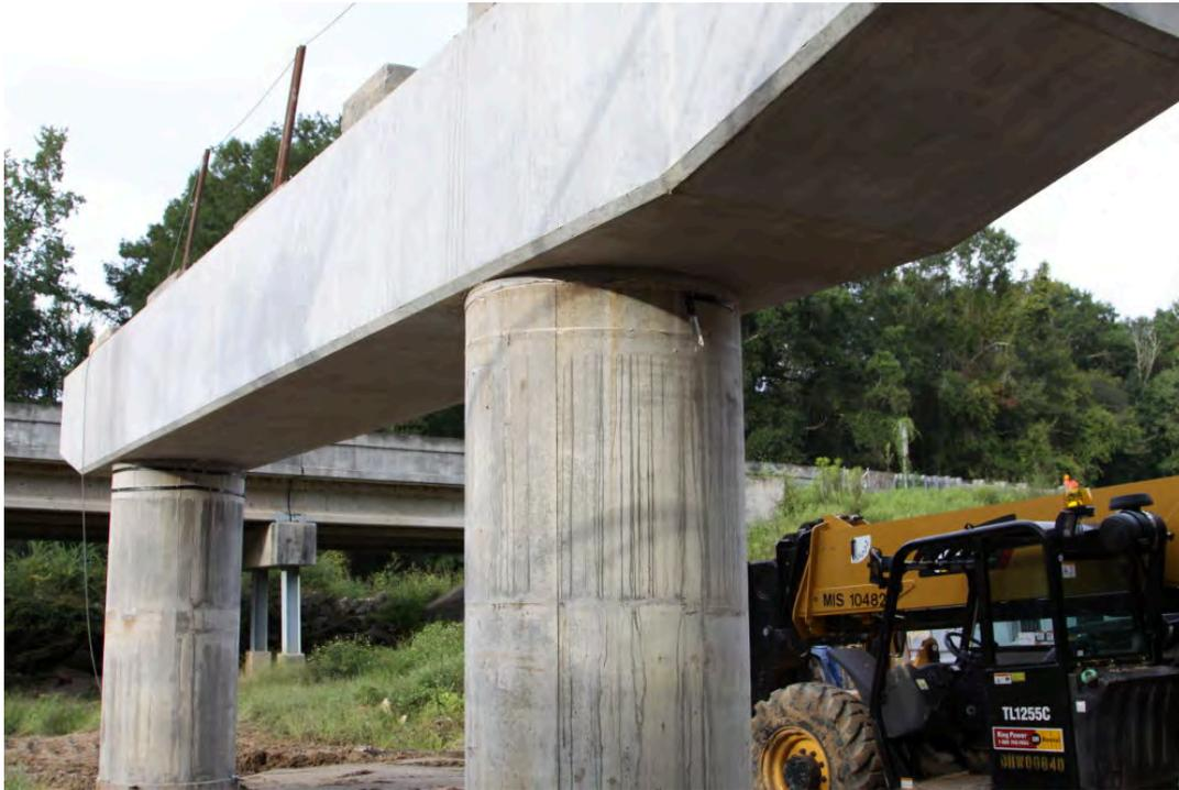
Fig. 2-38. Completed Intermediate Bent for Little River EB (September 18, 2014)
