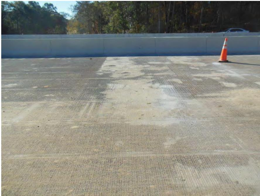
**Fig. 4-53. Deck Surface, Milled and Grooved**
