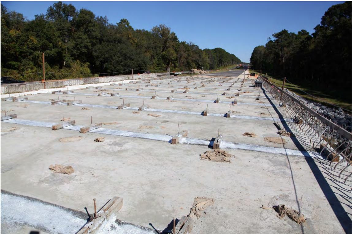
Fig. 4-45. Closure Pours and Curing Compound on Hurricane Creek EB
