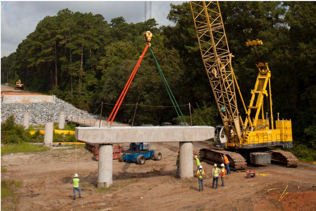
Fig. 1-1. Setting a Precast Bent Cap Using a Two-Point Pick (July 24, 2015)
