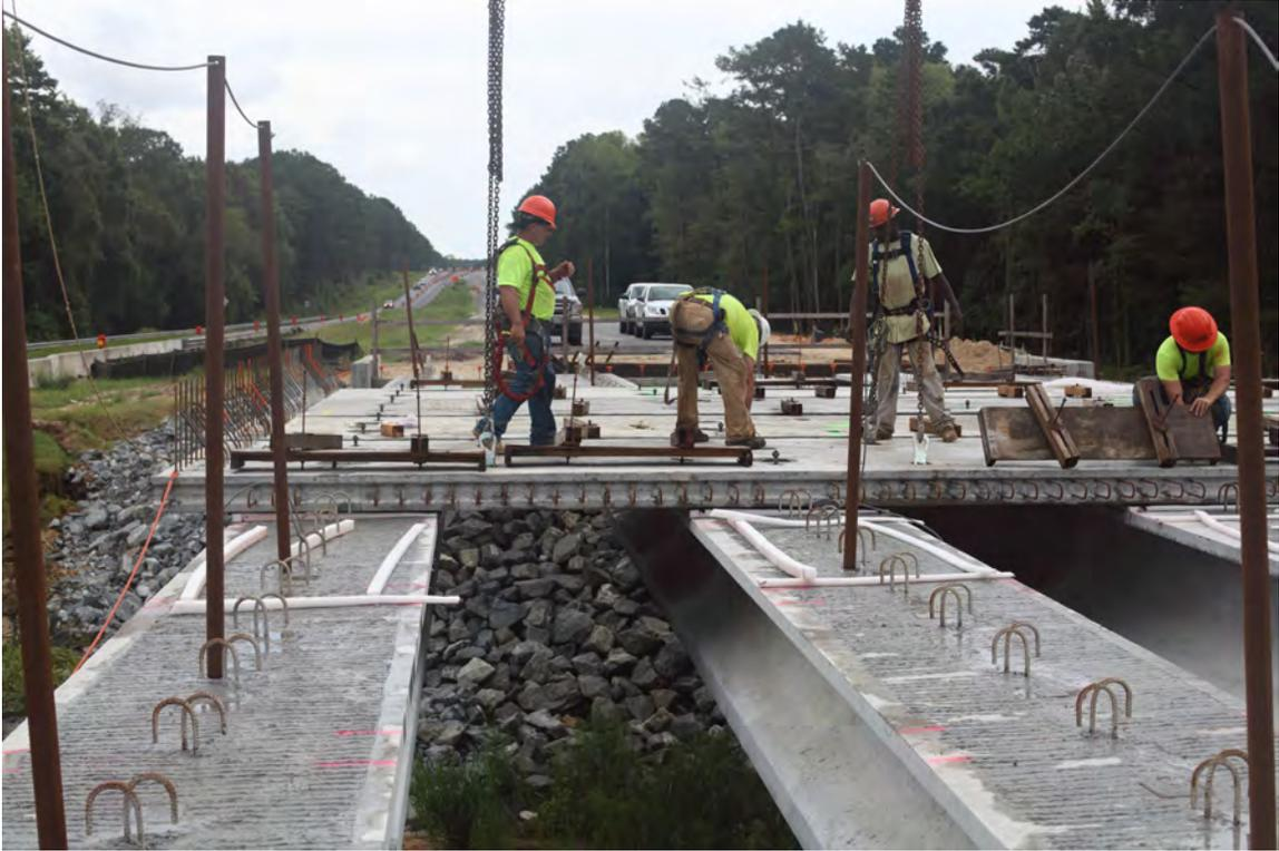
Fig. 2-18. Safety Lines Mounted to FIBs for Erecting Precast Deck Panels
