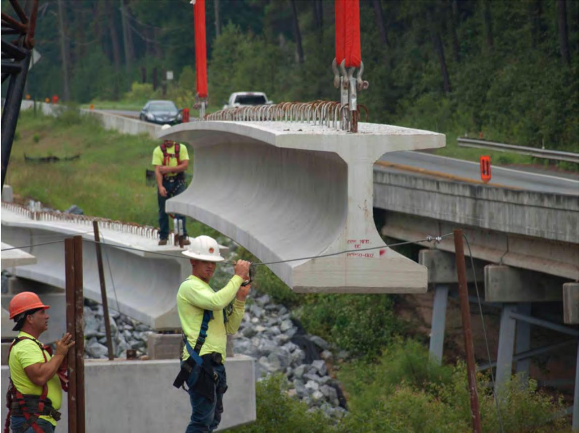
Fig. 3-20. Setting Girder on Little River EB – Camber is Highly Noticeable (September 19, 2014)
