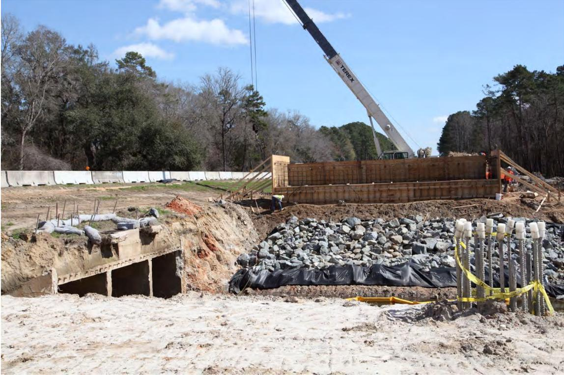
Fig. 2-6. Hurricane Creek EB – Looking East at Formwork for End Bent (February 19, 2014)
