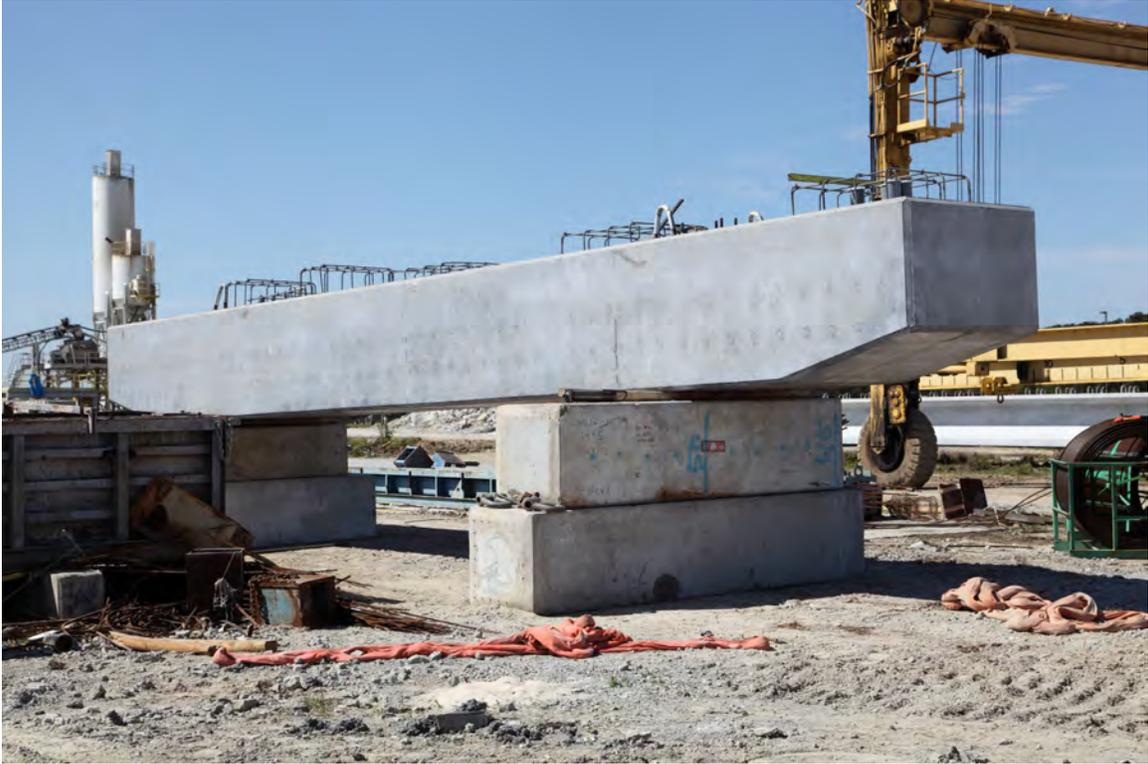
**Fig. 6-24. Precast Bent Cap Removed from Forms**
