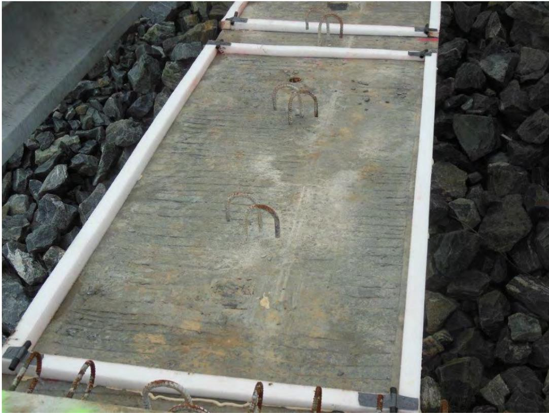
Fig. 3-51. Close-up of Polystyrene Forms
