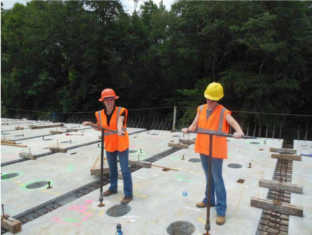
**Fig. 3-46. Adjusting Leveling Bolts to Raise/Lower Deck Panels**
