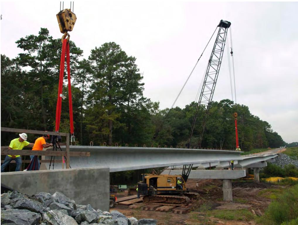
Fig. 3-17. Setting Girder on Little River EB – Side View (September 20, 2014)
