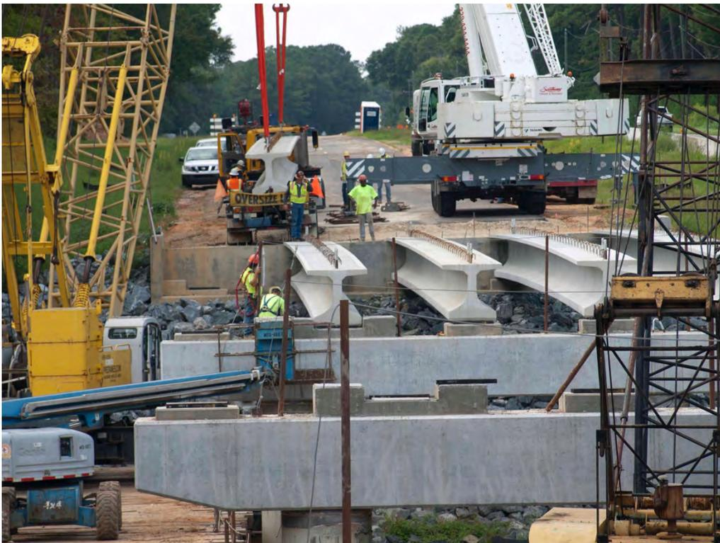
Fig. 3-15. Equipment for Setting Girders on Little River EB (September 18, 2014)
