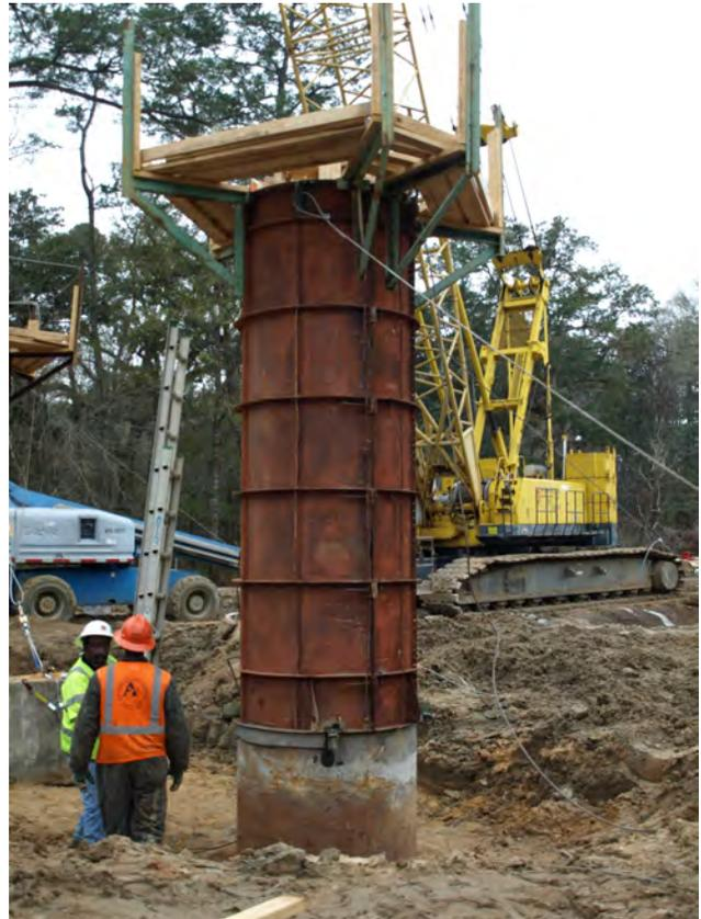
Fig. 2-16. Column Extending from Drilled Shaft for Little River Bridge Intermediate Bent
