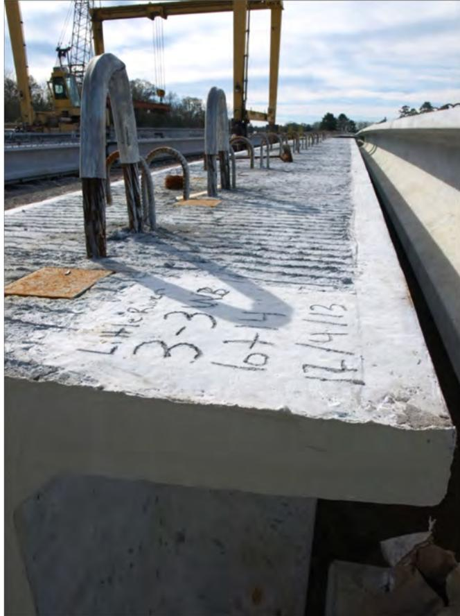
Fig. 3-56. Edge of Girder Top Flange Was Smoothed Longitudinally During Precasting
