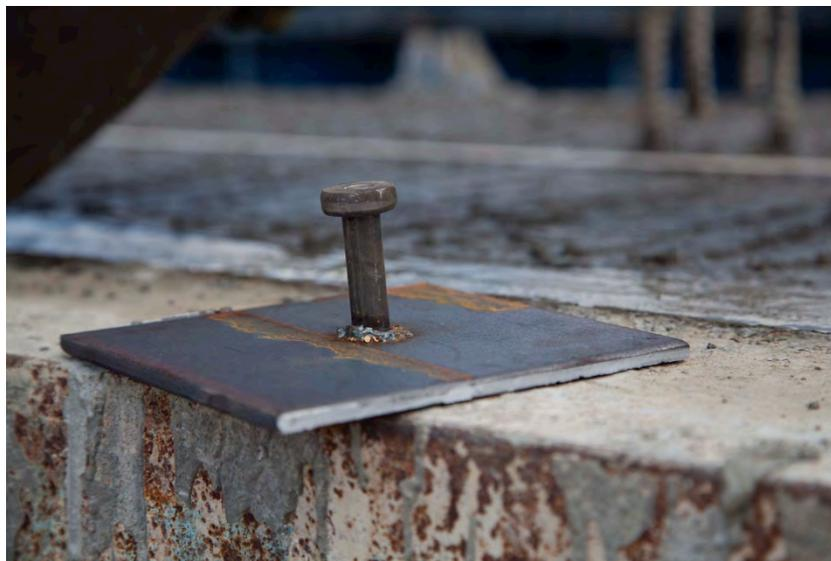
Fig. 2-15. Precasting Florida-I Beams: Close-up of Embedded Plate C Assembly Before Being Placed in Top of FIB
