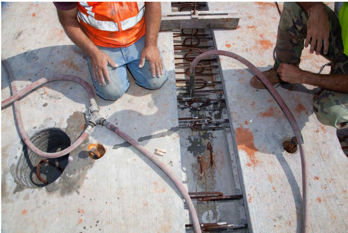
Fig. 4-22. Feeding Grout into Pipes for Shear Pockets on Hurricane Creek WB
