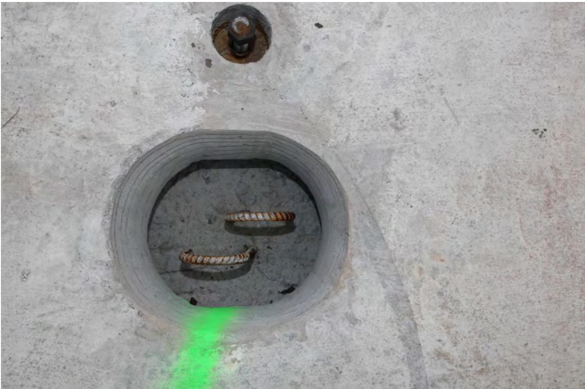
Fig. 4-3. Shear Pocket Without Additional #4 Bars on Little River EB
