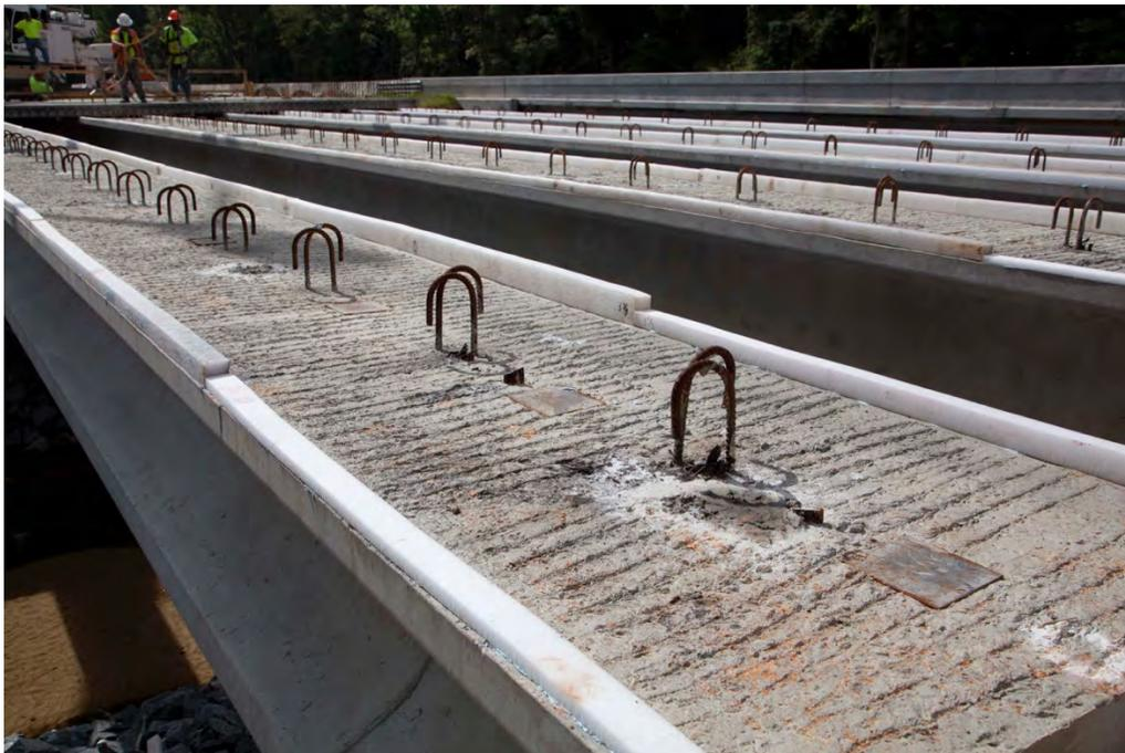
**Fig. 3-55. Polystyrene Forms Placed Along Entire Girder Length on Hurricane Creek WB**
