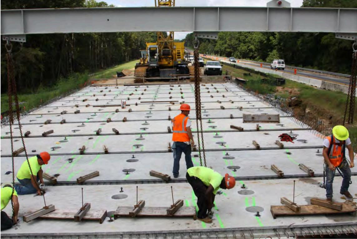
Fig. 3-40. Setting Precast Deck Panels on Hurricane Creek EB (September 9, 2014)
