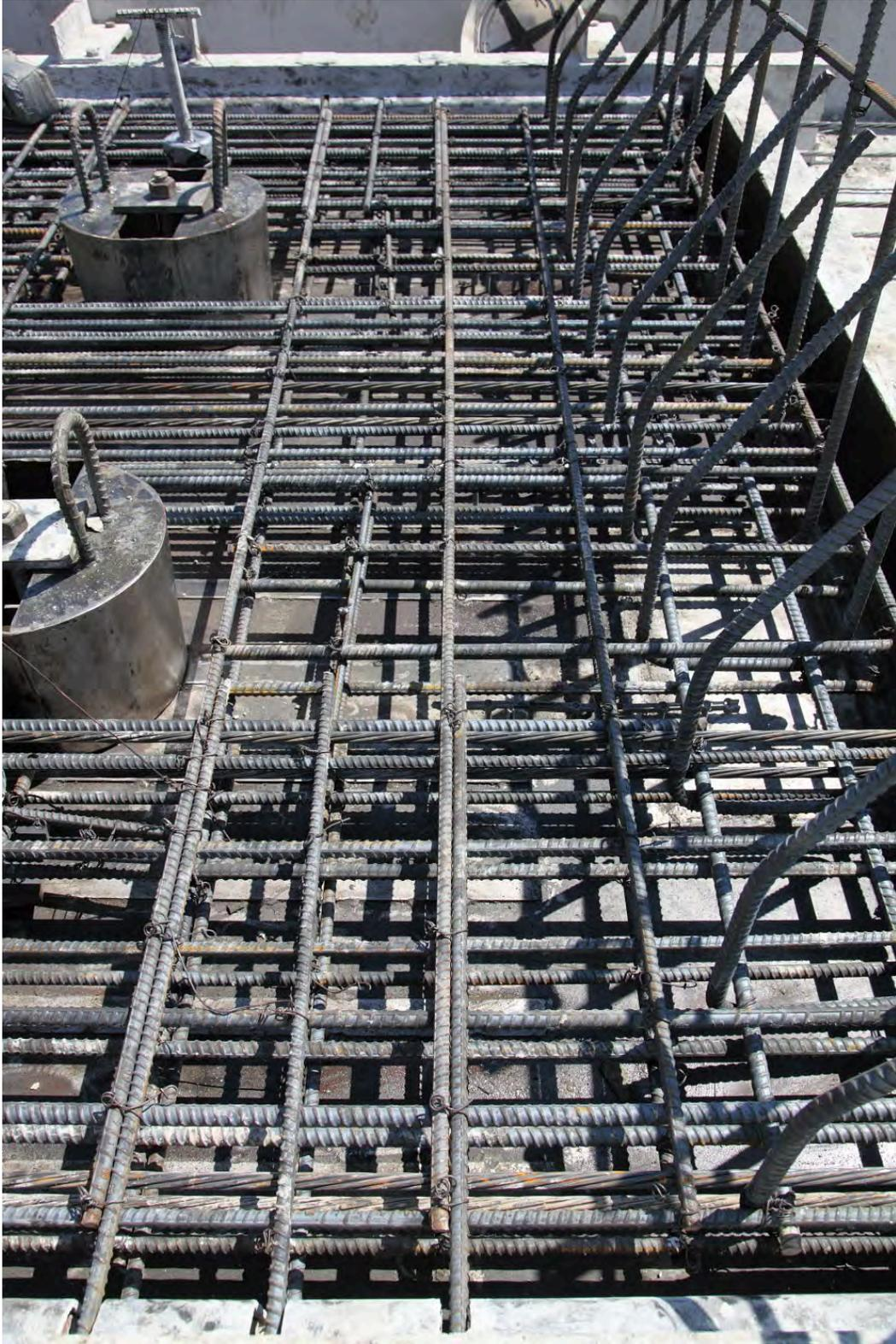
Fig. 5-11. Prestressed Precast Deck Panel, Reinforcement in Vicinity of Future Barrier
