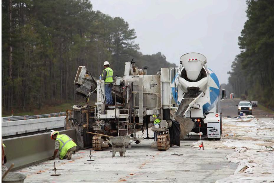
Fig. 4-49. Slip Forming Barriers on Little River WB – Slip Former and Concrete Truck
