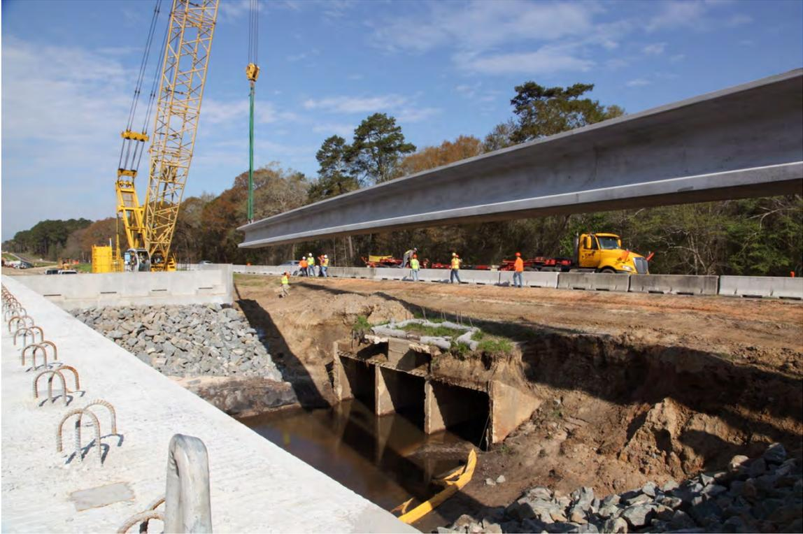
Fig. 3-6. Installing Girder on Hurricane Creek EB Bridge (March 24, 2014)
