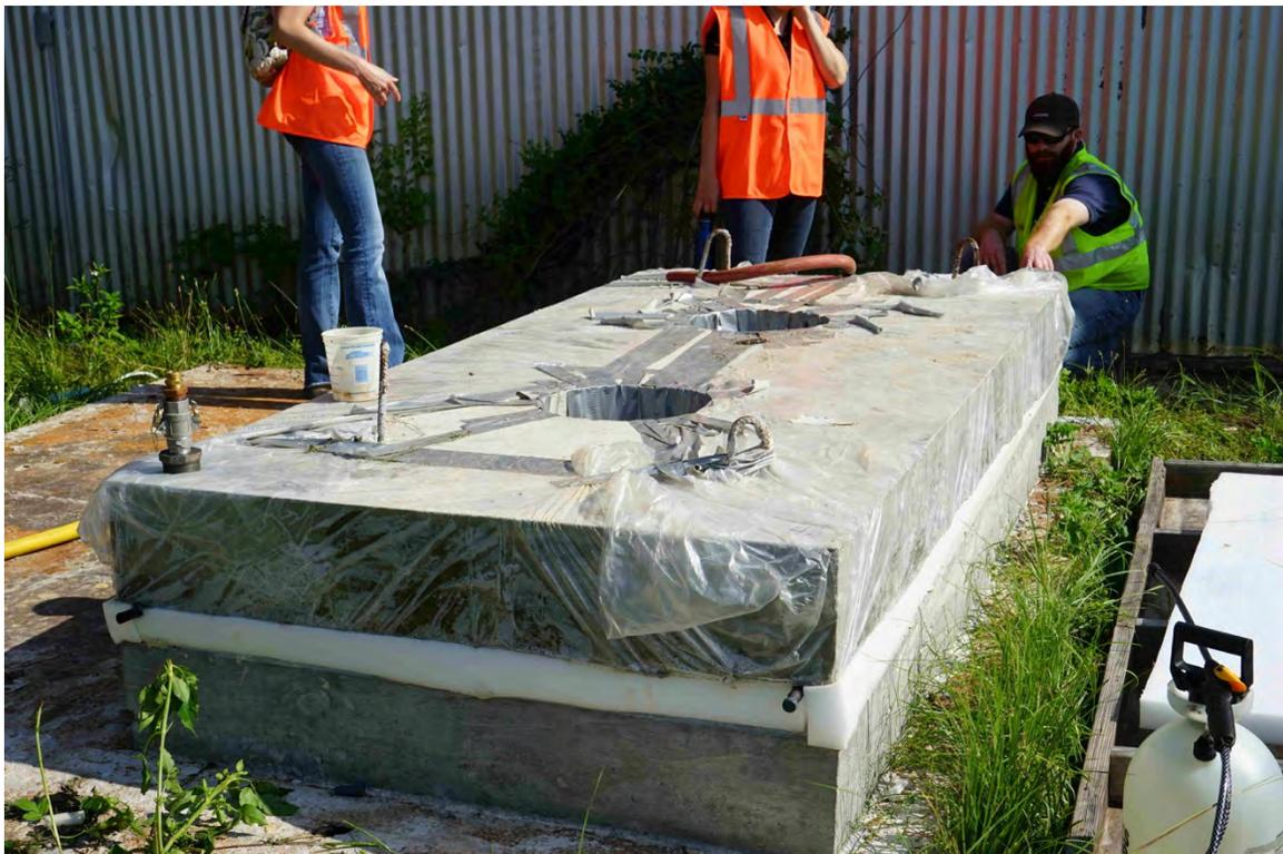
Fig. 5-14. Grout Mock-up for Precast Deck Panel, "Panel" and "FIB" in Place, with Polyethylene Forming the "Haunch"
