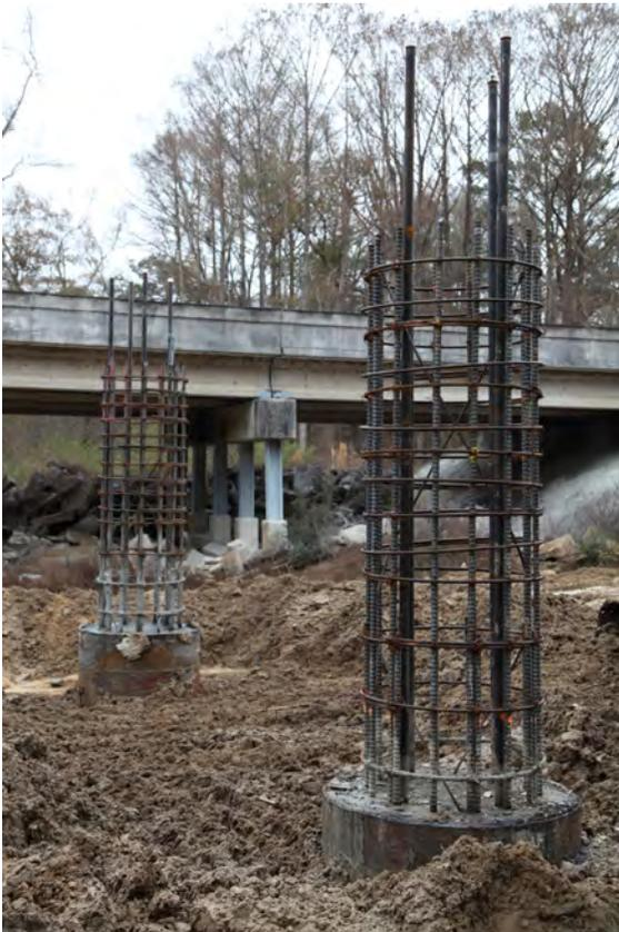
Fig. 2-15. Reinforcement Extending from Drilled Shafts for Connection to Columns for Little River Bridge Intermediate Bent
