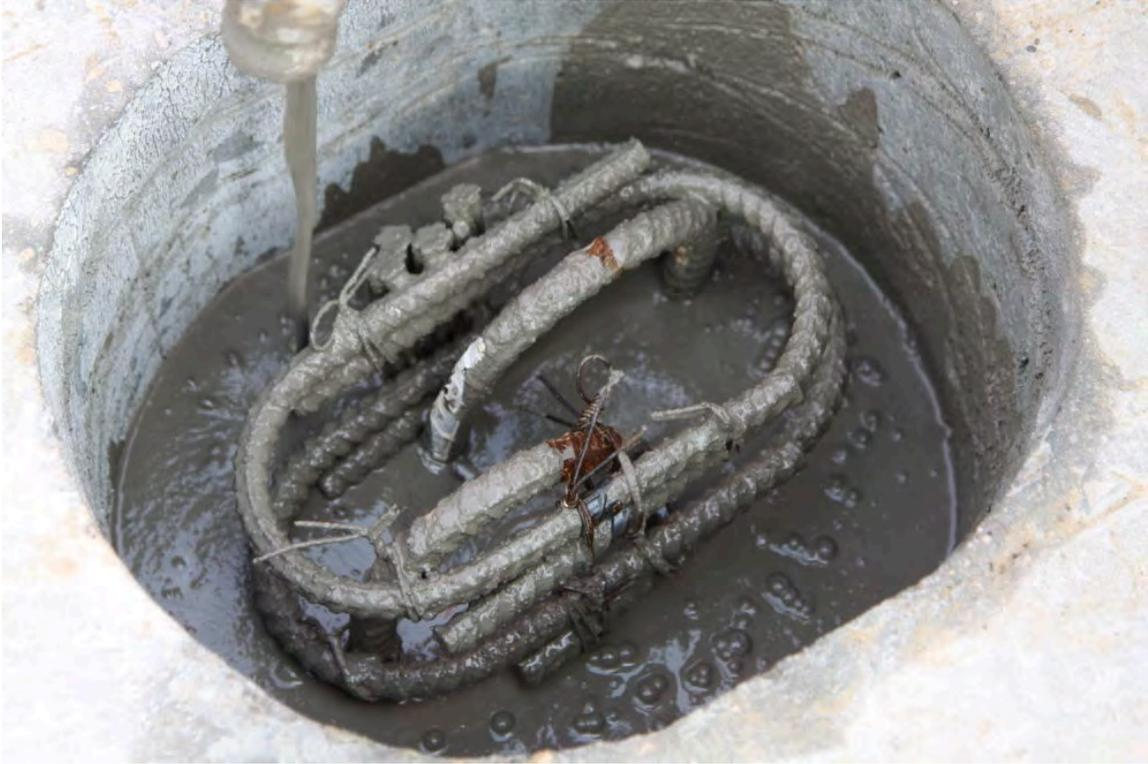
Fig. 4-23. Placing Grout Directly into a Shear on Hurricane Creek EB
