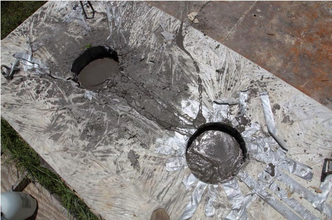
Fig. 5-18. Grout Mock-up for Precast Deck Panel, Grouting Completed, Top View of Panel
