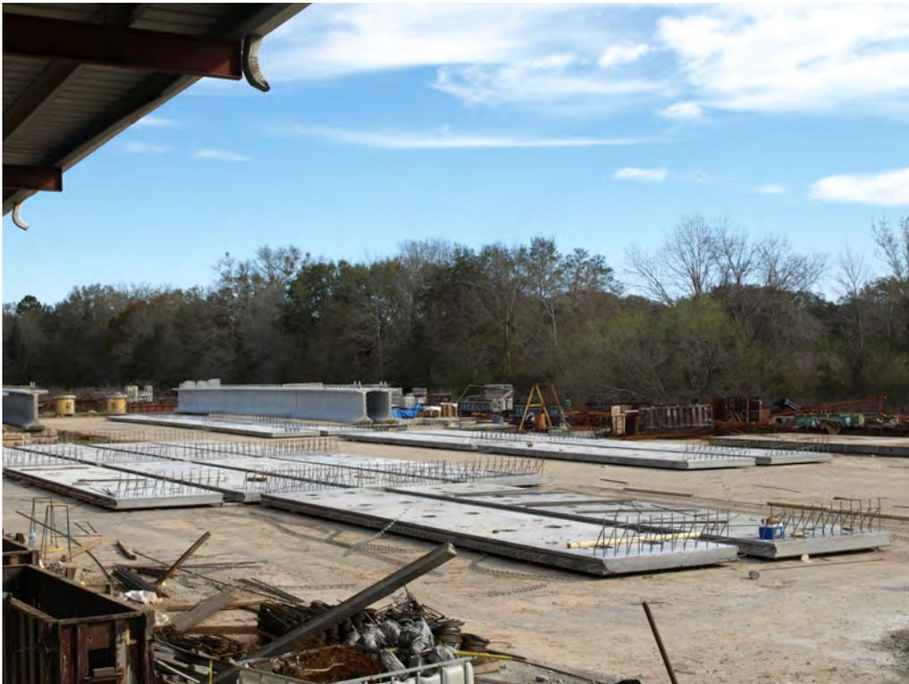
Fig. 4-7. Storage of Non-prestressed Precast Deck Panels in Casting Yard
