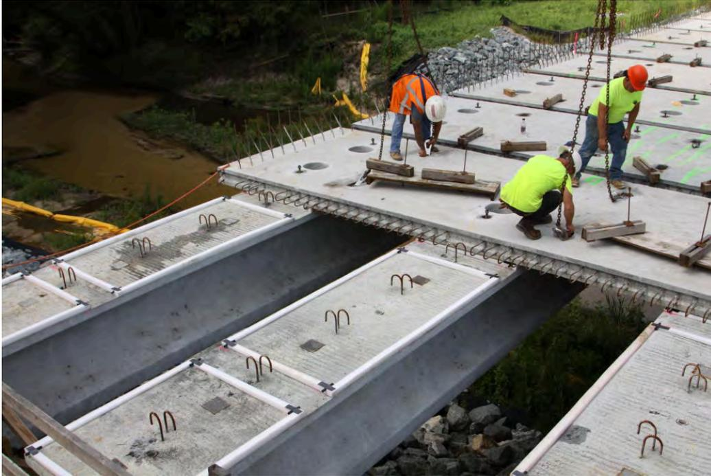
**Fig. 3-54. Setting Precast Deck Panels on Hurricane Creek EB (September 9, 2014)**
