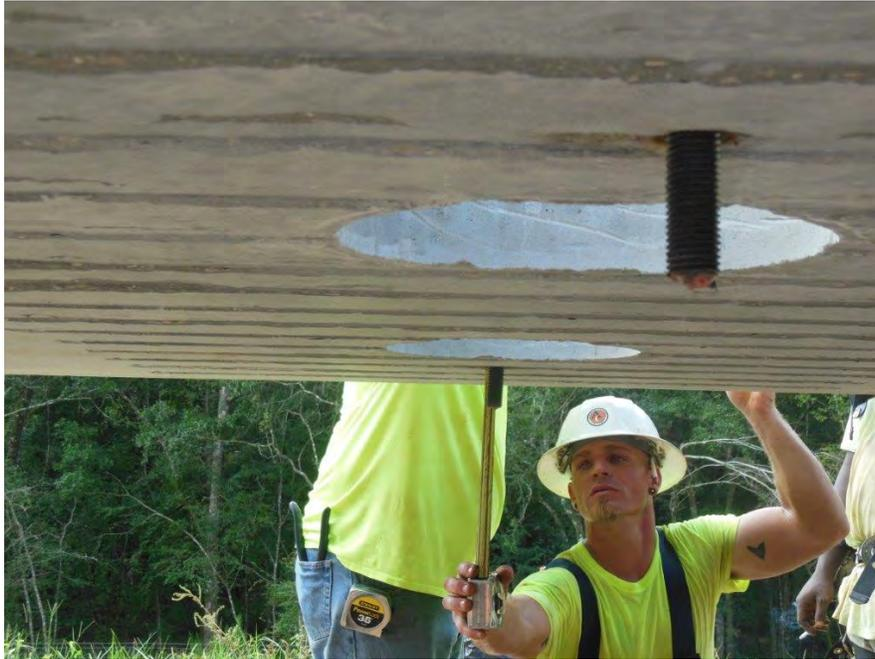
**Fig. 3-31. Measuring Leveling Bolt Extension for Adjustment**
