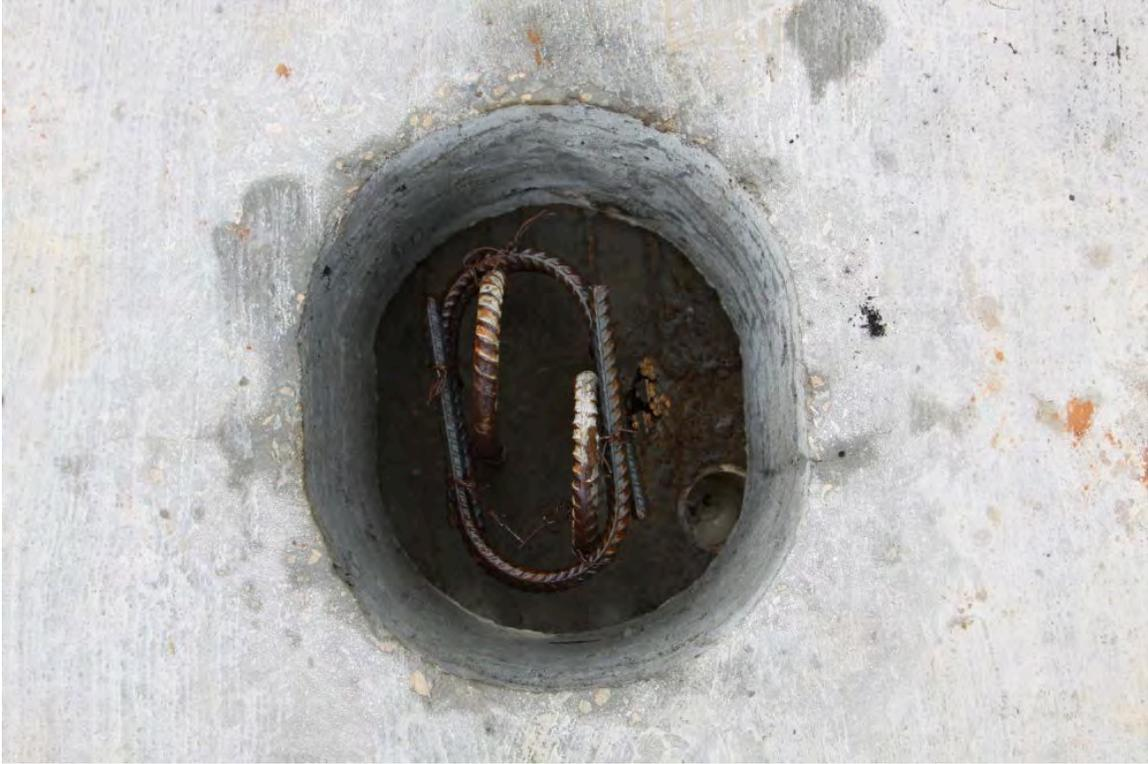
Fig. 4-2. Additional #4 Bars Wrapped Around the "J" Bars to Fortify Connection to the FIB – Hurricane Creek EB
