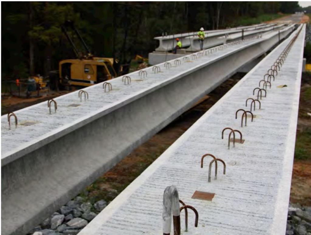
Fig. 2-17. Florida-I Beams Erected on Little River EB Bridge
