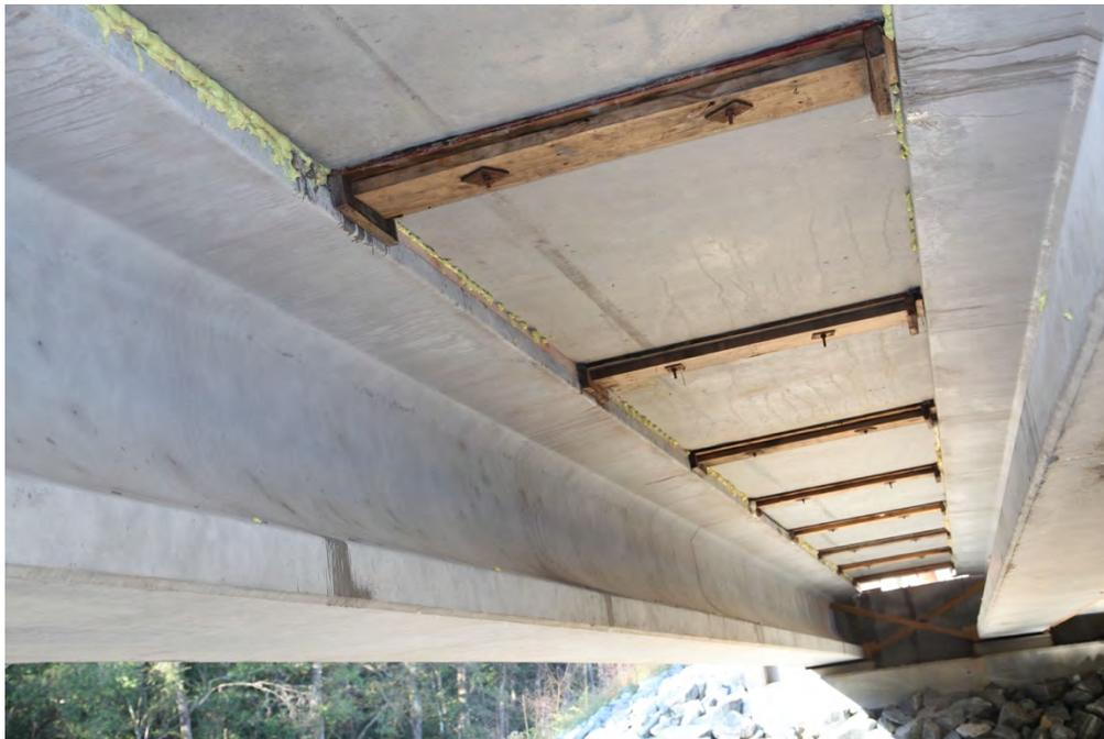
Fig. 4-37. Closure joint Forms, View from Underneath Hurricane Creek EB
