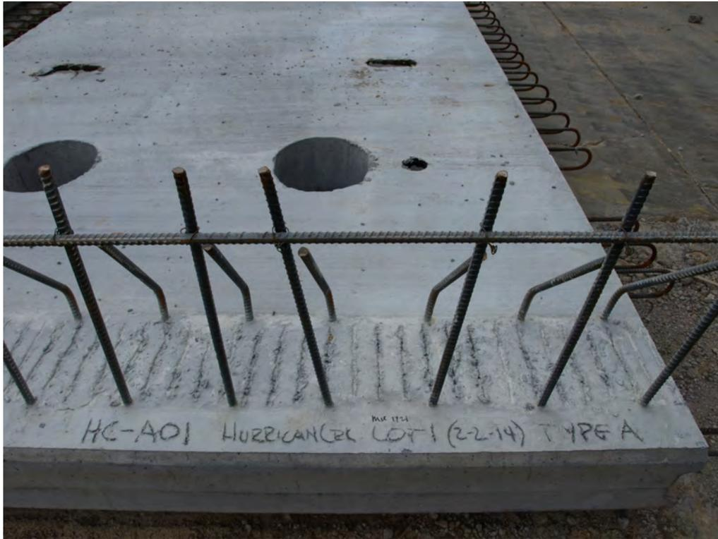
**Fig. 4-10. Designations Marked on Precast Panel**
