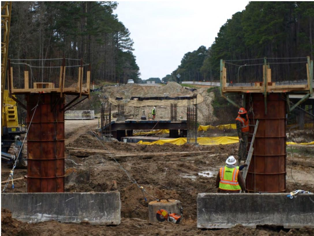
**Fig. 2-10. Both Columns Formed for Little River EB Intermediate Bent (February 6, 2014)**
