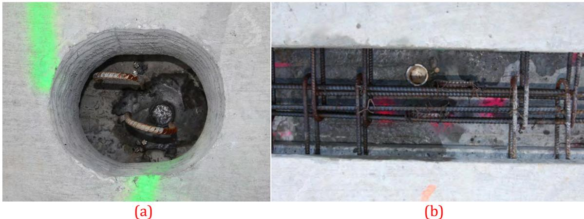
**Fig. 2-24. Top View of Circular Sleeves Embedded in FIBs for Fall Protection. (a) Grouted Sleeve Below Precast Deck Panel Shear Pocket, (b) UngROUTED Sleeve Below Panel Closure Joint.**
