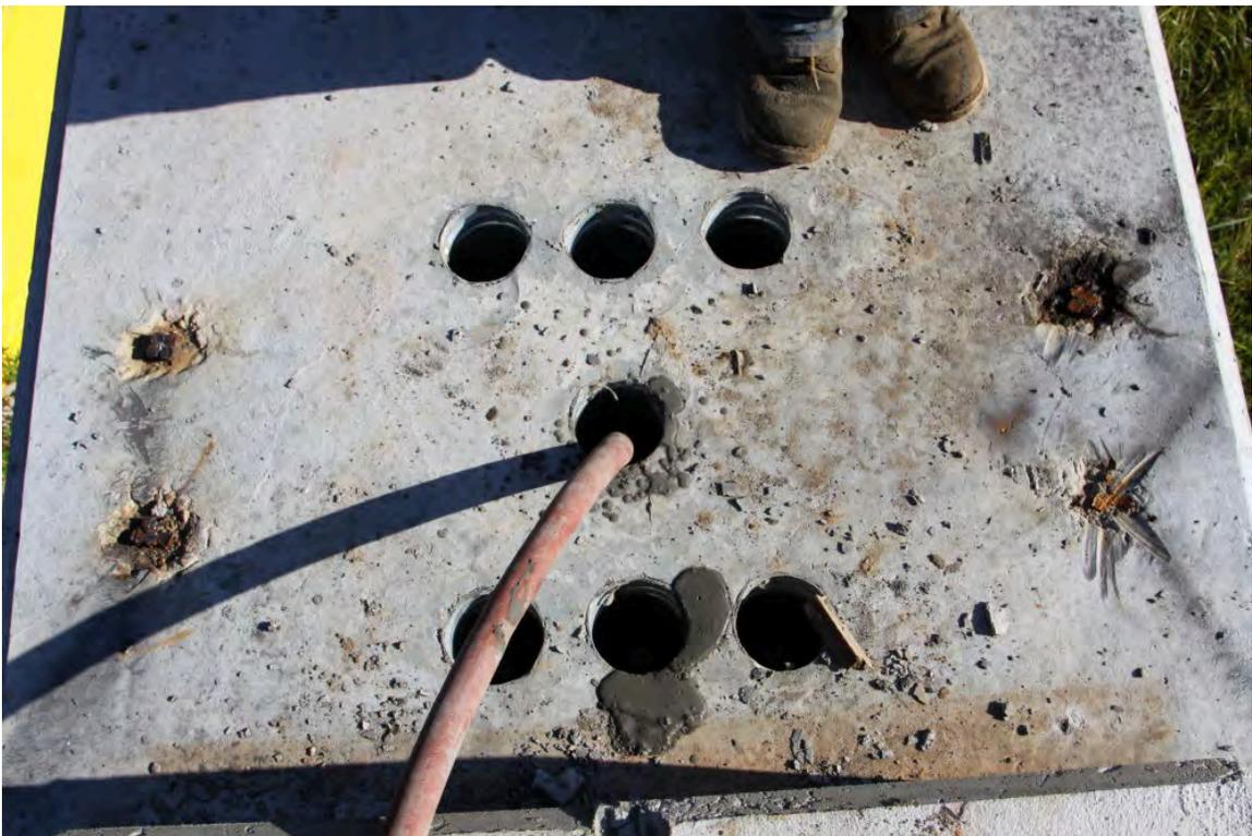
Fig. 2-33. Grouting Bent Caps on Little River EB, Filling in 7th Hole (September 14, 2014)
