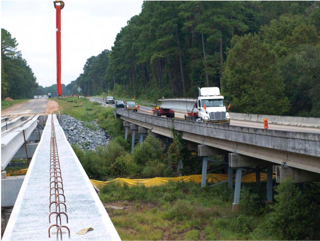
Fig. 3-10. Girder Being Delivered by Truck to Little River EB (September 20, 2014)
