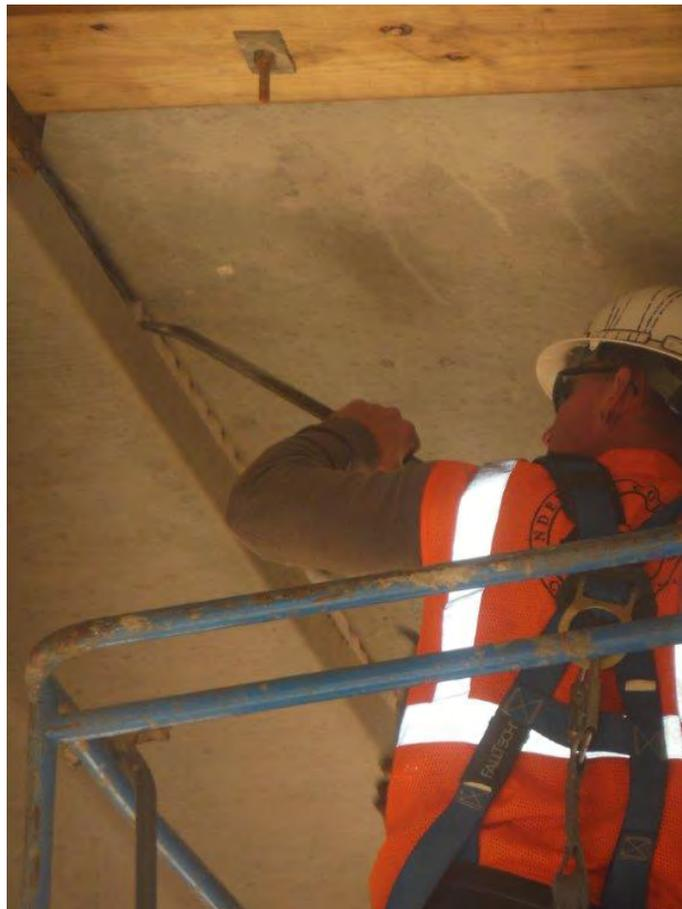
Fig. 3-59. Removing Polyethylene Forms from Haunch
