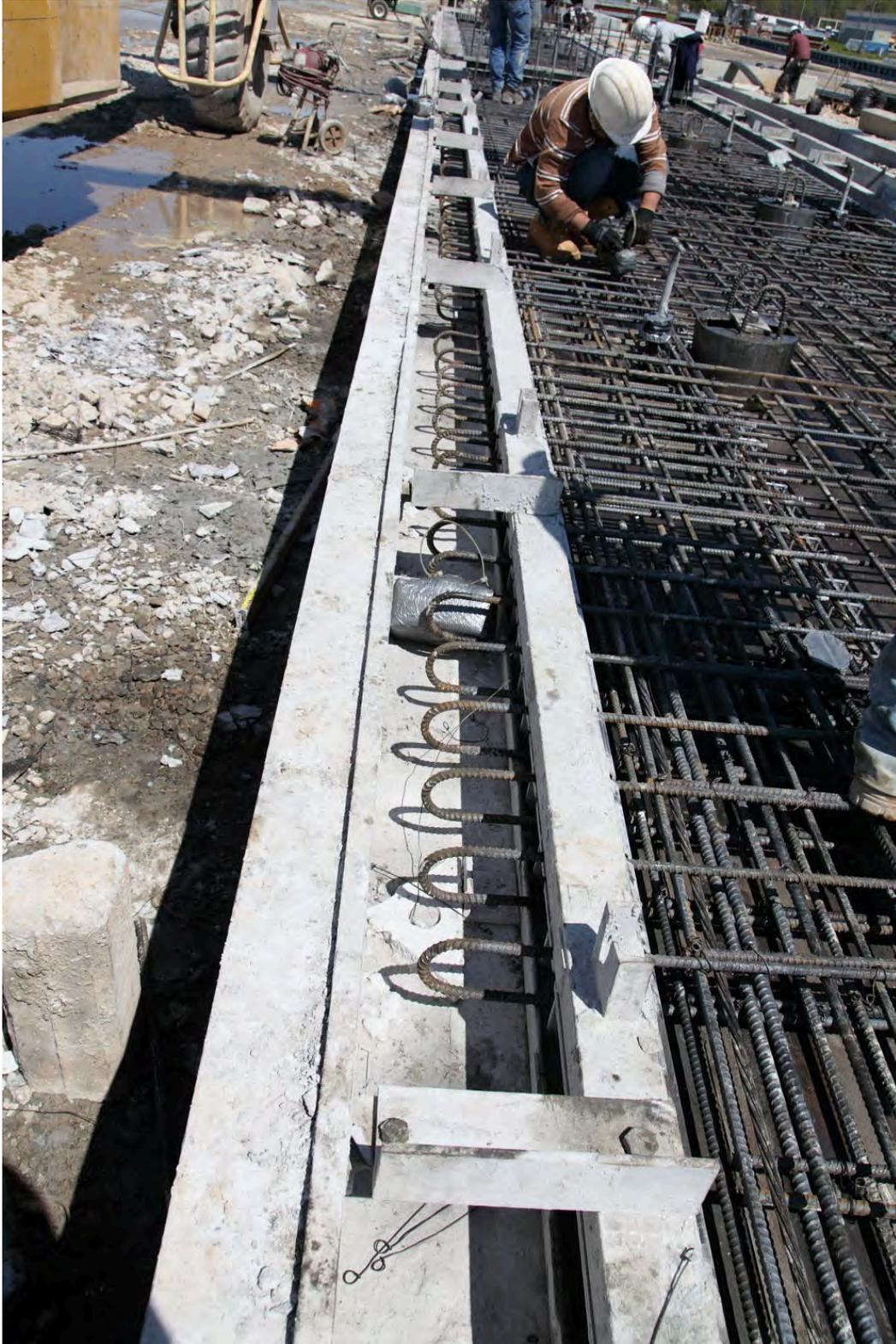
Fig. 5-9. Prestressed Precast Deck Panel, Reinforcing Steel Along Long Edge
