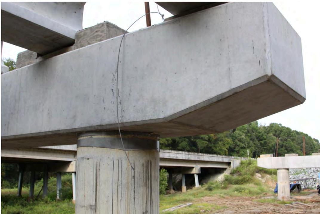
Fig. 2-39. FIBs Set on Little River EB Bent Cap, Some Sealant is Visible at Top of Column (September 18, 2014)
