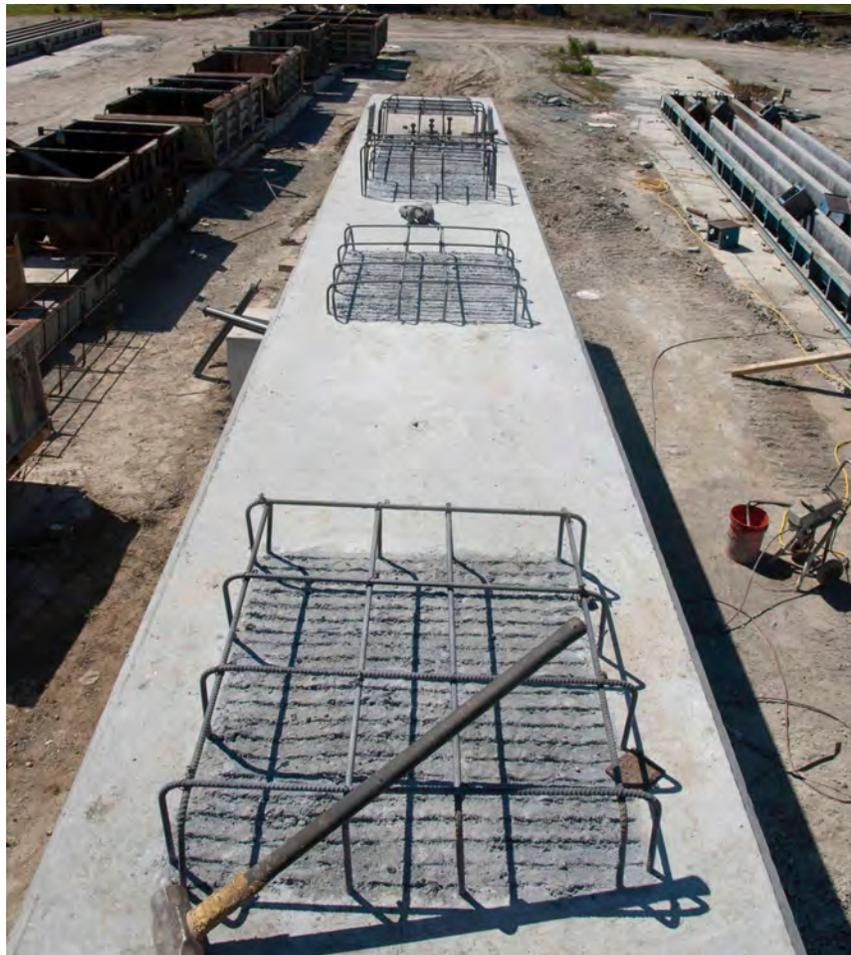
Fig. 6-21. Precast Bent Cap, Reinforcing Steel for Cast-in-Place Bearing Pad Pedestals
