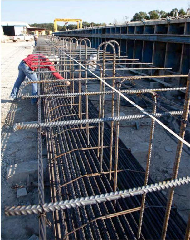
Fig. 2-5. Precasting Florida-I Beams: Close-up of Bars 4M, 5Z and 5J, Strands N
