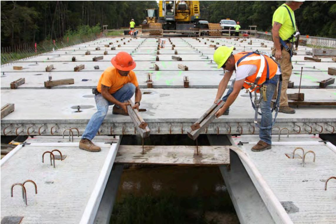
**Fig. 4-35. Positioning Closure Joint Forms on Hurricane Creek EB as Panels Were Placed**
