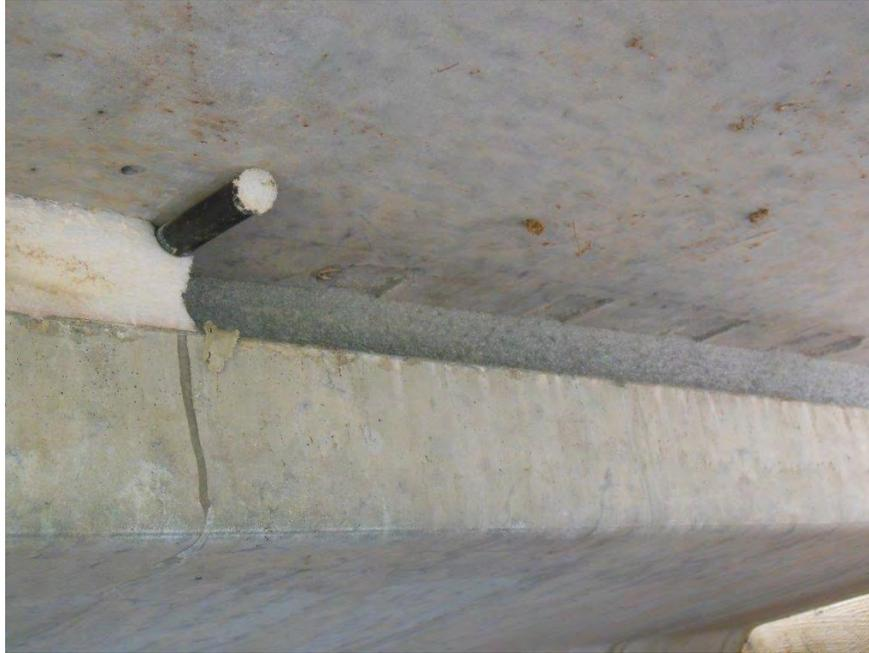
Fig. 3-60. Polyethylene Forms Removed from Haunch (to the Right of the Grout Port Left Behind)
