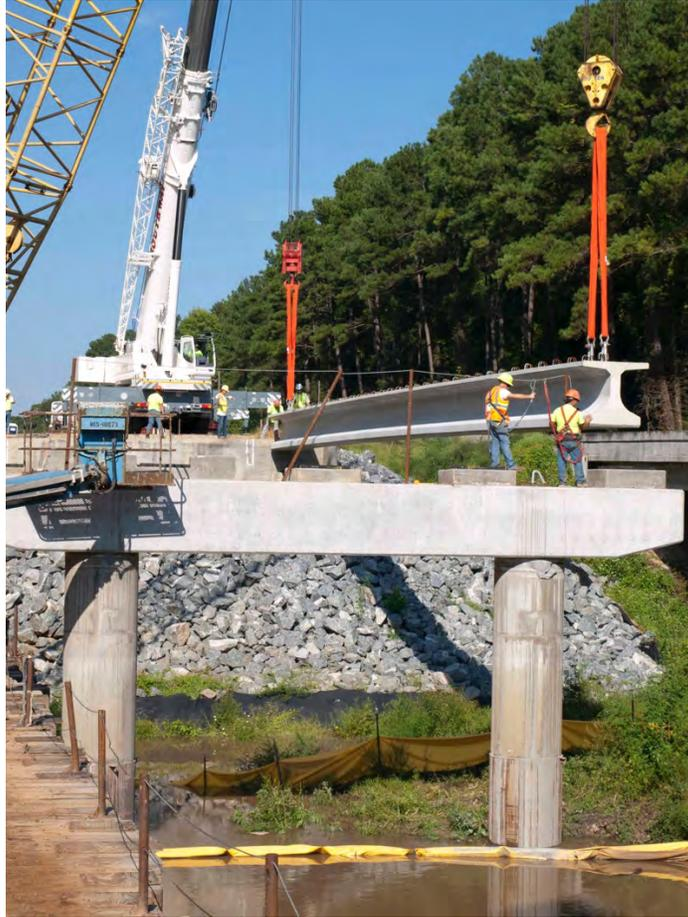
Fig. 3-12. Setting Girder on Little River EB (September 18, 2014)
