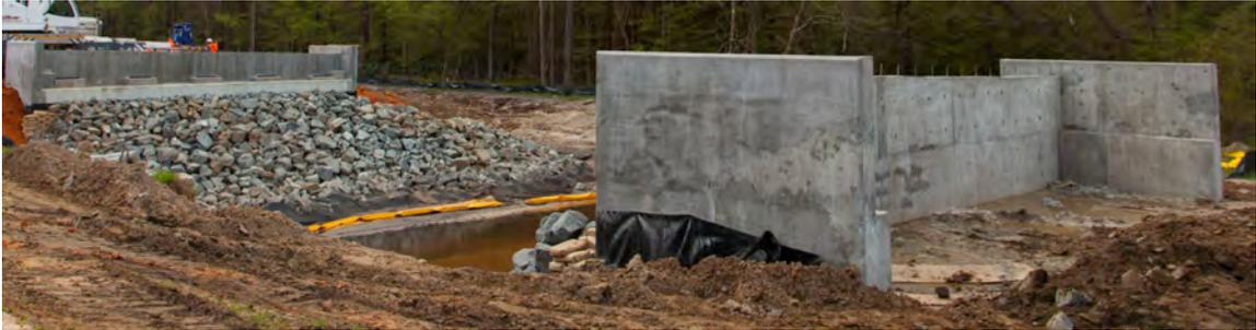
Fig. 2-14. End Bents on Both Ends of Hurricane Creek EB Bridge
