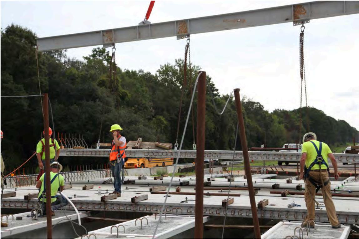
Fig. 3-36. Setting Precast Deck Panels on Hurricane Creek EB (September 8, 2014)
