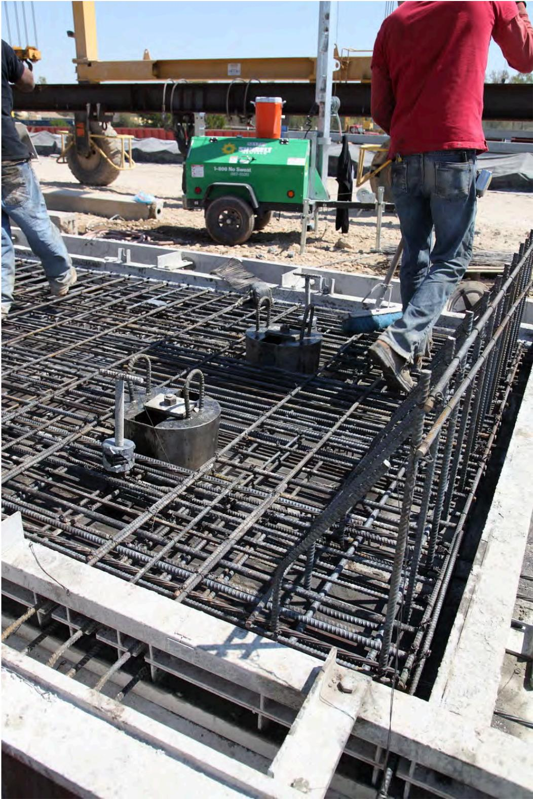
Fig. 5-10. Prestressed Precast Deck Panel, Reinforcing Steel Along Short Edge
