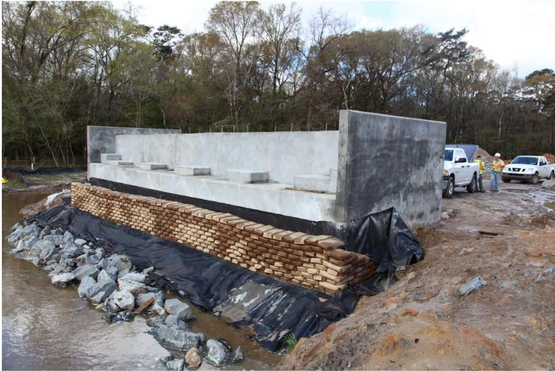
Fig. 2-8. Hurricane Creek EB – Completed End Bent on West (March 18, 2014)
