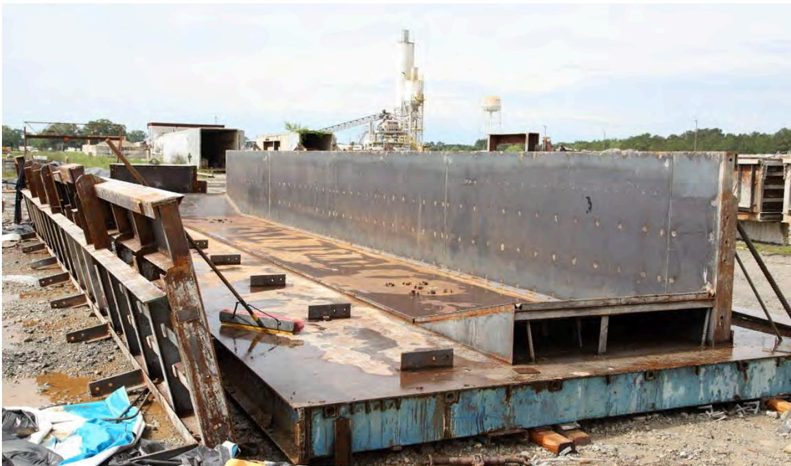
Fig. 6-5. Precast Bent Cap Forms, with Left Side Not Yet Installed
