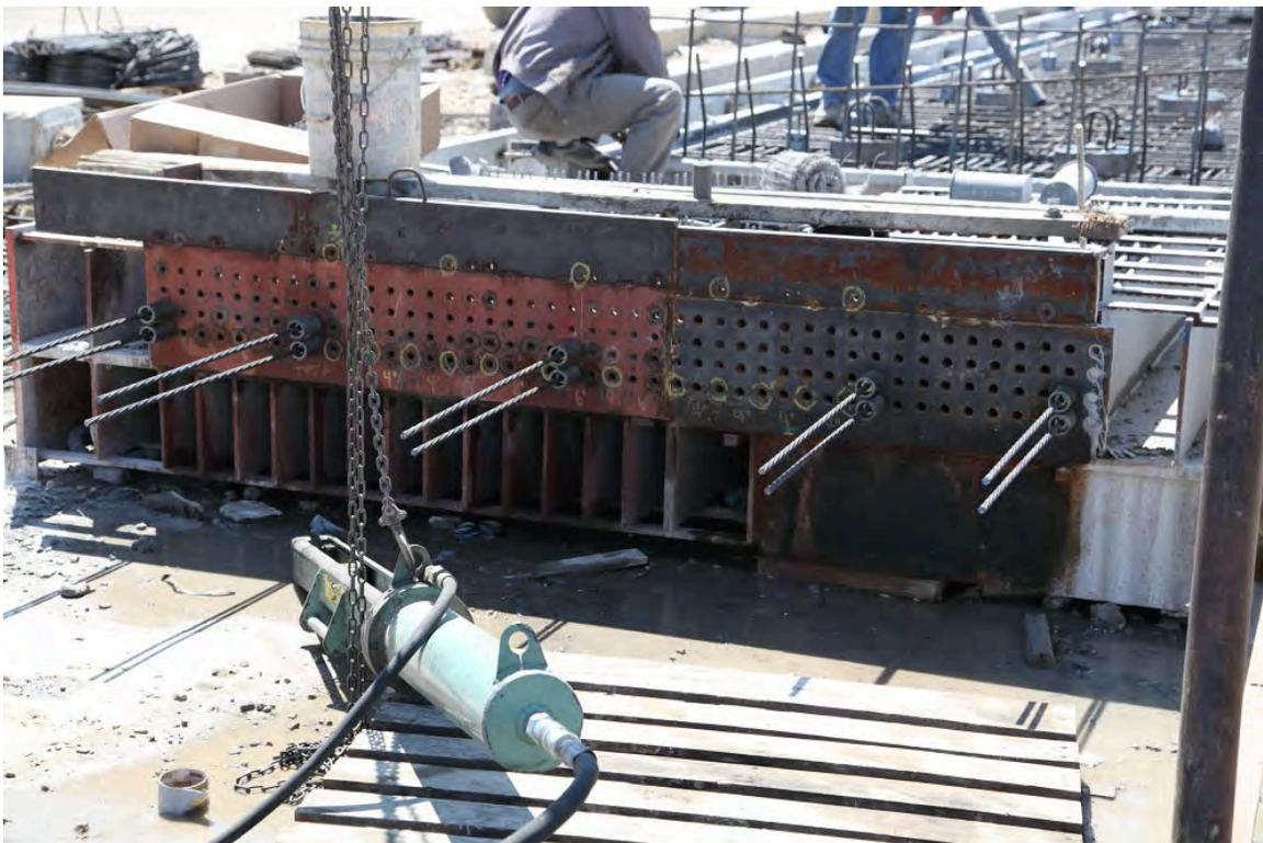
Fig. 5-7. Prestressed Precast Deck Panel Casting Bed, Stressing End and Strand Pattern
