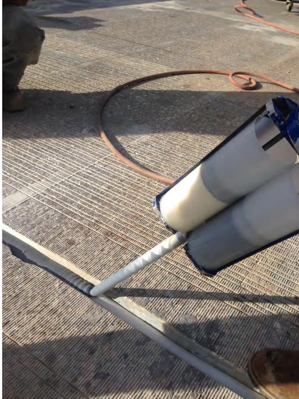
Fig. 4-56. Filling Expansion Joint with Sealant
