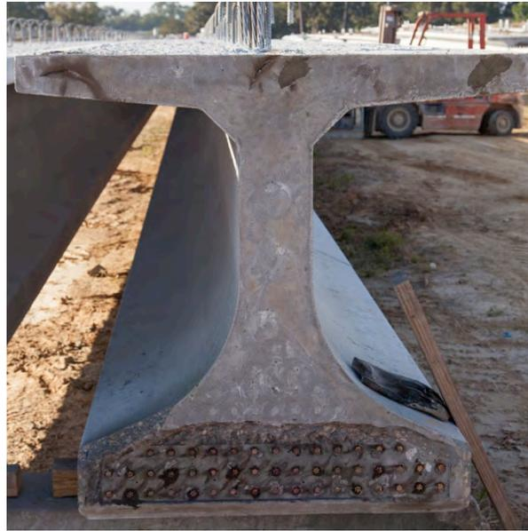
Fig. 2-8. Photo of Florida-I Beam in the Casting Yard
