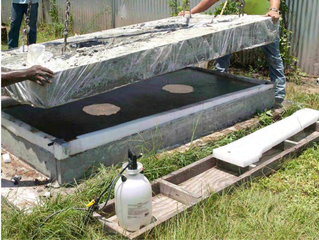
Fig. 5-13. Grout Mock-up for Precast Deck Panel, "Panel" Being Lowered onto "FIB"
