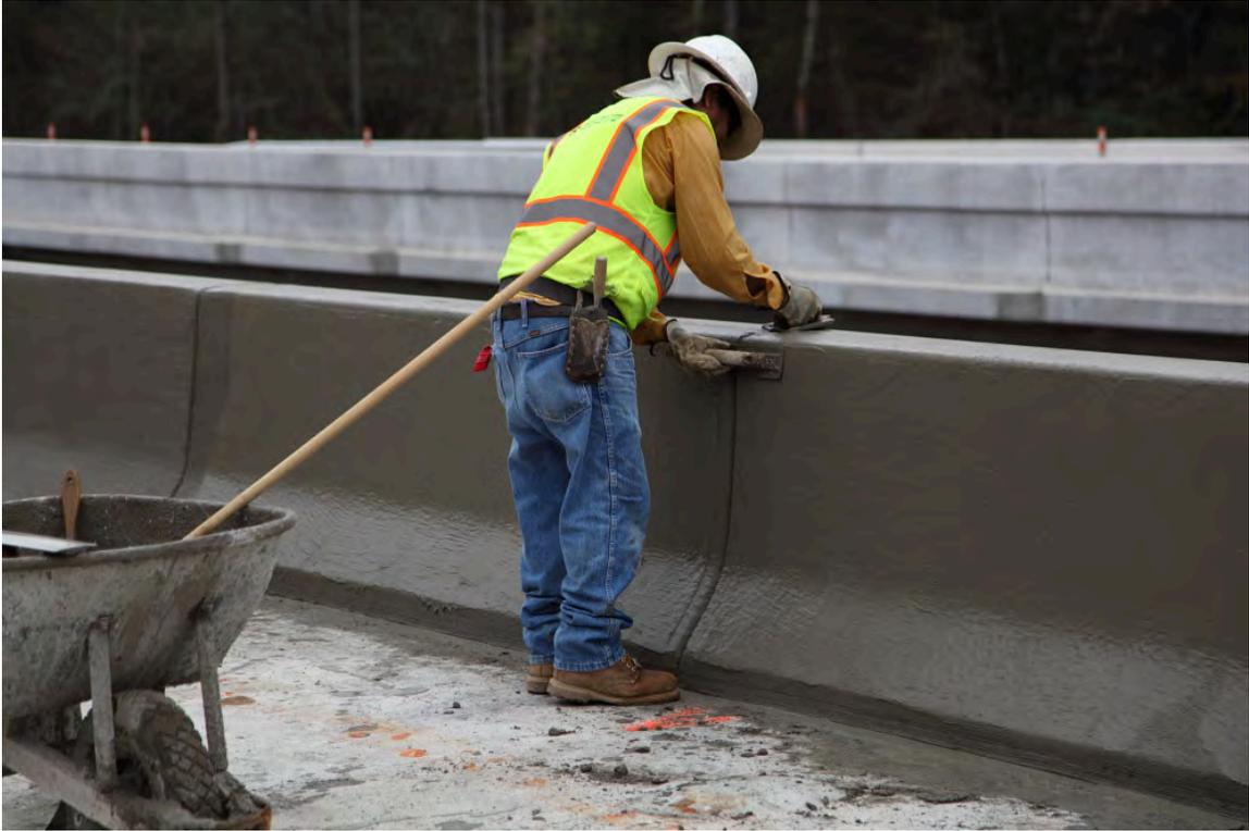
Fig. 4-51. Finishing Barriers on Little River WB
