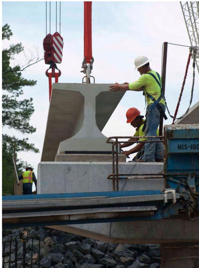
Fig. 3-19. Setting Girder on Bearing – Little River EB (September 18, 2014)
