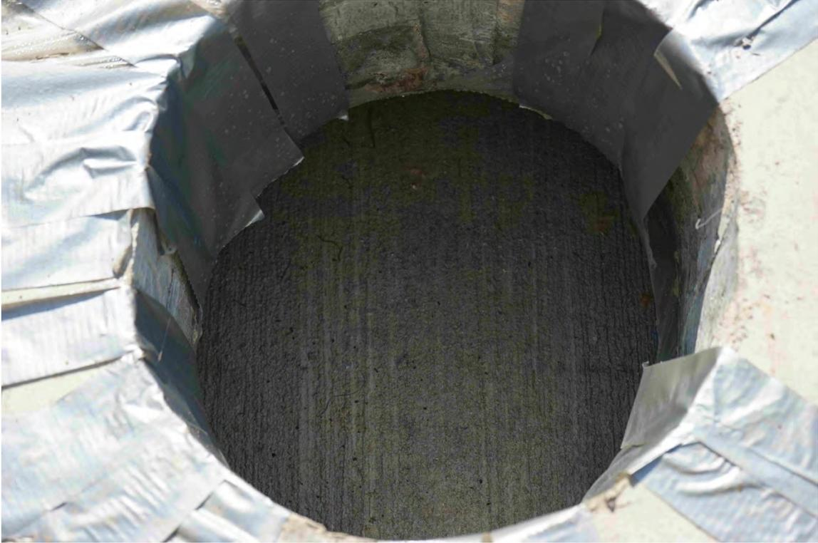
Fig. 5-15. Grout Mock-up for Precast Deck Panel, Shear Pocket in "Panel"
