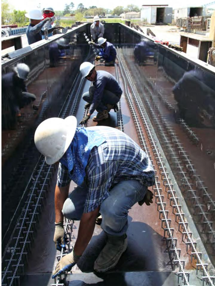
Fig. 6-7. Precast Bent Cap Forms, Getting Ready to Set Reinforcing Steel
