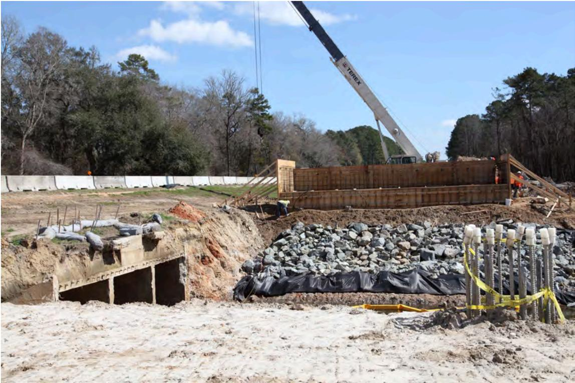
Fig. 2-9. Hurricane Creek Bridge, Looking East at End Bent Formwork
