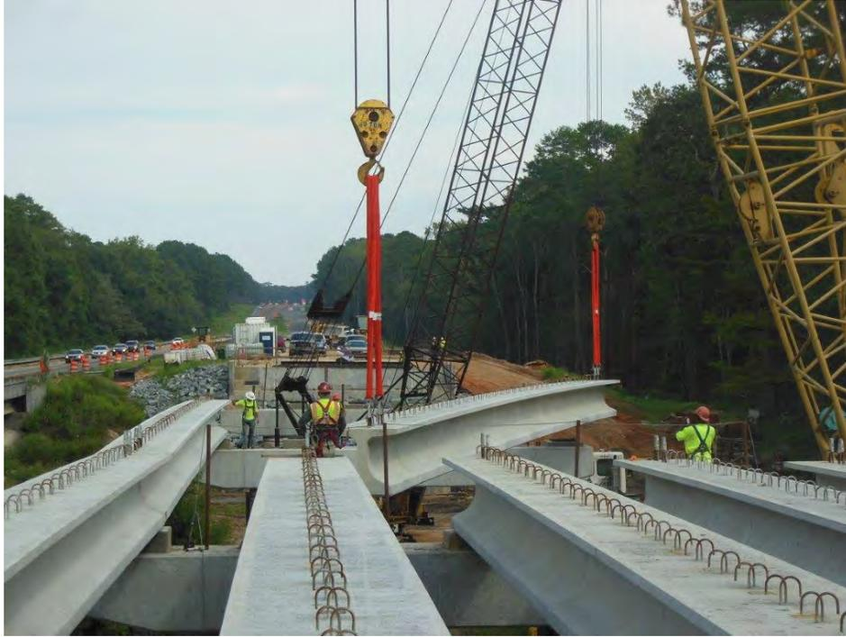
Fig. 3-18. Maneuvering a Girder into Position
