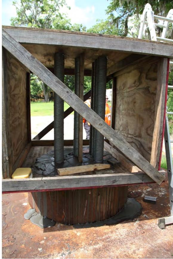
Fig. 5-5. Grout Mock-up for Precast Bent Cap, Side View, Wooden “Bent Cap” Forms on Top of Steel “Drilled Shaft” Casing
