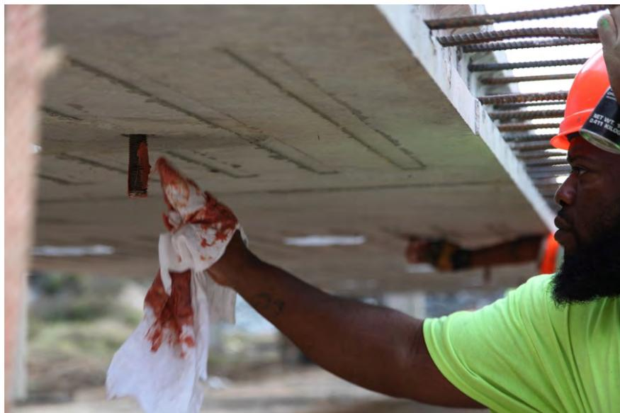
**Fig. 3-32. Greasing Leveling Bolts on a Panel Before Erection (October 30, 2014)**
