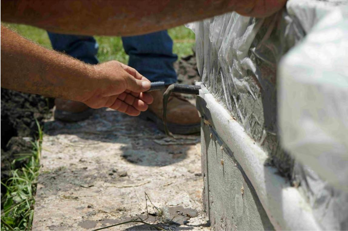
Fig. 5-17. Grout Mock-up for Precast Deck Panel, Plugging Corner to Stop Grout Flow
