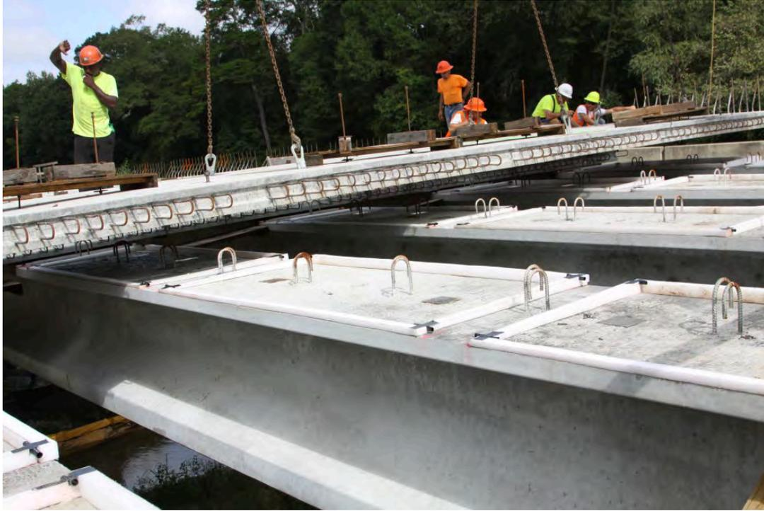
Fig. 3-52. Setting Precast Deck Panels on Hurricane Creek EB – Polystyrene Forms in Foreground
