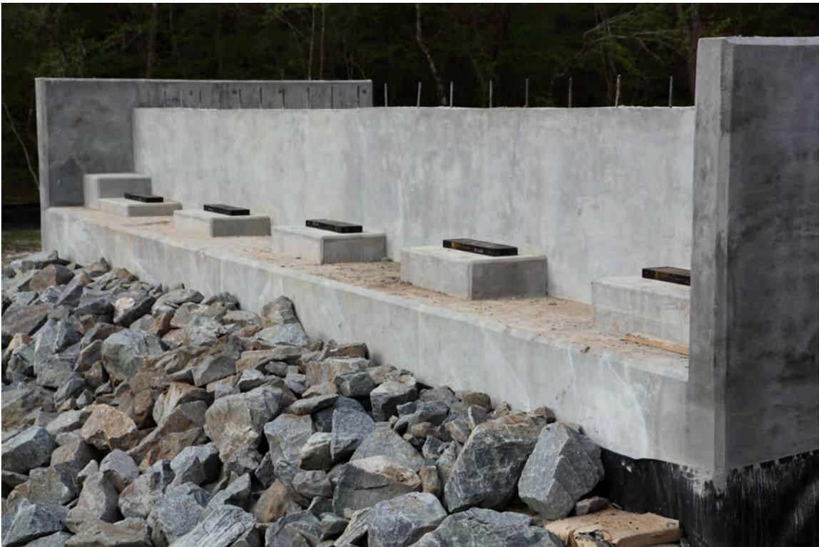
Fig. 2-13. Hurricane Creek Bridge, Completed West End Bent, with Pedestals and Bearing Pads in Position
