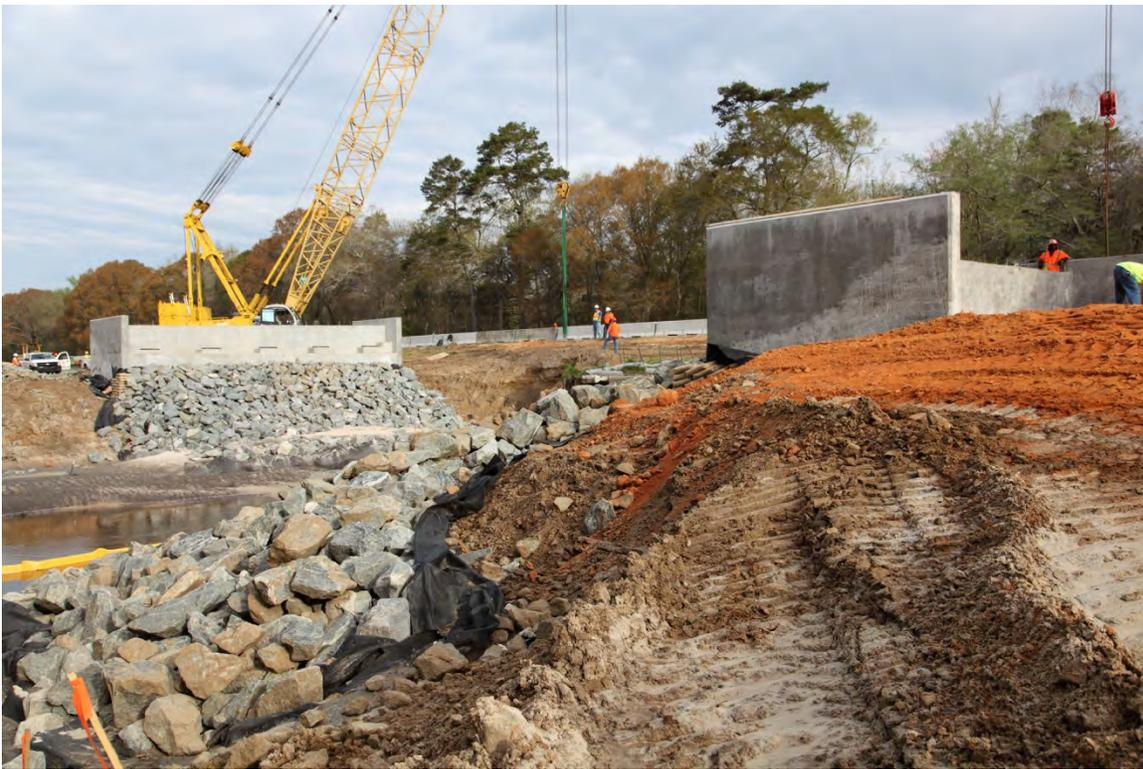
**Fig. 3-1. Hurricane Creek EB Bridge – Ready for Girder Installation (March 24, 2014)**
