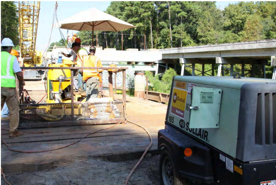
**Fig. 4-4. Equipment for Grouting**
