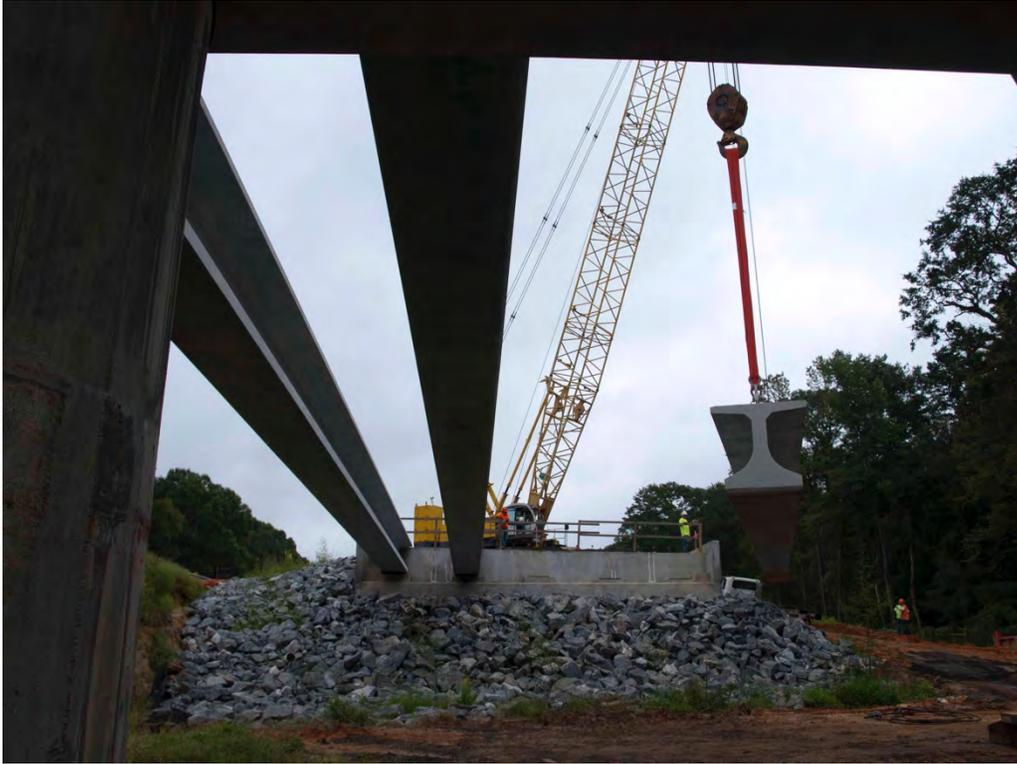
Fig. 3-16. Setting Girder on Little River EB – View under Bridge (September 20, 2014)
