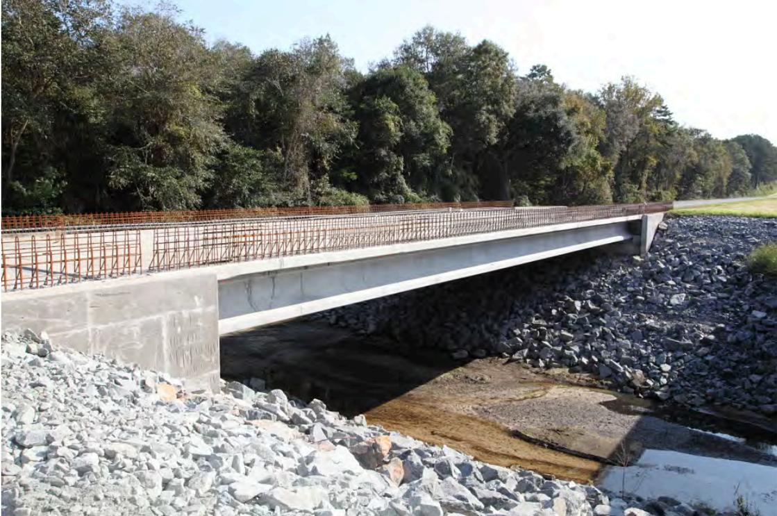
Fig. 4-47. Barrier Reinforcing Steel for Hurricane Creek WB
