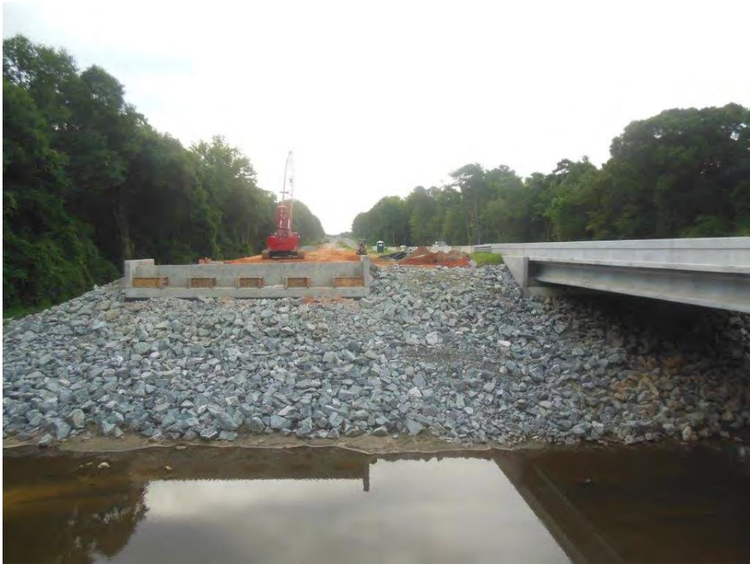
Fig. 2-7. Completed End Bent and Rip Rap Rubble
