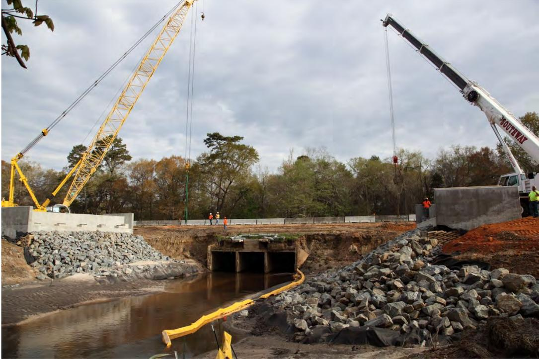
Fig. 3-2. Cranes at Abutments for Girder installation on Hurricane Creek EB Bridge – Looking North (March 24, 2014)
