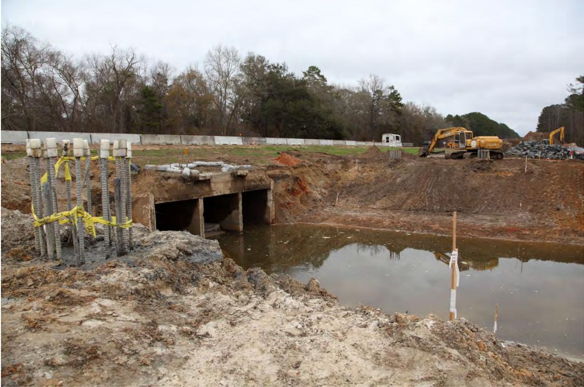
Fig. 1-8. Hurricane Creek EB Bridge Site, Looking East from End Bent. Existing EB Bridge Has Been Demolished and Existing WB Bridge Remains. (February 3, 2014)
