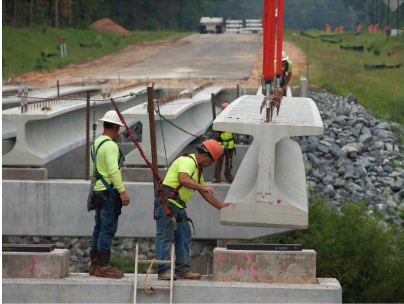
Fig. 3-22. Setting Girder on Bearing on Little River EB (September 19, 2014)
