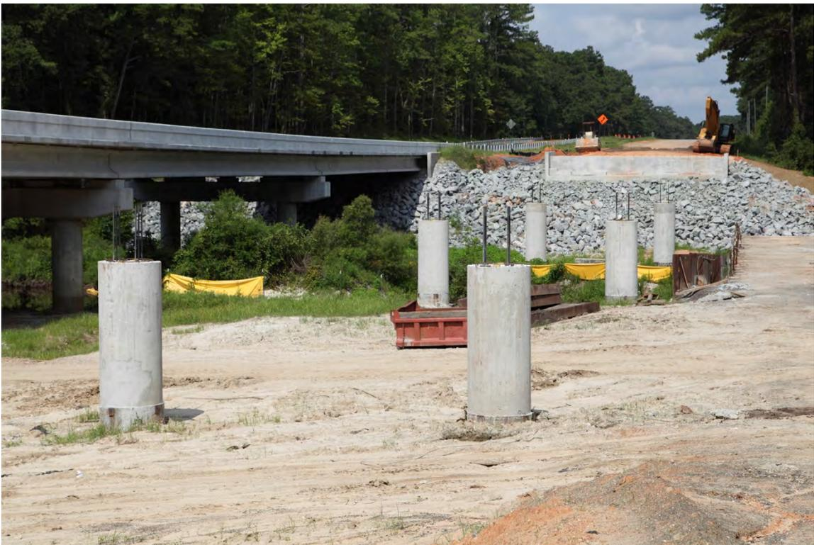
Fig. 2-16. Six (6) Columns for Little River WB Intermediate Bents (July 21, 2015)
