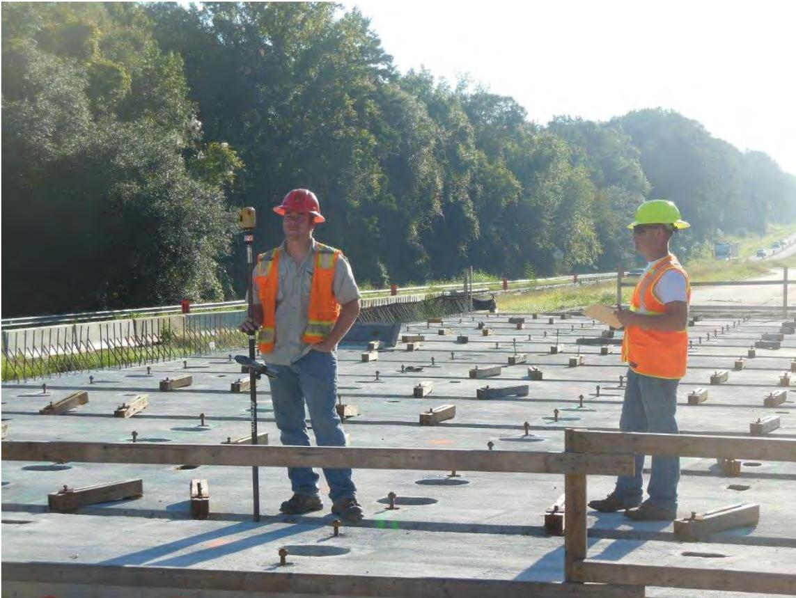
**Fig. 3-45. Surveying After Placing Deck Panels**
