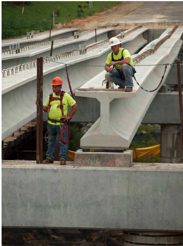
Fig. 3-23. Girder on Bearing Pedestal on Little River EB (September 20, 2014)
