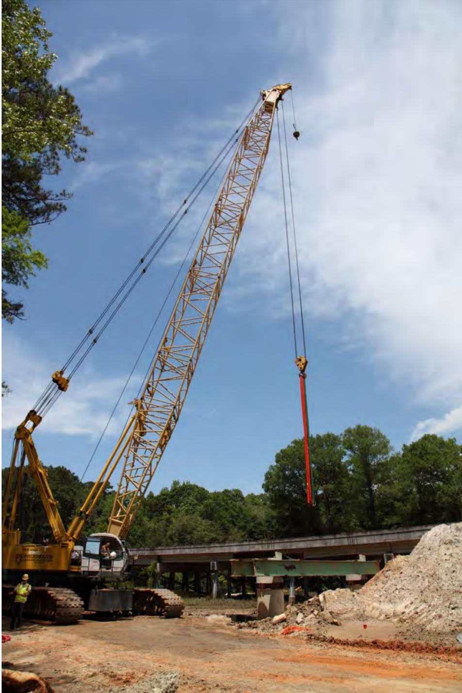
Fig. 2-21. Crane for Setting a Precast Bent Cap on Little River EB (May 7, 2014)
