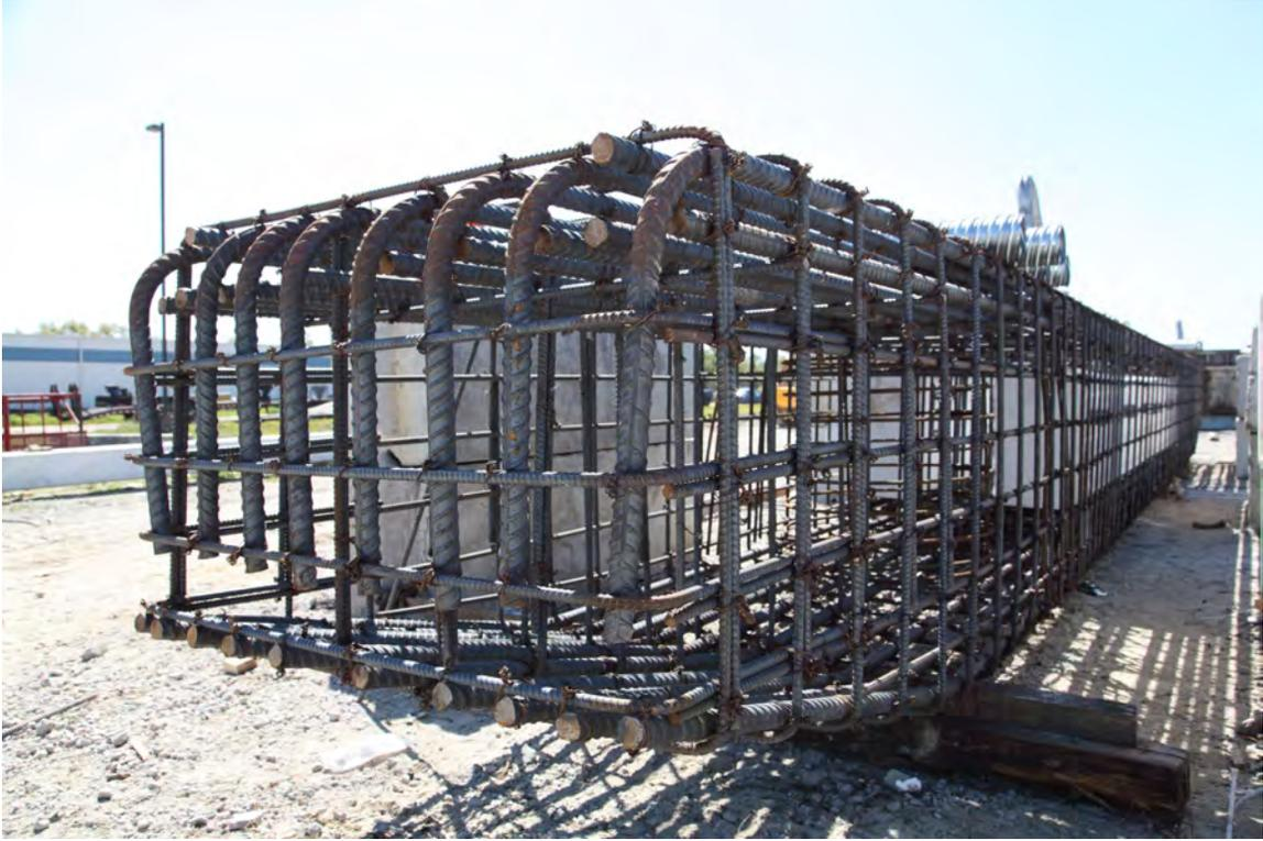
Fig. 6-9. Precast Bent Cap, Reinforcing Steel Cage
