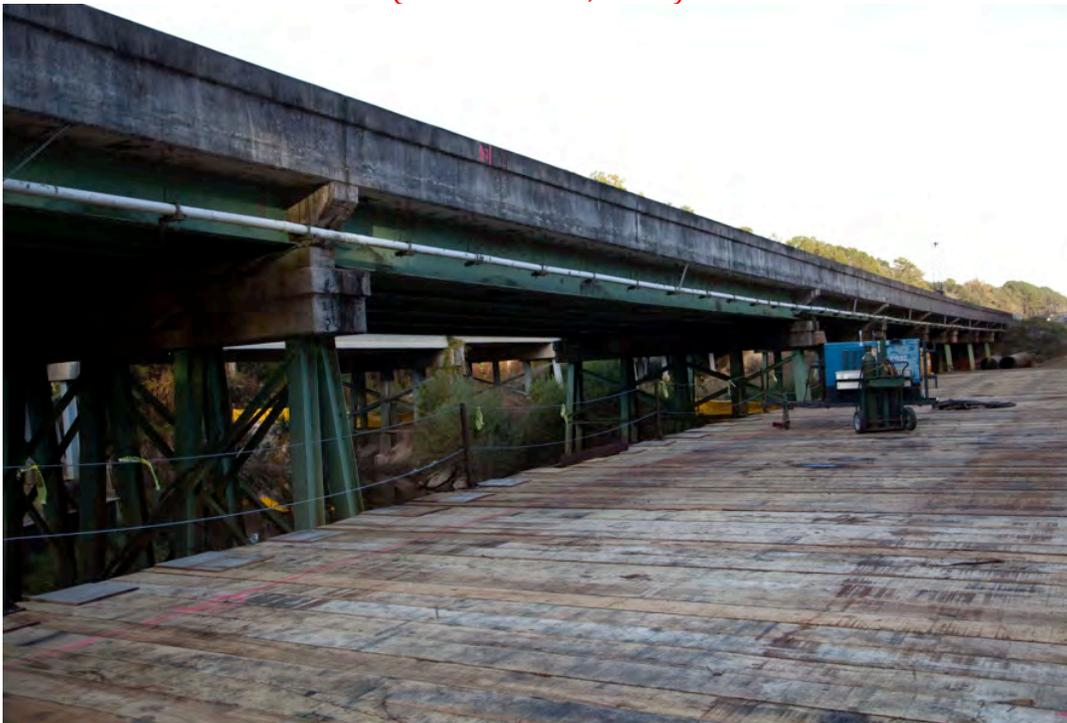
Fig. 1-11. Existing Little River EB Bridge During Construction: Temporary Work Bridge, Southwest Corner, Looking East (November 11, 2013)
