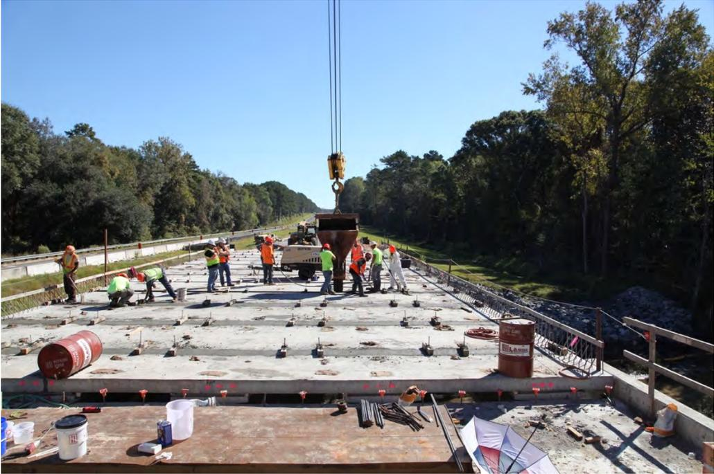
**Fig. 4-42. Casting Closure Joints on Hurricane Creek EB**
