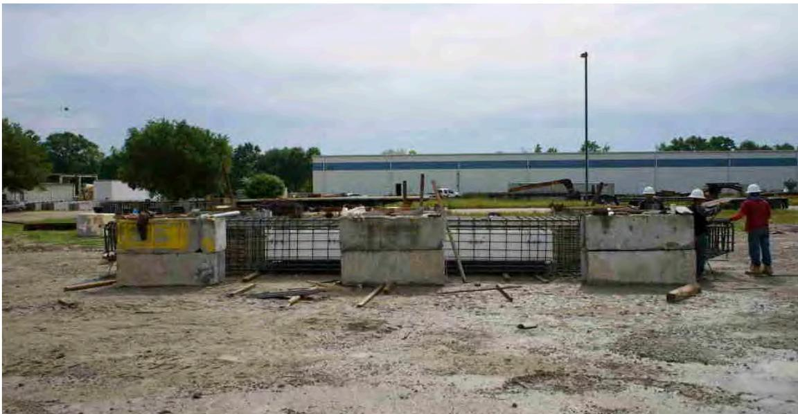
Fig. 6-8. Precast Bent Cap, Tying Reinforcing Steel Cage (Concrete Blocks are Partially Obstructing View)
