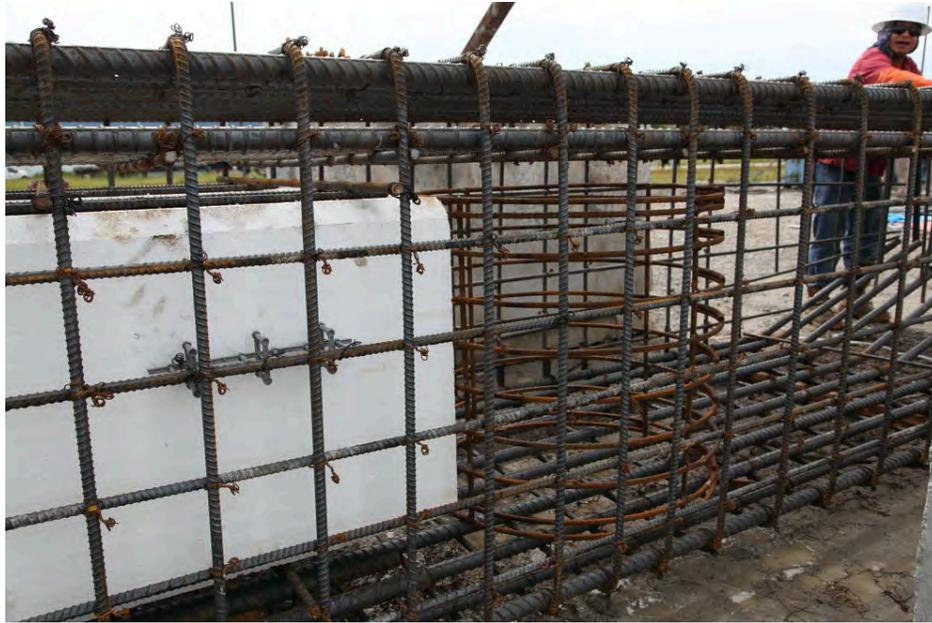
Fig. 6-20. Precast Bent Cap, Reinforcing Steel Cage and EPS Blockout, Side View
