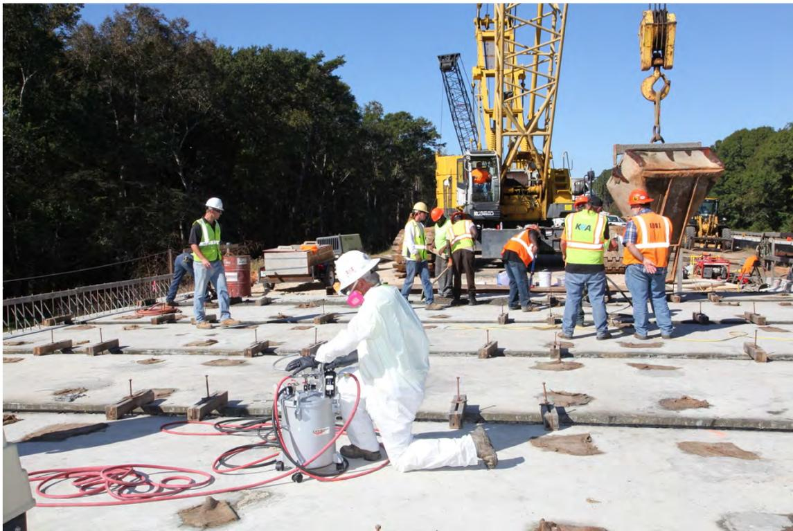
**Fig. 4-41. Epoxy Bonding Agent was Sprayed to Panel Keys Before Casting Closure Joints**
