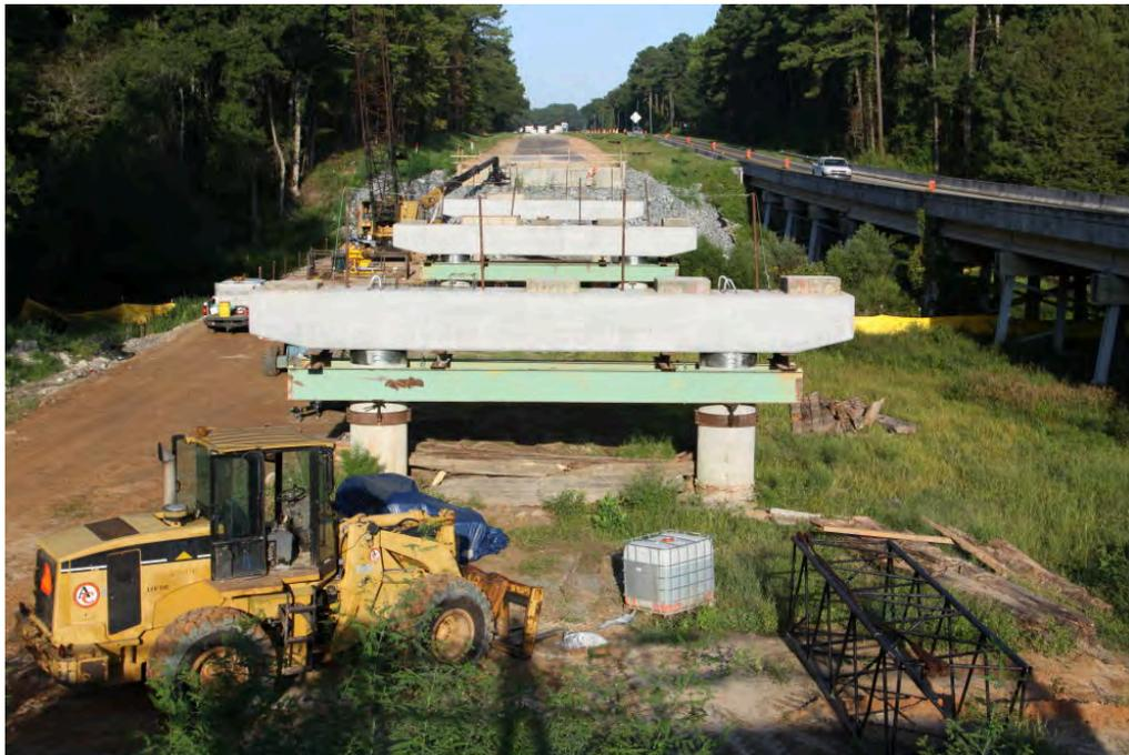
Fig. 2-26. Friction Collars for Precast Bent Caps on Little River EB (September 11, 2014)
