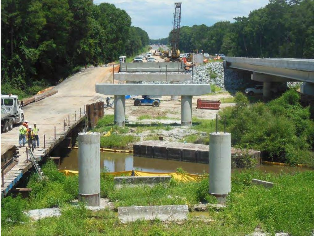
Fig. 2-27. Friction Collars not Used on Little River WB (July 24, 2015)
