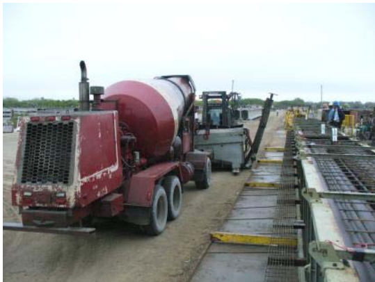
Figure 22–Concrete delivery (left) and placement (right)
