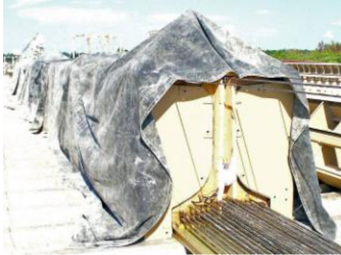
Figure 27–Girders covered with tarps
