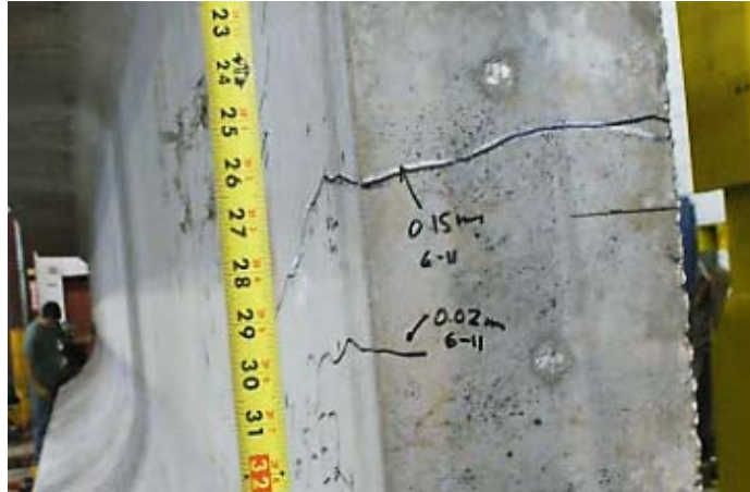
Figure 63–Web crack measurements (view from end of specimen)
