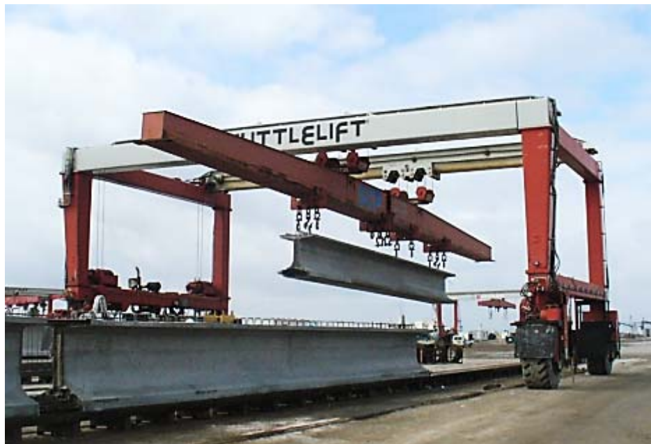
Figure 26–Girder lifted by crane
