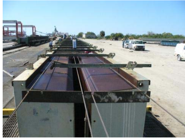
Figure 21–Form release application (left) and form cross-ties (right)
