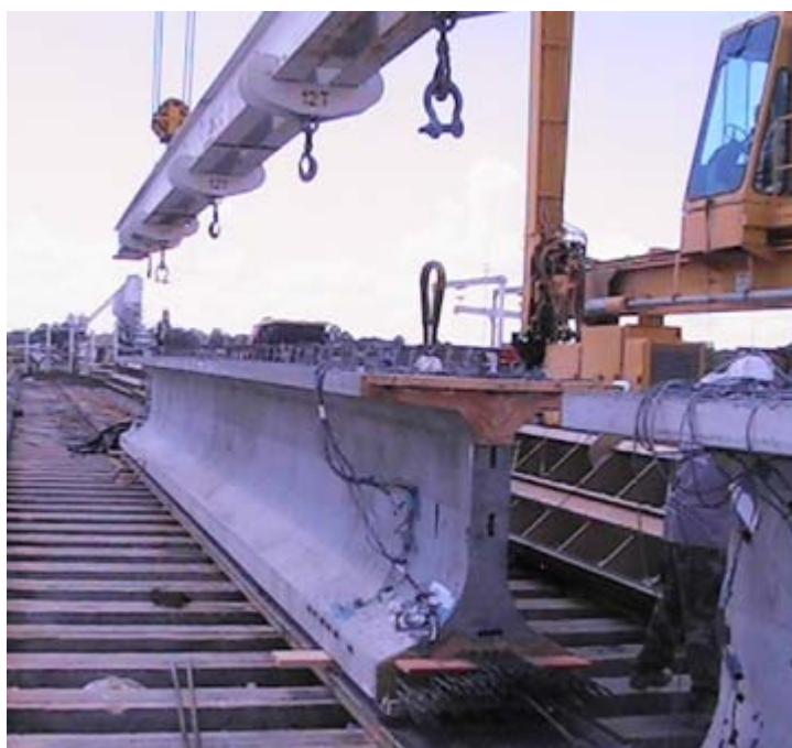
Figure 30–Girder resting on dunnage above stressing bed
