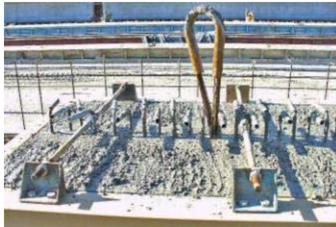
Figure 26–Girder finished surface
