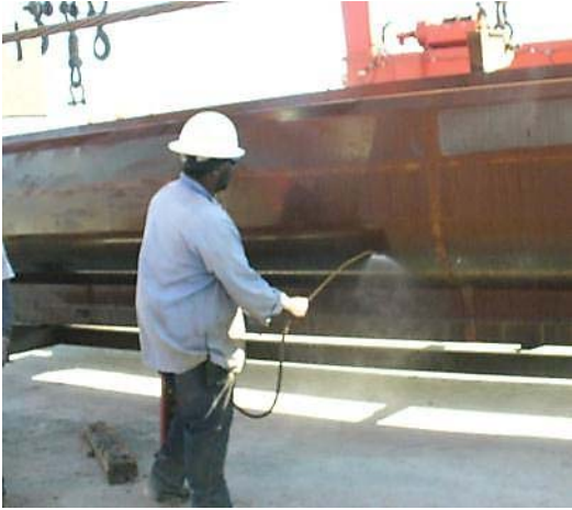
Figure 21–Form release application (left) and form cross-ties (right)
