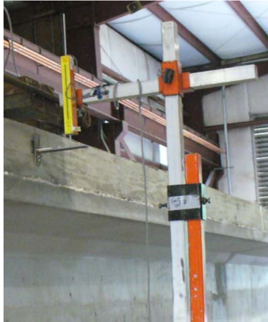
Figure 45–LVDT and support frame
