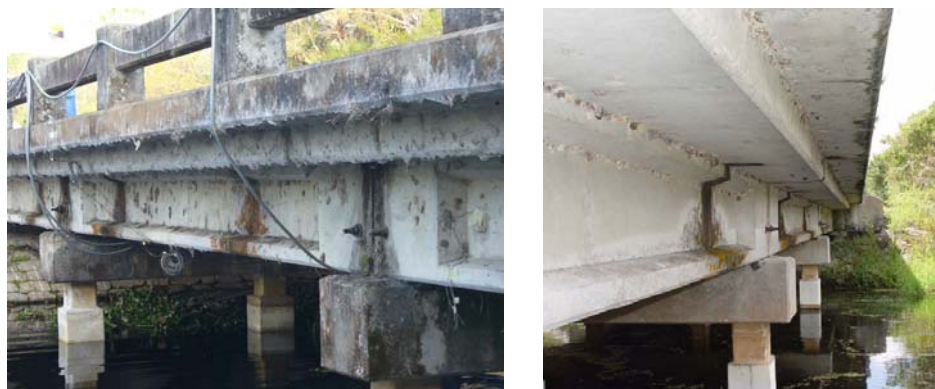
Figure 1–Existing bridge prior to girder removal
