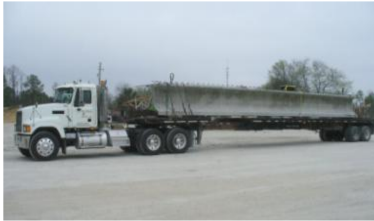
Figure 31–Girder H on truck prior to transit
