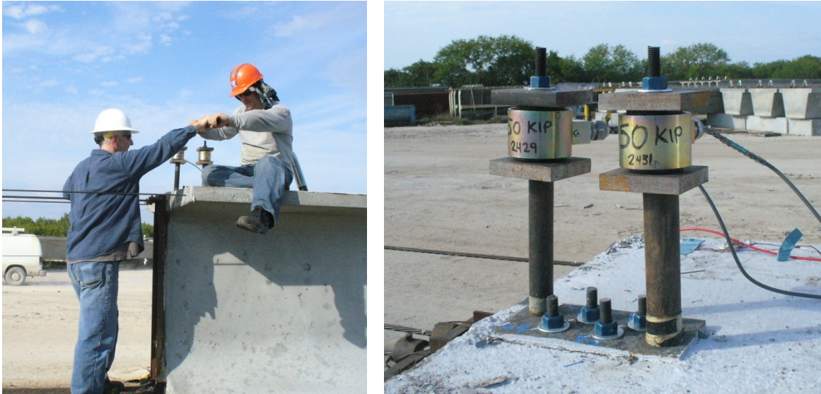
Figure 24–Post-tensioning specimen PT (left) and load cells and anchor plate (right)
