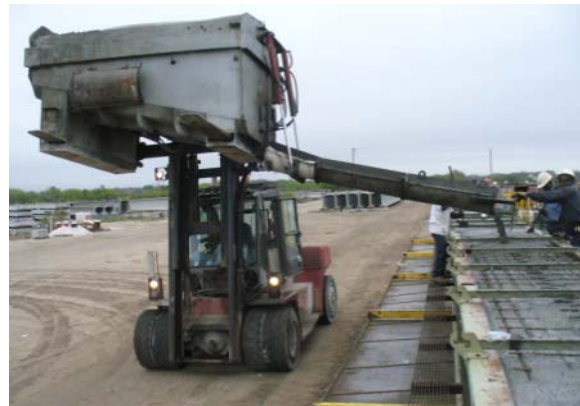
Figure 22–Concrete delivery (left) and placement (right)
