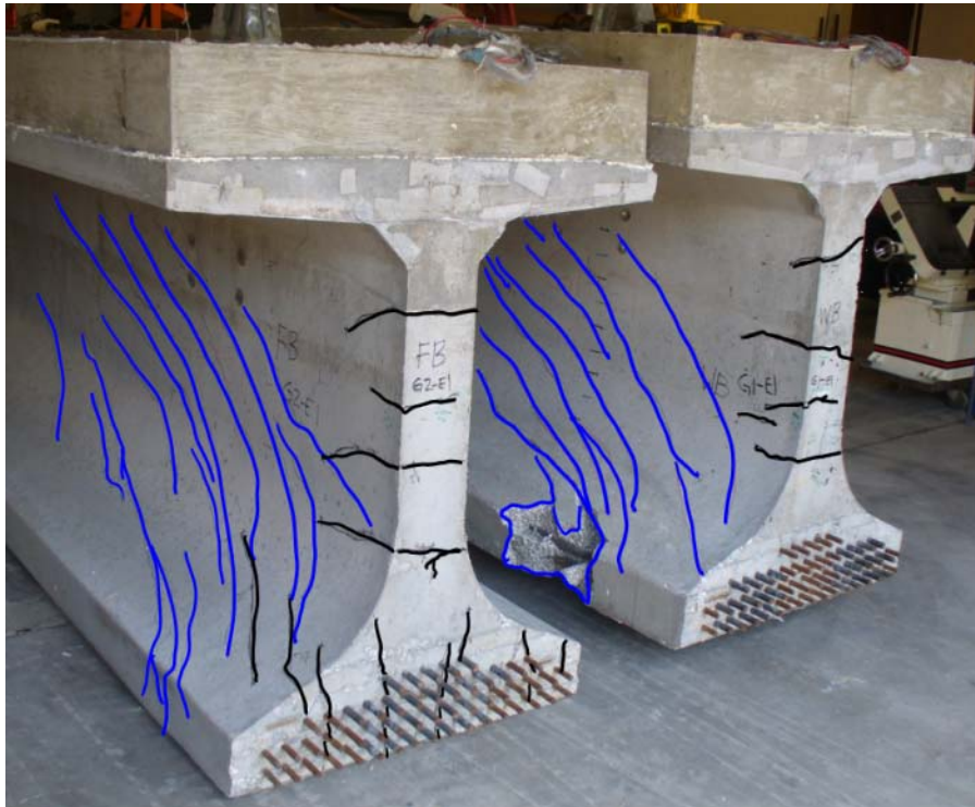
Figure 119–Comparison of FB (left) and WB (right) (release cracks shown black; final cracks shown blue)
