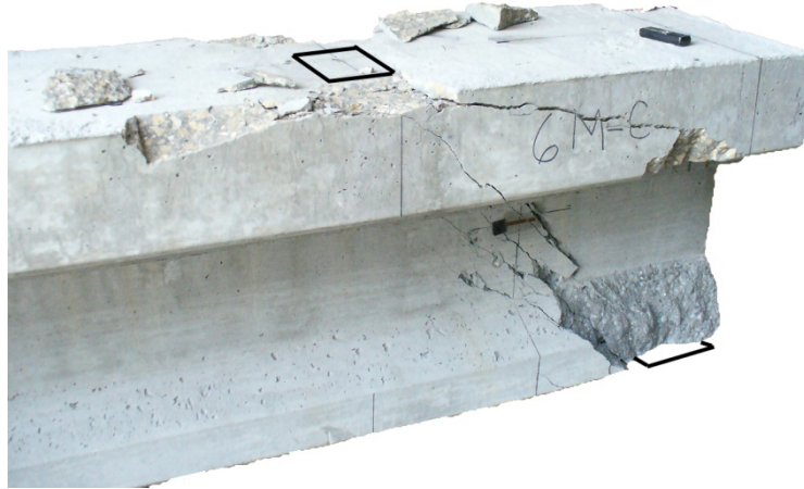
Figure 19–Bond-flexure failure mode (B6M-C)
