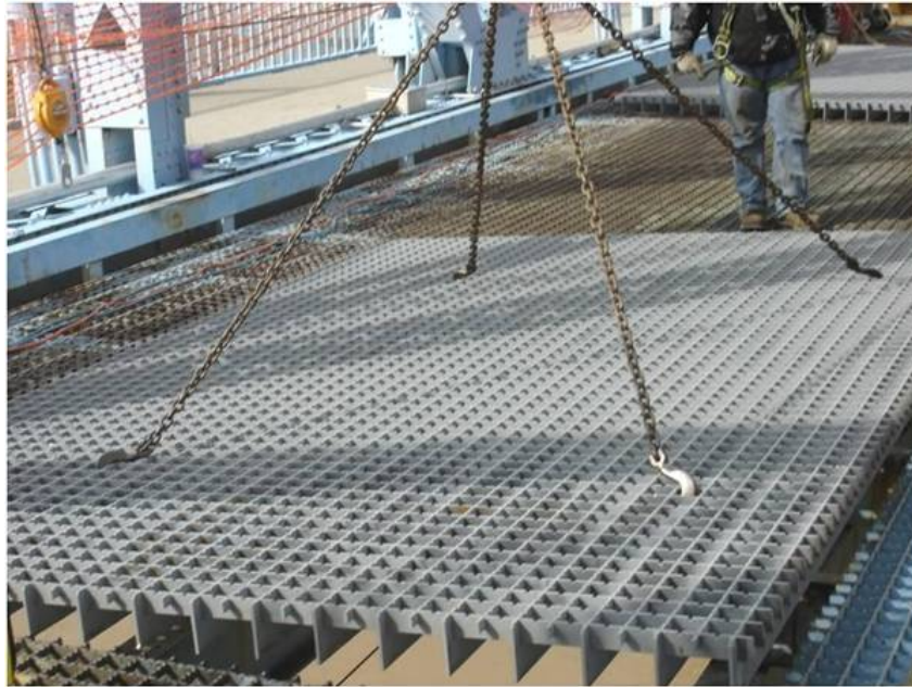
Figure 2.6: Open Grid Deck
