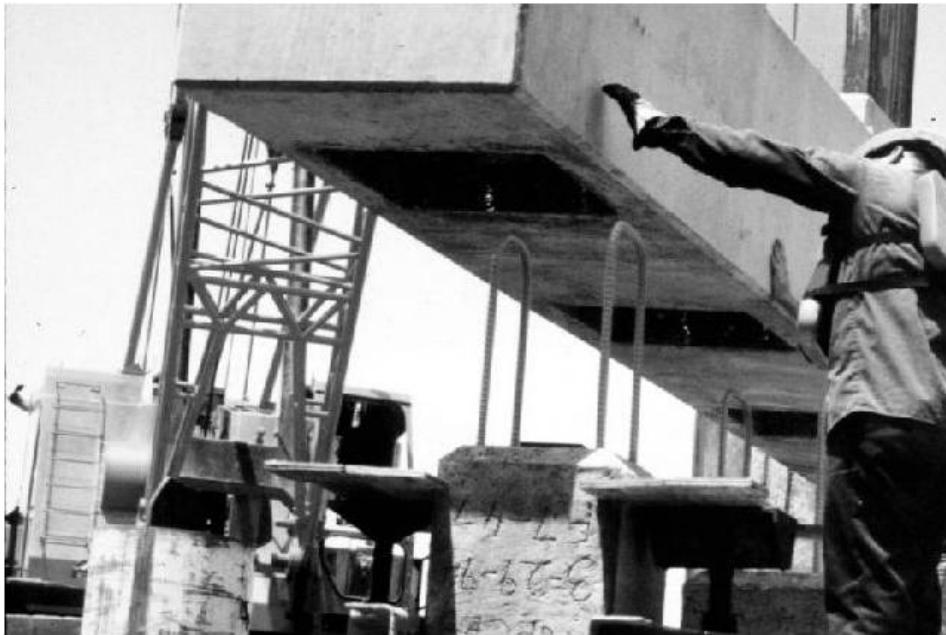
Figure 2.12: Placement of Precast Bent for Redfish Bay Bridge ( www.fhwa.dot.gov/bridge/prefab/all.cfm?view=31 )
