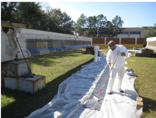
Figure 9-4: CFRP wrapping application
