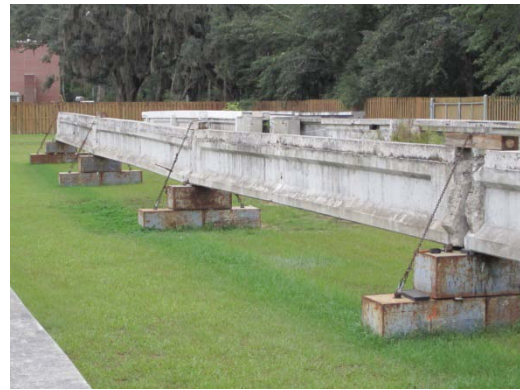
Figure 9-3: Girder preparation for wrapping
