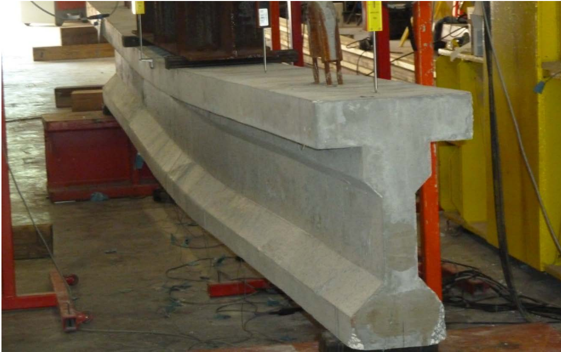
Figure 4-21: Half-scale control girder displaying excessive deflection under loading
