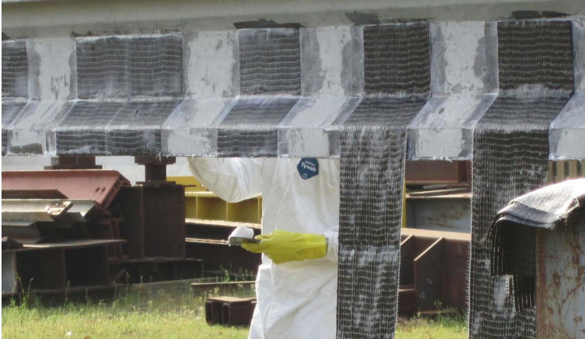
Figure 3-16: Wet layup application of CFRP fabric laminates on PS girder
