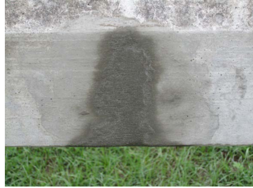
Figure 9-2: Repair of the concrete damage
