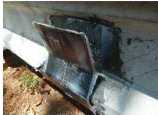
Figure 4-24:(left) Rupture of longitudinal CFRP, (right) Debonding of CFRP U-wrapping
