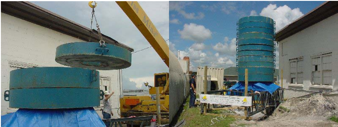
Figure 146 Loading process and final load applied
