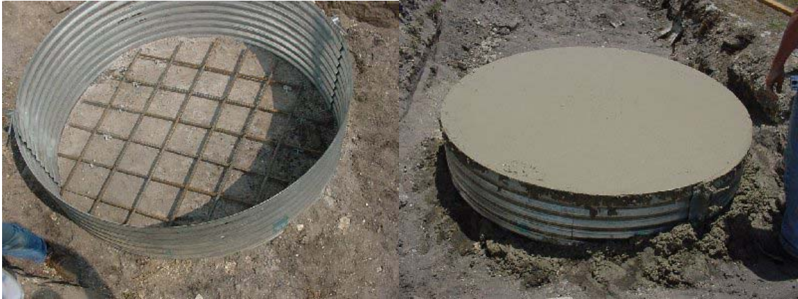
Figure 140 Footing before and after the casting of the concrete
