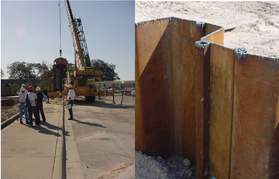
Figure 117 CZ128 pile driving (a), and inclinometer casing attached to CZ128 (b)
