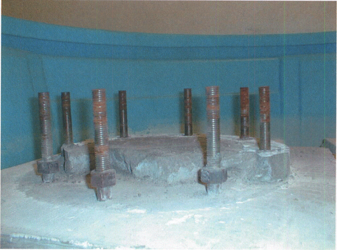
Figure 5.13 : Picture Of Anchor Bolts In Base Plate Arrangement With Grout B Material As Grout Pad After 14 Weeks Of Wet – Dry Cycling Of Salt Solution.
