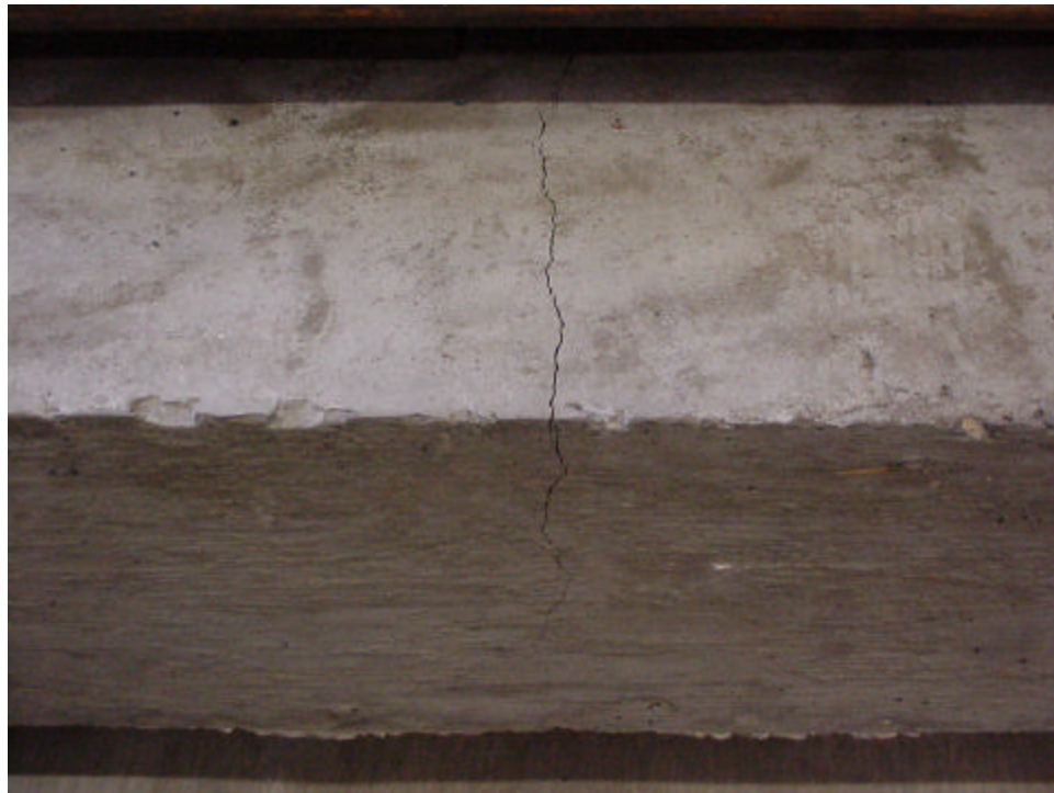
Figure B.11 – Specimen D Splitting failure
