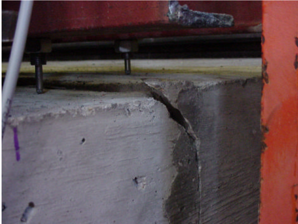
Figure C.11 – Specimen D3 yielding failure
