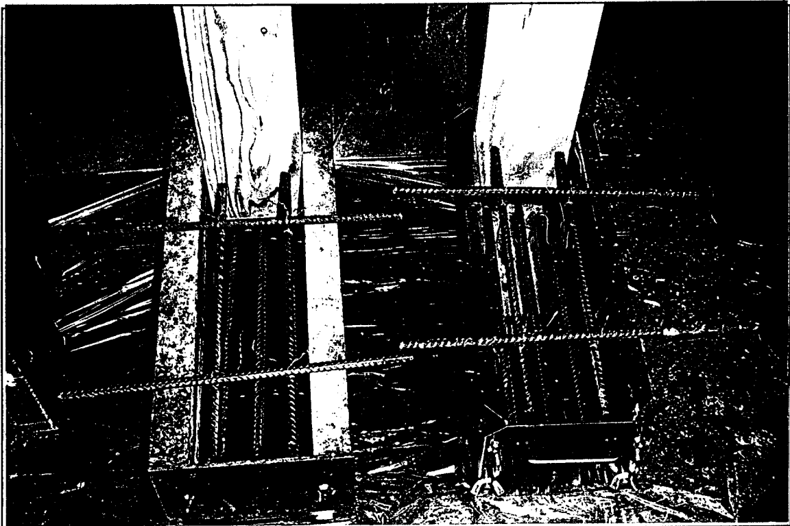
Figure 2.2 Control beams prior to casting of concrete
