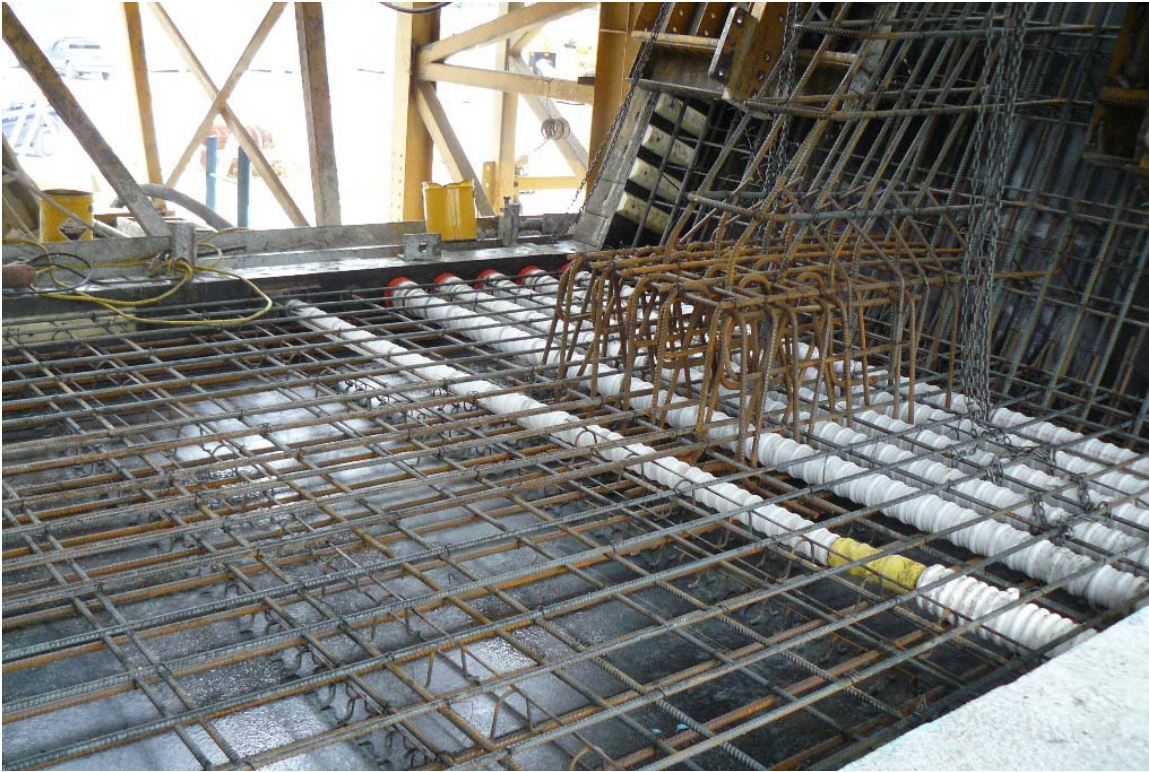
Figure 20.4-1 Reinforcing in Deviation Segment
