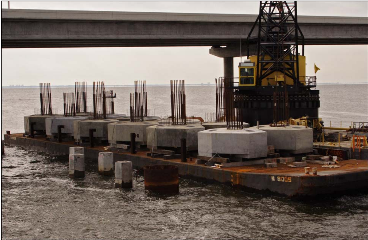
Figure 25.4.3.6-3 Precast Footing Installation
