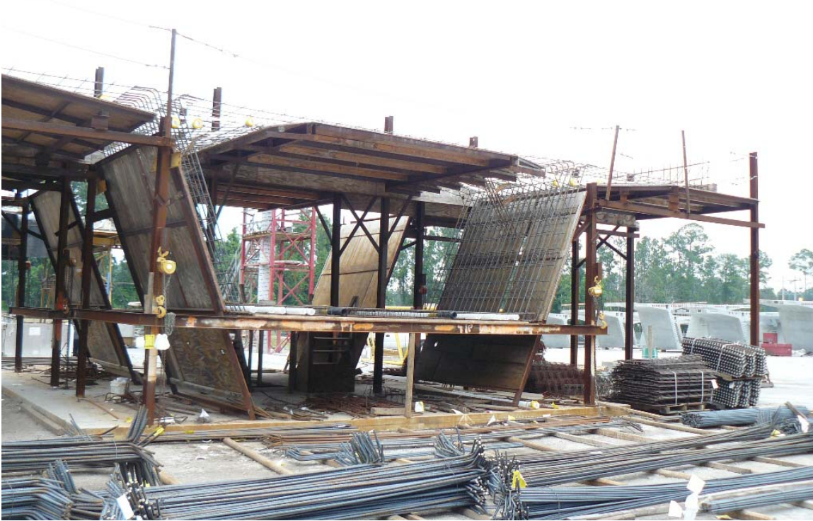
Figure 20.1-1 Reinforcing Jig for Variable Depth Segment
