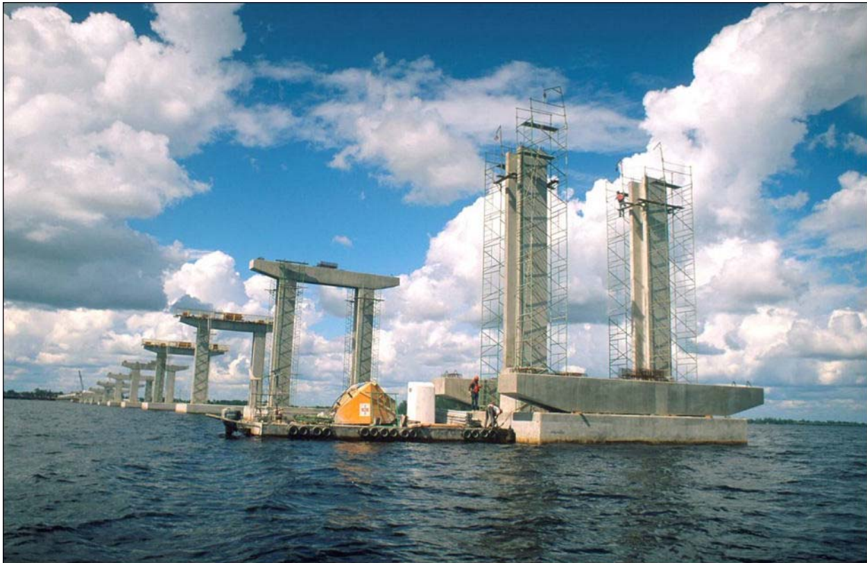
Figure 25.4.3.3-1 Precast Pier Cap Installation
