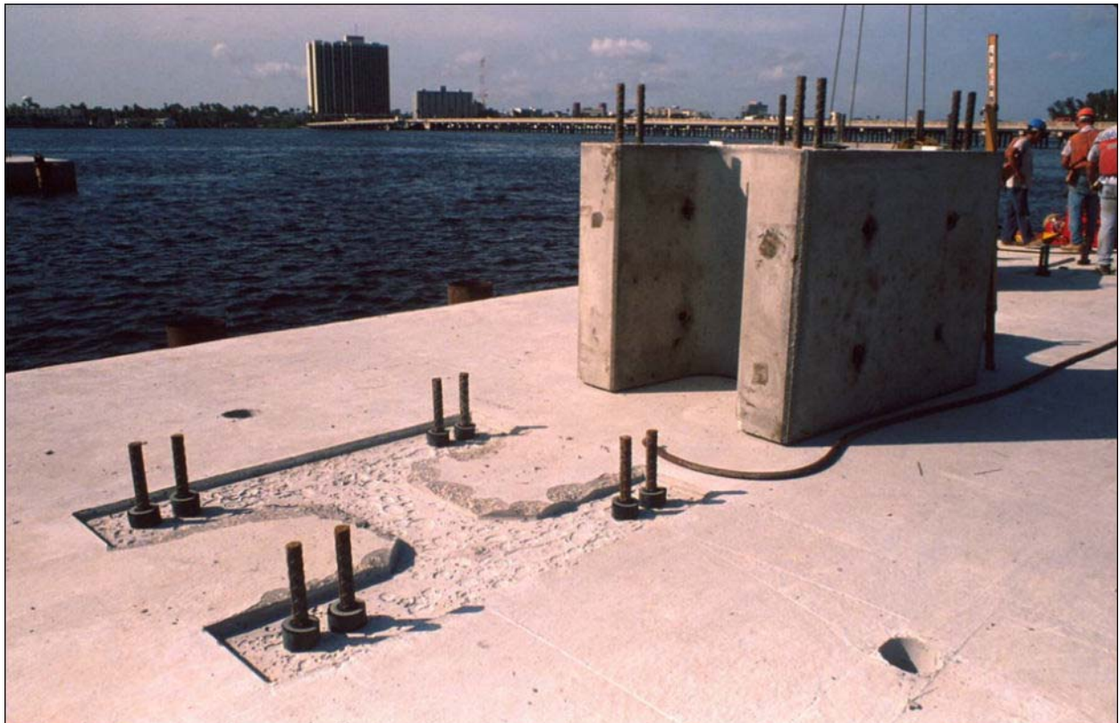
Figure 25.4.3.2-3 C.I.P. Foundation and Precast H-Section Pier Column
