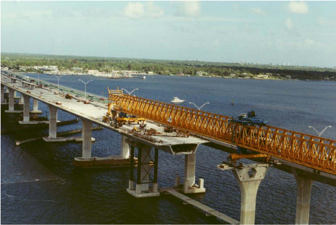
Figure 20.9.1-5 Gantry with Leg on Pier Segment
