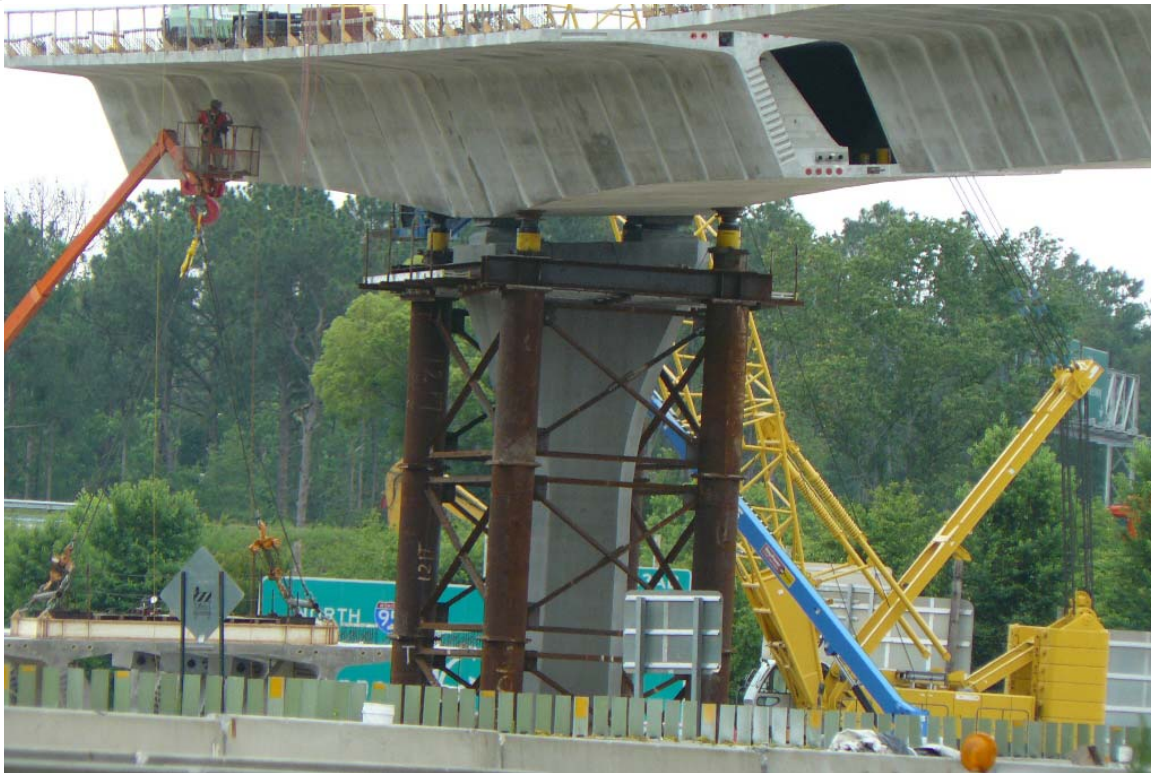
Figure 20.9.1-2 Stabilization of Balanced Cantilever
