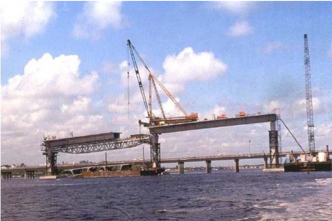
Figure 20.9.2-1 Span by Span Construction
