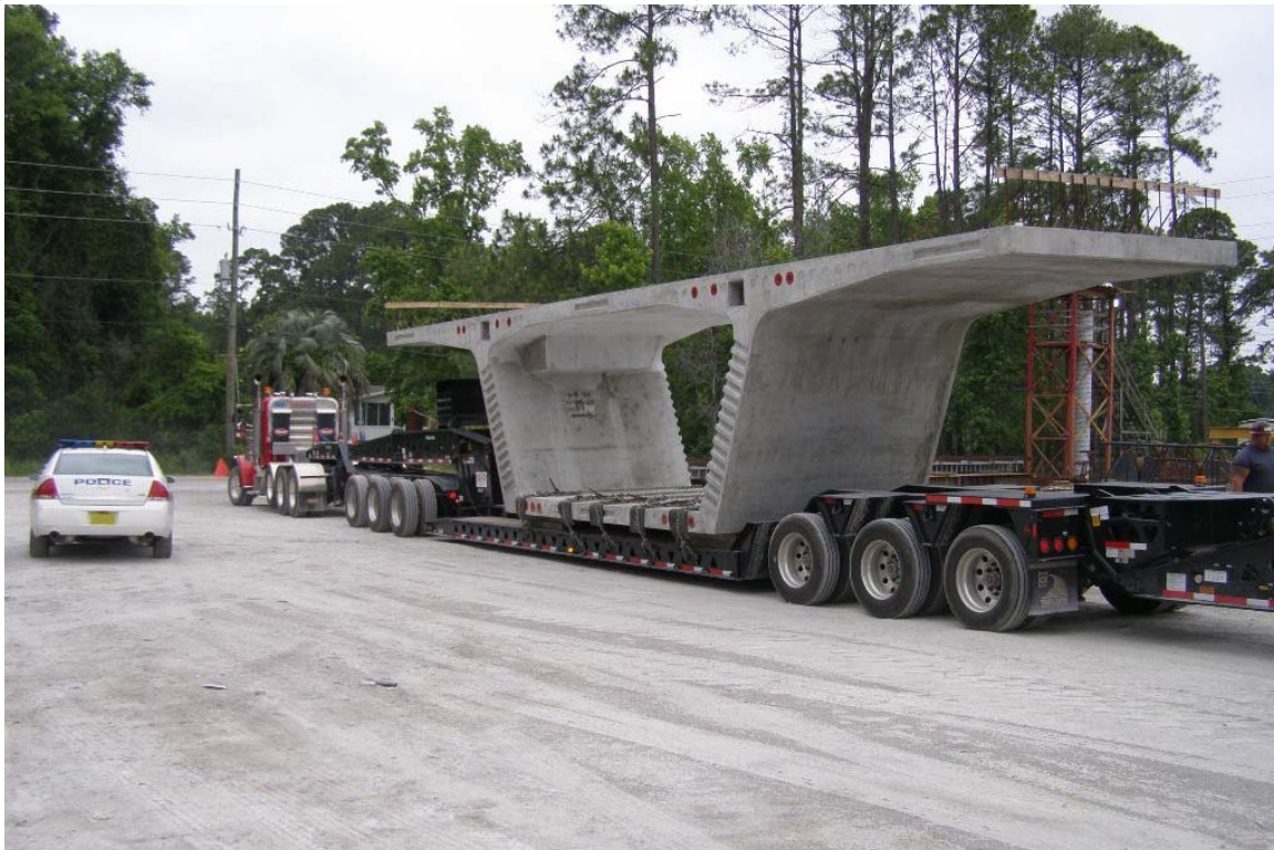
Figure 20.9.2-5 Truck Loaded with Segment
