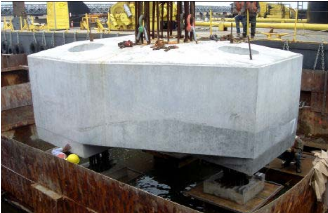
Figure 25.4.3.6-3 Precast Footing Installation
