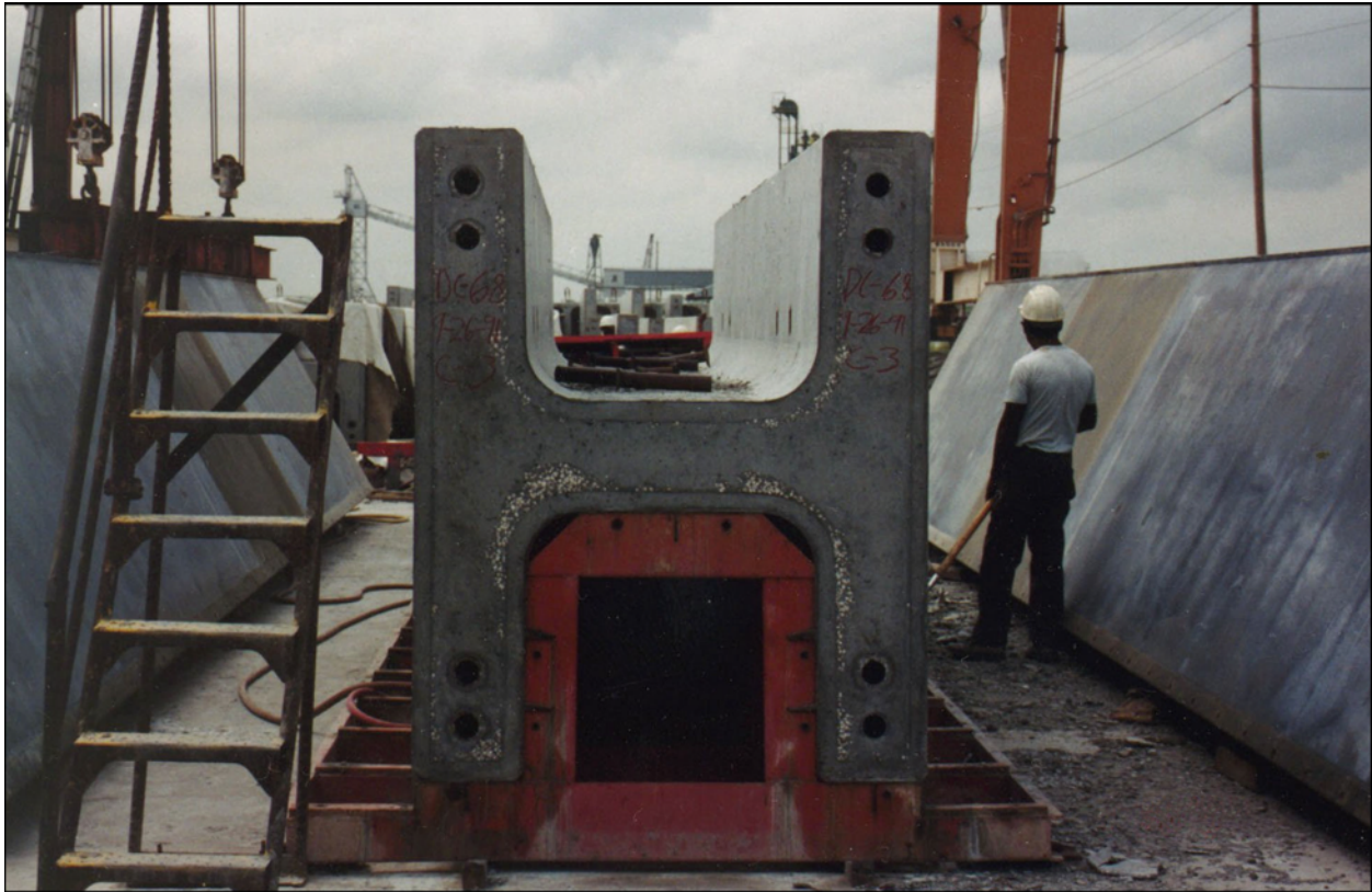
Figure 25.4.3.2-3 C.I.P. Foundation and Precast H-Section Pier Column
