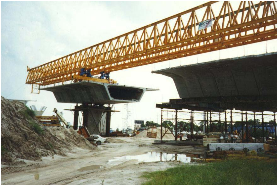
Figure 20.9.1-4 Gantry and Stabilization Towers
