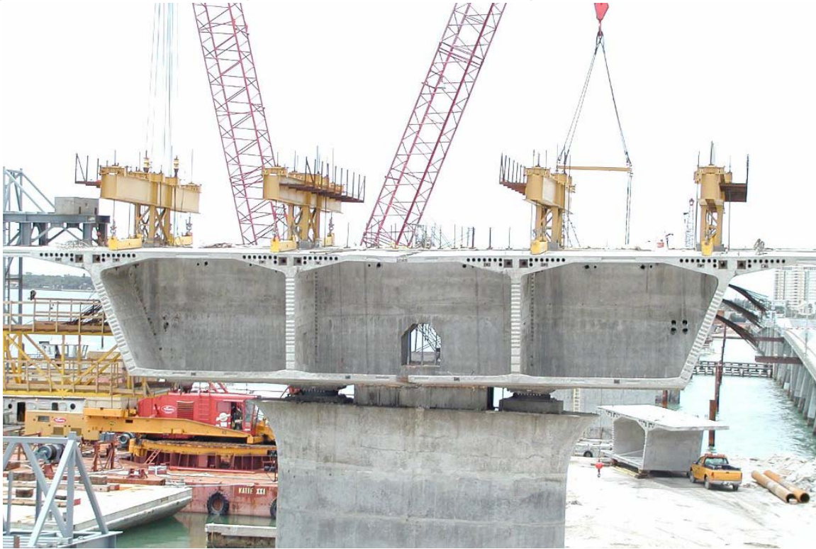
Figure 20.9.1-3 Setting Geometry with Strongbacks
