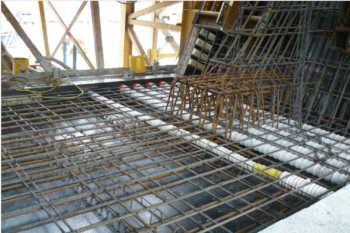
Figure 20.4-1 Reinforcing in Deviation Segment
