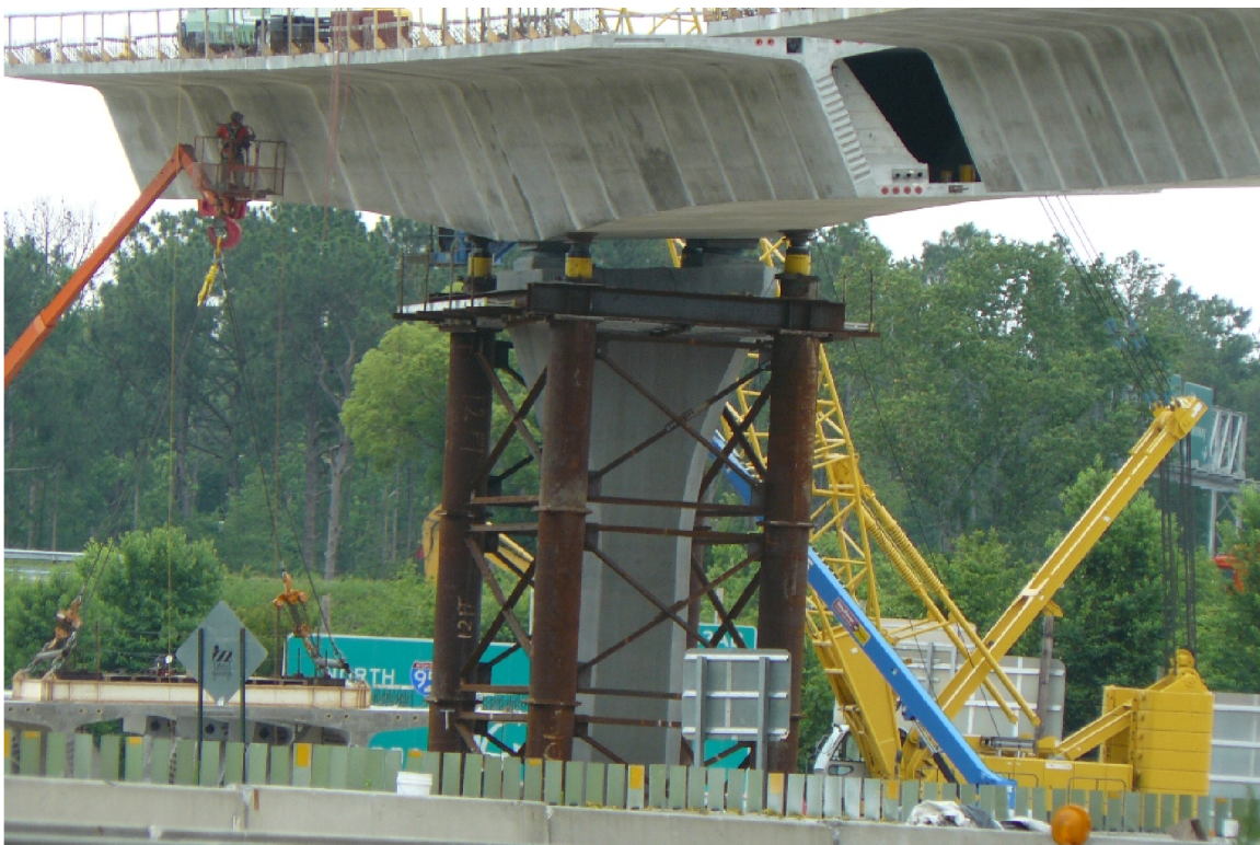
Figure 20.9.1-2 Stabilization of Balanced Cantilever
