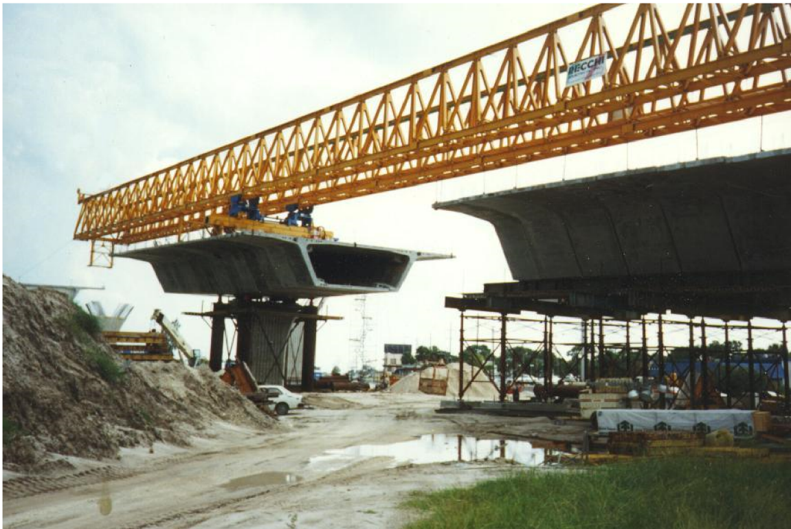
Figure 20.9.1-4 Gantry and Stabilization Towers
