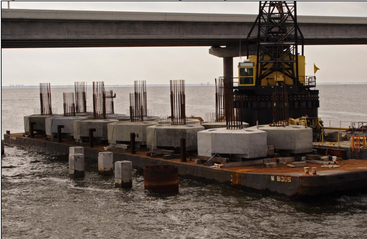
Figure 25.4.3.6-3 Precast Footing Installation
