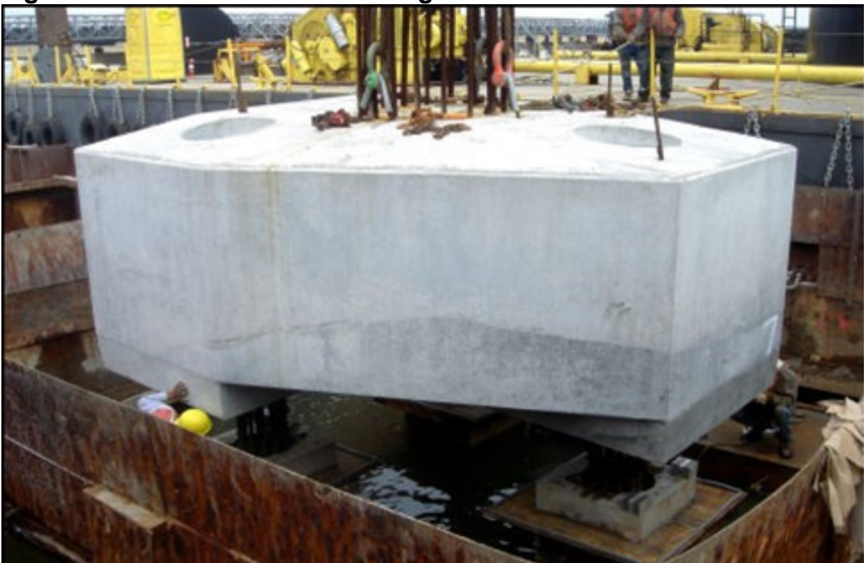
Figure 25.4.3.6-3 Precast Footing Installation
