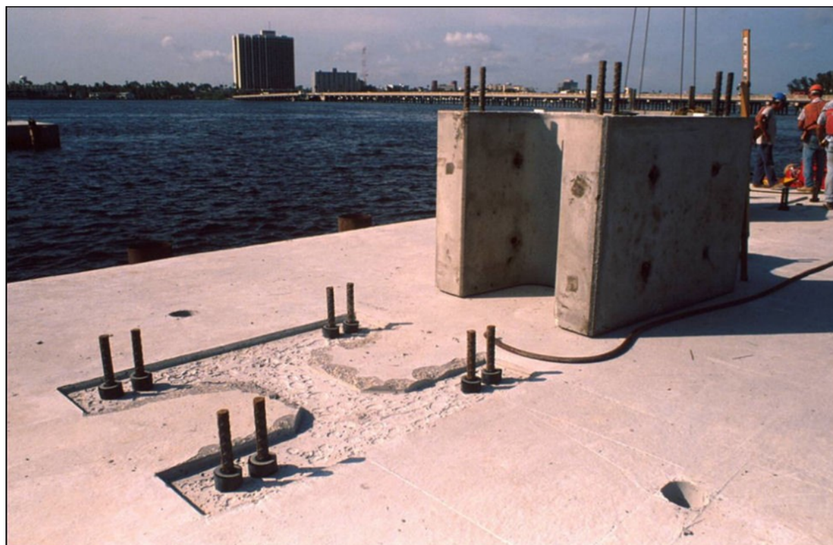
Figure 25.4.3.2-3 C.I.P. Foundation and Precast H-Section Pier Column
