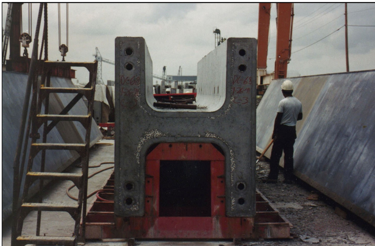
Figure 25.4.3.2-3 C.I.P. Foundation and Precast H-Section Pier Column
