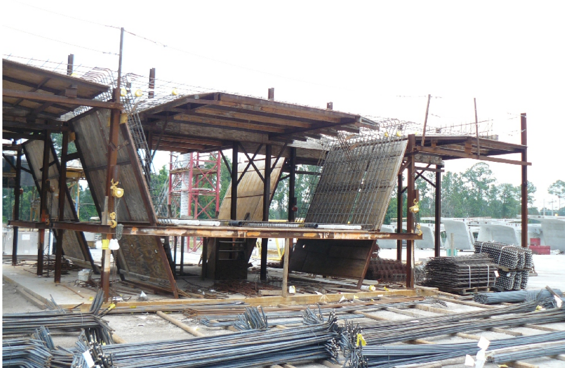
Figure 20.1-1 Reinforcing Jig for Variable Depth Segment
