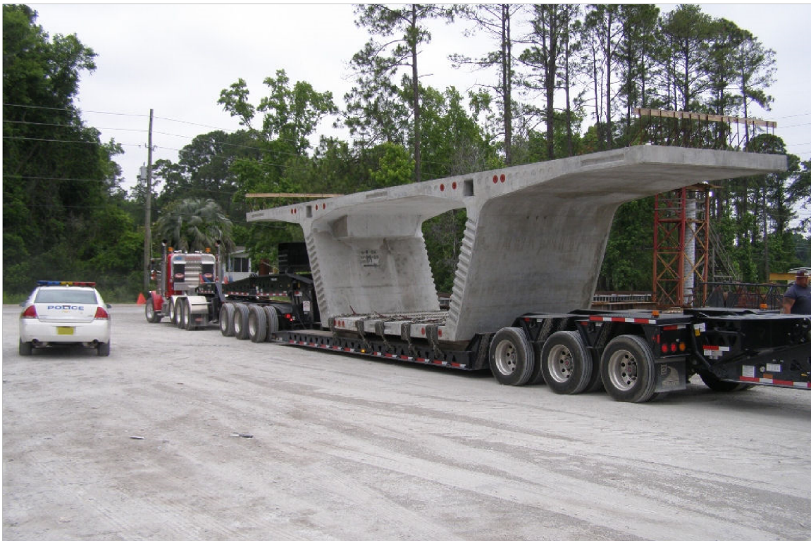
Figure 20.9.2-5 Truck Loaded with Segment
