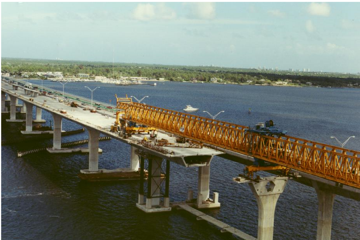
Figure 20.9.1-5 Gantry with Leg on Pier Segment
