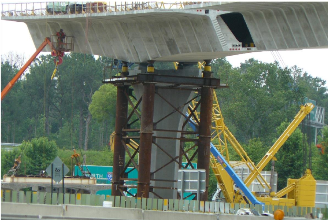
Figure 20.9.1-2 Stabilization of Balanced Cantilever
