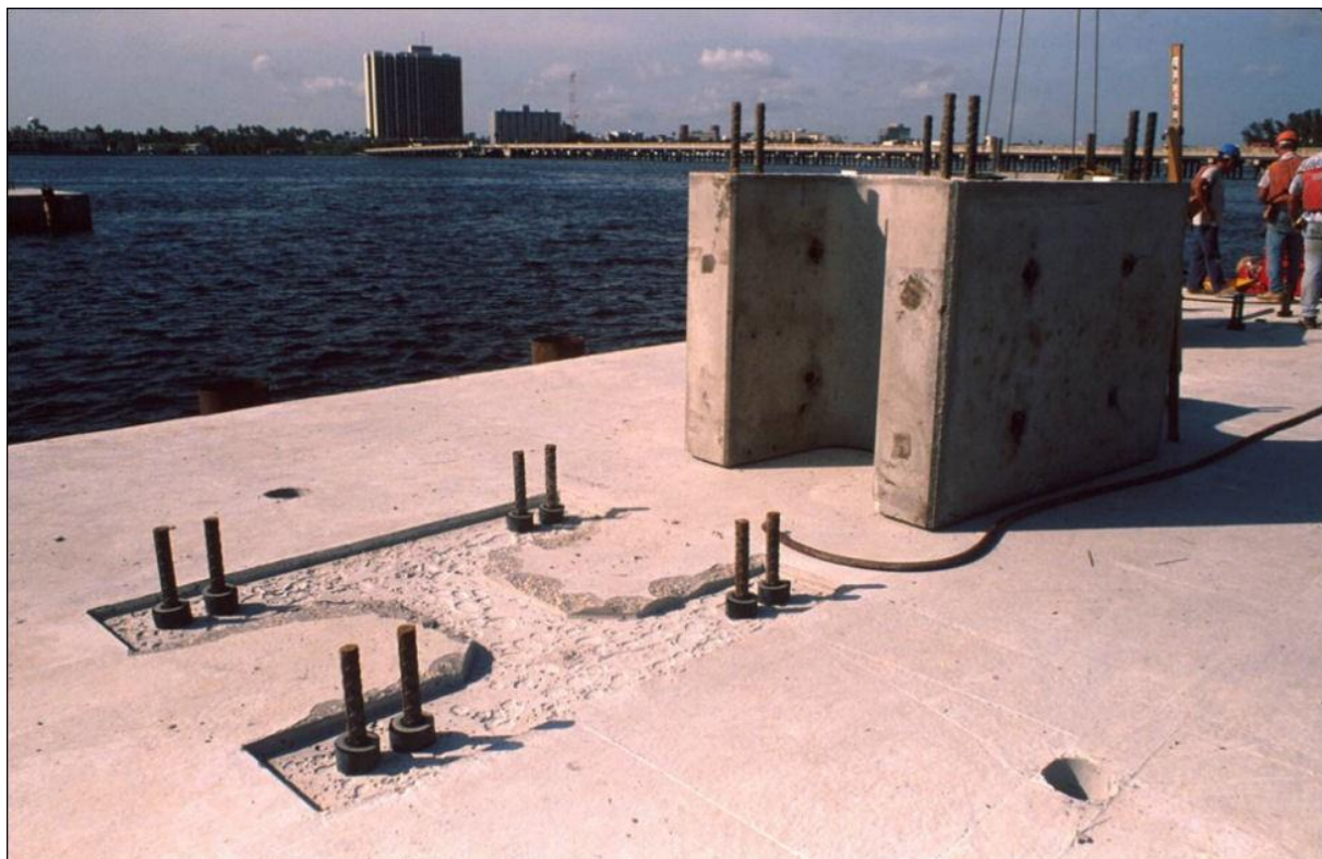
Figure 25.4.3.2-3 C.I.P. Foundation and Precast H-Section Pier Column
