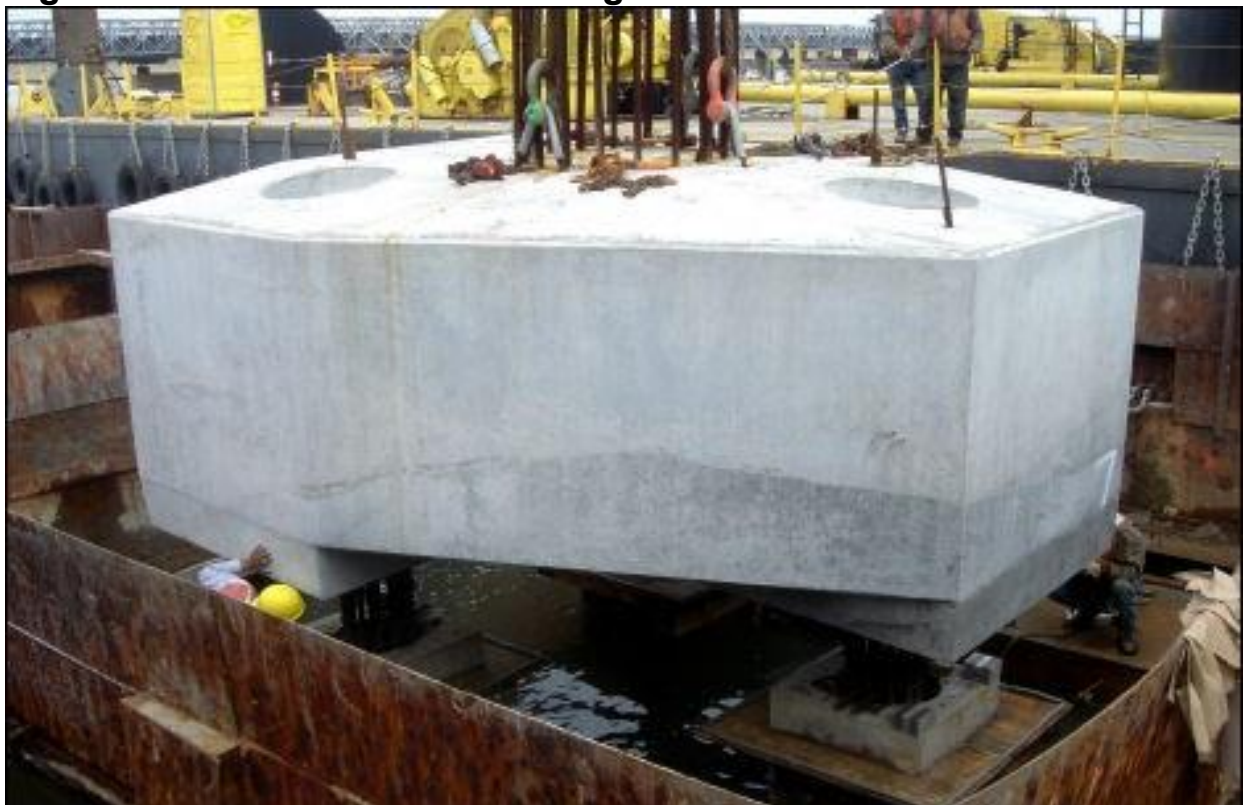
Figure 25.4.3.6-3 Precast Footing Installation
