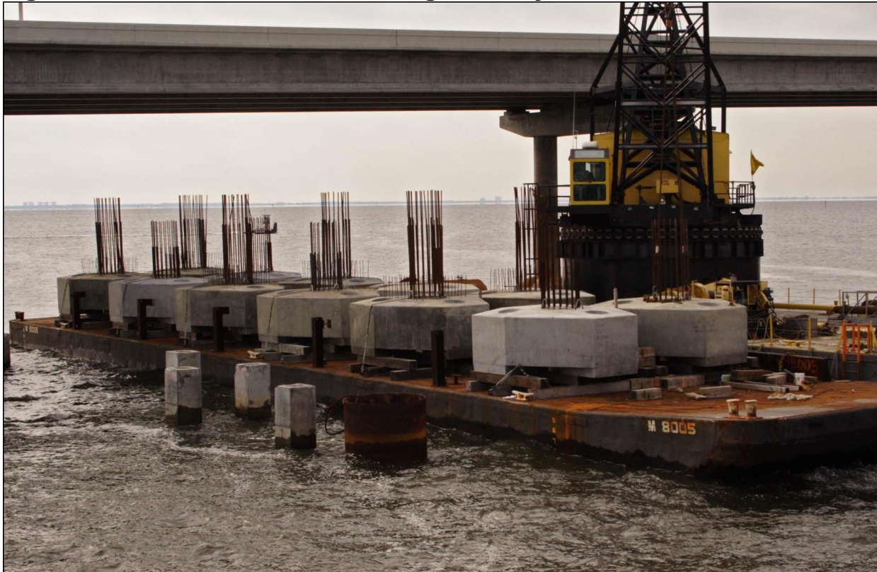
Figure 25.4.3.6-3 Precast Footing Installation
