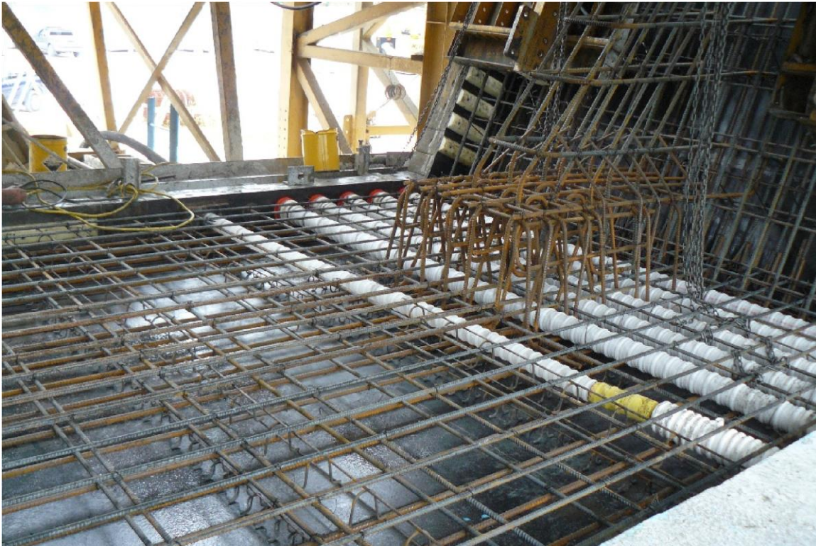
Figure 20.4-1 Reinforcing in Deviation Segment
