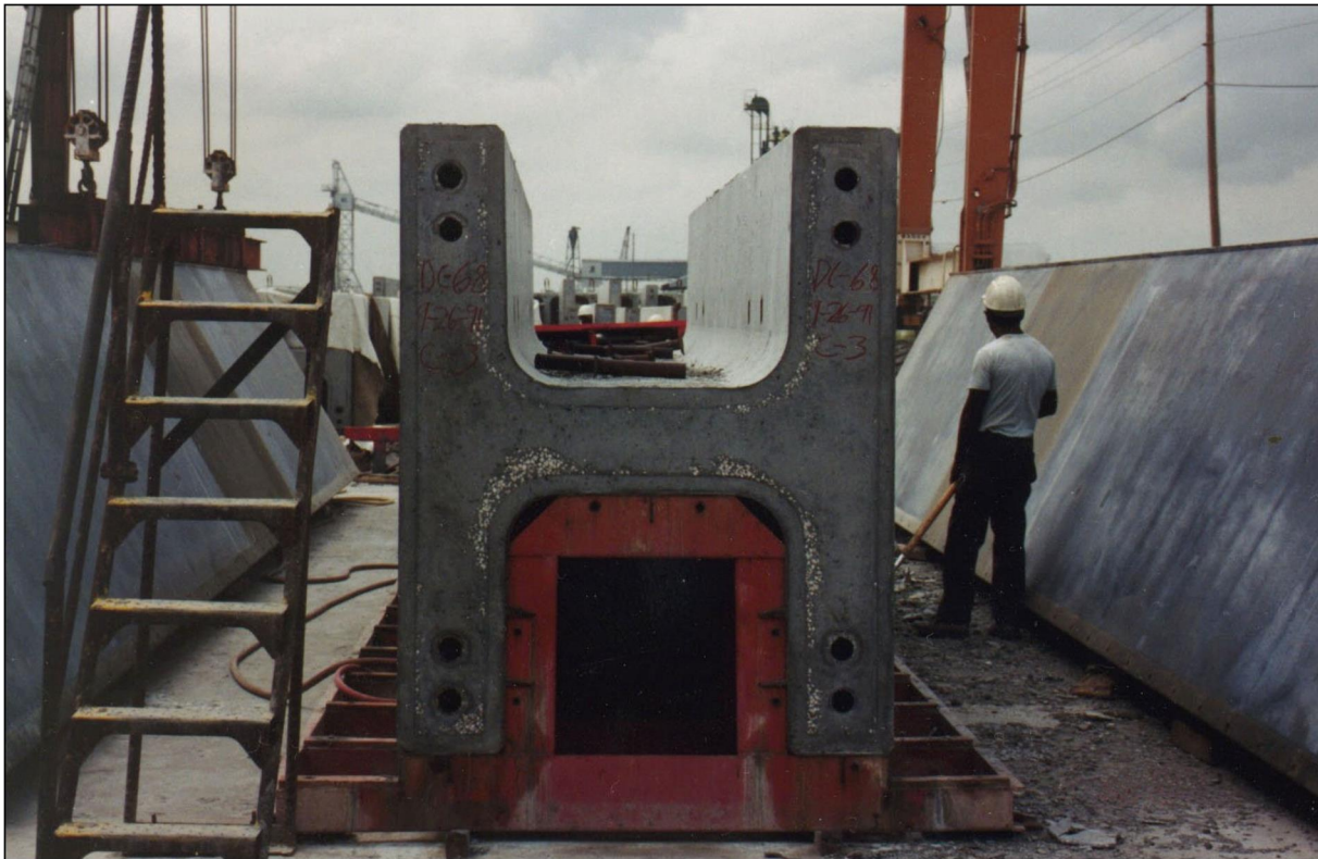
Figure 25.4.3.2-3 C.I.P. Foundation and Precast H-Section Pier Column
