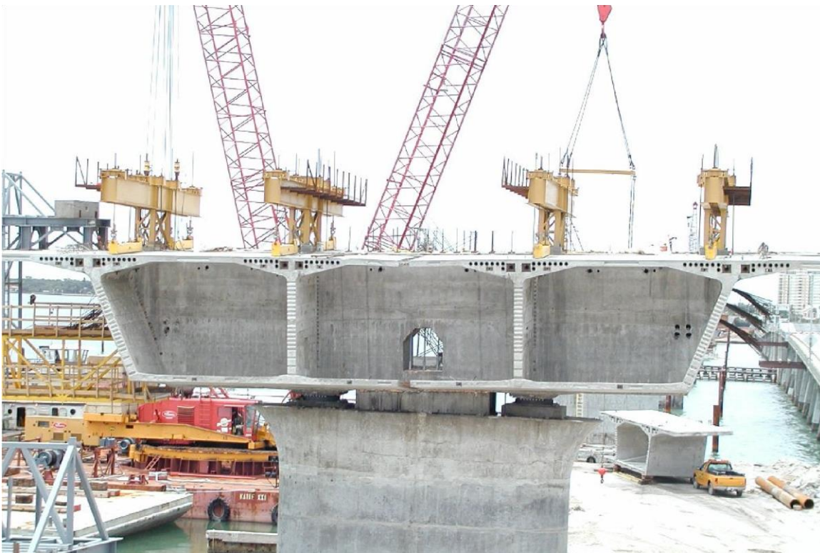
Figure 20.9.1-3 Setting Geometry with Strongbacks
