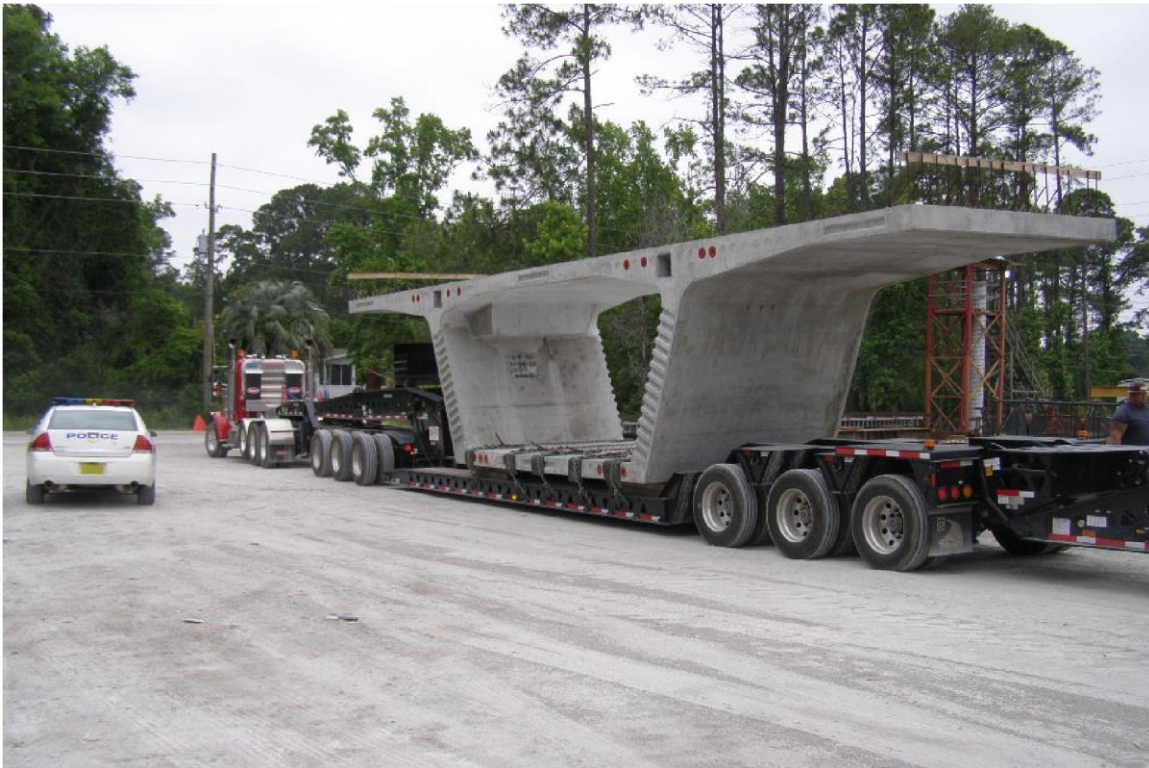
Figure 20.9.2-5 Truck Loaded with Segment
