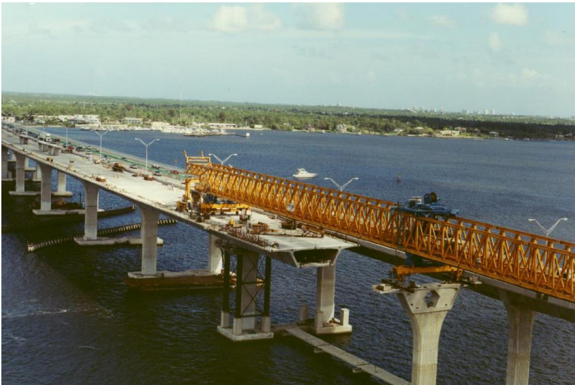
Figure 20.9.1-5 Gantry with Leg on Pier Segment
