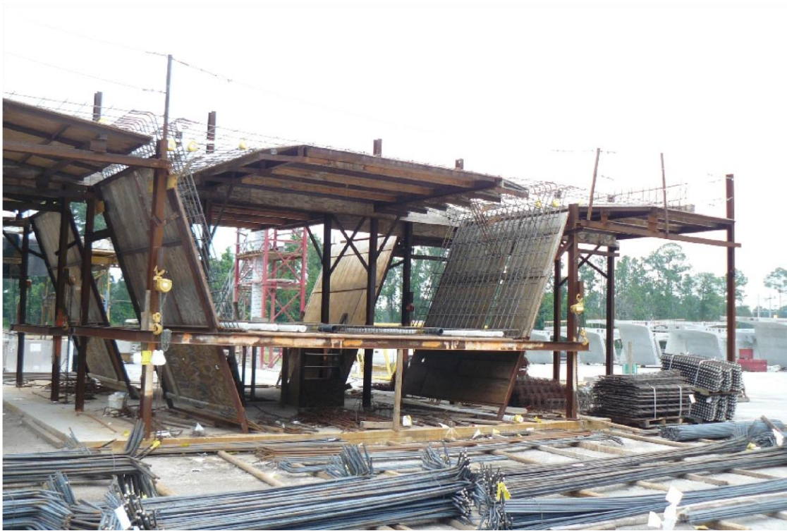
Figure 20.1-1 Reinforcing Jig for Variable Depth Segment
