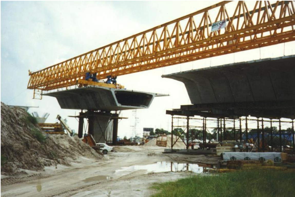
Figure 20.9.1-4 Gantry and Stabilization Towers
