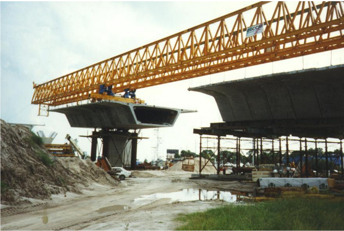
Figure 20.9.1-4 Gantry and Stabilization Towers
