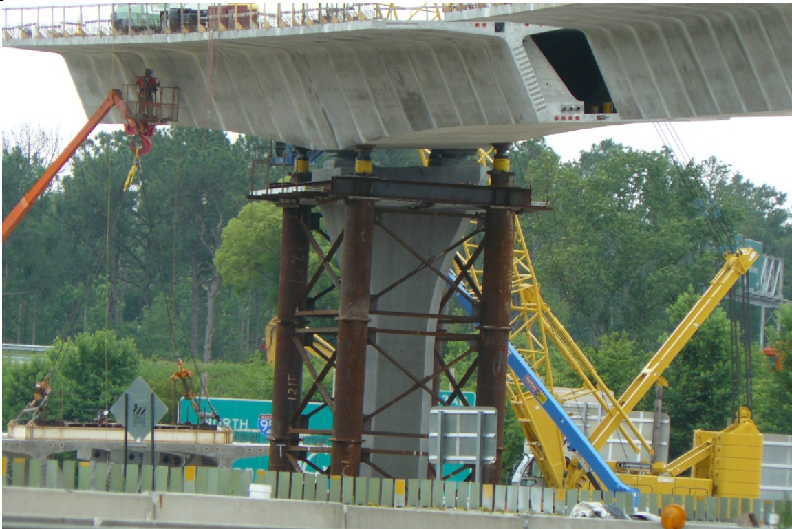
Figure 20.9.1-2 Stabilization of Balanced Cantilever
