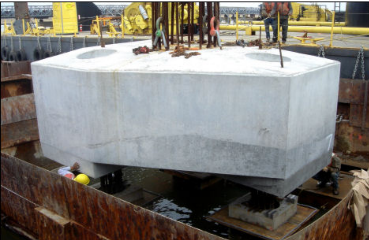
Figure 25.4.3.6-3 Precast Footing Installation
