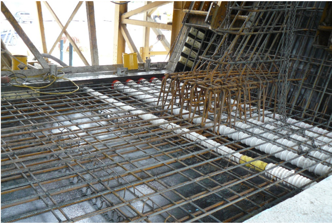
Figure 20.4-1 Reinforcing in Deviation Segment
