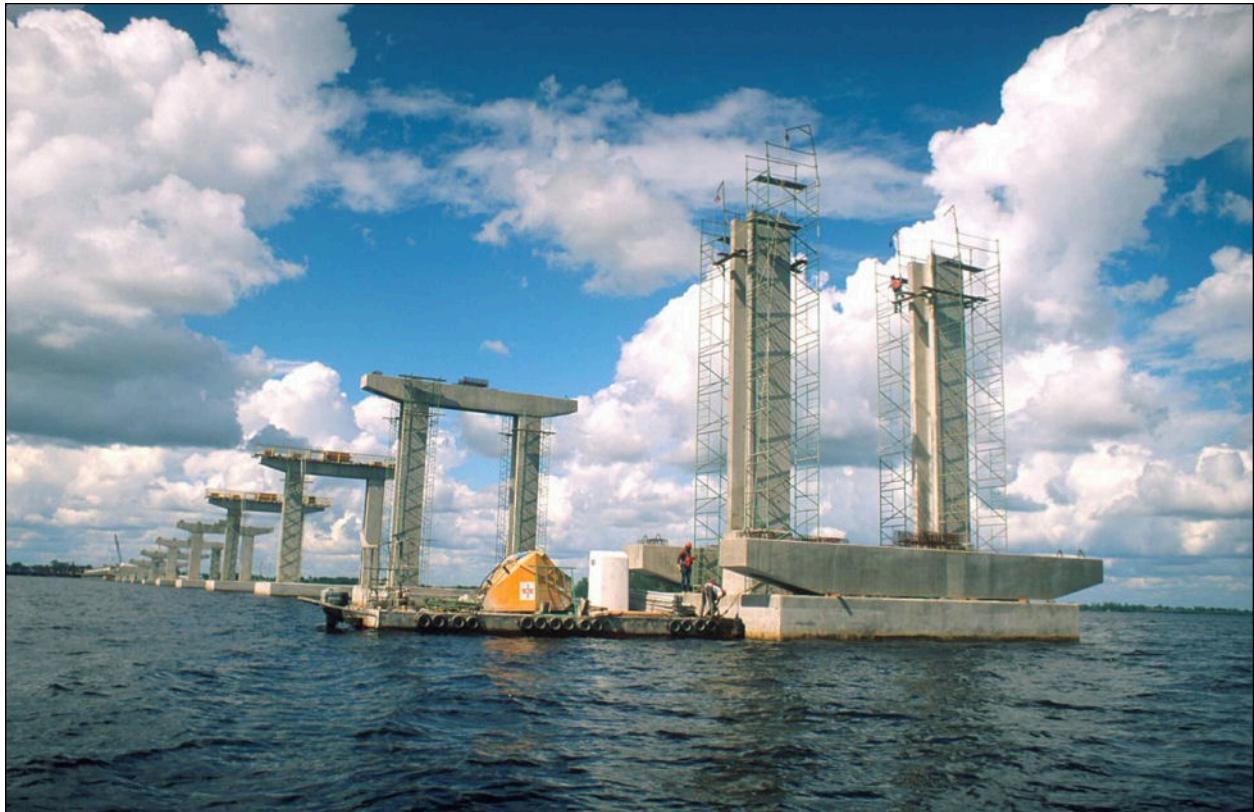
Figure 25.4.3.3-1 Precast Pier Cap Installation
