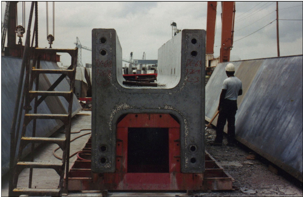
Figure 25.4.3.2-3 C.I.P. Foundation and Precast H-Section Pier Column
