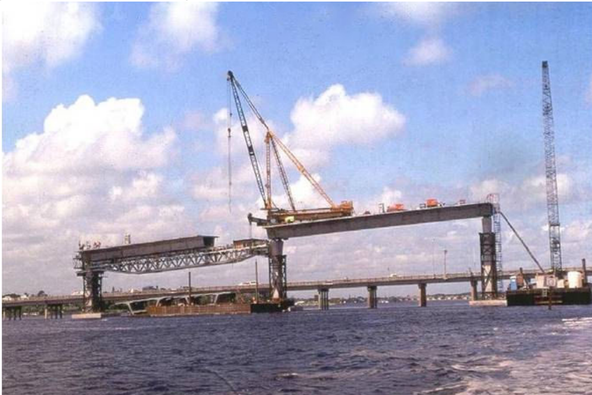
Figure 20.9.2-1 Span by Span Construction
