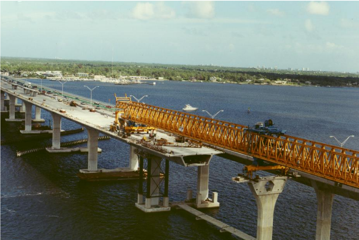
Figure 20.9.1-5 Gantry with Leg on Pier Segment
