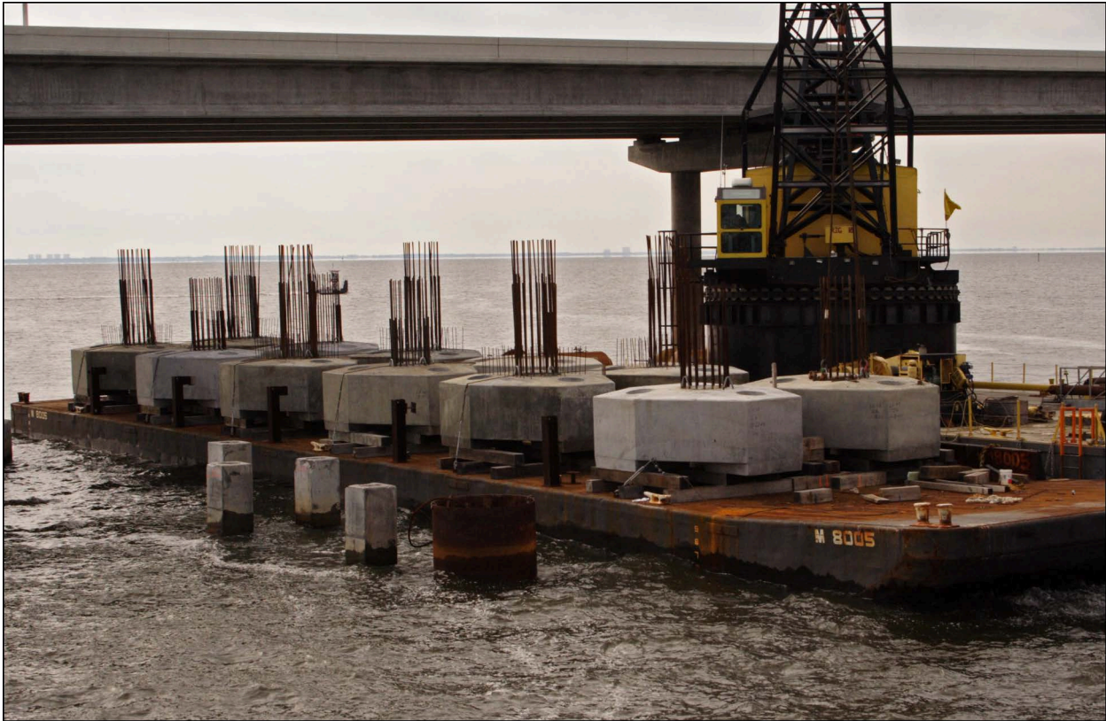
Figure 25.4.3.6-3 Precast Footing Installation
