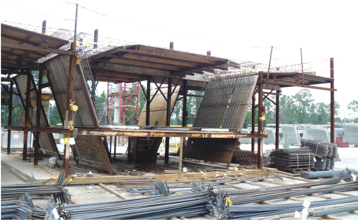
Figure 20.1-1 Reinforcing Jig for Variable Depth Segment
