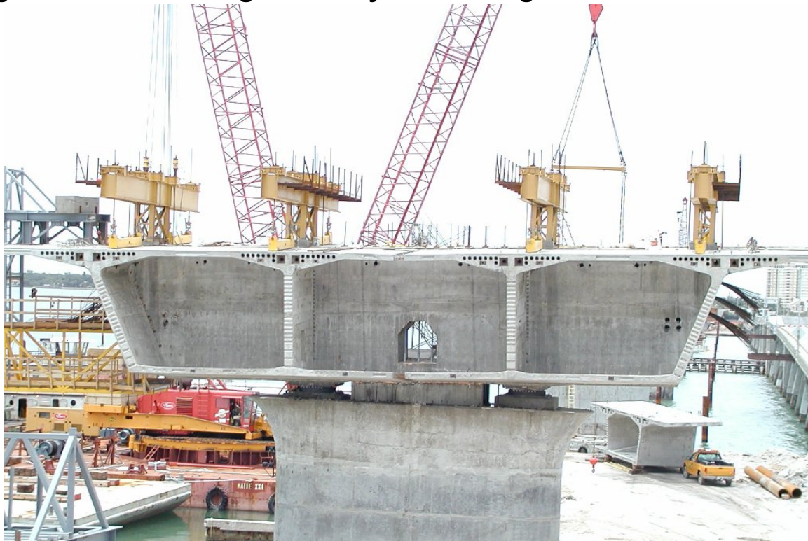
Figure 20.9.1-3 Setting Geometry with Strongbacks
