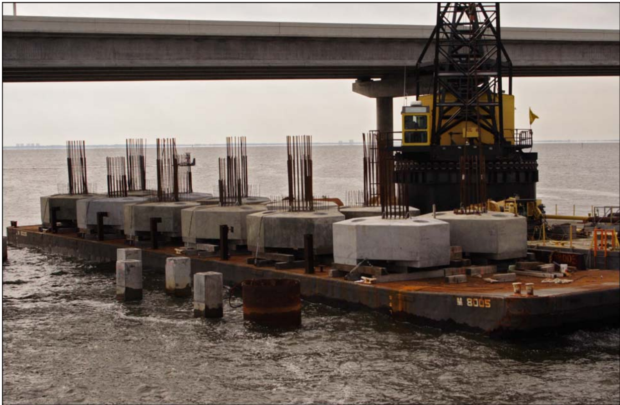
Figure 25.4.3.6-3 Precast Footing Installation
