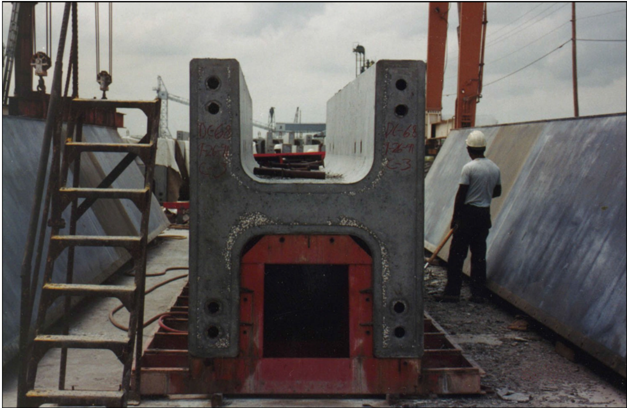
Figure 25.4.3.2-3 C.I.P. Foundation and Precast H-Section Pier Column
