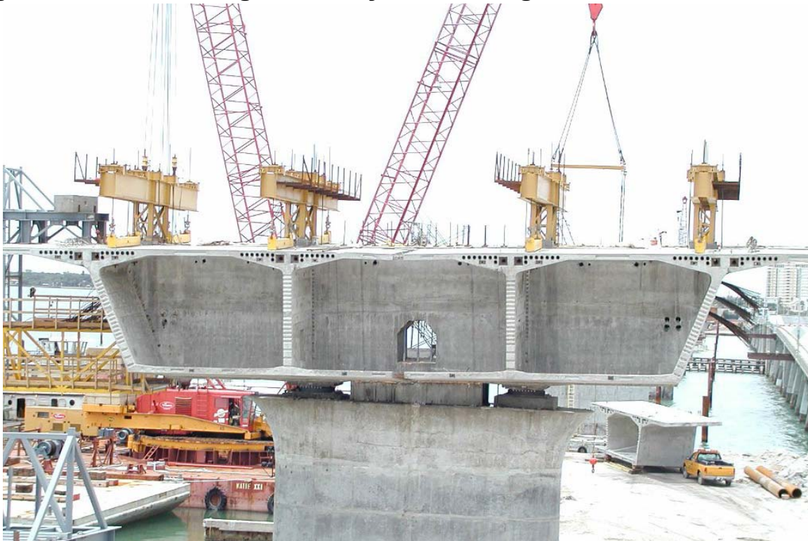
Figure 20.9.1-3 Setting Geometry with Strongbacks
