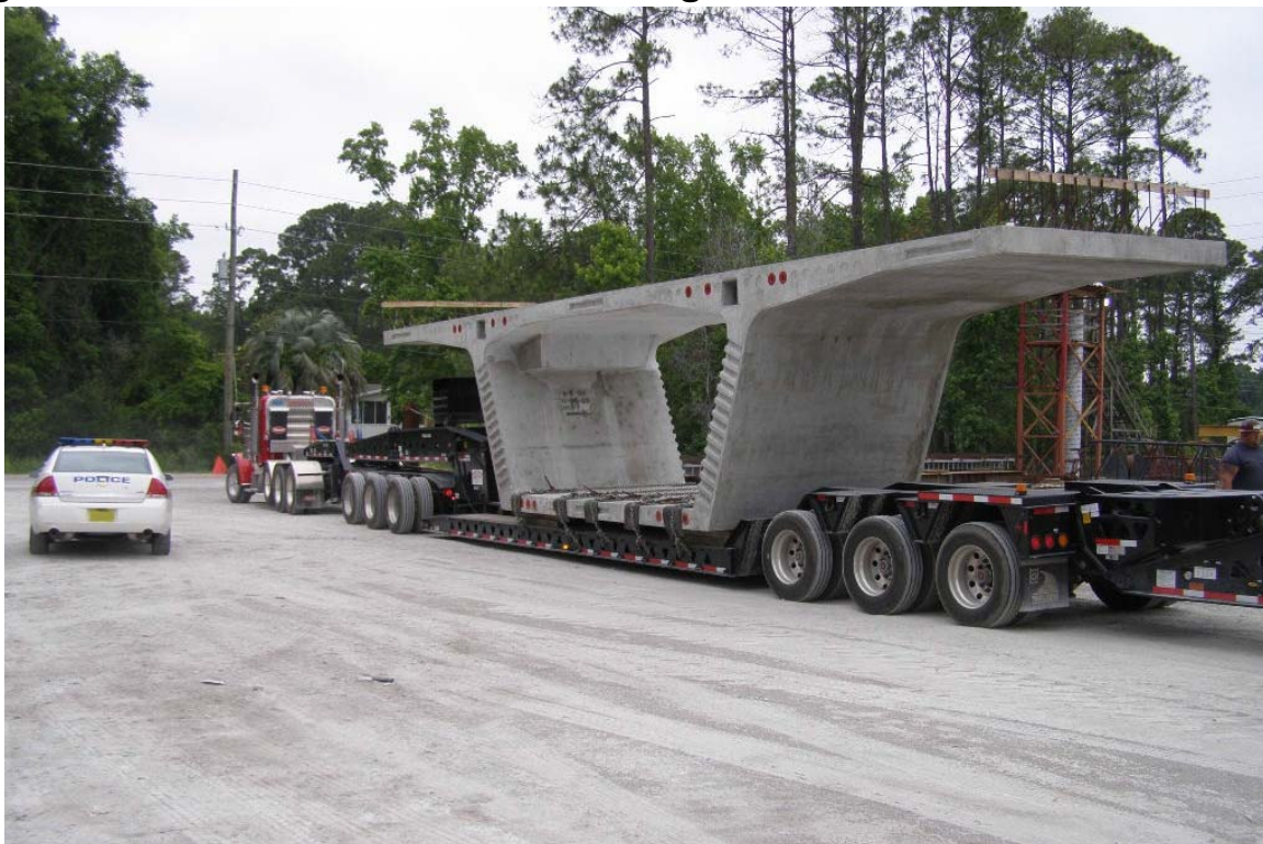
Figure 20.9.2-5 Truck Loaded with Segment
