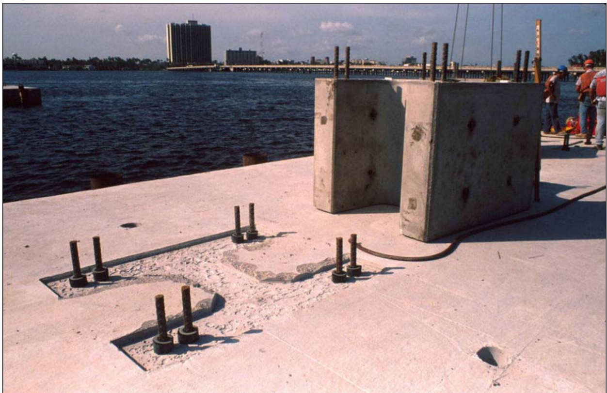
Figure 25.4.3.2-3 C.I.P. Foundation and Precast H-Section Pier Column
