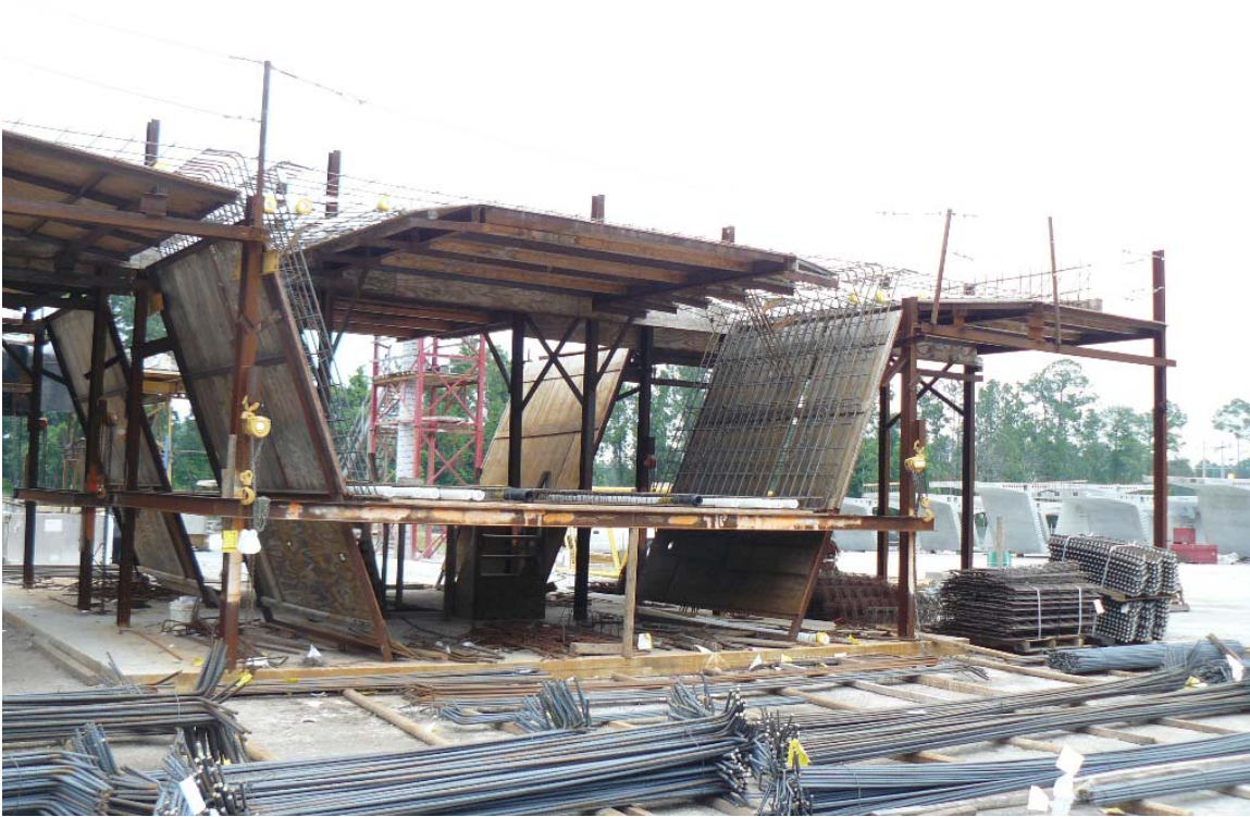
Figure 20.1-1 Reinforcing Jig for Variable Depth Segment
