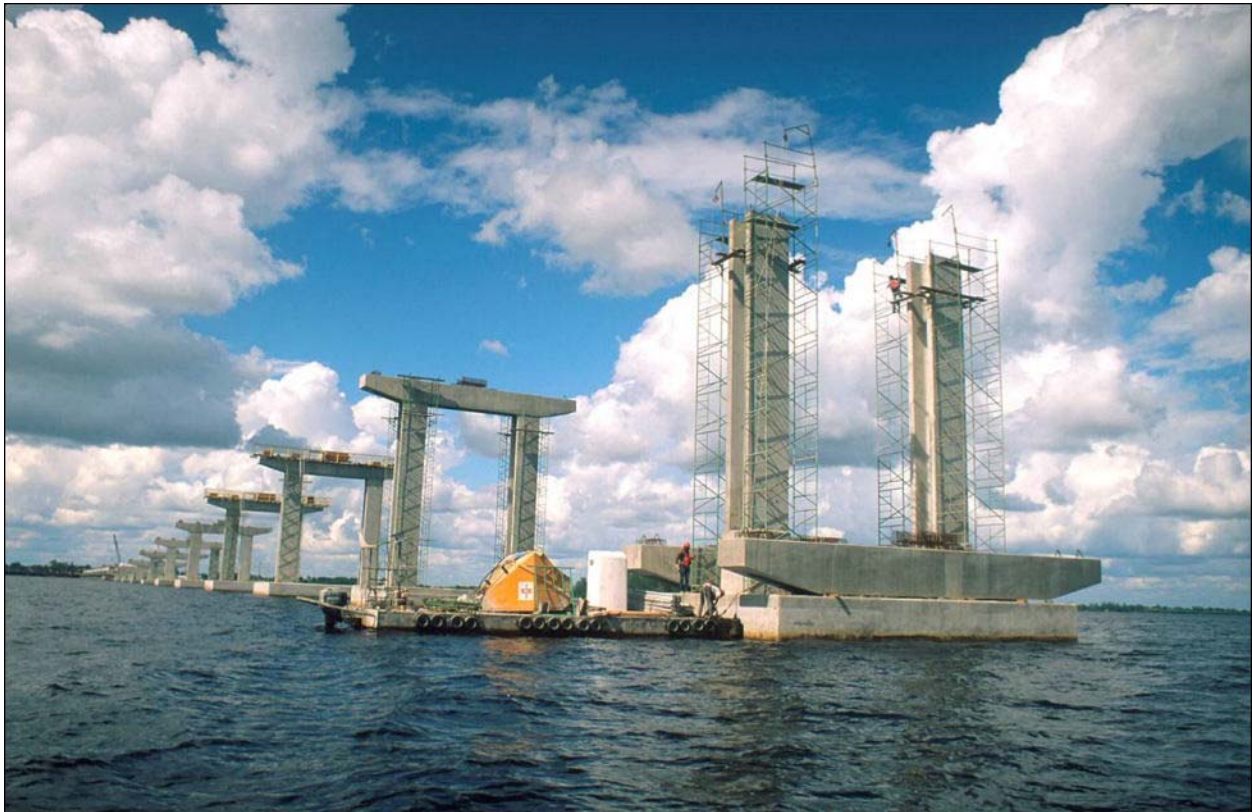
Figure 25.4.3.3-1 Precast Pier Cap Installation
