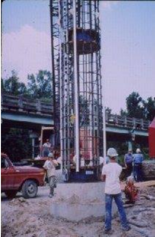
Figure 38, Osterberg Load Cells
