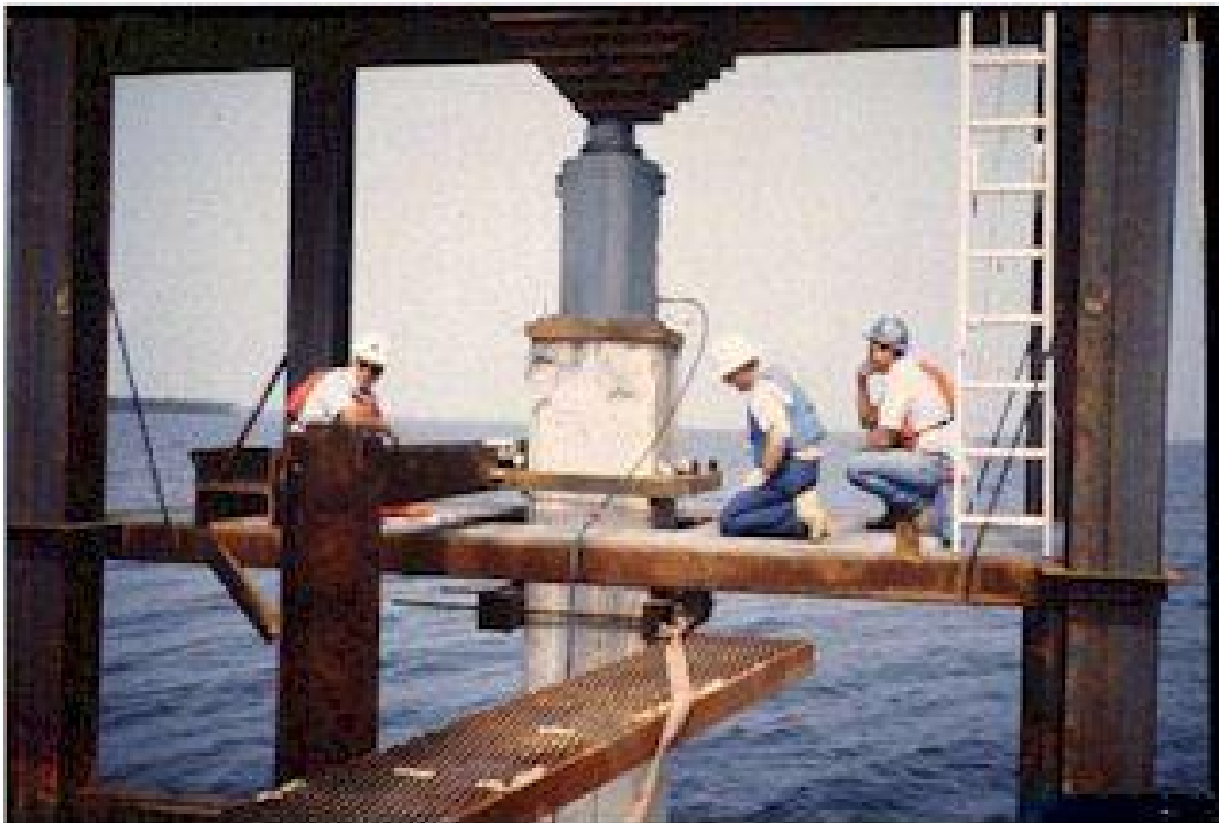
Figure 35, Static Load Test
