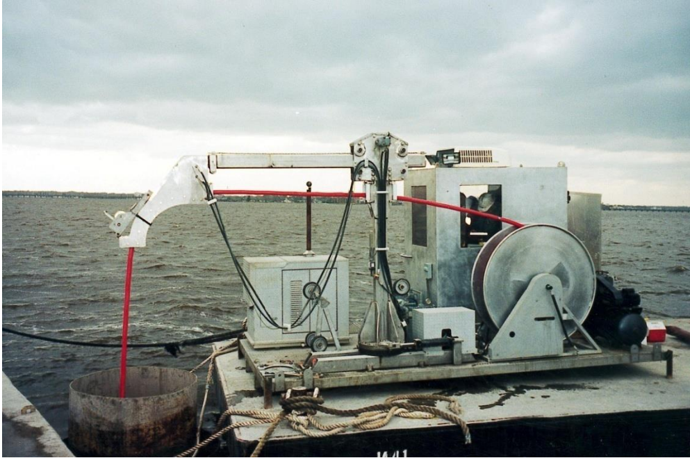
Figure 40, Shaft Inspection Device
