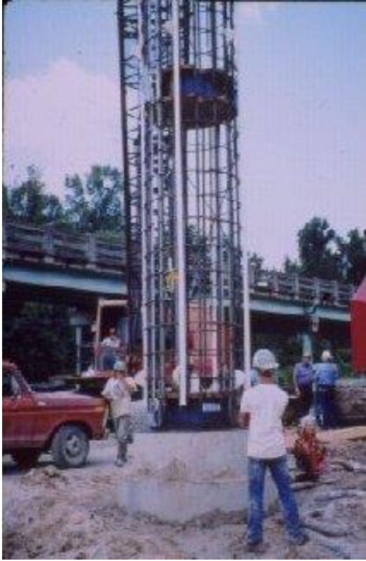
Figure 38, Osterberg Load Cells
