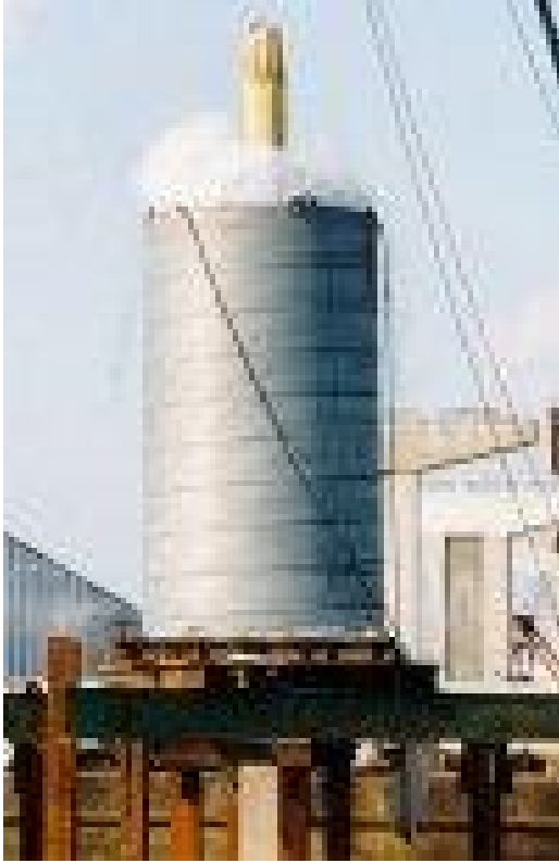
Figure 36, Axial Statnamic Load Test
