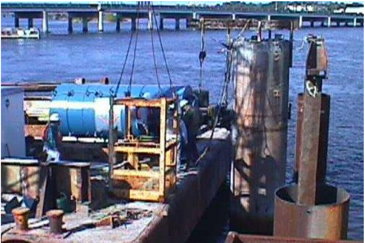
Figure 37, Lateral Statnamic Load Test
