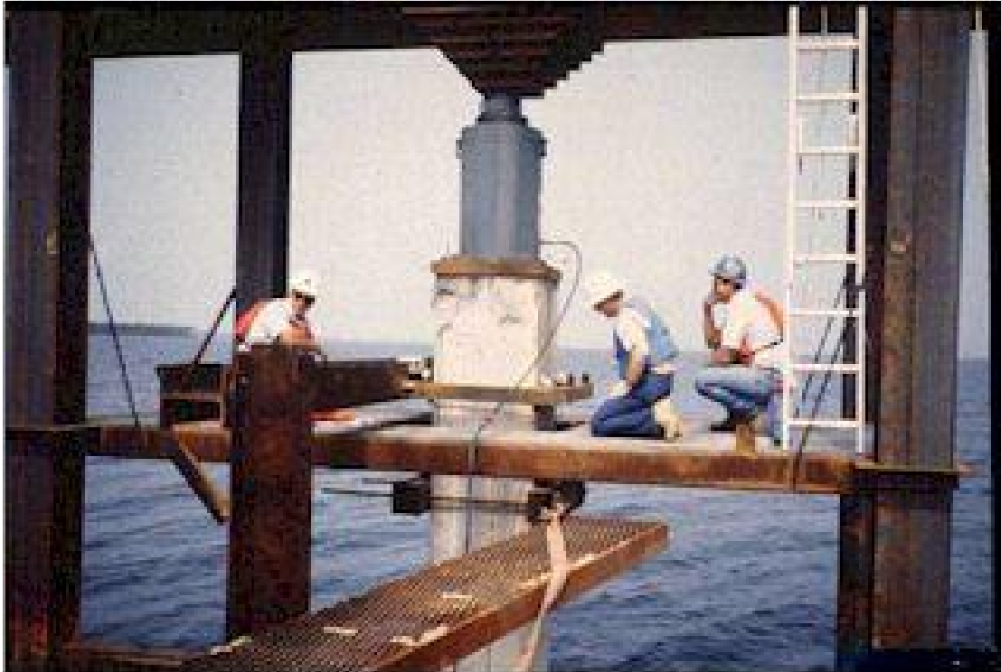
Figure 35, Static Load Test
