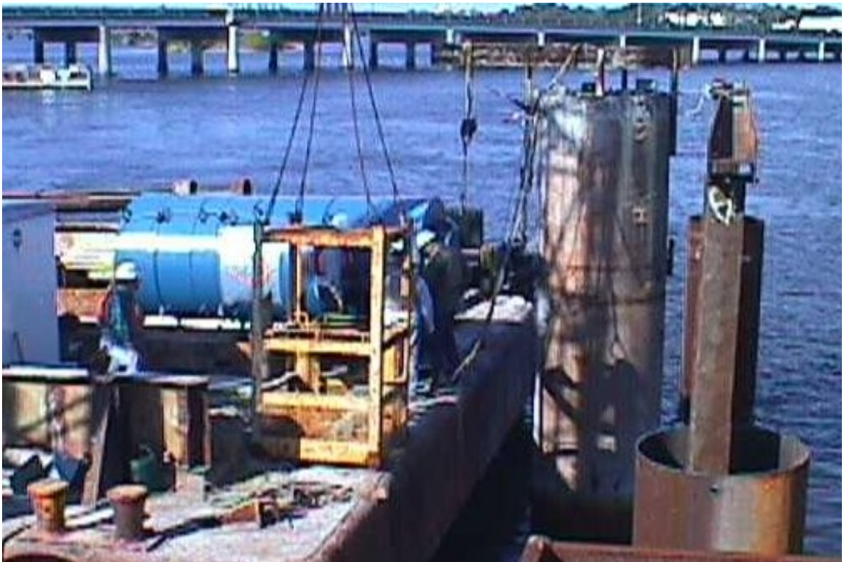
Figure 37, Lateral Statnamic Load Test
