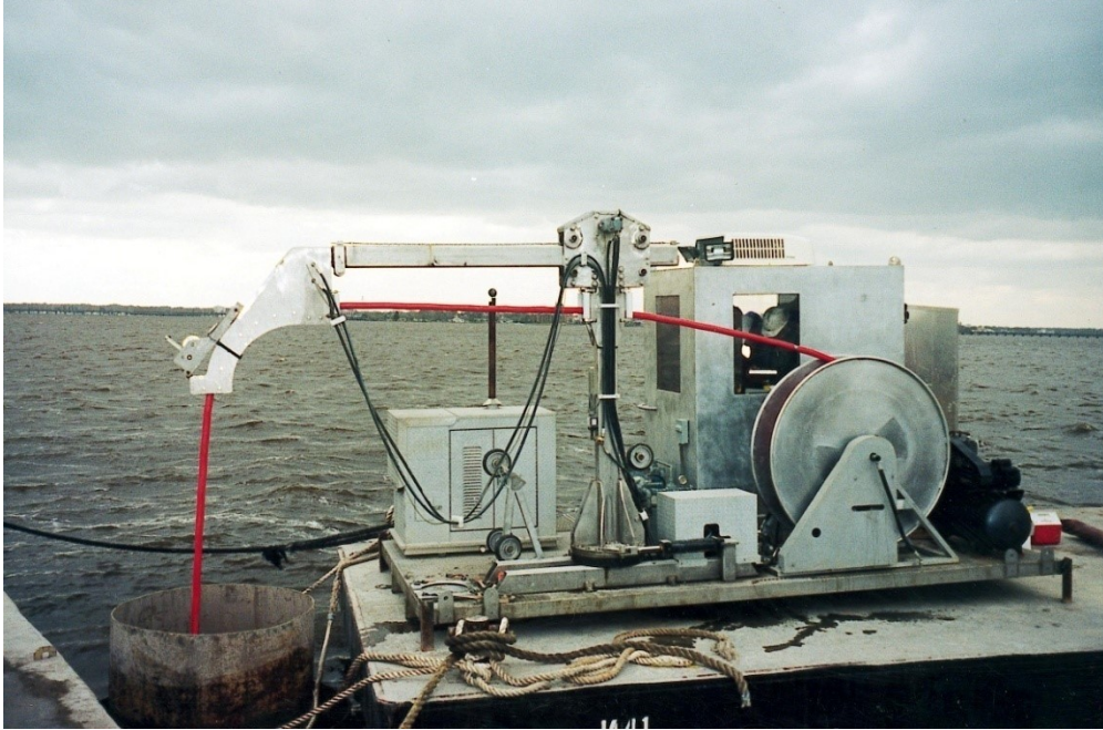
Figure 40, Shaft Inspection Device
