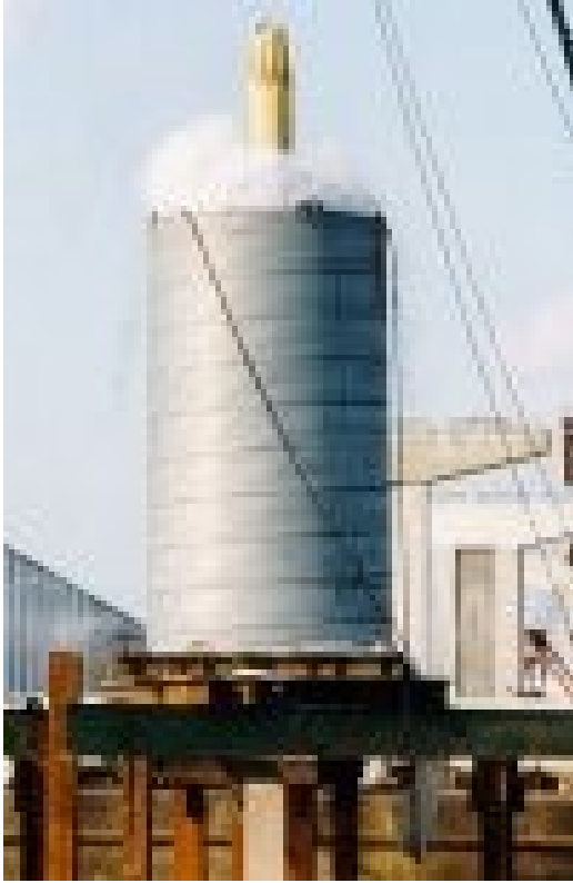
Figure 36, Axial Statnamic Load Test
