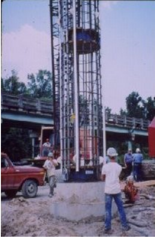
Figure 38, Osterberg Load Cells
