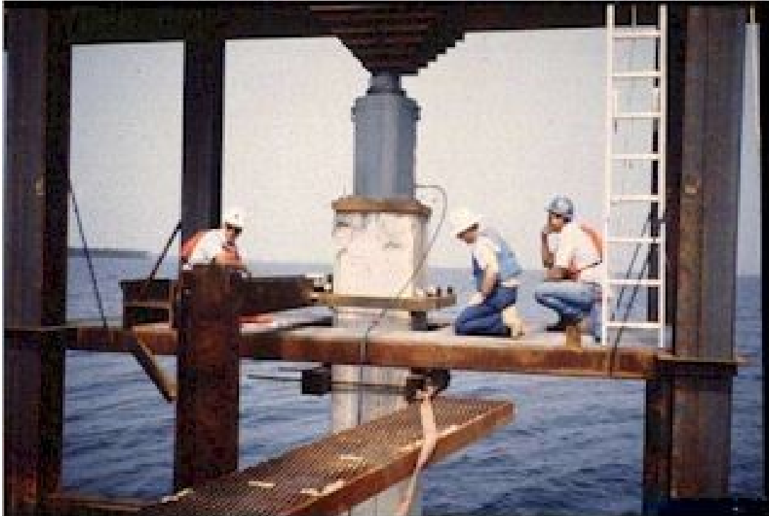
Figure 35, Static Load Test
