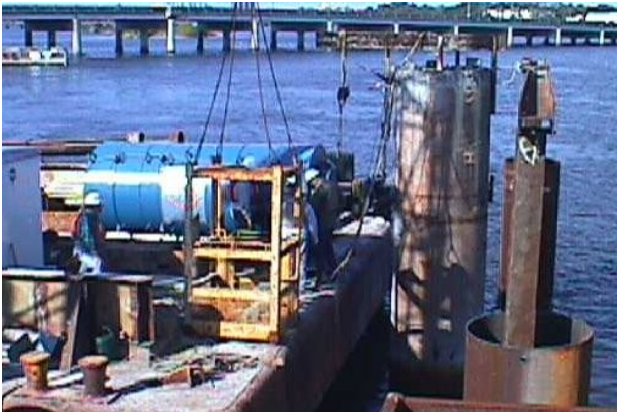
Figure 37, Lateral Static Load Test
