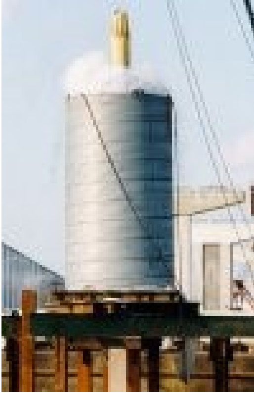
Figure 36, Axial Static Load Test
