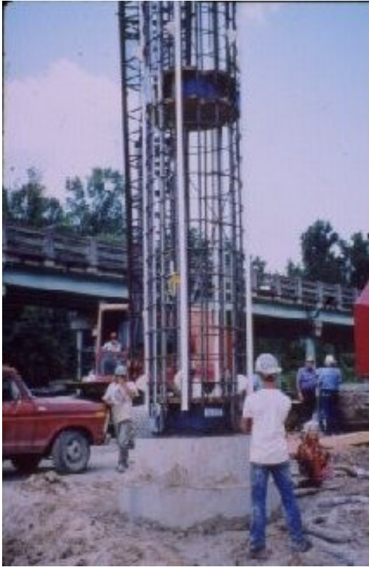
Figure 38, Osterberg Load Cells
