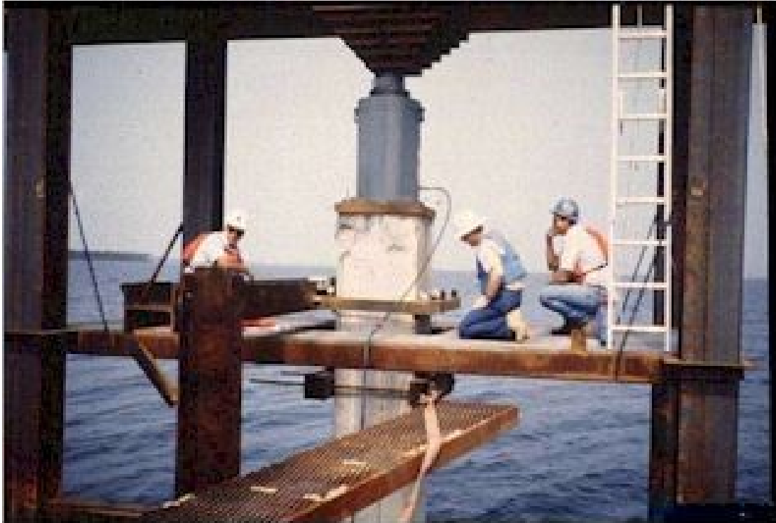
Figure 35, Static Load Test
