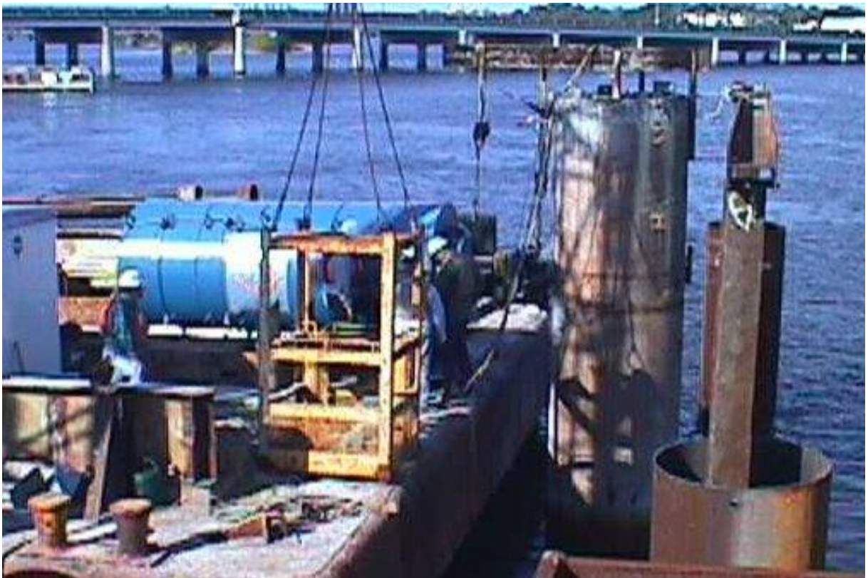
Figure 38, Lateral Static Load Test
