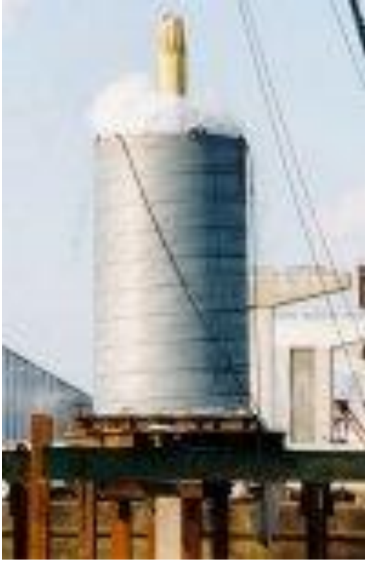
Figure 37, Axial Statnamic Load Test
