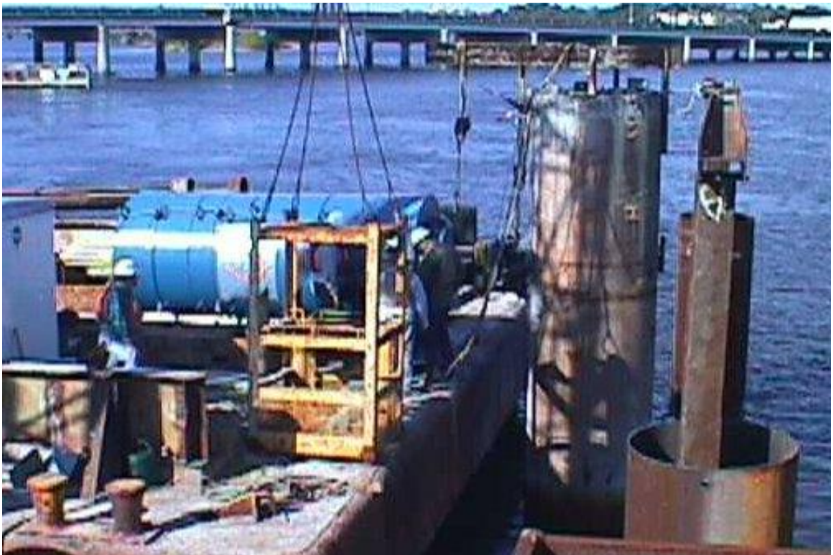
Figure 38, Lateral Statnamic Load Test
