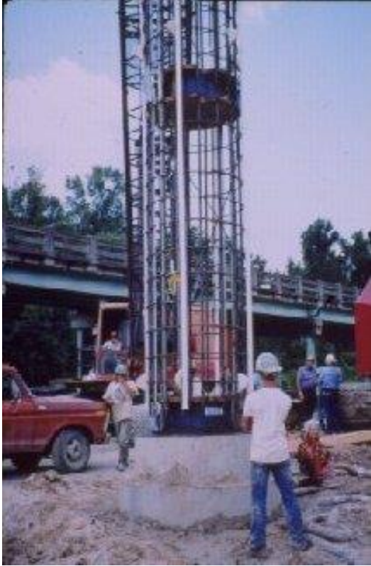
Figure 39, Osterberg Load Cells
