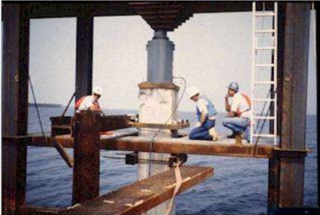
Figure 36, Static Load Test
