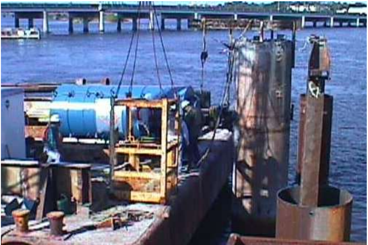
Figure 40, Lateral Static Load Test
