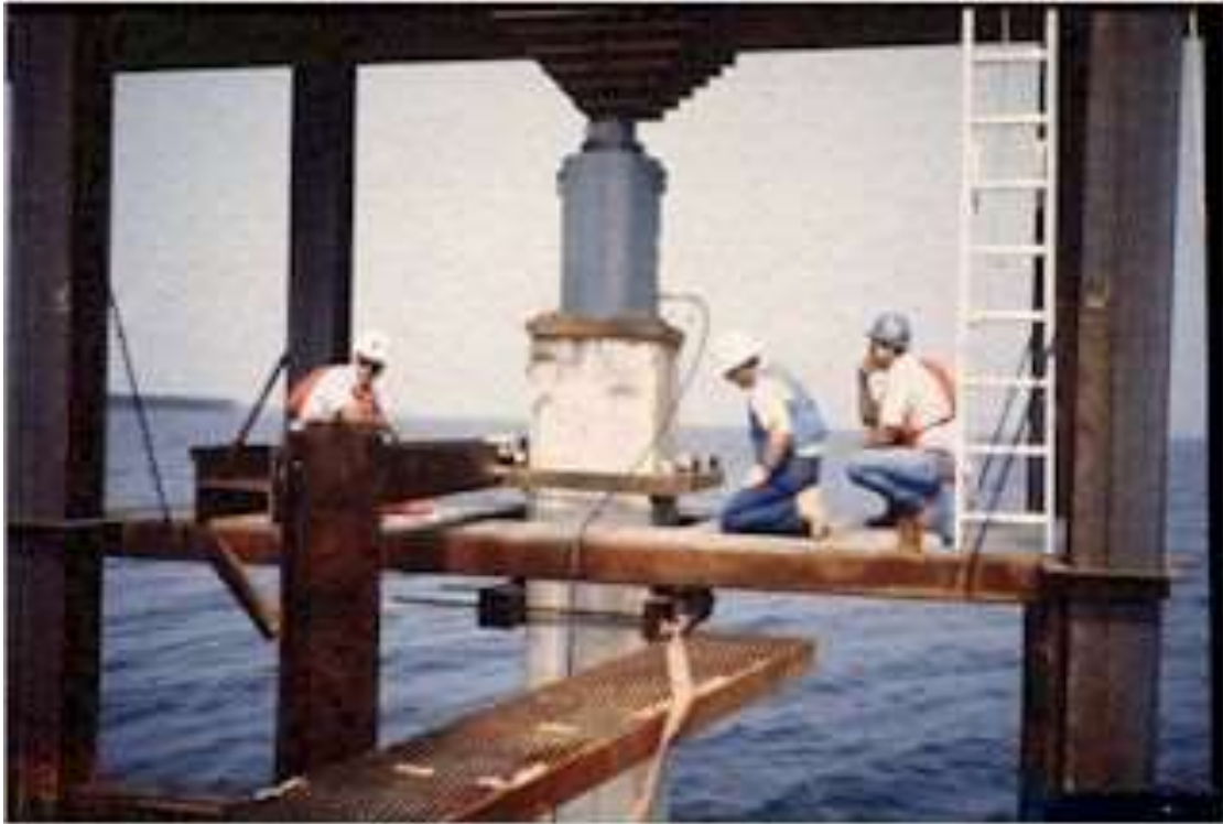
Figure 38, Static Load Test
