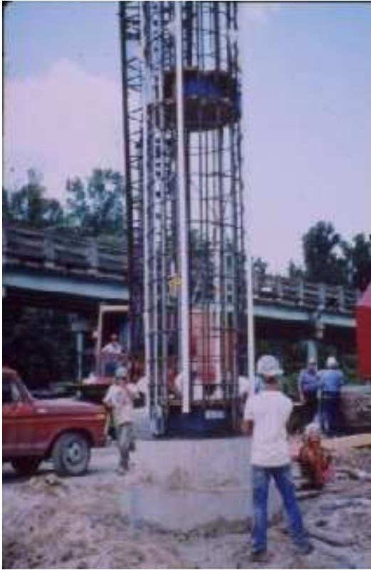
Figure 41, Osterberg Load Cells
