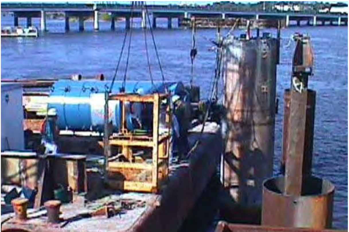
Figure 40, Lateral Statnamic Load Test
