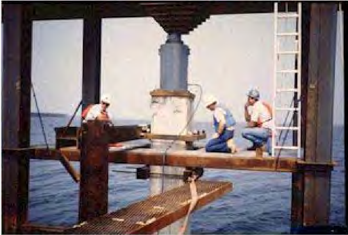
Figure 38, Static Load Test
