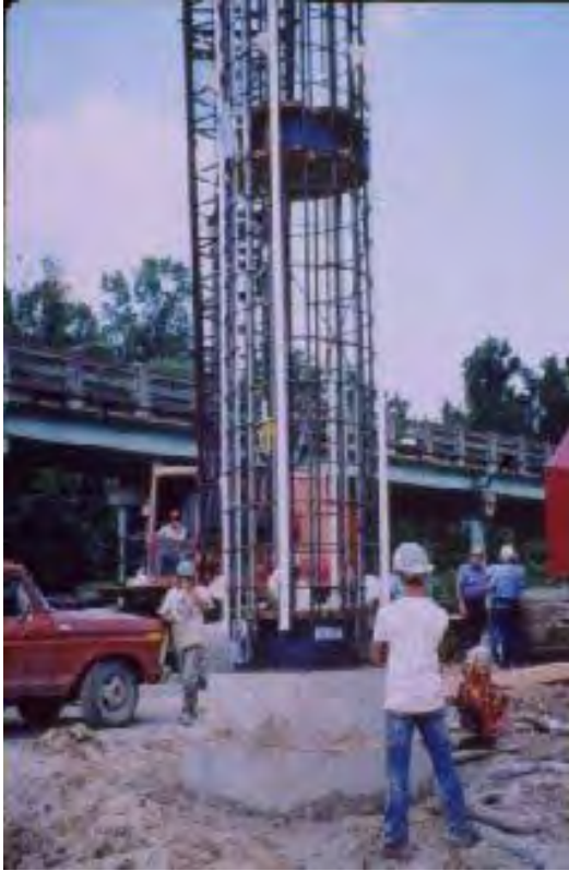
Figure 41, Osterberg Load Cells
