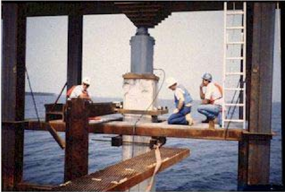
Figure 38, Static Load Test
