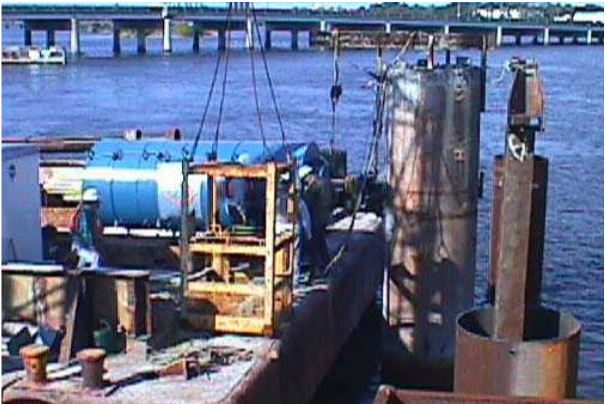
Figure 40, Lateral Statnamic Load Test
