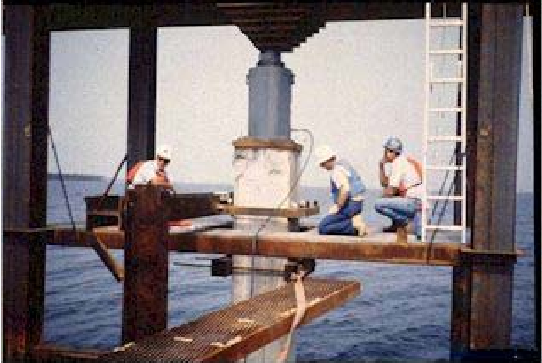
Figure 38, Static Load Test
