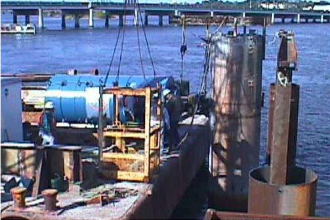
**Figure 37, Lateral Static Load Test**
