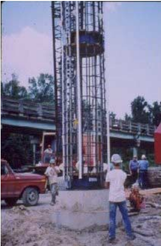
Figure 38, Osterberg Load Cells
