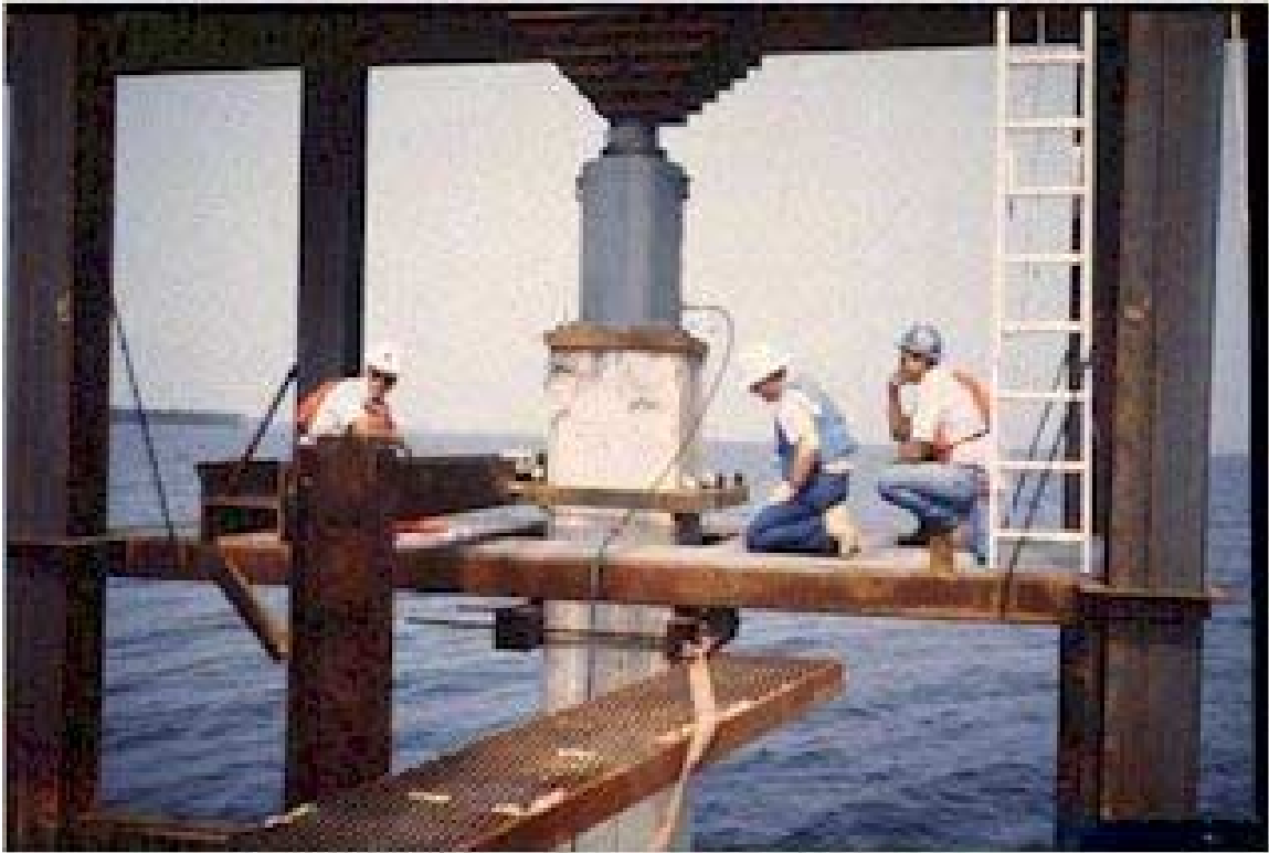
Figure 35, Static Load Test
