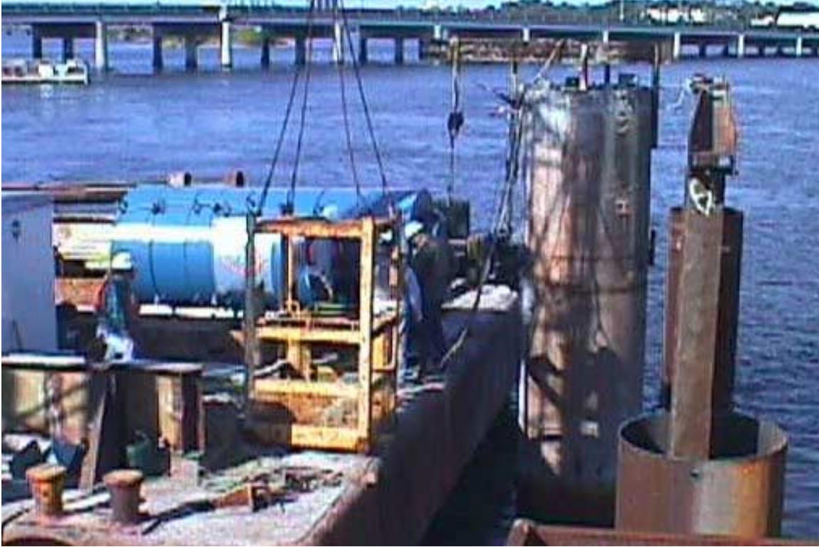
Figure 37, Lateral Static Load Test
