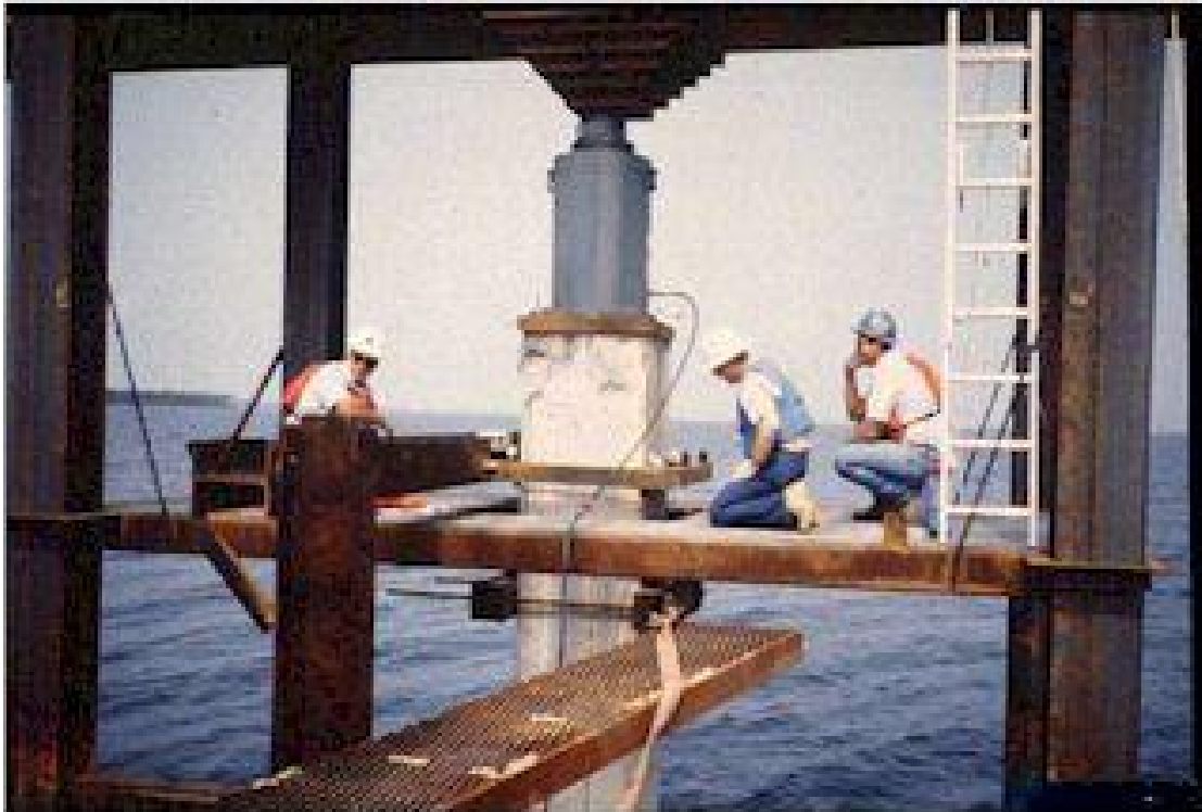
Figure 35, Static Load Test
