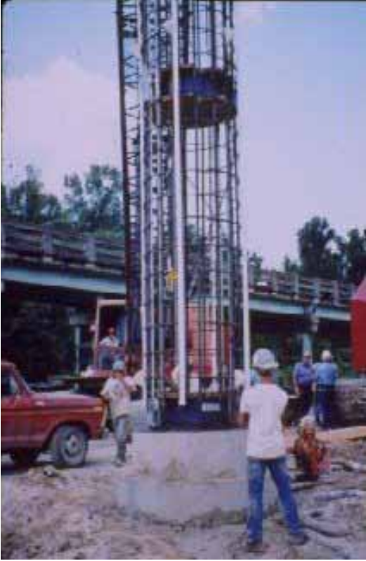
Figure 41, Osterberg Load Cells
