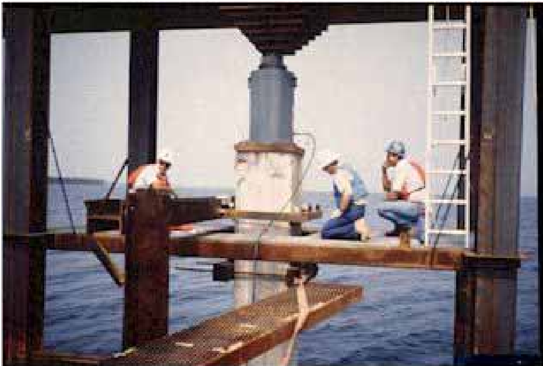
Figure 38, Static Load Test
