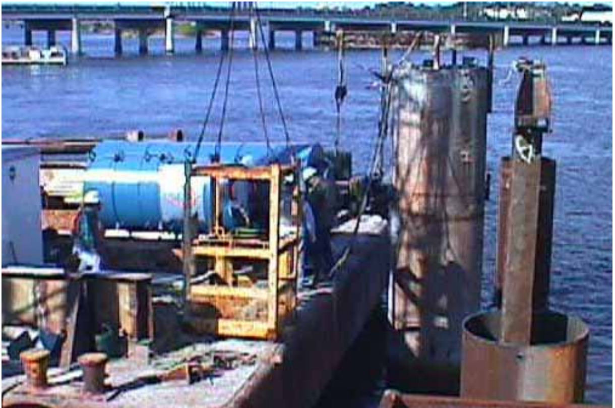
Figure 40, Lateral Statnamic Load Test
