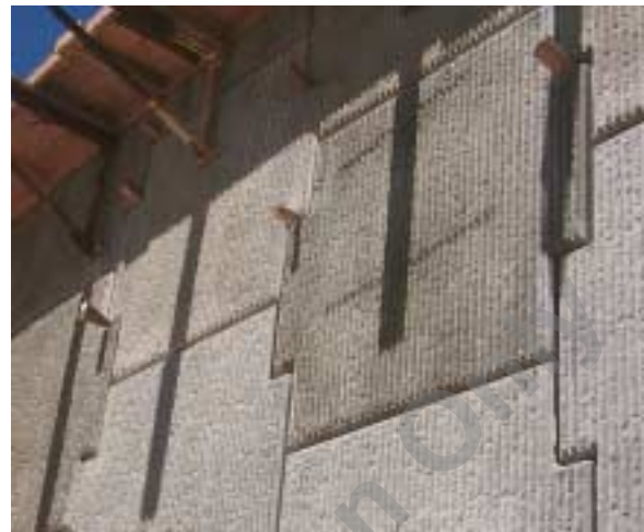
Figure 44, Wooden Wedges
