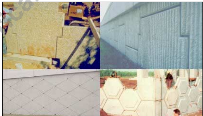
Figure 4, Some Panel Finishes and Shapes
