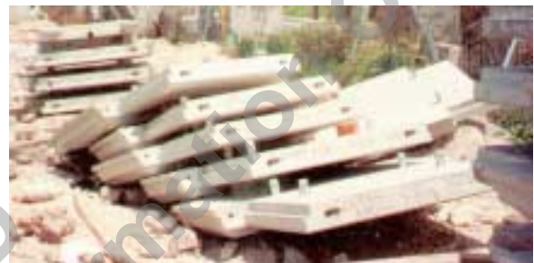
Figure 10, Improper Panel Storage
