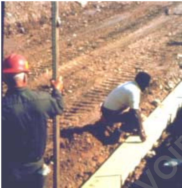
Figure 3, Leveling Pad
