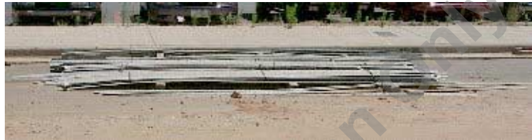
Figure 15, Reinforcement Storage
