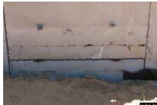
Figure 35. Attach Filter Fabric
