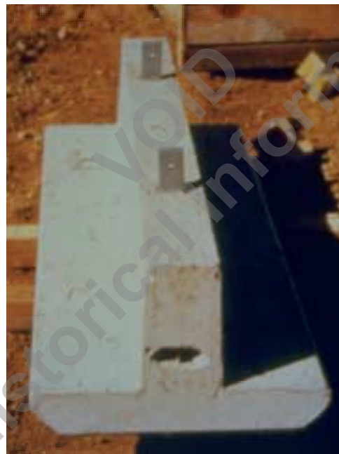
Figure 6, Slip Joint
