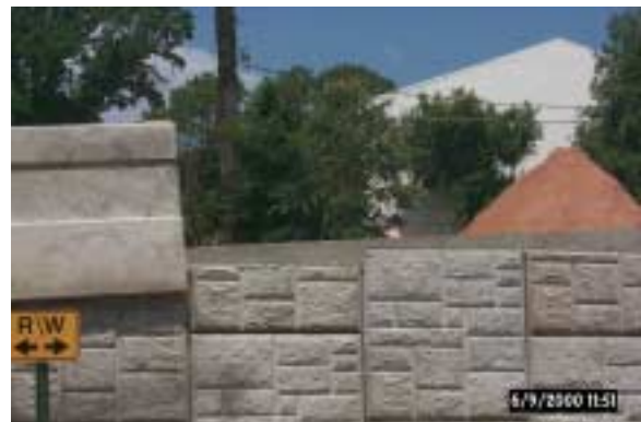
Figure 16, Leveling Course for Coping/Barrier
