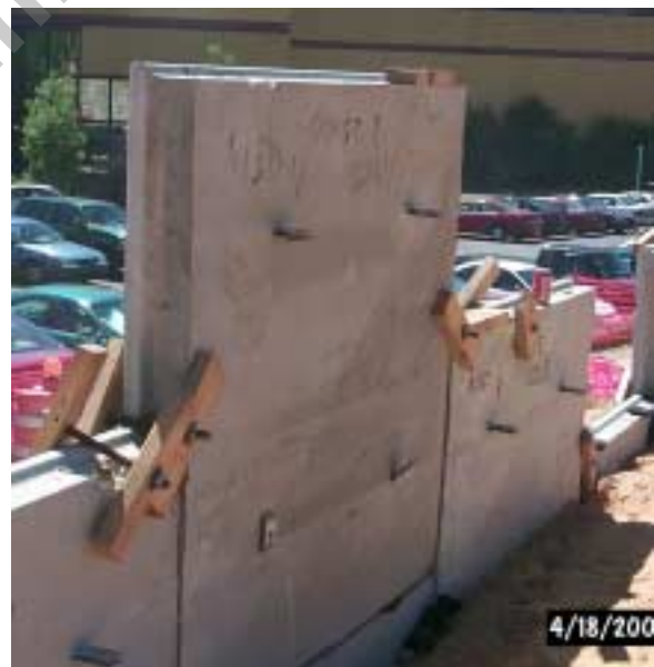
Figure 11, Damaged Tabs
