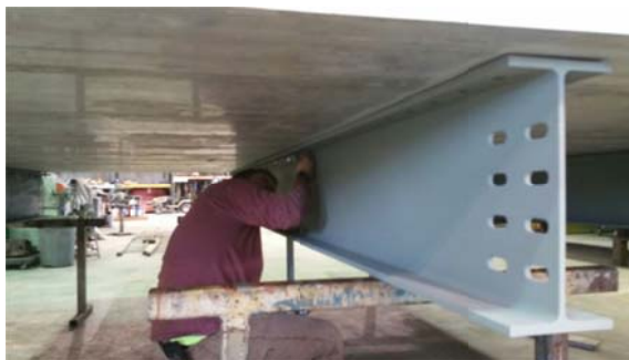
Figure 20 – Bolt Installation
