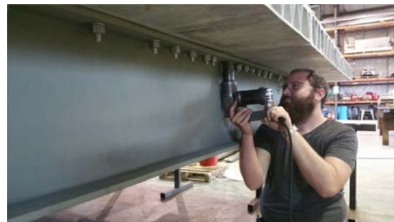
Figure 21 – TC Bolt Tightening
