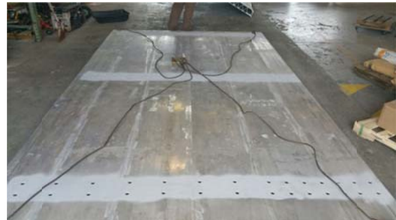
Figure 19 – Sand Blasting Panel Bottom
