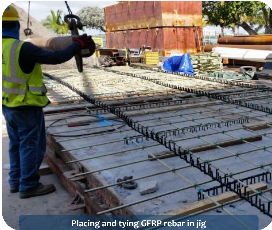
Hoisting GFRP rebar mat for placement in form
