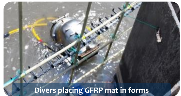
Hoisting GFRP rebar mat for placement in form
