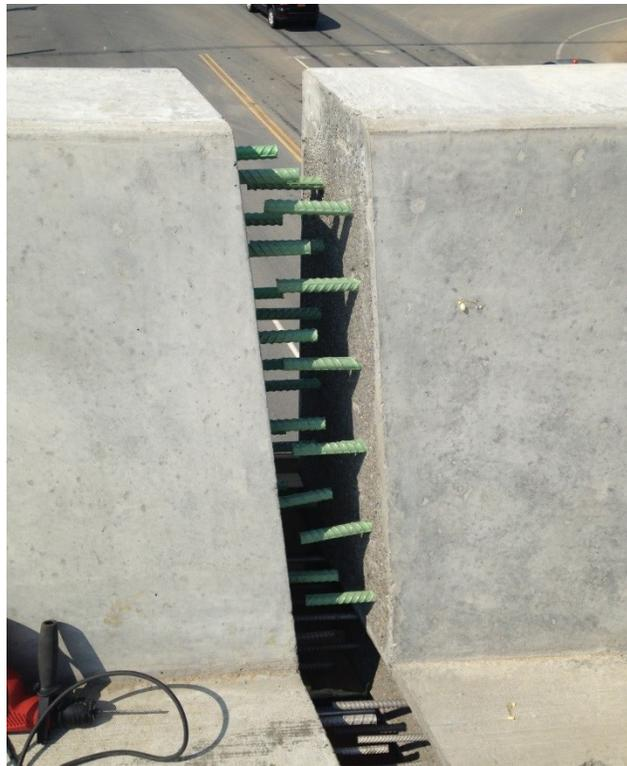
**Figure 135. Photo. Example of interlaced reinforcement in a UHPC connection.**
