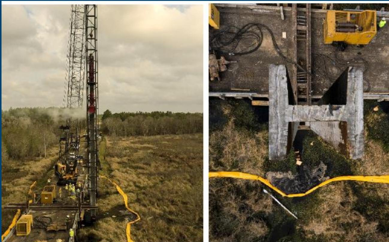
Pile driving photos courtesy of Cor-Tuf UHPC
