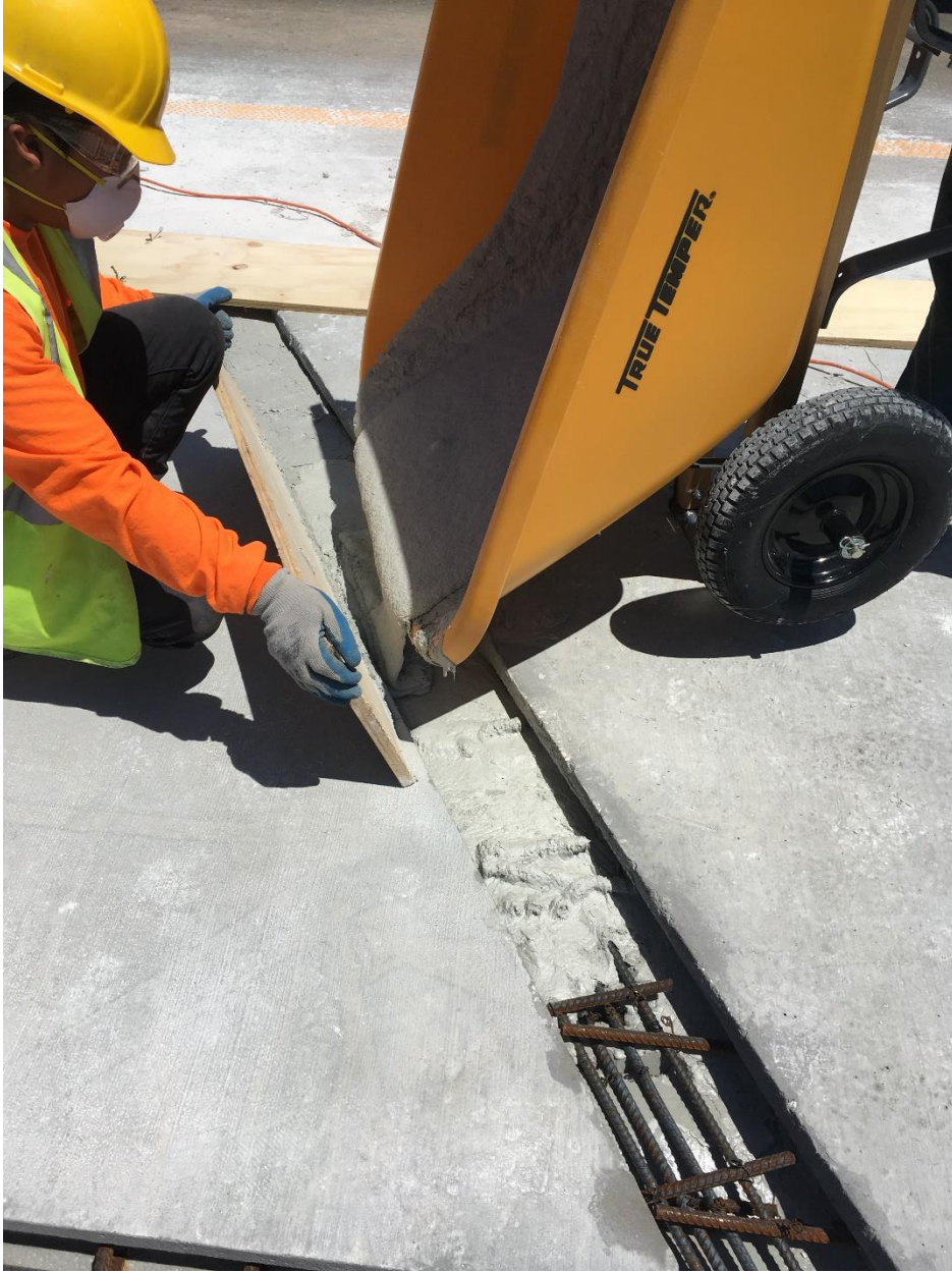
Figure 2-13: Wheelbarrow placing of UHPC in joints
