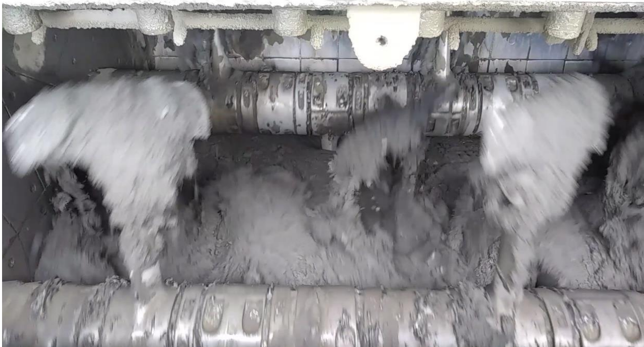
Figure 2-12: Double-shaft mixer with UHPC Placing & Finishing
