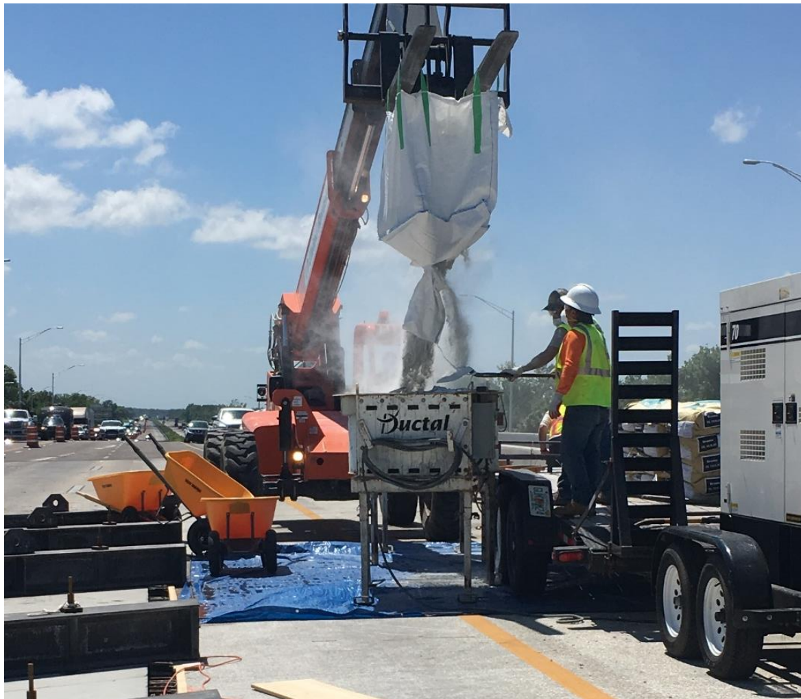
Figure 2-10: Dust is created as premix is added to mixer
